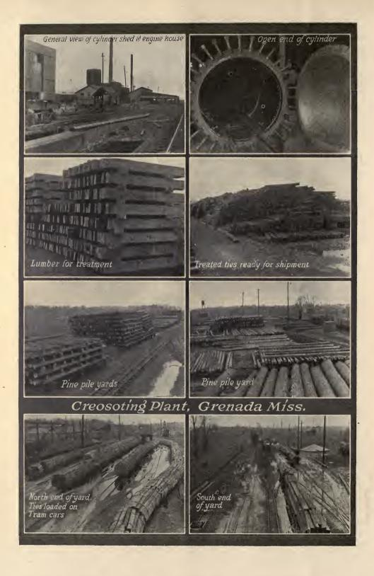
which the trucks are operated in the timber and tie yard. These trucks loaded with the material to be treated are run into the cylinders by means of a snatch block in the far end of the cylinder through which is passed a wire rope. The wire rope as well as the trucks are, of course, in the cylinder during the full treatment.
