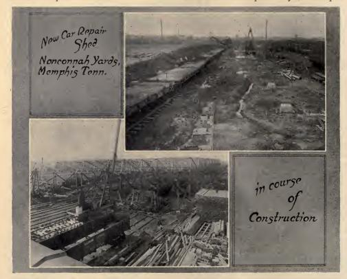
The excavation for the concrete piers supporting the columns was done by hand. The concrete mixing plant was located adjacent to the building and the concrete wheeled to the individual piers. There were one hundred and ninety-five piers which required four hundred and seventy-eight cubic yards of concrete.
