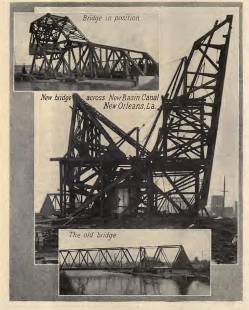
count of crossing the canal at an angle, the clear opening for boats is only 60 ft. The moving leaf operates by rotating about the main trunnion pin directly over the pier. One of the accompanying pictures shows the completed bridge closed for the passage of trains, and another shows the bridge open during the erection. It was necessary to erect the bridge in this position so as not to interfere with the passage of boats. All steel was erected by company gang under Foreman Perry.
