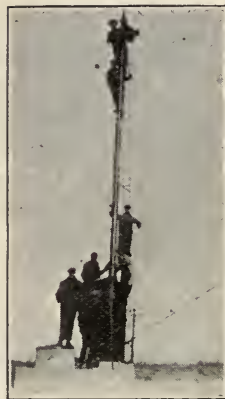
Loading signal cases and fitting up new signals on the Kentucky division
