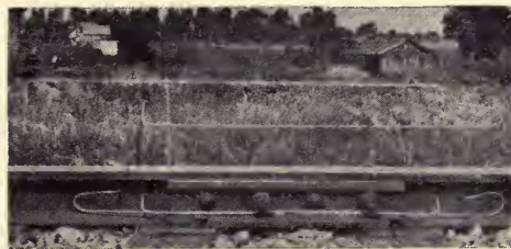
Bonding. The top wire shows the way the wire is bent before it is applied to the rail. The second wire shows the way the wire is bent after one end has been applied and the loop is made to apply the other end.
