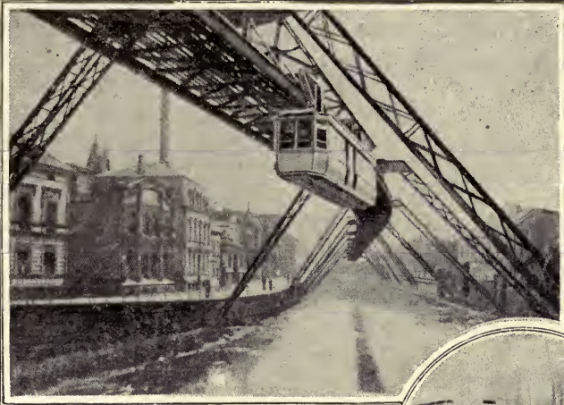
The famous suspended railroad of Elberfeld. By making use of the space above a canal, the elevated road is made possible without obstruction of street traffic.
