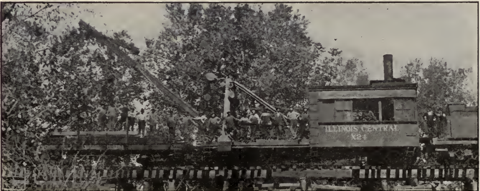
This picture shows a portion of a temporary bridge constructed on May 13 over the Sioux River on the Iowa division. On this date this bridge, consisting of seventeen 5-pile bents, with an average height of 18 feet and a length of 225 feet, was entirely destroyed by fire. Men were assembled and material loaded and moved to the location in record time, with the result that not a passenger train was delayed—the Iowa division still maintains its usual record of "passenger trains 100 per cent on time."
