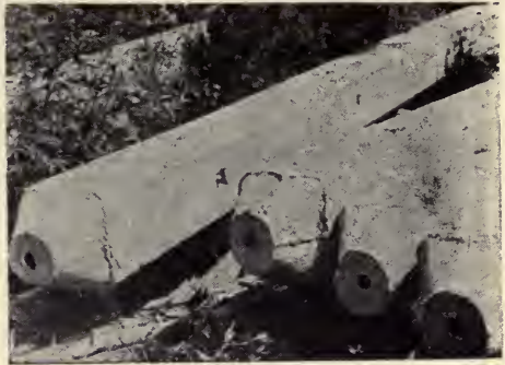
Fig. 3. Bignell piling.
