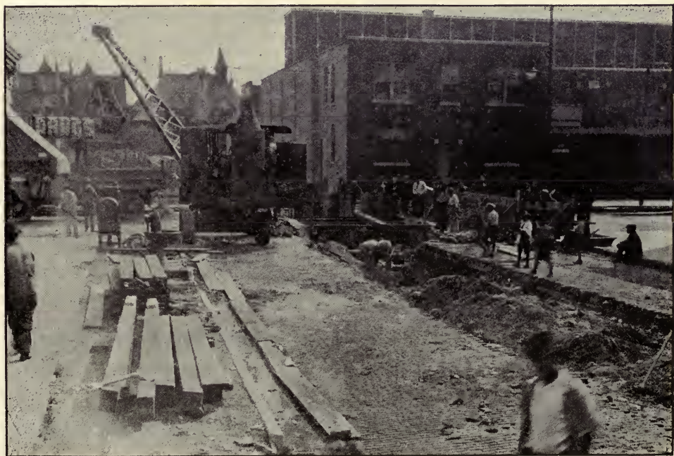
Figure 4. Steam shovel at work on Rhodes Avenue sewer
