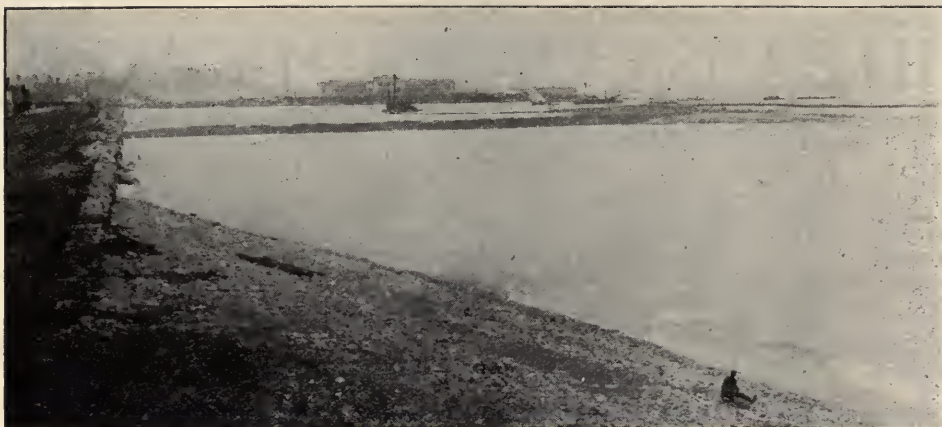
Figure 2. View of 23d Street dam looking north, showing suction dredge placing fill
