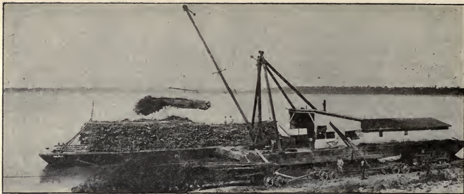
Floating derrick transferring willow brush from log wagons, hauled by tractors, to barge, to be floated to site of bank revetment construction.
