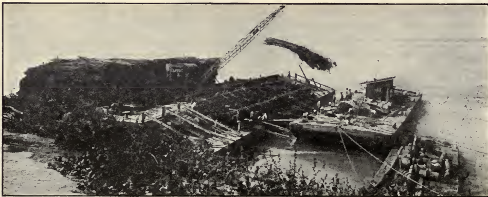
Beginning the construction of willow mat to be used in repairing bank revetment at Cottonwood, Miss., season of 1921. Showing the method of handling willow brush from barge by locomotive crane.
