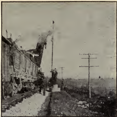
Derrick outfit placing mast on signal case
