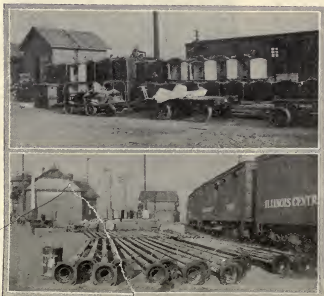
Above: Local wiring installed in signal cases at Nortonville. Below: Signal masts fitted at Nortonville.
