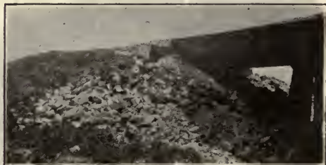
Where embankment was washed away at the bridge—hole now filled with earth, gravel and rip-rap.
