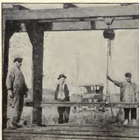
Method of handling frog to be repaired
