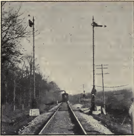
New automatic signals in service. Train No. 195 is shown in the block
