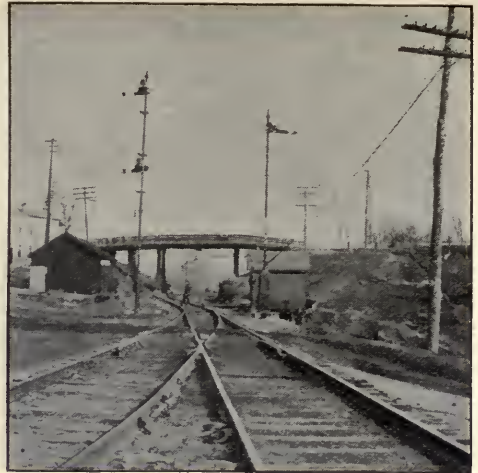
New signals in service; interlocking signals at left; automatic signal at right
