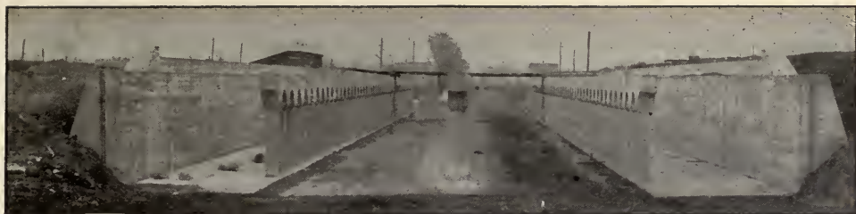
Concrete work for Markham yard subway at Harvey
