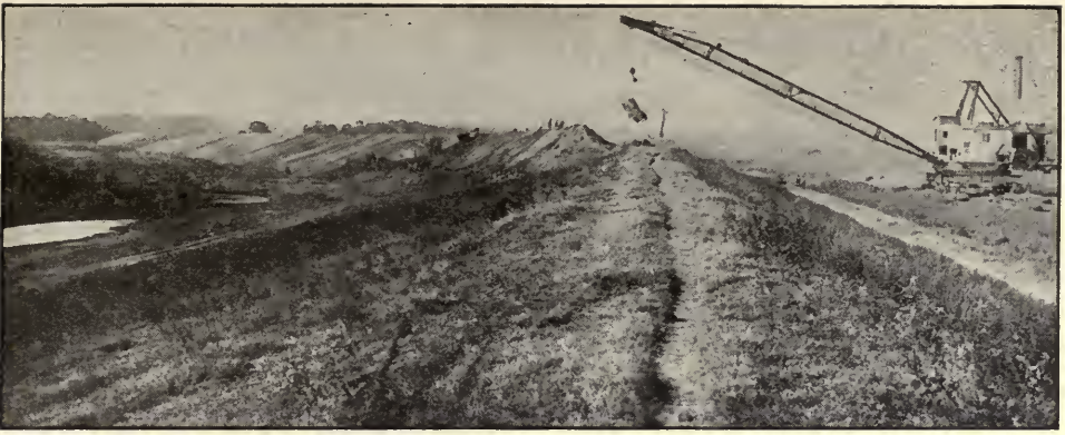
One of the types of machines used in levee construction on the Mississippi River—the revolving drag-line, Unit No. M.R.C. B-7. A stretch of completed levee enlargement also is shown.
