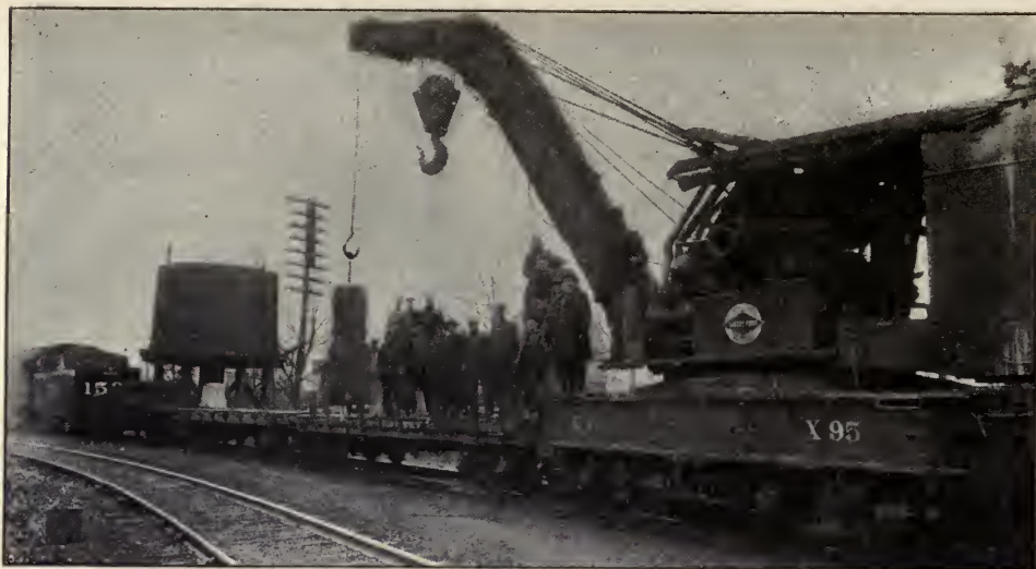
Derrick outfit unloading signal foundations and signal cases at the Paducah, Ky., yard. Derrick Foreman Joseph McCarthy, Signal Supervisor J. P. Price and Signal Foreman C. C. Sauer are standing on the derrick.
