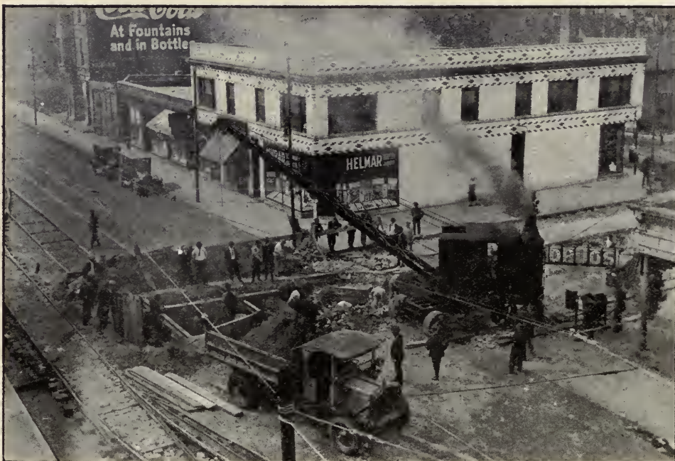
Figure 5. Excavating for junction of 7-inch and 20-inch sewers at Rhodes Avenue and 39th Street
