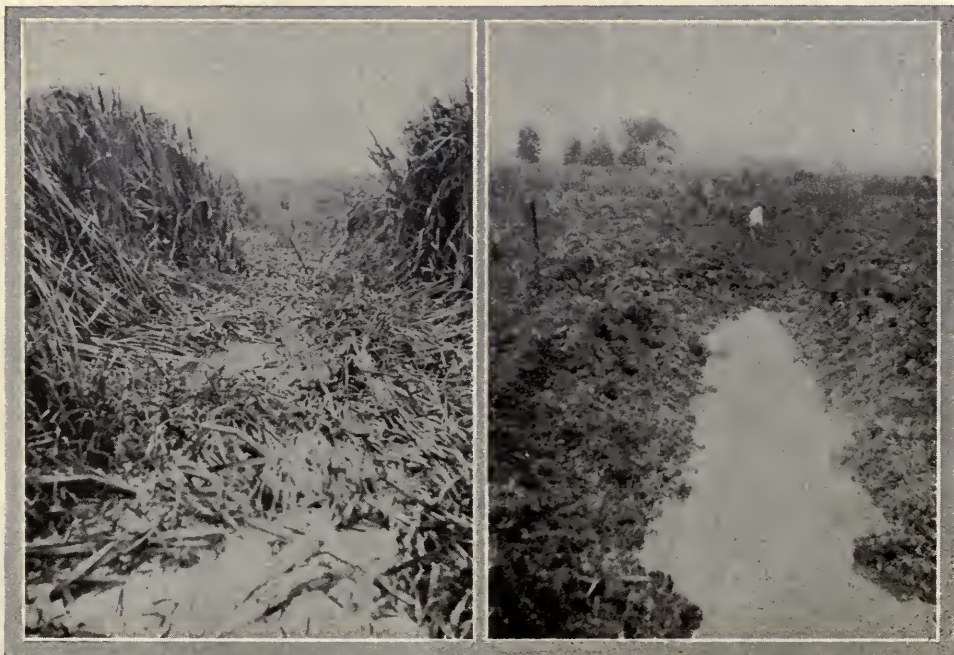
Before and after explosion of dynamite in swamp
