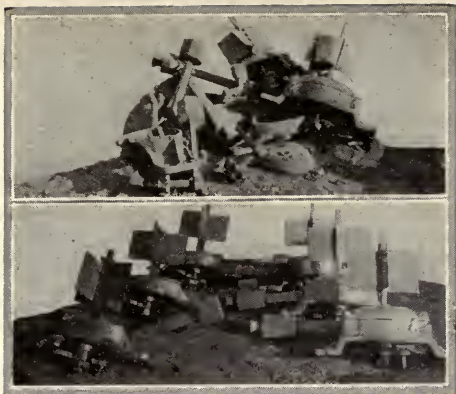
Switch stands before and after welding
