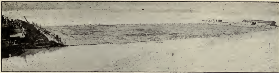
Construction of willow mat in progress, Princeton, Miss., season of 1921. The mat as shown is 250 feet wide and 500 feet long. It was completed to a length of 1,000 feet. Upper bank has been graded. A connecting mat fills the "pocket" remaining between the mat and the low water line.
