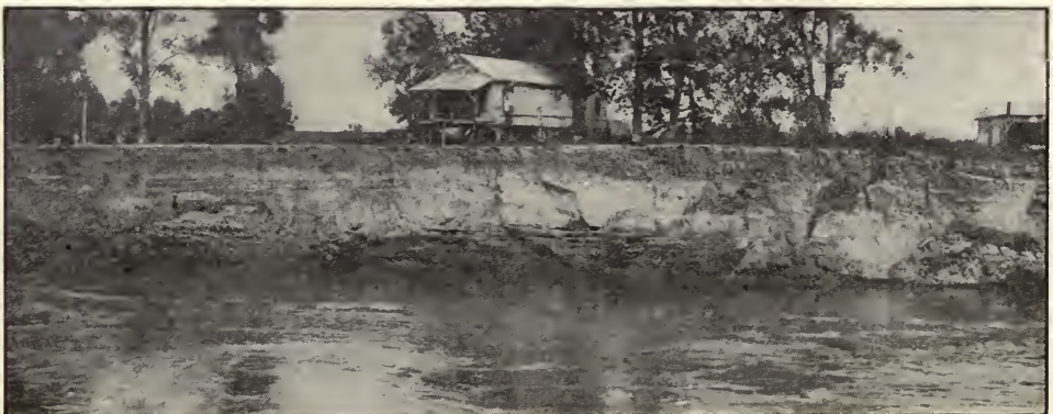
Riverton Landing, near Rosedale, Miss., in October, 1921. The caving bank threatened to cut under the store and take it into the river. This stretch has now been revetted.
