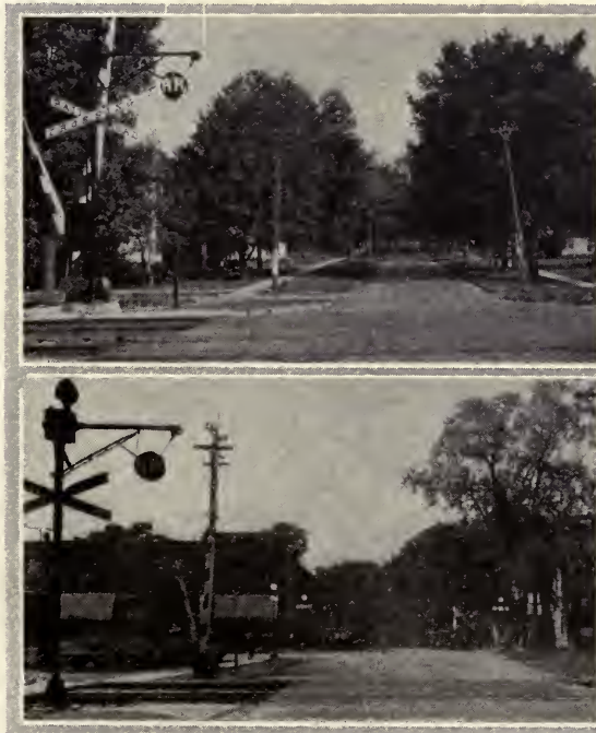
Top, left: Electric wigway crossing signal at First Street, South, Onarga, Ill., replacing hand-operated crossing gates. Below, left: Similar equipment at First Street, North, Onarga. At right: Gang which installed the new signals at Onarga. Top row, left to right: E. H. Brown, George Ringo, Guy Fox; middle row: Alpha Rose, Arthur Cohea, Charles Hildebrandt; front row: Leo Reynolds, Kenneth James, James Bright. Photographs from S. C. Hoffman, supervisor of signals, Illinois division.
