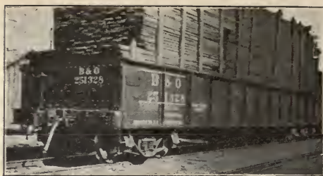
B&O-251328, loaded by the W. W. Gary Lumber Company, Percy, Miss., contained 34,219 feet of lumber weighing 142,000 pounds.
