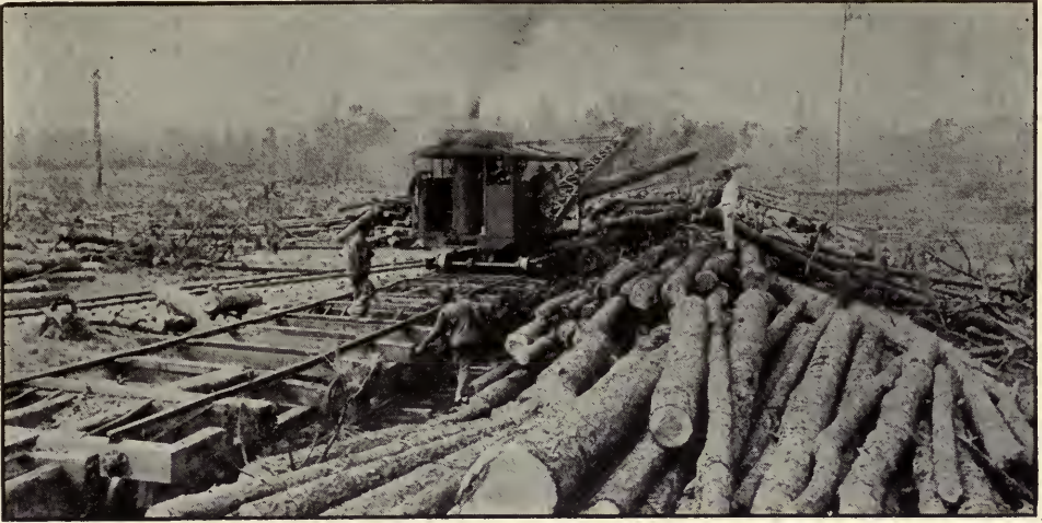
Loading derrick has track on tops of cars.
