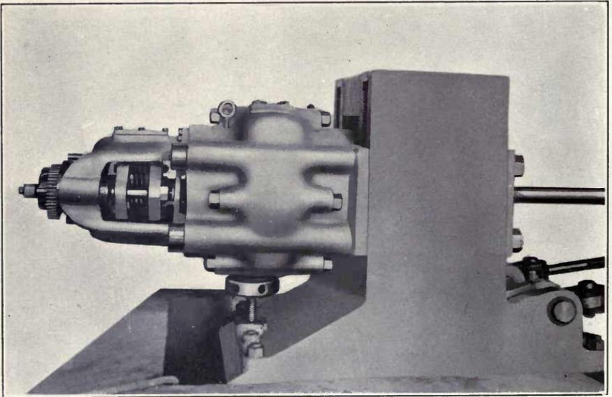
FIG. 49. THE WEIGHING HEAD AND PEDestal OF THE DYNAMOMETER.
