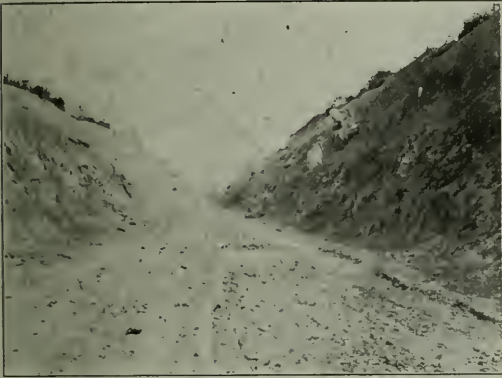
Soldiers' Home Cut, Johnson City, Tenn. 85 ft. at center. 500,000 cu. yds. removed.
