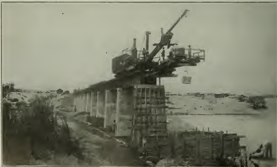
Fig. 13—Conchos River Bridge; Method of Depositing Concrete in Bases.
