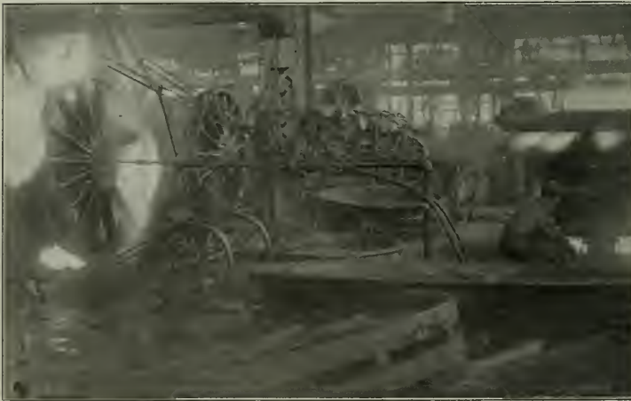
Crude Oil Tire Heating on the Lehigh Valley.
