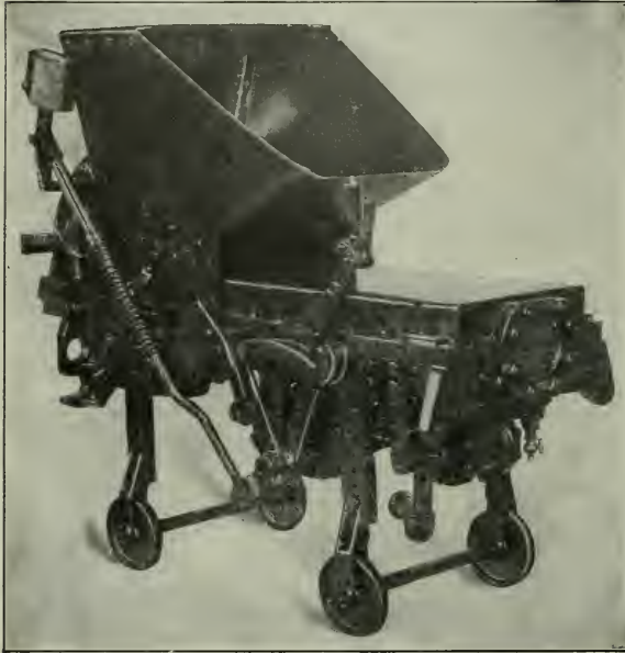
Strouse Locomotive Stoker.
