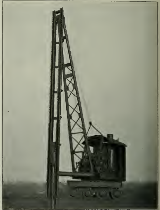
Fig. 3—Driving Pile at Angle With Track.
