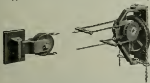
Fig. 2—Loose Pulley or Transmission Bracket.
