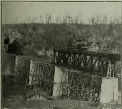
Bridge Over South Fork of Holston River. Steel Work for This Structure Was Erected Complete in 11 Working Days.
