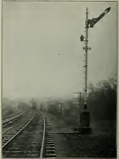
Fig. 8—Automatic Three-Position Block Signal—One Block Clear.
