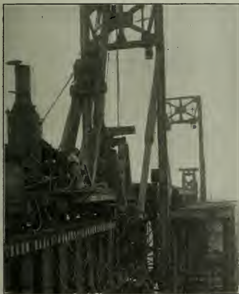
Fig. 5—New Span Lowered Part Way.
