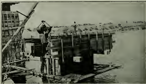
Fig. 12—Method of Sinking Wooden Cofferdams.
