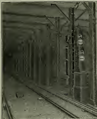
Typical Block Signal, New York Subway, showing also Train Stop.
