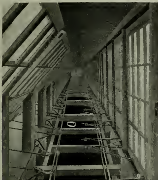
Fig. 1—Pond Operating Device in Clearstory.
