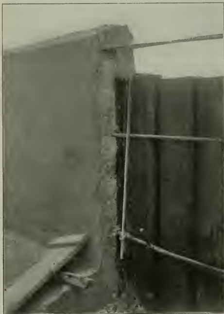
Detail of Reinforcement.
