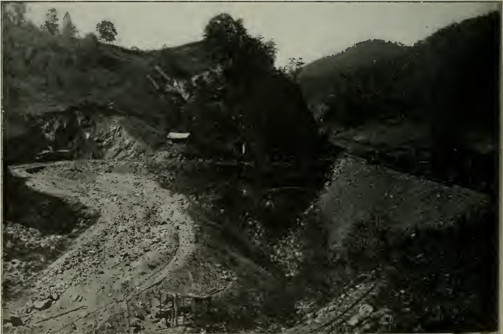
Fill Over Doe Branch, 125 ft. Deep at Center. Contains About 250,000 cu. yds.
