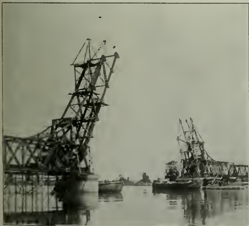
Erection of North and South Leaves.
