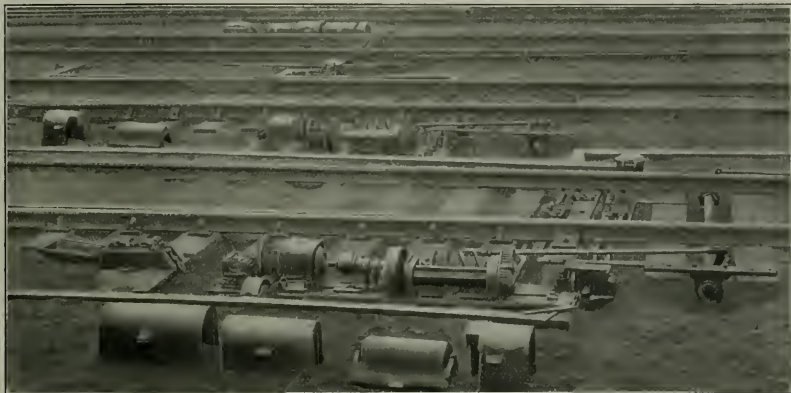
Union Electric Switch and Lock Movements.
