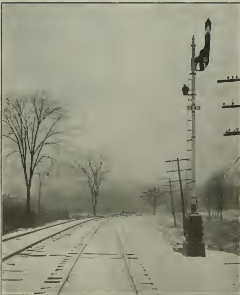
Fig. 7—Automatic Three-Position Block Signal—Two Blocks Clear.
