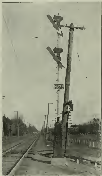
Fig. 11—Centrally Pivoted Semaphore near East Hartford.
