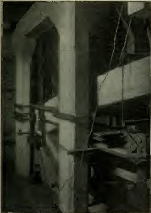
Fig. 2—Plumb Line and Microscope Used in Adjustment of Arch.
