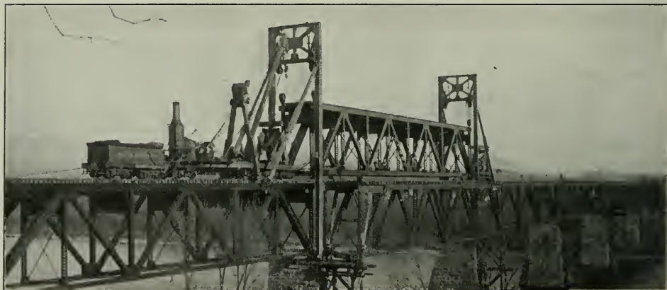
Fig. 3—Old Span Moved Out and New Span Ready to be Lowered.
