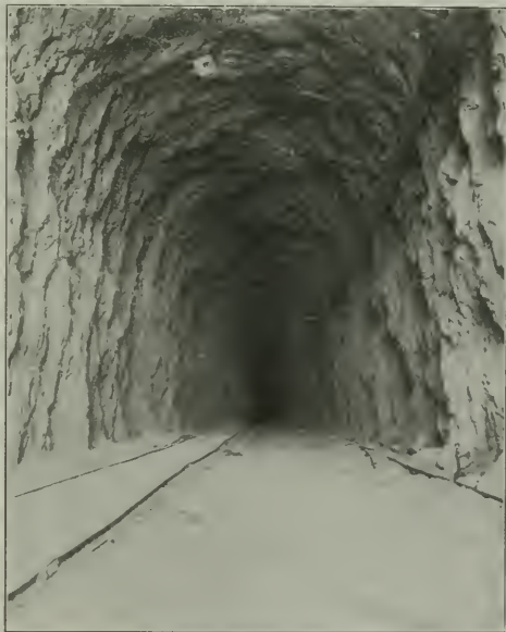
Interior of Unlined Tunnel.
