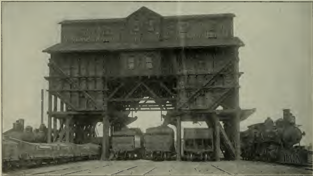
Fig. 2—Hunt Measuring Chute. Chesapeake & Ohio Yards, Richmond, Va.
