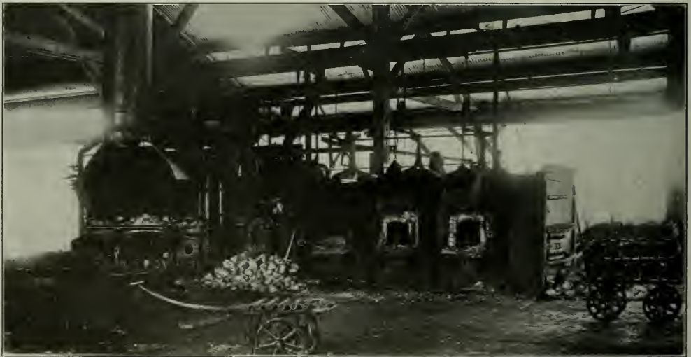
Three-Door Oil Reverberatory Furnace.
