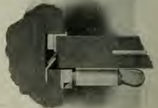
Cross Section Showing Side Weather Strip.
