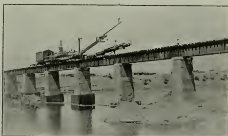
Fig. 11—Removing Extension Track.
