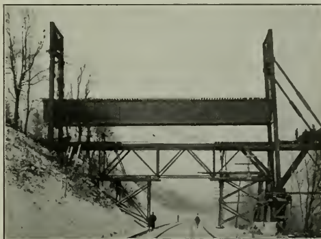
Fig. 6—Placing Approach Girder Span. Rails and ties partly removed from old span.
