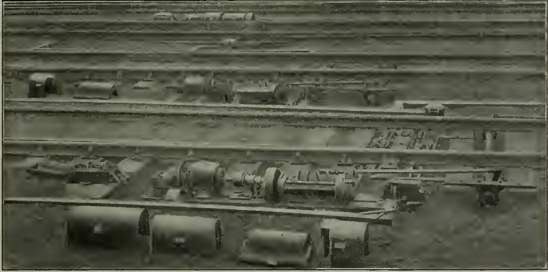
Union Electric Switch and Lock Movements.
