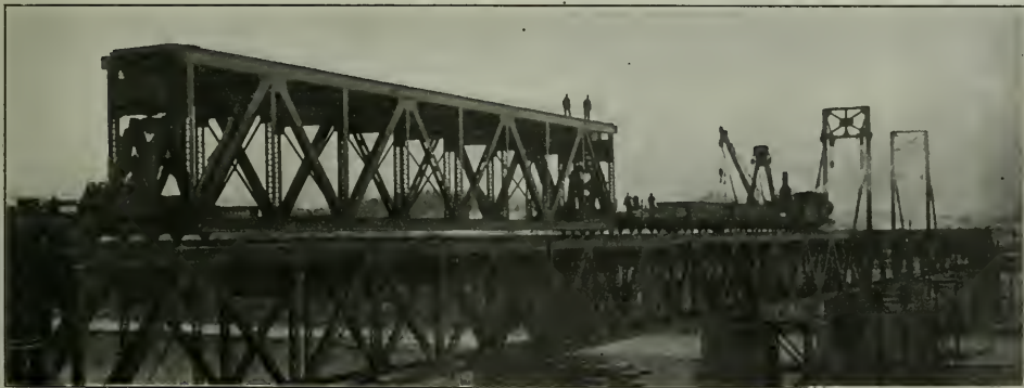
Fig. 1—New Span on the Way to Position.
