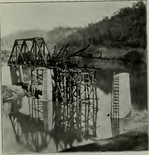
Clinch River Bridge at Starnes Bend. 3 spans of 120 ft. each.
