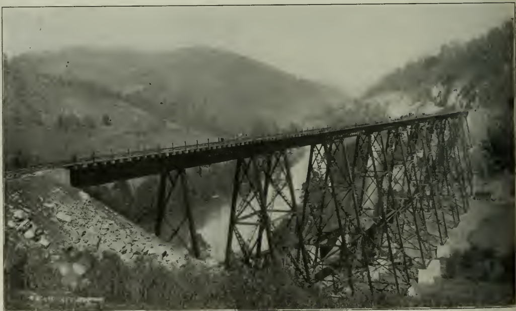
Copper Creek Viaduct, near Clinchport, Va. (1,360 ft. Long. 168 ft. Base of Rail to Stream.) Erected Complete in Five Weeks.
