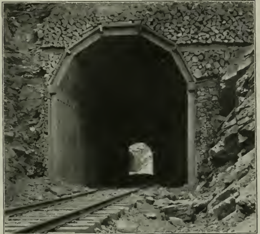
Tunnel Portal, Showing Packing and Inclined Strata.
