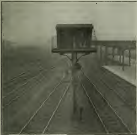
One-Arm Route-Signal and Indicator at Crewe.
