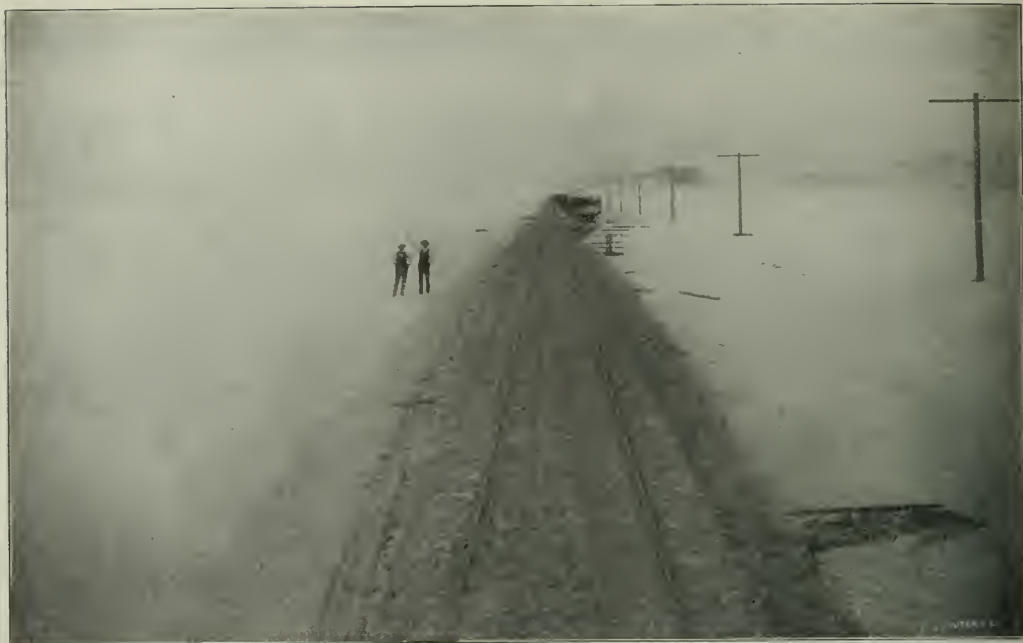
Roadbed of Solid Salt. Track before being raised and finished.
