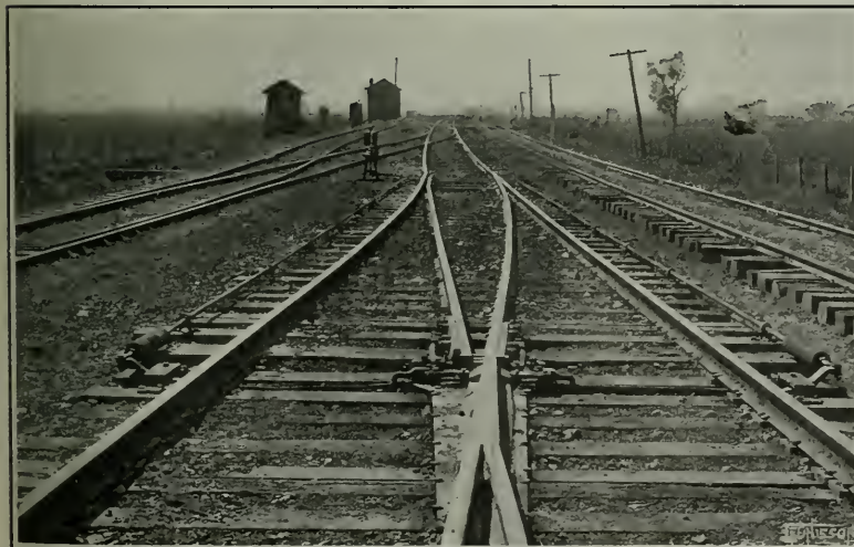
Fig. 2—Continuous Rail in Line for Turn-out.
