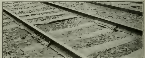
Williams Boltless Rail Joints in North Western Track.
