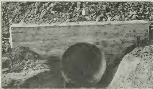
Typical Corrugated Iron Pipe Culvert with Concrete Head Wall.
