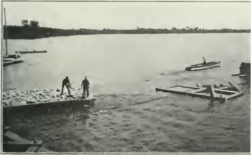
Fig. 1—Motor Boat Towing a Barge of Rock for Riprap.
