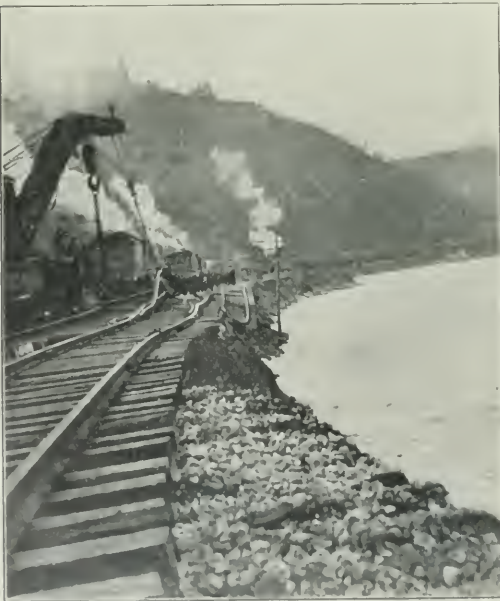
Picking 500 Ft. of Track out of the River with a Wrecking Outfit.
