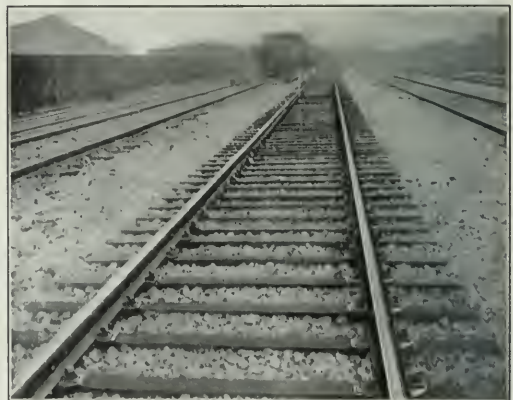
Steel Tie Track on Pittsburgh & Lake Erie Insulated with Fibre Shims.
