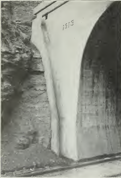
Concrete Drain for Carrying Water from Back of Parapet Wall Down to Roadway Ditch.
