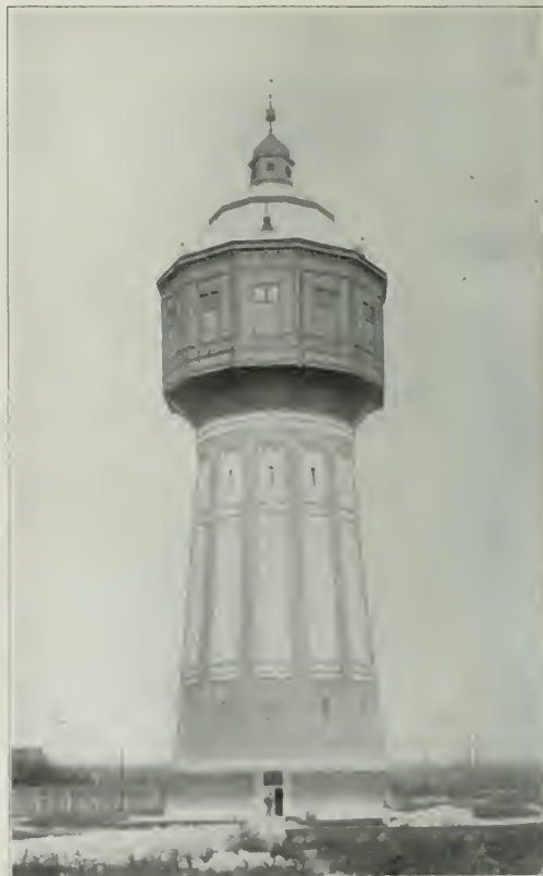
Engine House Water Tank 140 Feet High and Having 300,000 Gals. Capacity; Hungarian State Railways.
