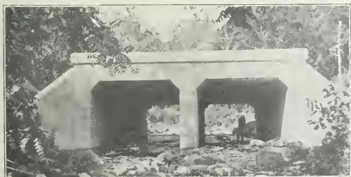
Fig. 2—Typical Slab Type Culvert for Waterway.
