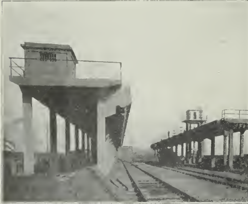
Hungarian State Railways Engine House, Showing Location of Ducts and Stacks for Carrying Out the Smoke and Gases.
