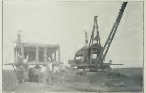
Filling Cars from Hopper Which Was Fed by the Drag Line.
