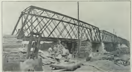
Building Substructure for New Deck Girder Structure.
