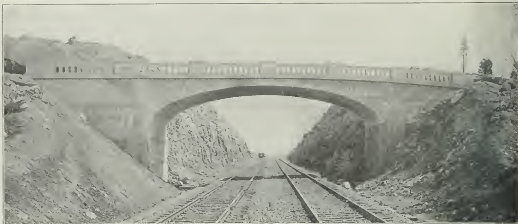
Fig. 4—Elliptical Arch Carrying Highway Over Tracks.
