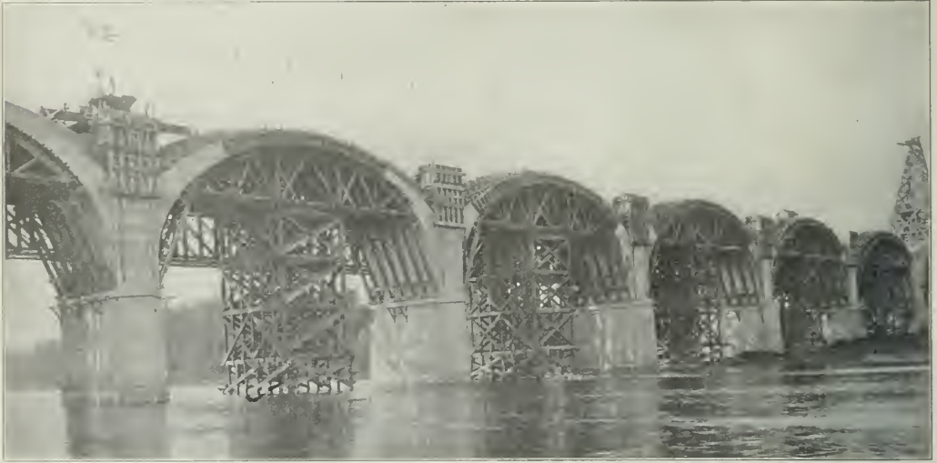
Fig. 8—Looking Upstream, Showing Arch Centering and Forms.
