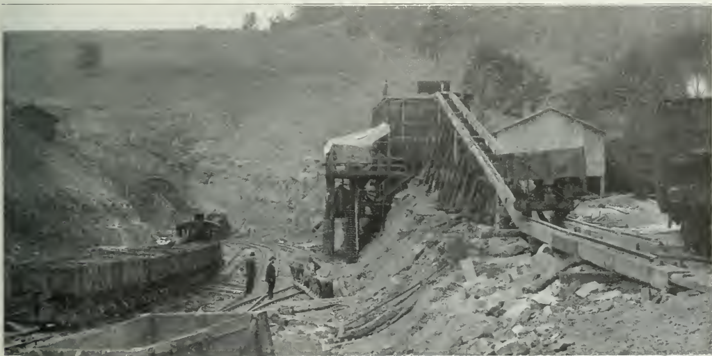
General View of Concrete Mixing Plant at East Portal.
