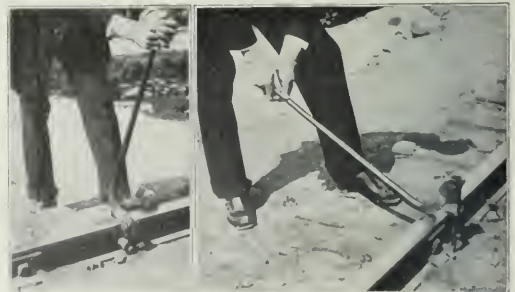
Spike Puller for Track Spikes.
