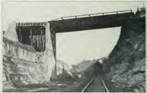
Box Abutment Under Construction for Woodland Ave.
