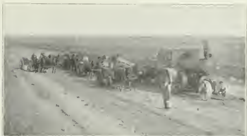
Considerable Light Grading Was Handled by Grading Machines, in this Case Pulled by a Traction Engine.
