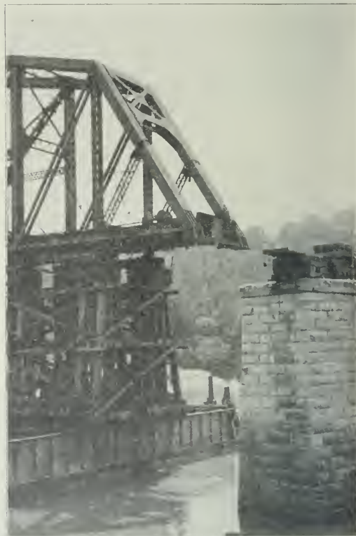
Barge Arriving at Pier Preparatory to Lowering Span onto Blocking.
