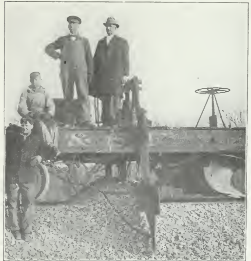
The Spreader Working In Stone Ballast.
