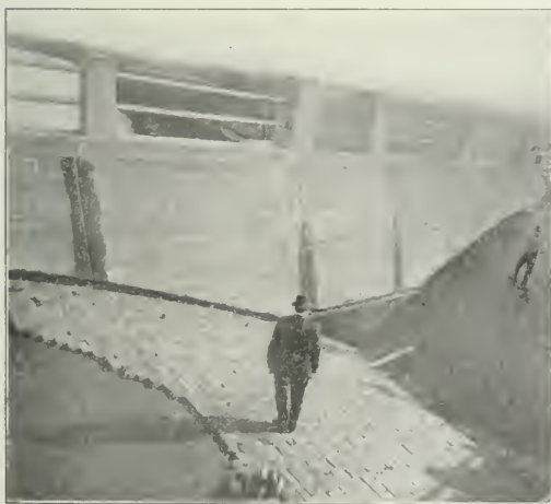
Fig. 11—Waterproofing Over Arches and Brick Covering.
