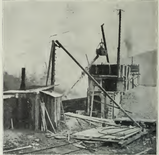
Concrete Mixing Plant, Material Hoppers at Top, Proportioning Platform Below, Mixer at Bottom.
