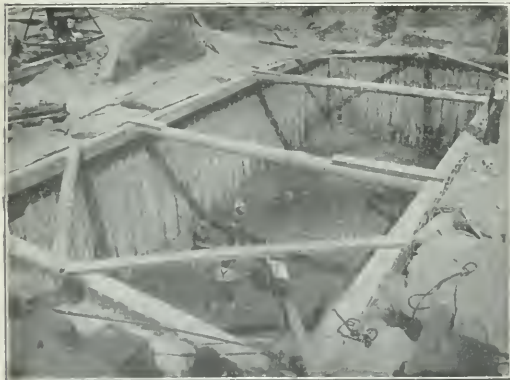
Cofferdam, 30 ft. \times 60 ft., of Straight Web Section Lackawanna Steel Sheet Piling; Buffalo Creek Railroad.
