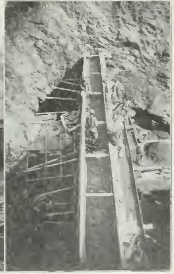
Concrete Car with Two High Levels for Shoveling into Upper Portion of Forms. Placing Concrete in Parapet Wall at Portal by Shoveling Twice.
