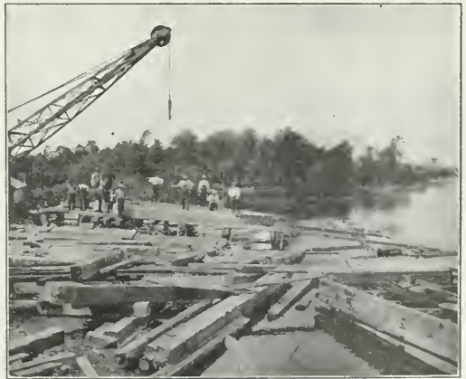
Fig. 2—Framing Timber Caissons for Richelieu River Bridge.
