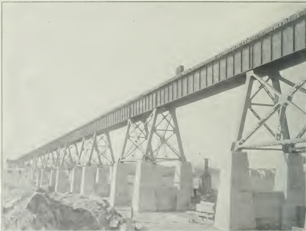
Weldon Viaduct Showing Web Struts Connecting Pedestal Piers.
