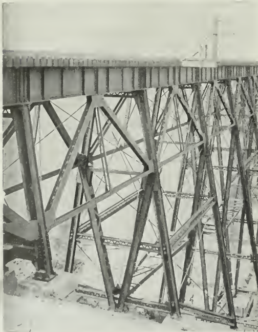
Details of Reinforced Viaduct, Pere Marquette.
