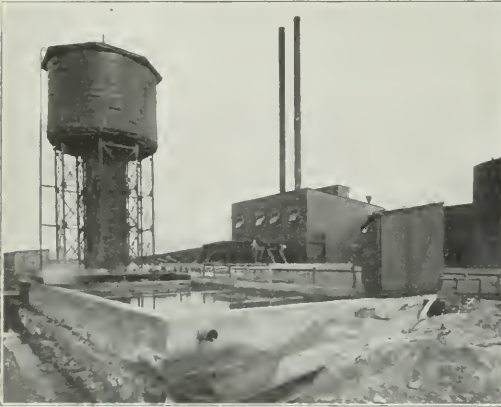
Concrete Settling Tank for Collection of Creosote.
