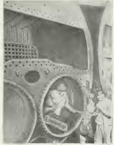
A Marine Boiler After Cutting Out Damaged Flue Sheet with Oxy-Acetylene Blow Pipe.
