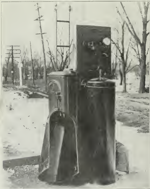
Acetylene Tank and Regulator for Flash-Light Signal.
