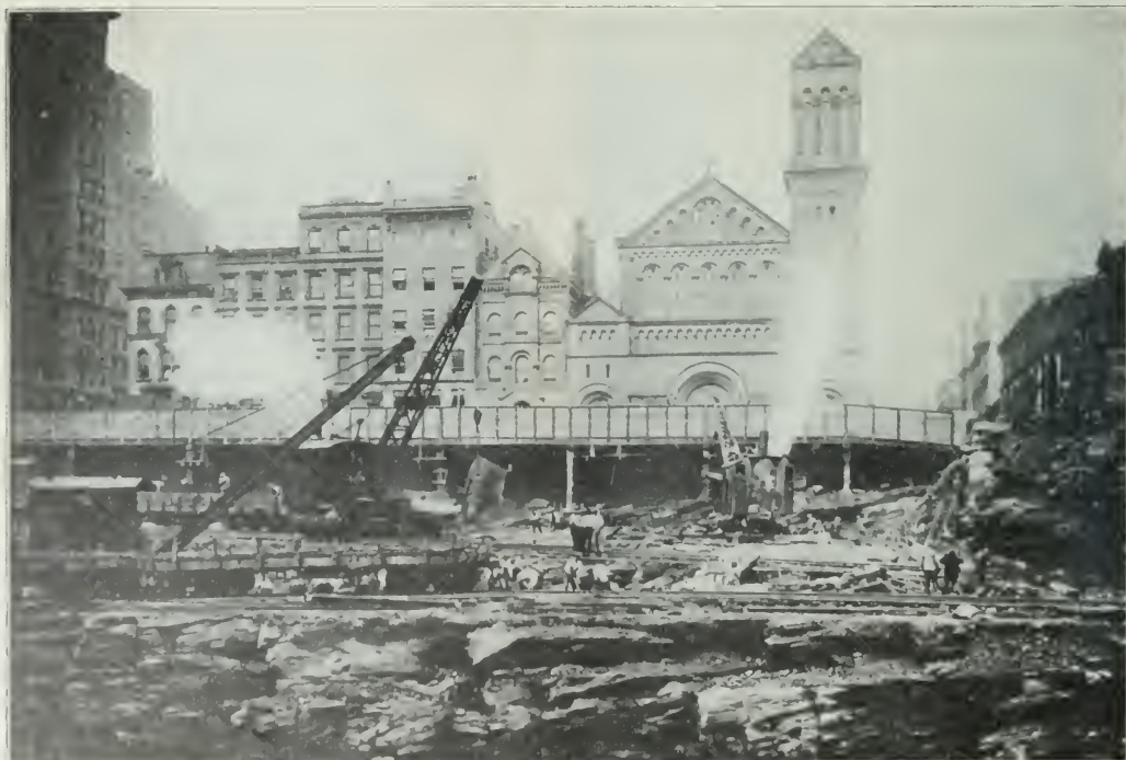
Browning Cranes Handling Rock Excavation for the New Grand Central Station, New York.
