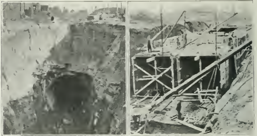
Circular and Rectangular Sections of O. K. Creek Sewer.
