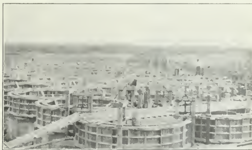
Forms for Concrete Grain Storage Bins with Jacks Used in Raising Forms.
