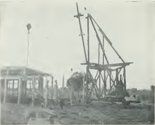
Fig. 2—Stiff Leg Derrick for Erecting Units of Roundhouse.
