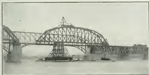
Launching Second Channel Span.
