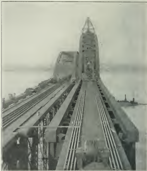
Deck of New Bridge Showing Track on Which Span Was Moved.
