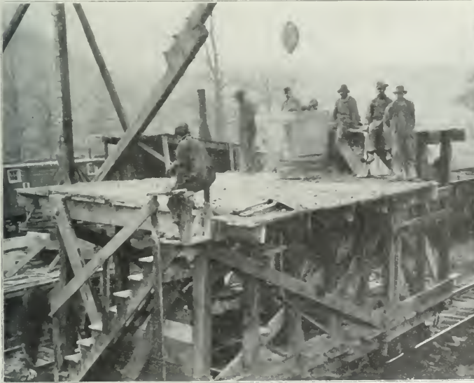
Concrete Car with Two High Levels for Shoveling into Upper Portion of Forms. Placing Concrete in Parapet Wall at Portal by Shoveling Twice.
