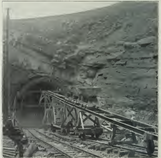
View Showing Steel Forms at East Portal and Incline for Bringing in Concrete.
