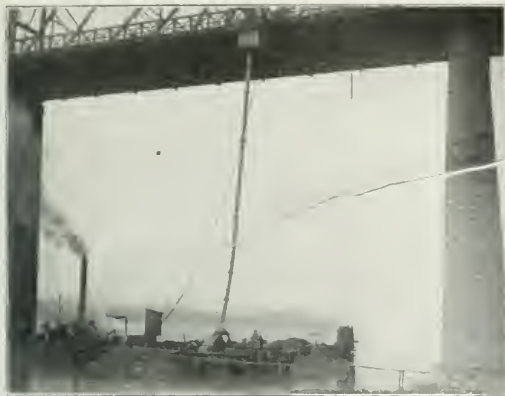
Dropping Concrete 115-ft. Into Bridge Piers.
