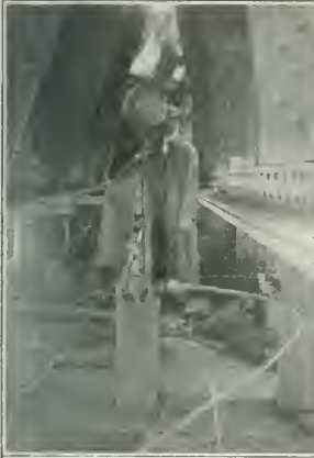
Jacking Up a Span.
