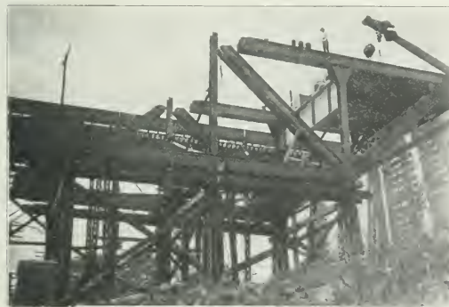
Erecting Deck Truss on False Work with Derrick Car.
