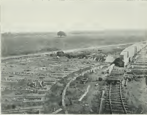
Fig. 1—Roundhouse Site Showing Foundations and Slab Yard.
