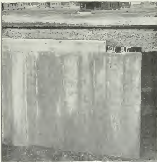
Lackawanna Protected Steel Sheet Piling.
