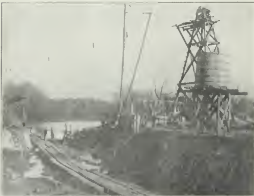
West Bank of Cape Fear River, Showing Forms for Shore Pin, Cable Tower and Pit from Which Puddling Clay Was Taken.
