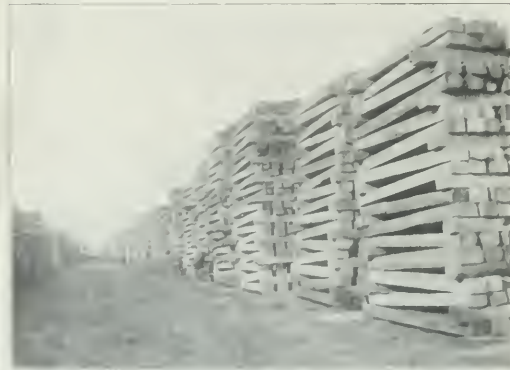
Fig. 7—View in Tie Yard Showing Method of Stacking Ties.
