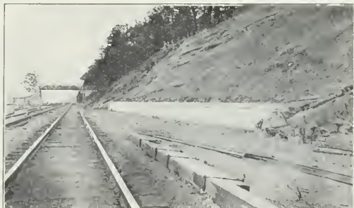
Completed Slope Showing No Indication of Rock Face in Original Cut.
