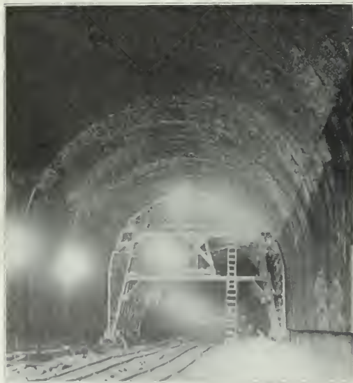
Inside of New Tunnel Showing Brick Facing Over Crown of Arch.
