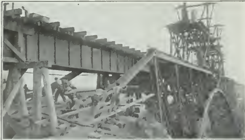
Adjusting Cantilever Arms Before Closure.
