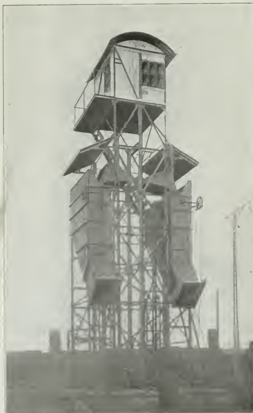
Steel Ash Hoist and Conveyor; Hungarian State Railways.
