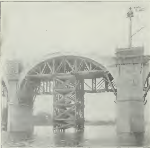
Fig. 9—Arch Centers and Falsework.
