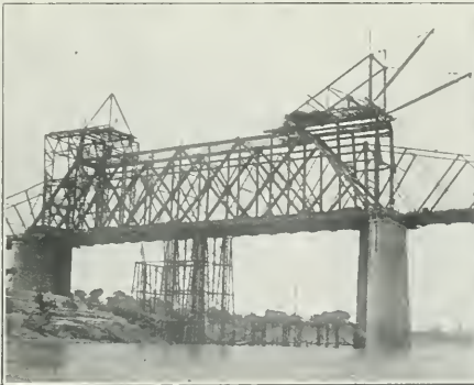
Portal View of Kentucky & Indiana Shore Span Erected. Traveler Used for this Span Bridge Across the Ohio River at Louisville, Ky.
