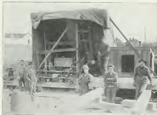
Tie Dapping Machine Operated by Automobile Engine.
