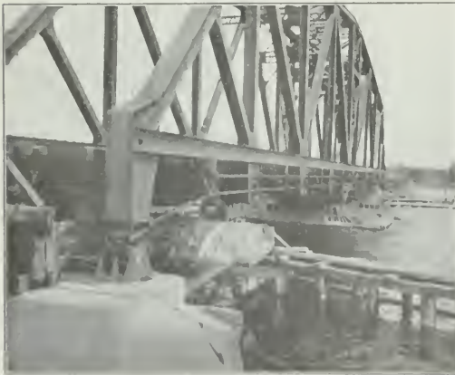
Fig. 4—New Span In Place on Completed Rest Piers, Showing Construction of Center Pier and Protection Work.
