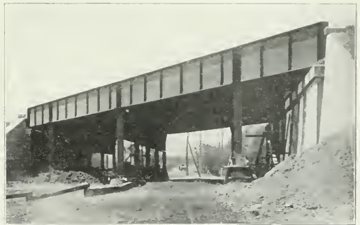
Four-Span Subway Carrying Omen Street West Under the Grand Trunk.
