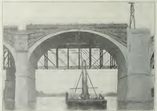
Fig. 10—Spandrel Wall Forms.
