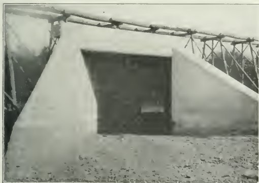
Typical Concrete Box Culvert on the N. C. & St. L.
