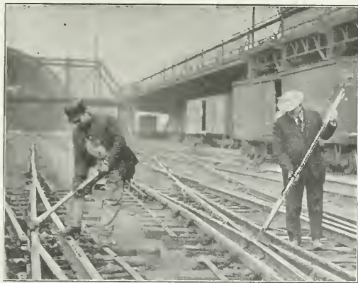
Using Blow Torch and Pick for Removing Ice.
