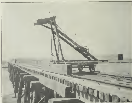
Small Hand Derrick for Lifting Heavy Timbers.
