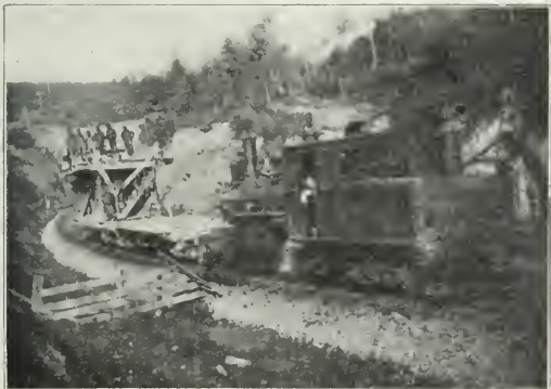
Train Used for Carrying Concrete from Mixing Plant to Tunnel.
