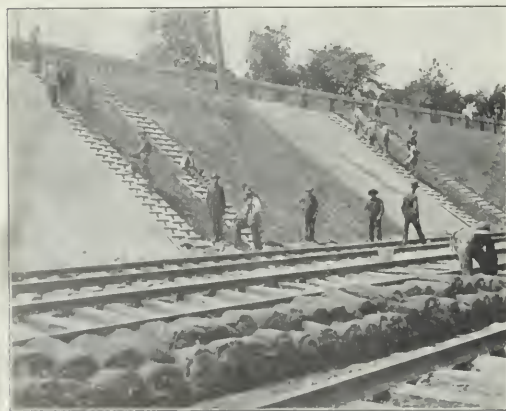
Laying Sod on New Slope in a Cut.
