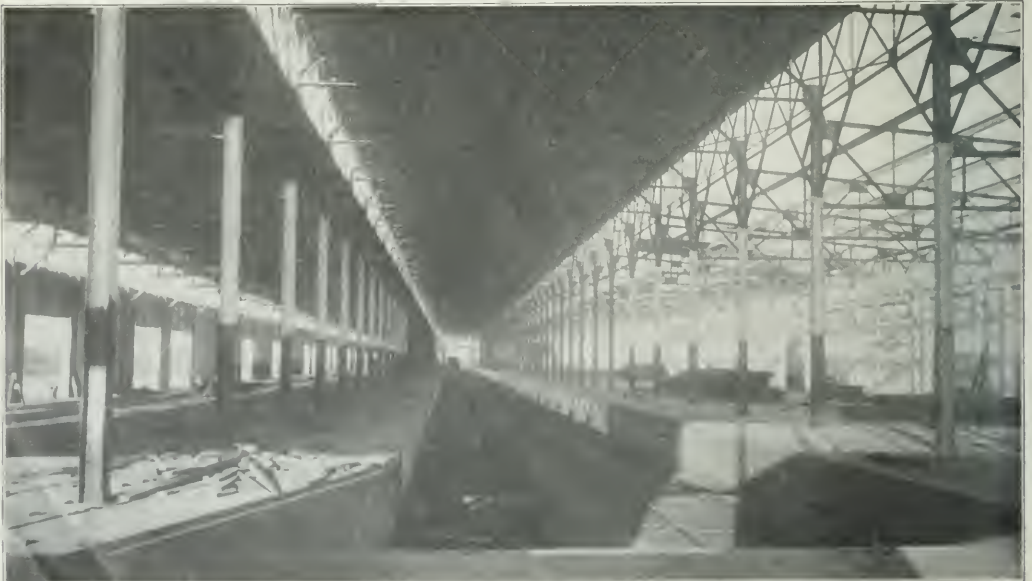
Interior of Pier Showing Track Well, Platforms and Steel Superstructure.
