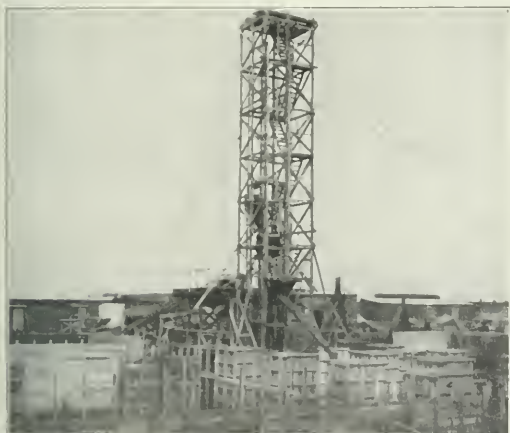
Stock Piles, Cement Houses, Mixer Plant and Distributing Tower at Elevator.
