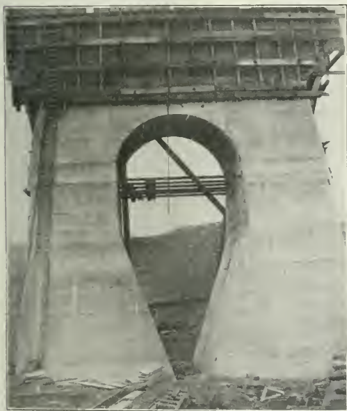
The High Abutment Before Forms for the Last Course Were Removed.
