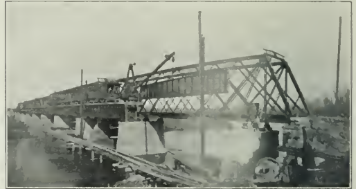
Erecting Down Stream Line of Girders.
