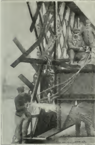
Cutting Up the Bellot Bridge with Oxy-Acetylene Blow Pipe at Havre, France.
