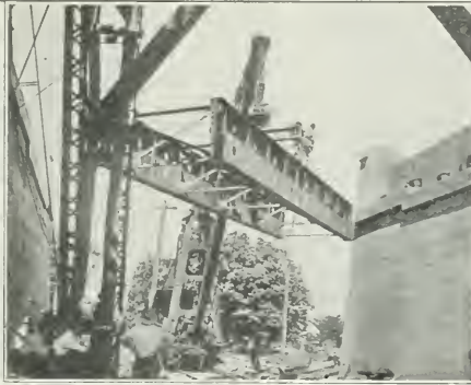
Erecting Plate Girders in North Approach.
