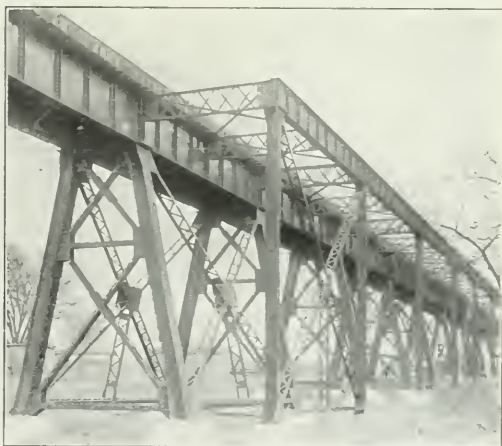
Portion of Weldon Viaduct Showing Steel Work for Station Platform.
