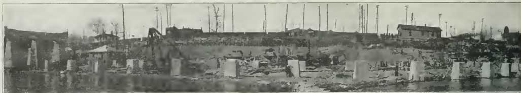
Panorama of Sunnyside Crossing Showing Abutment and Footings for Steel Trestle Approach.
