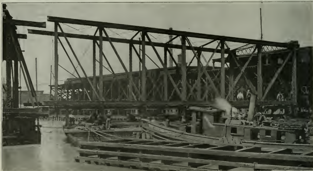
North Half of Old Span Supported on Scows and Completely Severed from the Rest of the Bridge
