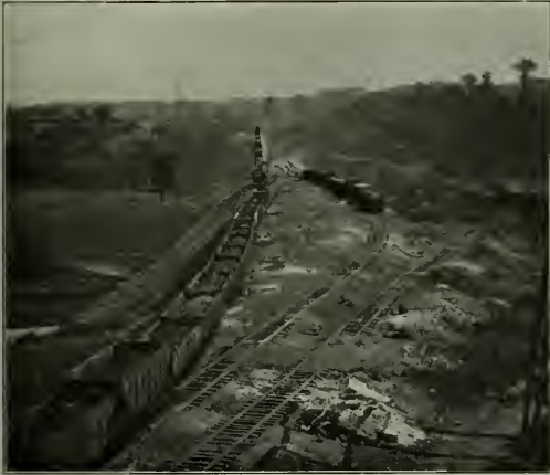
Looking Along the Fill Over the First Temporary Trestle. Second Trestle on First Bench at Right and Old Viaduct at Left
