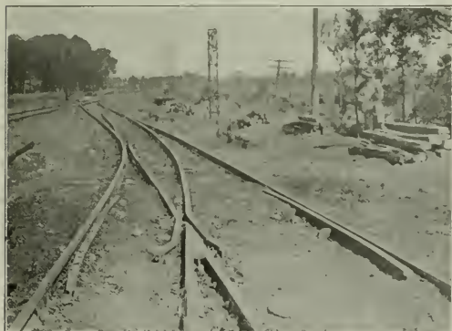
Arrangement of Switch Stands and Signals for Operating Crossing of a Narrow Gage Track and a Standard Gage Track
