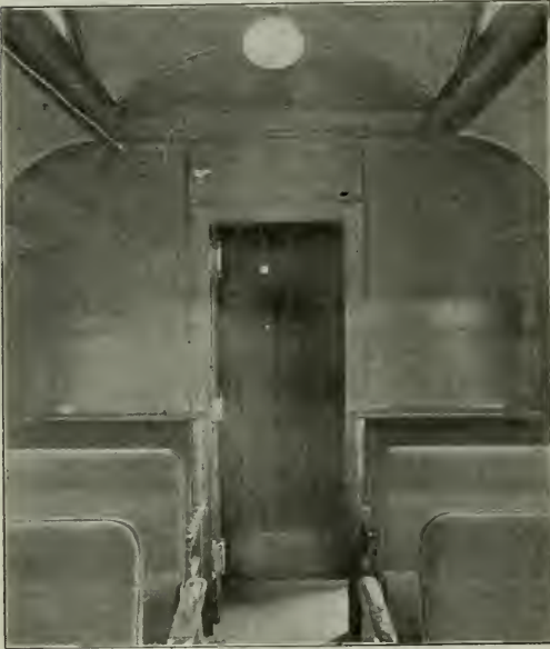
Veneered Steel Bulkhead in Canadian Pacific Steel Coach
