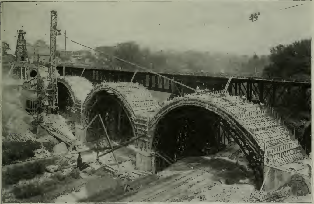
Concreting the Arch Ring and Spandrel Walls of the First Half Showing the Old Steel Bridge in the Background
