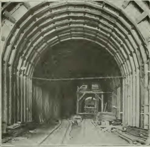
Interior of Point Defiance Tunnel Showing Timbering
