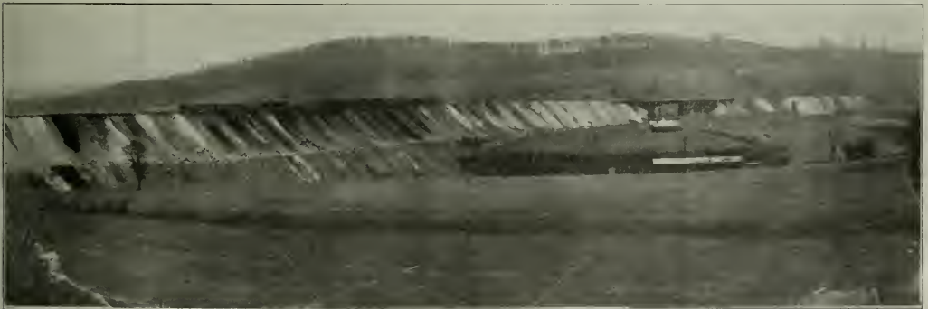
Panorama of Big Fill Near Culmerville During the Filling of the Temporary Trestle on the Second Bent
