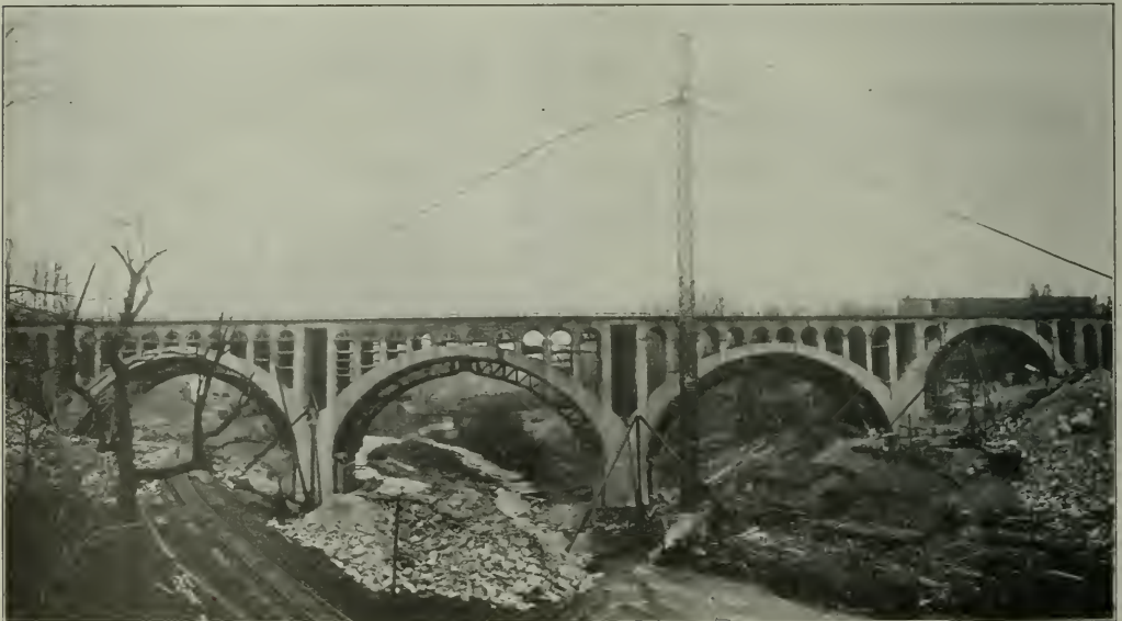
East Side of First Half Completed, Showing Concrete Distributing Tower in Position for Work on Second Half
