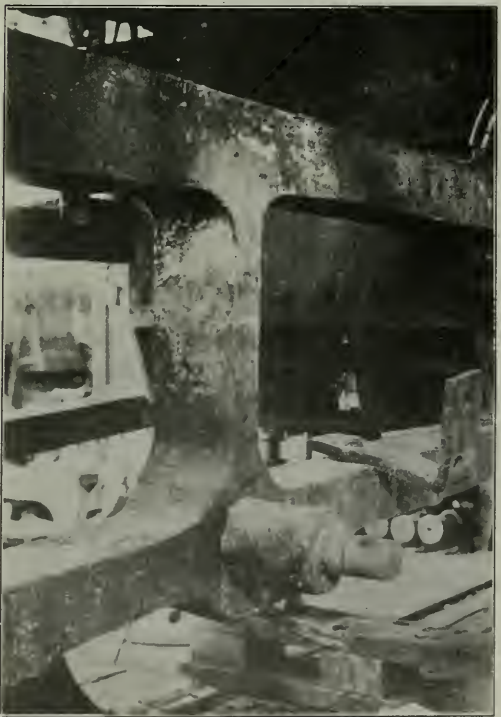
A Difficult Frame Weld Accomplished by the Oxy-Acetylene Process
