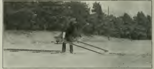
Lifting Section of Portable Track off Street Car Rails
