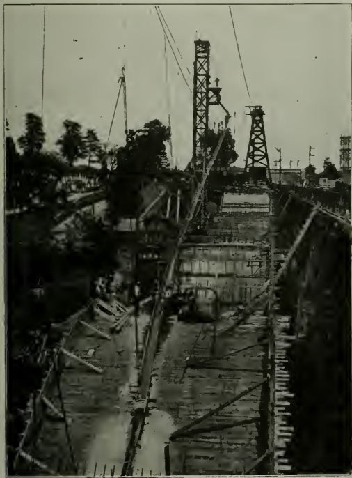
View Along Center Line of First Half, Showing Material Cableway and Concrete Distributing Tower
