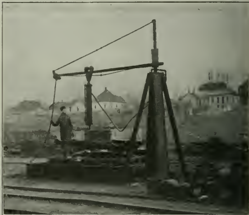
Crane and Vat for Immersing Reclaimed Material in Mixture of Asphaltum
