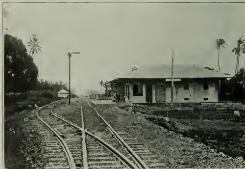
Typical Second Class Station at Sebonga Showing Passing Siding and Block Signal
