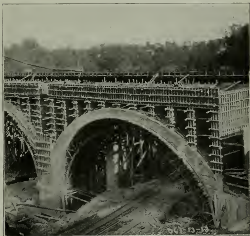
The Forms in Place for One of the Long Spans Showing Steel Arch Centers
