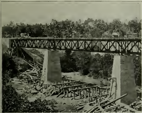
A Bridge with Enlarged Foundations on Soft Mud Foundation
