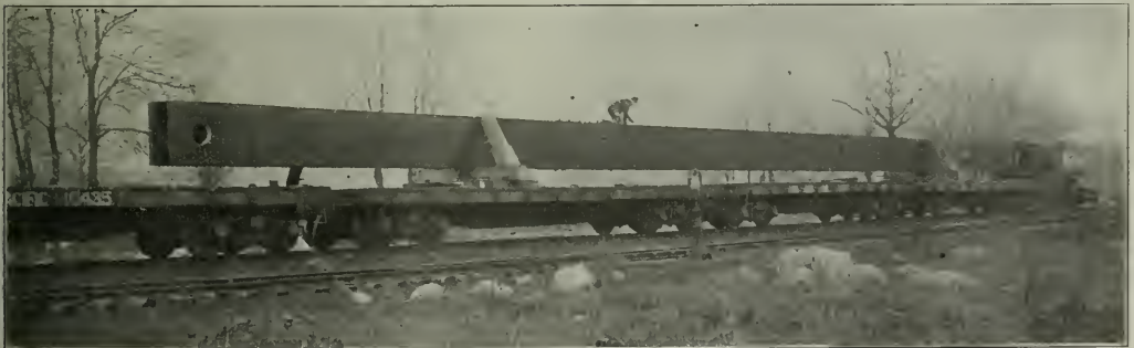
View Showing One Half of Diagonal Tension Member 108 ft. Long on Cars for Shipment
