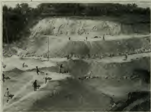
Constructing a 13,000 yd. Fill on the Island of Cebu
