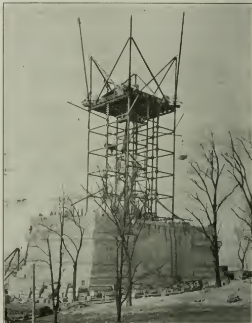
The Construction Plant Used in Building the East Abutment of the Hell Gate Arch
