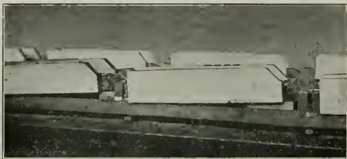
Special Device for Holding Shoes and Wedges on Planer
