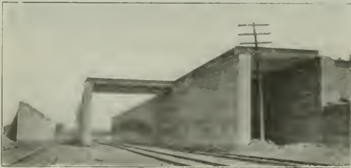
Crossing No. 4 With a Portion of the Deck Laid
