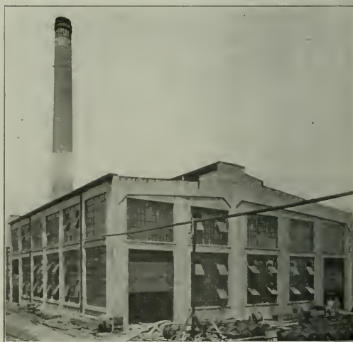
Powerhouse After Completion Showing Temporary End Construction Arranged for Ready Removal When Necessary to Extend the Building
