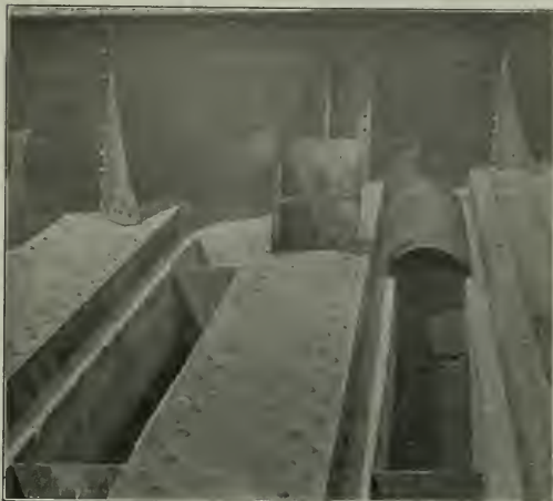
Typical Floor Construction on Trough Floor Subway, Using Blaw Steel Arch Forms
