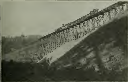
Constructing Heavy Fill at Approach to Patterson Lake
