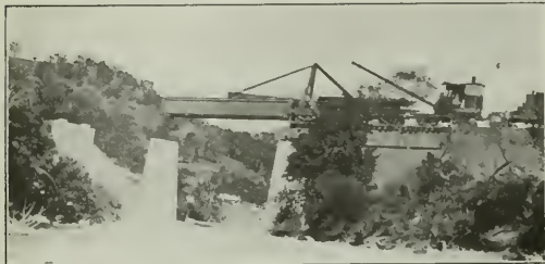
Placing 60 ft. Girder Span With Derrick Working on Adjacent Span
