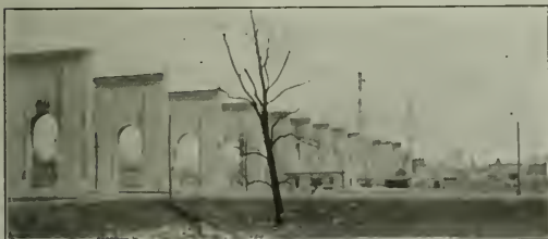
A Portion of the Long Island Viaduct Showing Concrete Towers Used in its Construction, Eastern Viaduct in the Background
