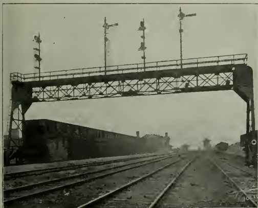
Fig. 1—Signal Bridge with Dwarf Signal Mounted Above Lower Chord
