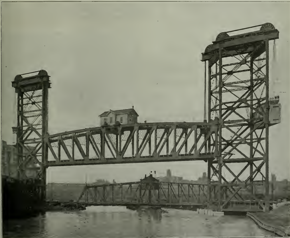
New Vertical Lift Bridge Over Chicago River Replacing Old Swing Span Shown Below
