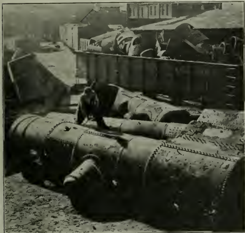
Old Boilers and Fireboxes are Cut with the Oxy-Acetylene Burners Into Pieces Convenient for Handling
