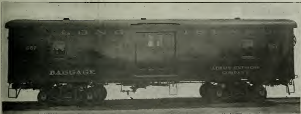
Light Baggage Car of Steel Construction for the Long Island
