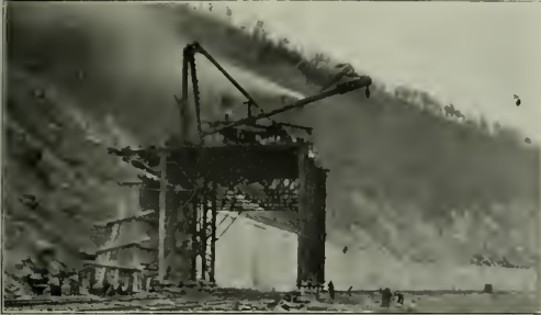
Traveller Used for Constructing Retaining Wall East of Paw Paw
