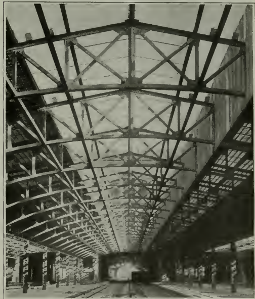
Portion of the Train Shed at Kansas City Station Showing Vertical Tiles Along Right Side of Smoke Duct
