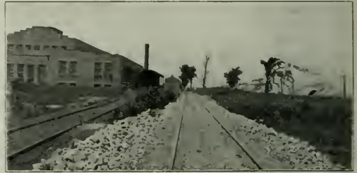
View Showing the Condition of the Track After Leveling Heavy Ballast with the Lawrence Spreader
