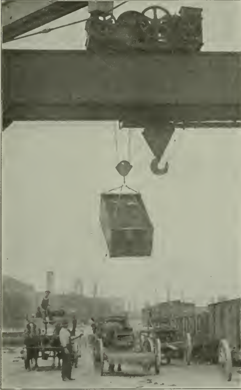
Fig. 2—Loaded Wagon-body, to be Emptied into Gondola
