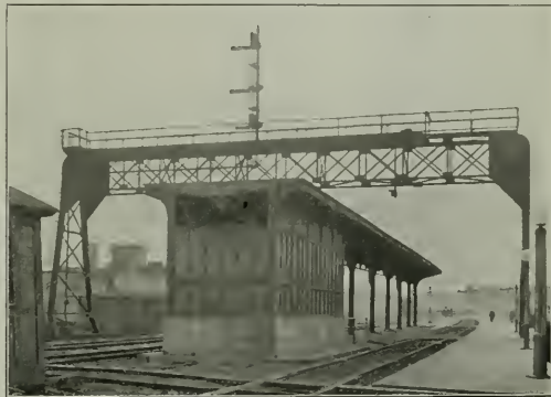
Fig. 3—Signal Bridge with Suspended Dwarf Signal
