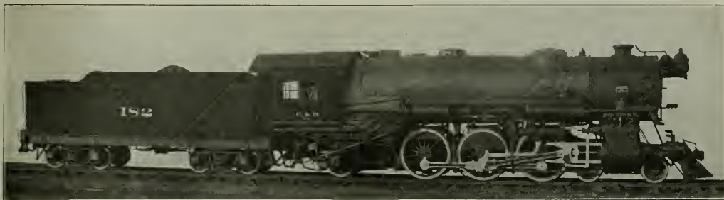
Chesapeake & Ohio Pacific Type Locomotive Which Has a Maximum Tractive Effort of 46,600 lb.
