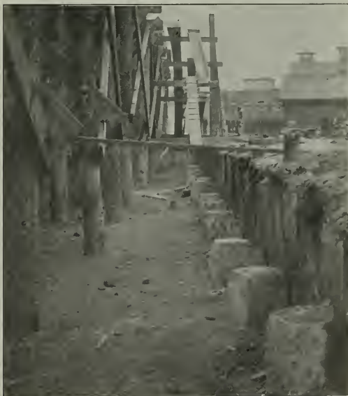
A Row of Concrete Piles in Place for Toe Supports, Under Retaining Wall
