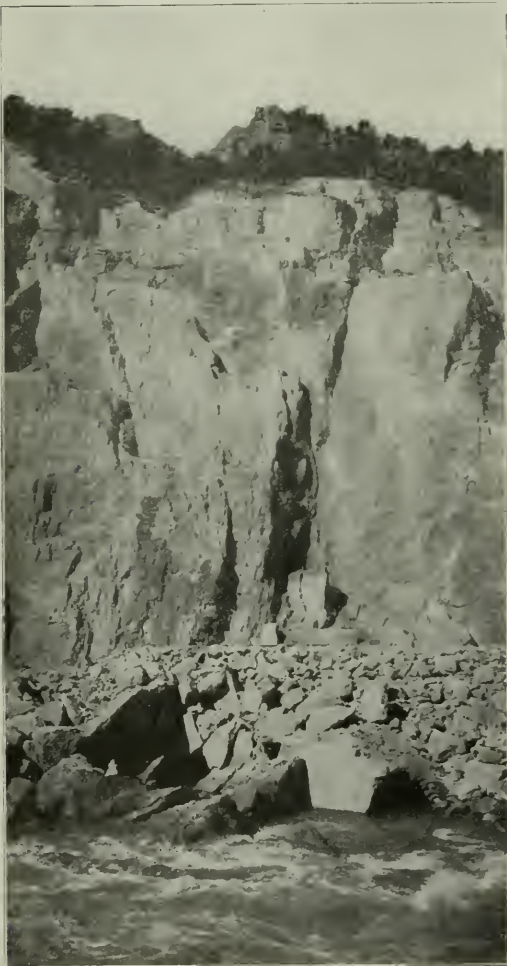
After the Heavy Shot was Fired, Bringing Down 30,000 cu. yds. of Rock
