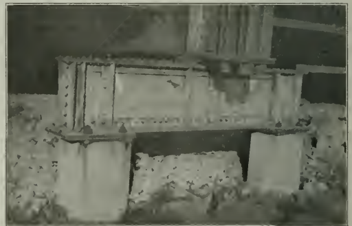
Fig. 4—Octagonal Concrete Casings Supporting Girders and Floor Beam
