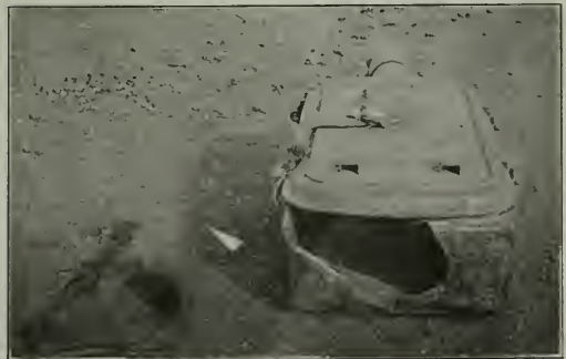
Broken Signal Post and Relay Box Awaiting Repairs
