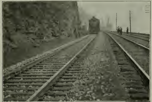
Main Line Passenger Track on the Pennsylvania Lines Laid With National Steel Ties
