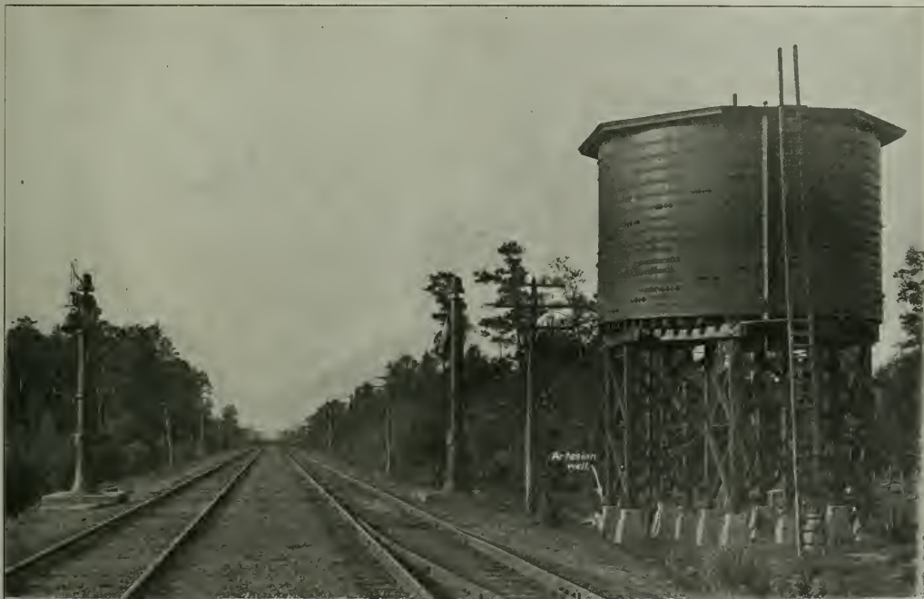
Illinois Central Water Station at Roseland, La., Securing Supply from an Artesian Well
