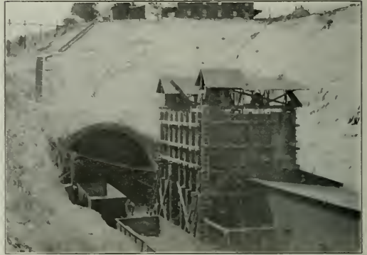
Concrete Mixing Plant at Entrance to Point Defiance Tunnel
