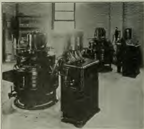
Interior of Pennsylvania Pump House Showing Motors and Controllers
