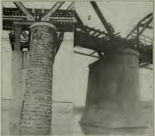
Pier 4. Showing Steel Bent Encased in Concrete
