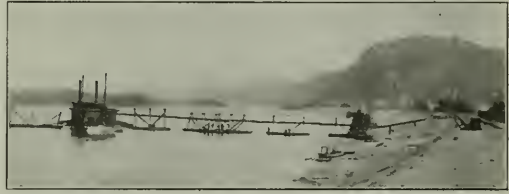
Completing a 300,000 cu. yd. Embankment at Lynxville, Wis.
