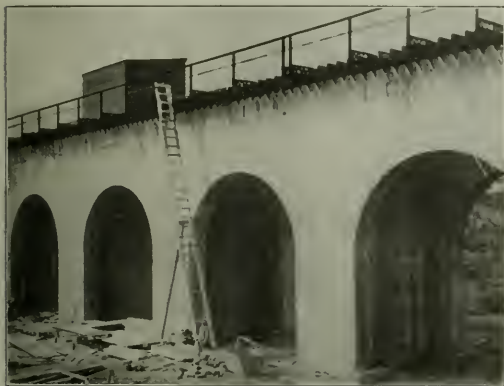
A Portion of the Concrete Trestle in Crossing No. 1. Concrete Deck Slab Has Not Yet Been Placed
