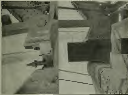
Truss Shoe Overhanging Bearing
