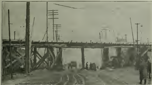
Temporary Trestle Over St. Clair Avenue, Showing Type of Construction Used and Provision for Street Traffic
