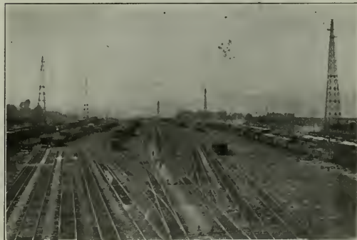
General View of the P. & L. E. Yard at McKees Rocks Showing 100-ft. Steel Towers Supporting 2400 Candlepower Lamps
