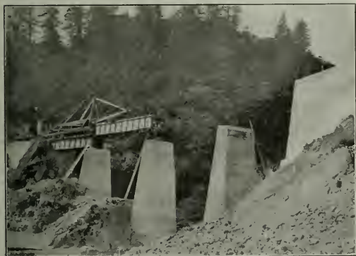
Lowering a 60 ft. Span Into Place
