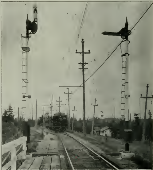
Automatic Signals at Entrance to Passing Track on the Oregon Electric
