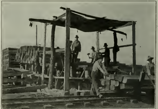
A Close View of One of the Skidways Showing the Inspection, Marking, Boring and Loading of Ties
