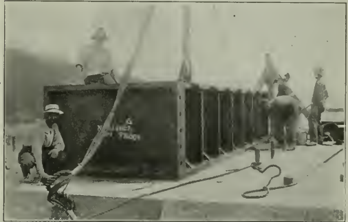
Placing One of the Four 40-Ton Castings That Form the Base of Each of the Main Shoes
