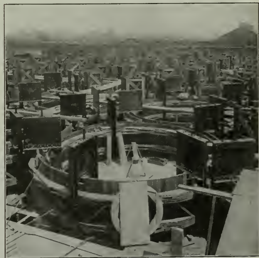
A Portion of the Storage Annex, Showing Yokes Carrying Circular Forms
