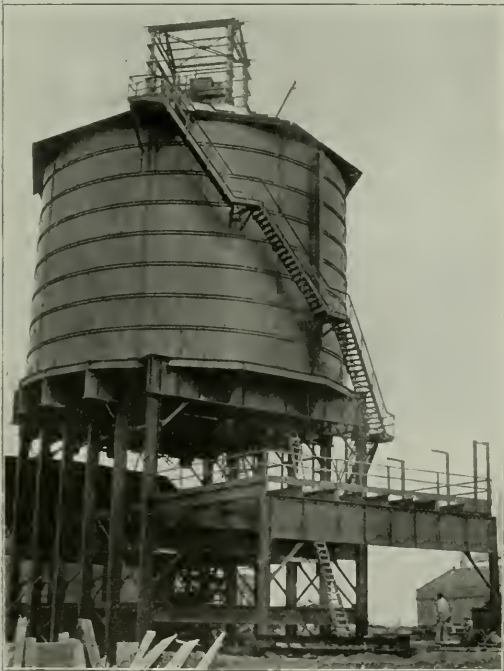
A 2,100-Ton Coal Bunker Lined With Concrete
