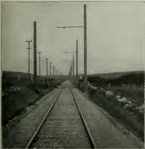
Typical View on Inland Division Showing Track and Single Catenary Construction for a. c. Operation
