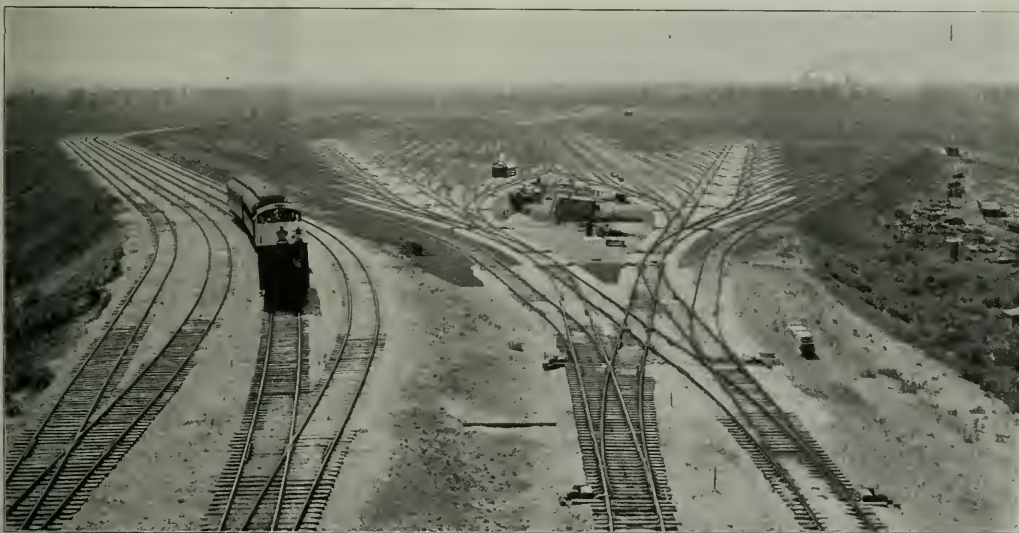
General View of West Half of Clearing Yard from the Hump, with the Four Eastbound Approach Tracks on Left, and Two Hump Tracks Leading to Classification Yards on Right
