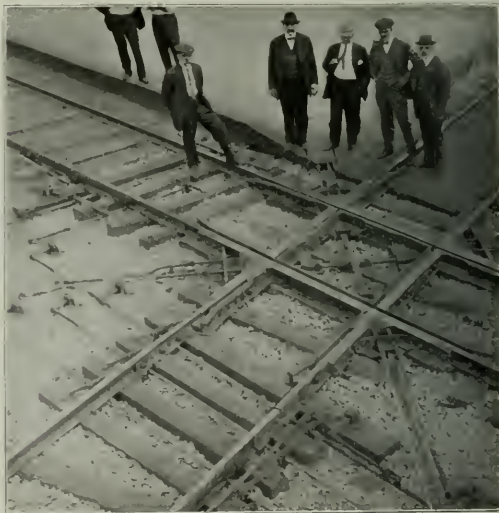
The Eymon Continuous Crossing Installed at Carrothers, Ohio, Showing Interlocking Connections
