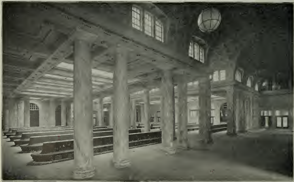
The Main Waiting Room in the New Station, Showing Vaulted Ceiling Over Passageway and Beam and Skylight Ceiling Over Seating Lobbies
