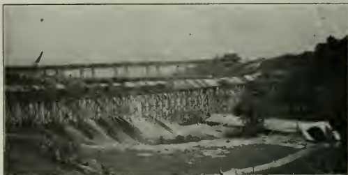
A Side View of the Second Trestle on the First Bench Showing 26-ft. Arch Carrying Bull Creek and the Old Viaduct in the Background
