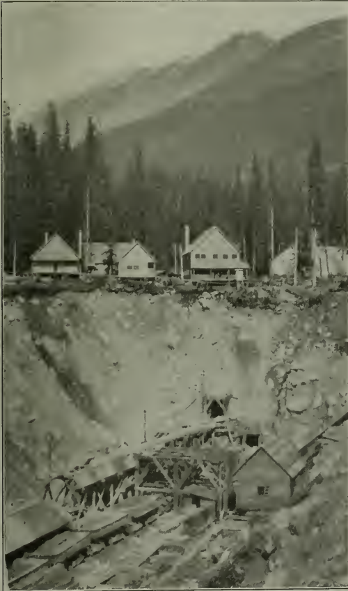
View of West Portal Showing Center and Side Drifts Through Earth. Mouth of Pioneer Tunnel in Background
