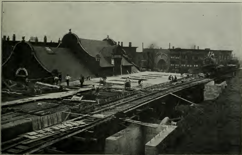
Roof of New Concourse at Euclid Avenue Station Under Construction
