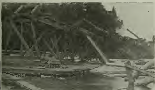
Making Fill Across a Sink Hole at Patterson Lake from a Trestle Carried on a Raft
