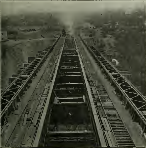
View Looking Back from the Traveler Showing the Four Lines of Rails Carrying the Traveler
