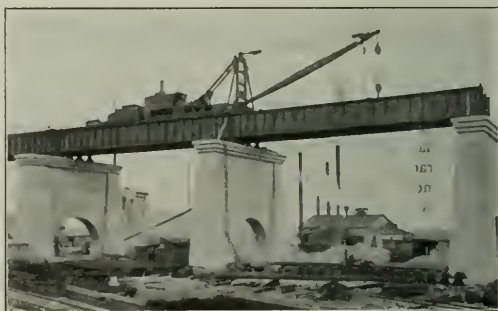
Erecting the Superstructure of the Bronx Viaduct
