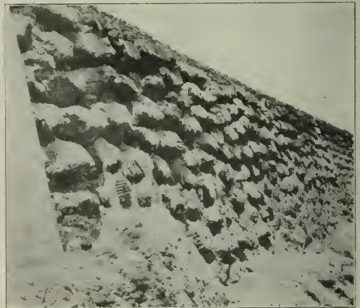
A Retaining Wall Built of Large Pieces of Open Hearth Slag Called "Ciscos"
