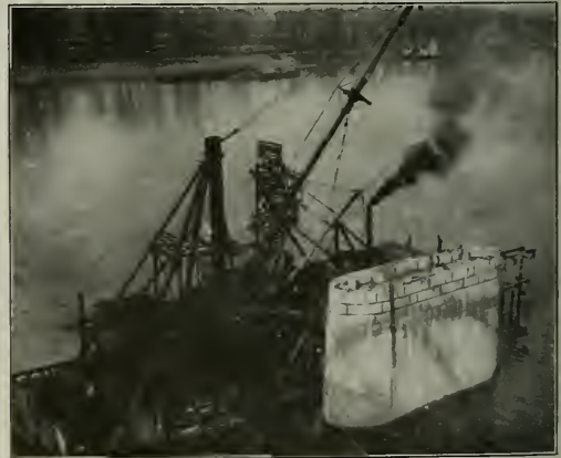
Placing the Upper Courses of Granite Facing on Pier II
