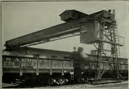
Storehouse and Gantry Crane, Showing Crane Trolley Wires
