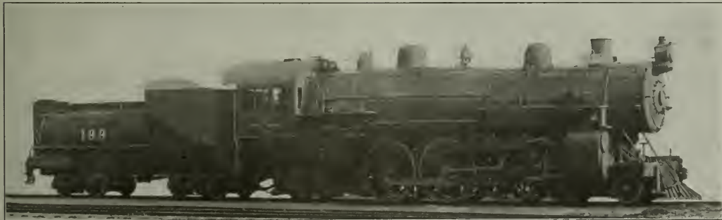
Latest Development of the Pacific Type Locomotive on the Union Pacific
