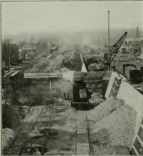
A View Through the Town During the Construction of the Retaining Walls, Showing Sectional Forms and Derrick Car for Handling Material
