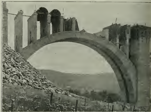
A Construction View at Tunkhannock Creek Showing Forms in Place for Spandrel Walls, Arches and Pilaster
