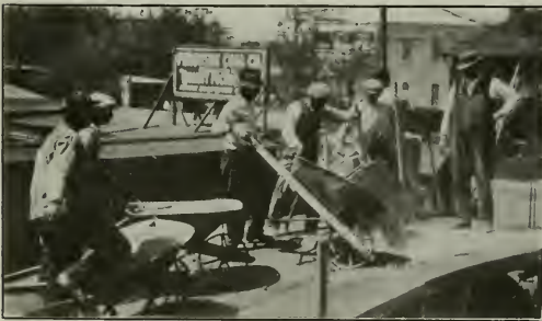
Dumping Bulk Cement Into a Hopper Over the Mixer Showing Absence of Dust
