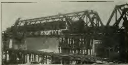
Placing One of the Long Girder Spans with Two Wrecking Cranes
