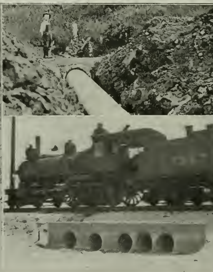
Fig. 2—A 24-in. Corrugated Iron Pipe Replacing a Failed Concrete Culvert
