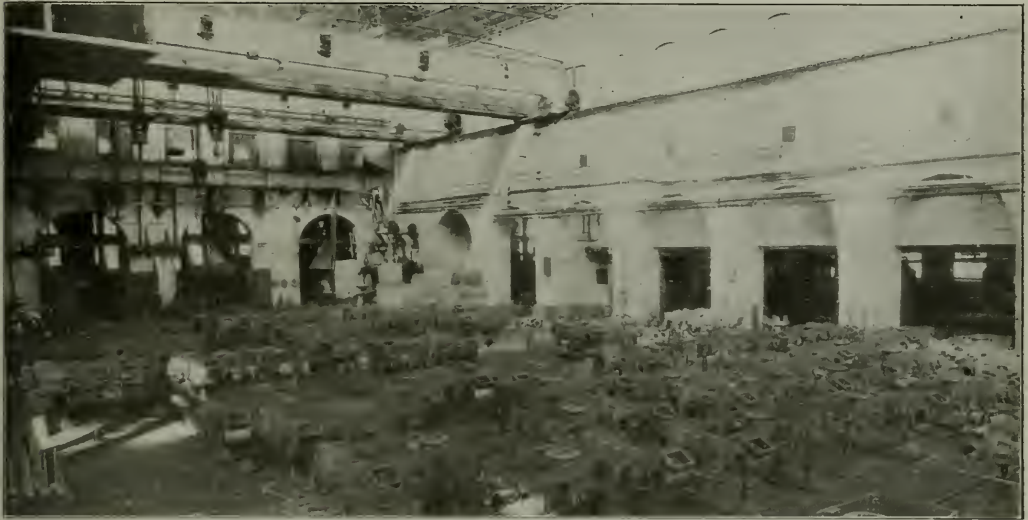
Running Gears of the Pechot Type Locomotives in the Philadelphia Erecting Shop; They Were Shipped to the Eddystone Plant in Automobile Trucks
