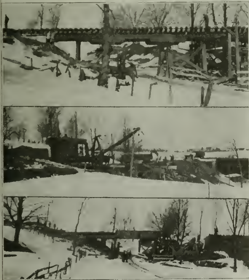
Progress in Erection of Steel Bridge Replacing Timber Trestle
