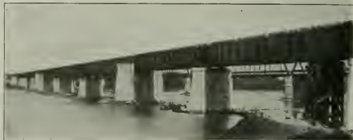
The Completed Deck Plate Girder Structure About 1,550 ft. Long
