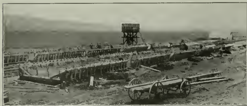
Concrete Slab Yard Near Judith River Viaduct
