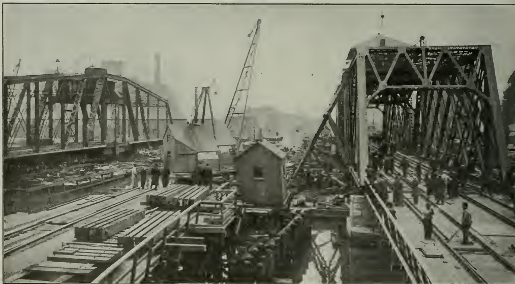
New Bridge in Final Location Before Scows Were Removed; Old Bridge Shown at Left Has Been Moved Downstream from Its Temporary Location
