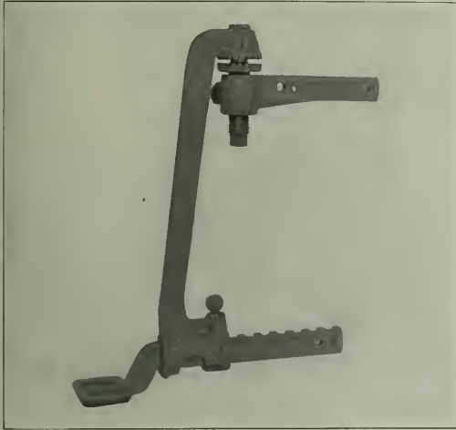
Adjustable Pedal Removed from the Fire Door
