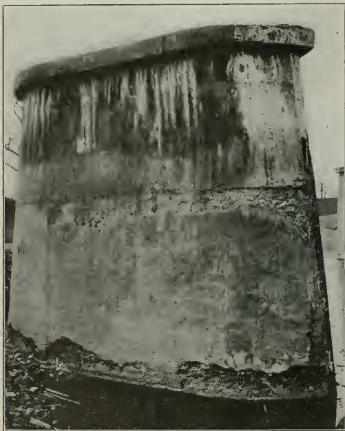
Disintegration of a Concrete Pier in Which Bank Run Gravel From the Pit Shown in the Other Illustration Was Used
