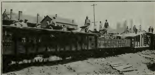
A Work Train, Including Mixer and Material Cars Equipped for Handling Bulk Cement
