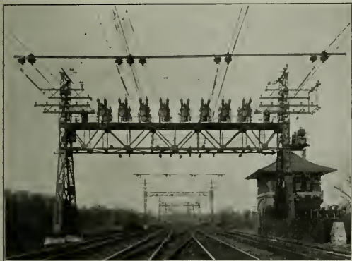
Four-Track Tangent Catenary Construction, Showing Anchor Bridge with Sectionalizing Switches Installed on It,
