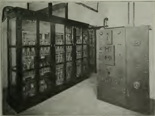
The Automatic Switch Board and Power Board.
