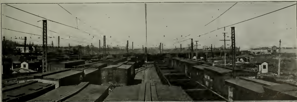
View in Westchester Yard, Harlem River Branch; the Cross Catenary Span in the Immediate Foreground Serves Ten Tracks
