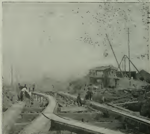
Concrete Mixing Plant and Distributing Tracks for Placing Concrete in Trent Avenue Subway
