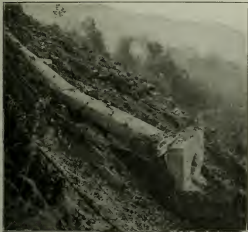
Fig. 5—A 4-ft. Concrete Arch Culvert Destroyed by a Sliding Fill Which Moved It a Distance of 70 ft.
