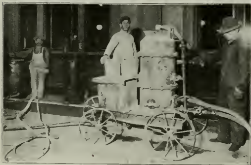
Cement Gun and Two Kelley Sand Blast Machines at Work in Cortlandt Street Ferry Terminal, New York
