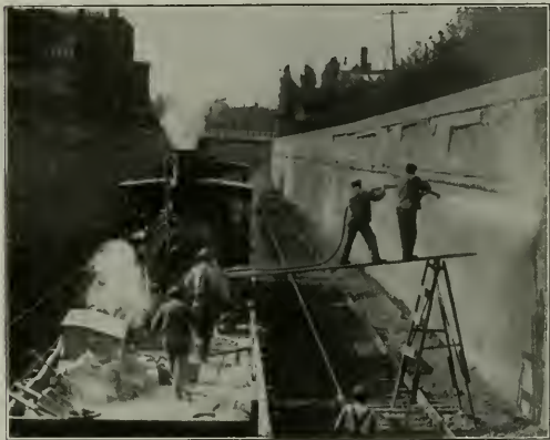
Repairing Retaining Walls on the D. L. & W. with the Concrete Atomizer Taking Steam from the Work Train Engine.
