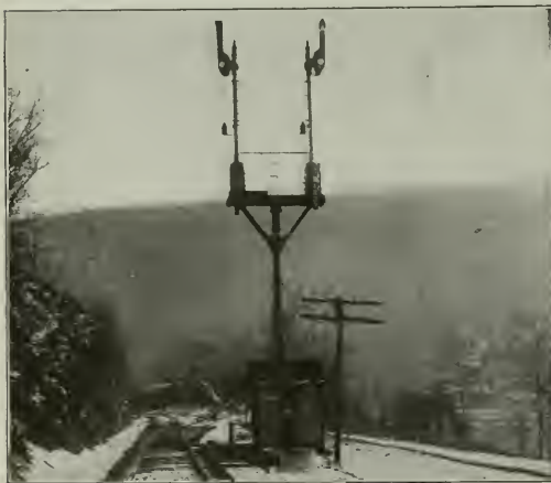
High Post to Make Signal Visible Beyond Hill
