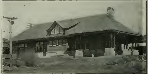
A New York Central Station with Concrete Base Course and Wooden Clapboards Above
