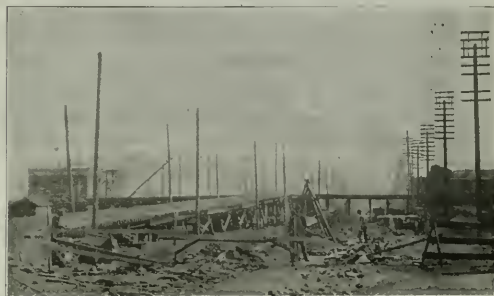
A Portion of the Temporary Trestles Carrying Street Cars and Team Traffic During the Regrading of Trent Avenue
