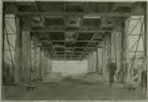
A Portion of the Main Deck Showing the Track Supports on the Movable Deck Overhead
