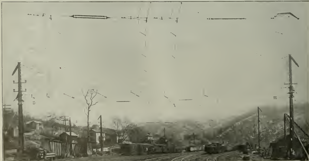
Fig. 7—Cross Catenary Construction Used in the Yards of the Norfolk & Western at Flat Top—Notice the Small Amount of Obstruction Offered by This Type of Construction
