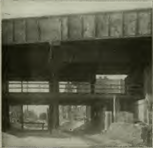
The Three Levels at Seventy-Ninth Street—Rock Island Above, Western Indiana in the Middle and the Street Partially Excavated Below
