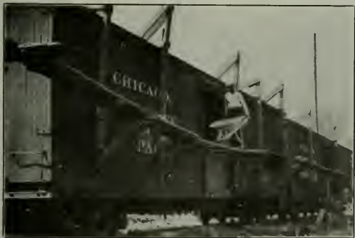
Runway for Unloading Bulk Cement from a Box Car Hung by Brackets from the Roof
