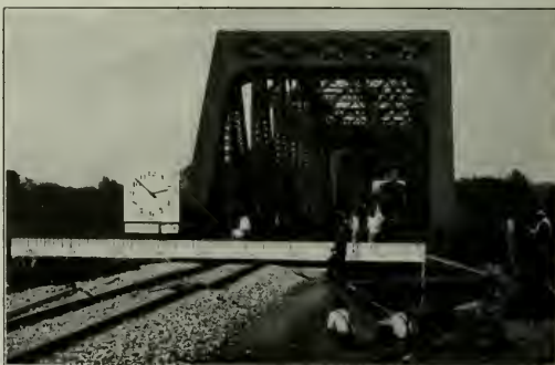
Moving in the New Bridge Showing Clock and Telltale for Indicating the Position of the Span and in the Distance One of the Two Derrick Cars Which Furnished the Power
