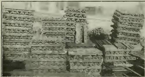
A Pile of Reclaimed Angle Bars Illustrating the Possible Saving from Scrap
