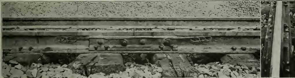
A Side and Top View of the Pennsylvania's New Anti-Creeping Tie Plate Extending Over Four Ties
