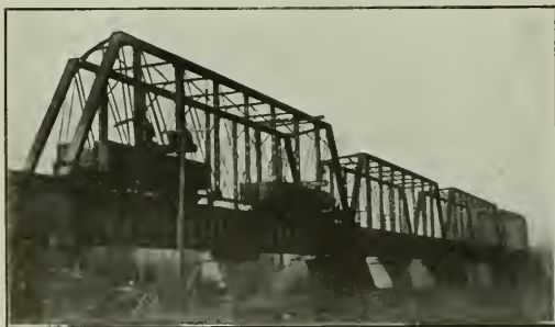
Raising the First Truss Span on Cars, Showing the New Girder Spans in Place
