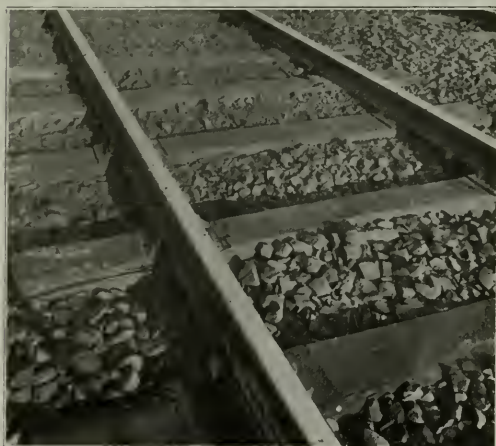
Effects of a Derailment Where Screw Spikes Were Partially Used. Weber Joint Badly Damaged. All Cut Spikes Had to Be Replaced, But Original Screw Spikes Show No Damage
