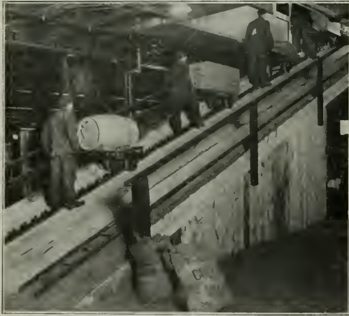
Handling Freight to the Upper Warehouse Floor of the Pere Marquette Station in Detroit on an Inclined Elevator.
