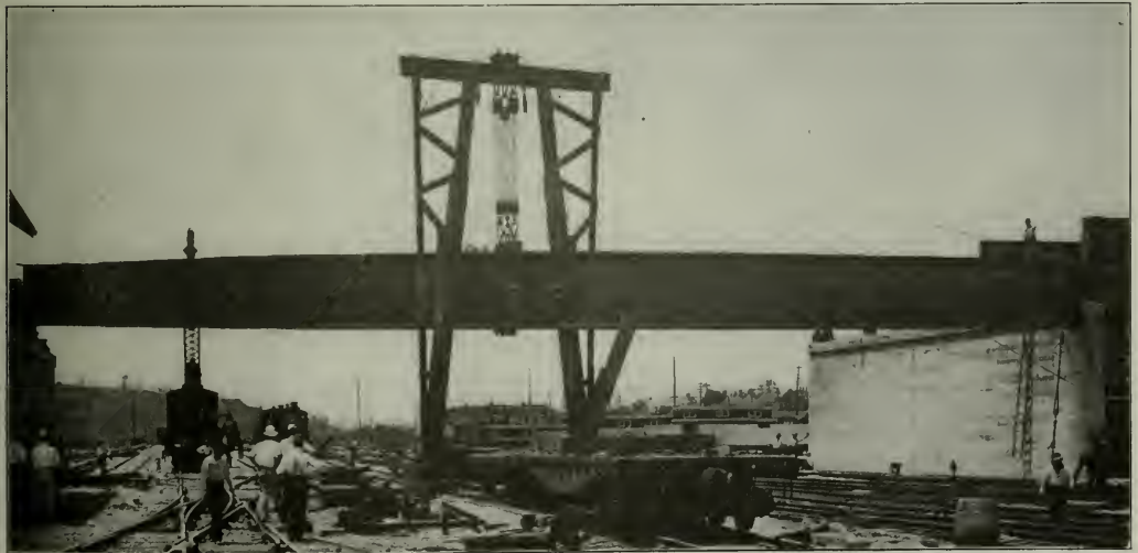
Erecting a 127 ft. 5 in. Girder at Pennsylvania Avenue
