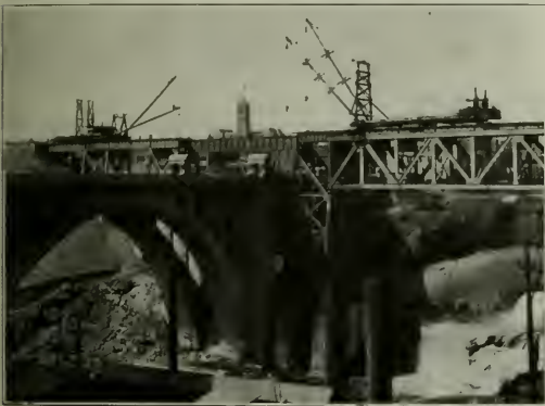
Placing the Last Span in the Structure Over the Monroe Street Arch and the Spokane Falls
