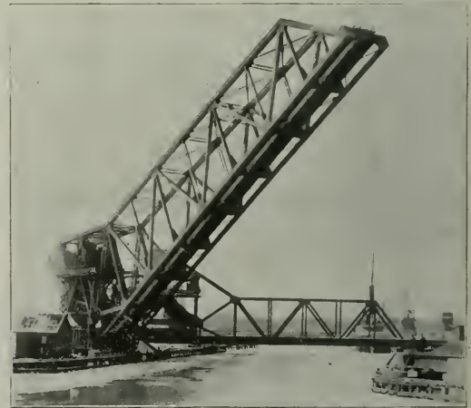
Two Scherzer Rolling Lift Bridges Operated from One Controller House.
