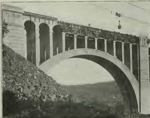
The End Span of the Tunkhannock Viaduct Showing the Pilasters at the Piers and the Spandrel Arches Partially Completed
