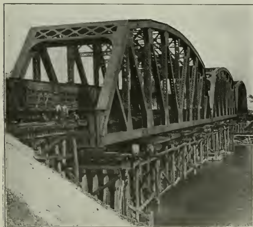
New Bridge Completed on Falsework 44 ft. 9 in. from Permanent Location
