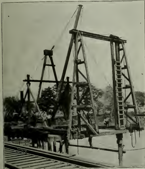
Special Pile Driver Placing Falsework Bents 30 Feet Ahead of Last Bent Driven and Designed to Drive Six Piles at One Setting
