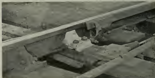
The New Adjustable Rail Brace in Track.
