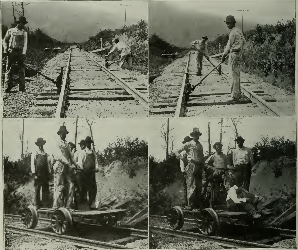
Pictures Used by the Carolina, Clinchfield & Ohio in Emphasizing Safe and Unsafe Methods for Trackmen. Above—the Use of Jacks; Below—the Arrangement of Men on a Hand Car
