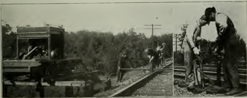
Two Men Operating the Pneumatic Tampers
