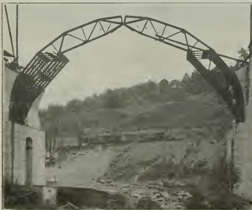
Erection of the Steel Centers for One Span at Martin's Creek in Progress Showing Details of Crown Connection and Adjustable Members in the Top Panel of Each Semi-Truss
