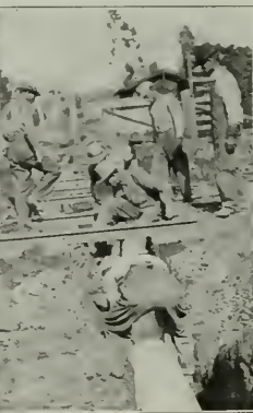
Fig. 10—A Gang Installing an Ingot Iron Corrugated Pipe Culvert Under the Tracks of the Southern Pacific
