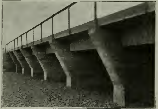
New Type of Concrete Pier and Slab Construction
