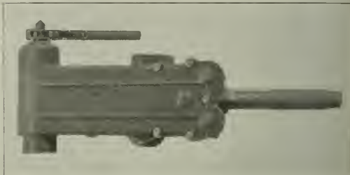
Drill for Use in Confined Spaces
