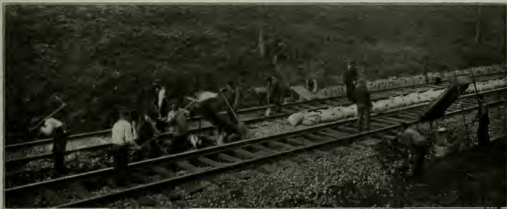
Cleaning Stone Ballast with Screens
