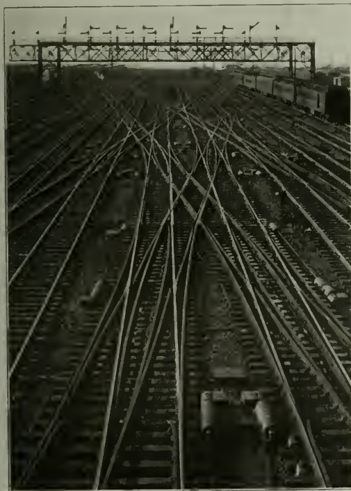
Looking West Through the Throat of the Yard Showing Double Crossed Ladders
