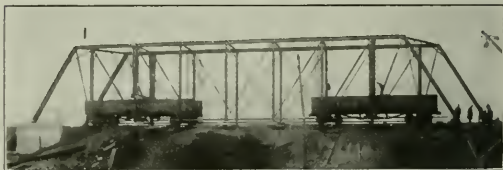
Lowering One of the Truss Spans from the Cars to Blocking Under the Panel Points
