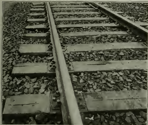
Chestnut Ties Placed in Tangent Track Carrying 12,000,000 Tons Per Annum in 1912. Ties Adzed and Bored Before Insertion, and Are Still in Excellent Condition
