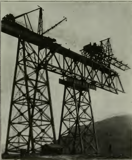
False Work Tower and Girder Caps Used in Erection of Snake River Viaduct
