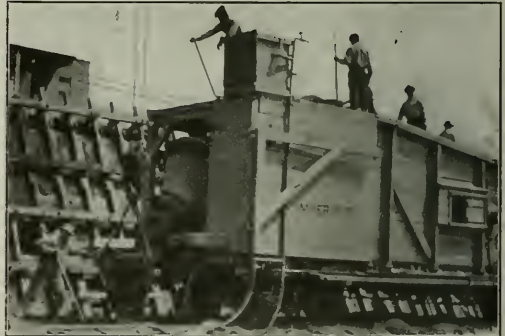
The Mixer in a Bulk Cement Plant Discharging Into Placing Buckets, One Mix Every 45 Seconds or 220 Yards per 10 Hour Day
