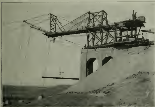
Traveler Placing the First Steel at Judith River Viaduct
