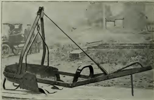
The Bucket Used with the "Economy" Excavator.
