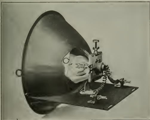
Method of Focusing the Lamp in the 14-in. Headlight Case
