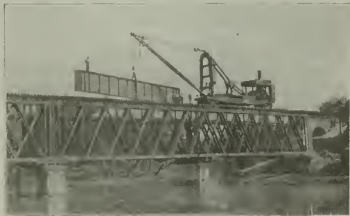
Replacing Howe Trusses with Deck Girder Spans on the New Haven
