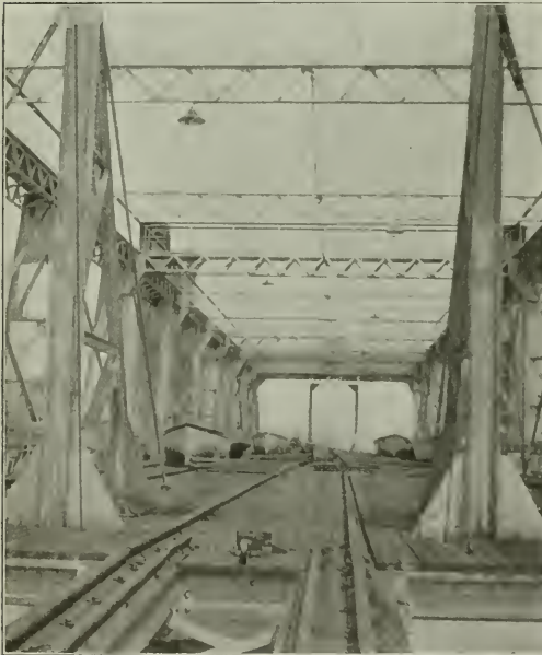
Looking Down One of the Tracks on the Movable Car Deck
