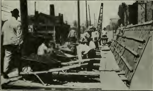
Unloading Material to Wheelbarrows Handled Over Double Gangways to Mixer Providing Runway in Each Direction
