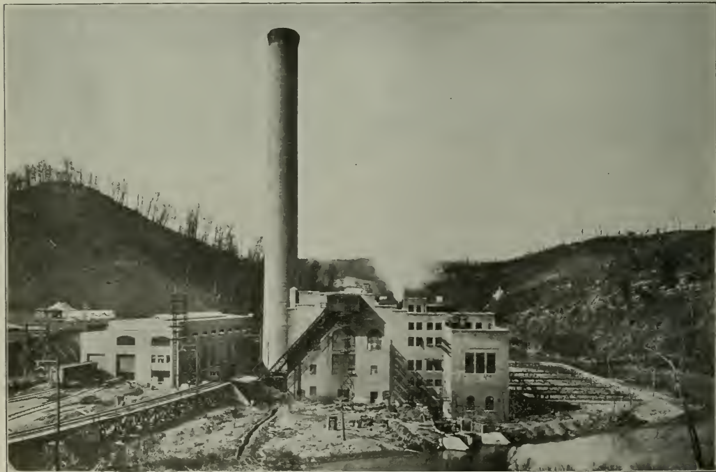
The extension or wing at the right end of the power house is a substation and the structures for carrying the outgoing feeders are shown. Fig. 10—General View of Power House from the West, Showing the Inspection Building to the Left, Intake Canal and Cooling Pond to the Right
