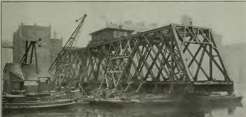
Floating the Milwaukee River Bridge on Four Scows Showing Diagonal Bracing for Distributing Loads on Two Main Scows
