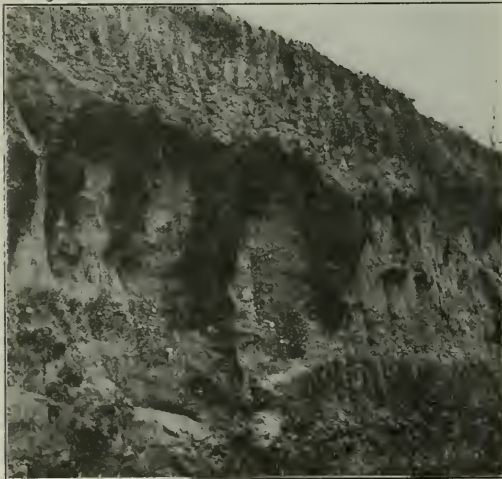
The Working Face of a Gravel Pit Containing Pockets of Clay and Loam
