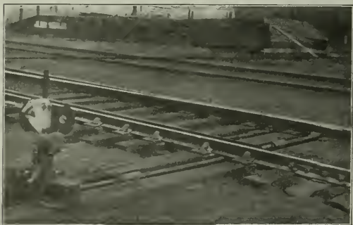
A Head Rod on the G. R. & I. Equipped with the Hardick Locked and Covered Turnbuckle
