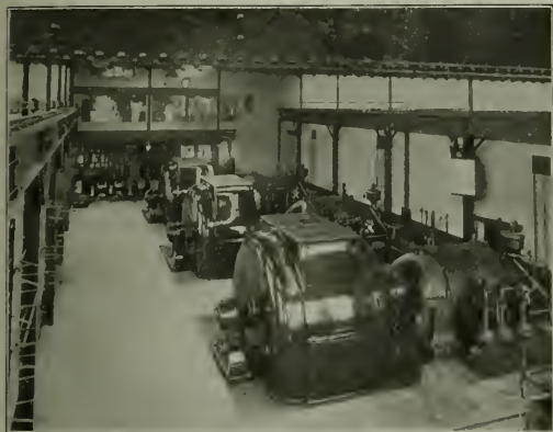
Fig. 11—View of Turbine Room from the West End Showing the Main Generating Units. The Operating Gallery is on a Level with Crane Track
