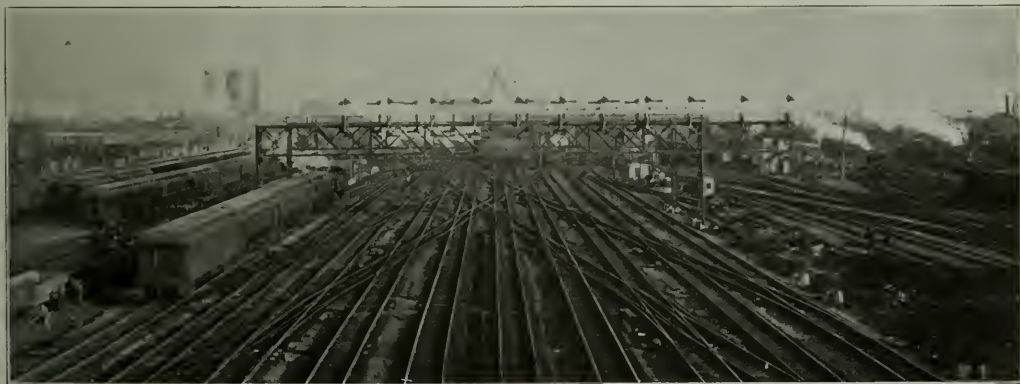
The Throat of the Yard Looking Towards the Station The New Signal Tower on the Right Is Partially Hidden by the Signal Bridge. The Car Repair Shed and Shop Buildings Are Shown on the Left
