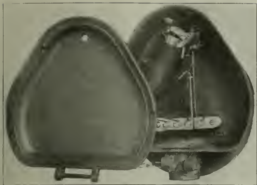
Direct Current Crossing Bell, Complete.
