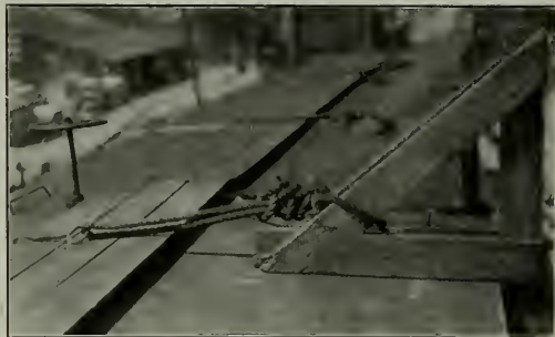
Wooden Bracket on Roof of Car Supporting a Runway
