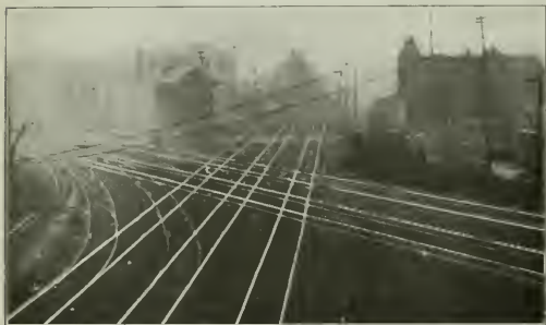
Looking South Over the Seventy-Ninth Street Crossing Before the Elevation of the Tracks of Either Road Showing Tem- porary Diversion South of Crossing
