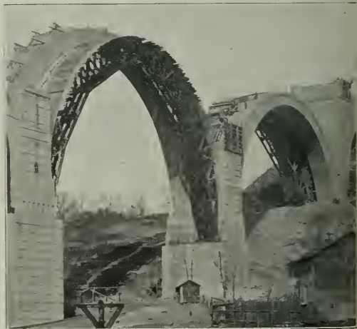
Two Spans of the Tunkhannock Viaduct in Each of Which One Rib Has Been Finished and the Centers Are Now in Place Under the Second Rib
