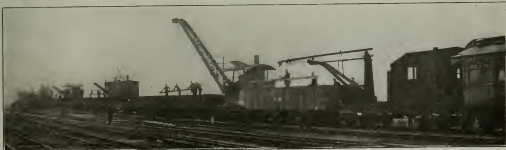
A Work Train on the Lehigh Valley with Six Rail Loading Machines
