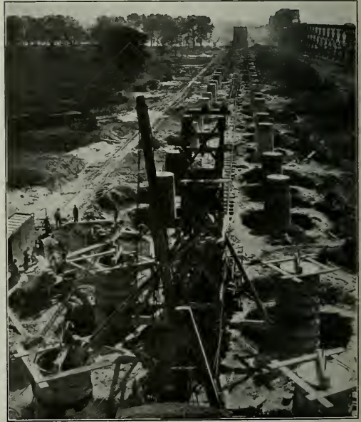
Placing Concrete in Steel Pedestal Forms for Western Approach Viaduct
