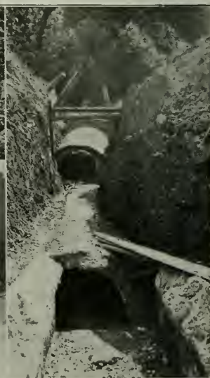
Fig. 4—Failure of a Concrete Culvert under Shifting Load, Later replaced by a Corrugated Iron Pipe
