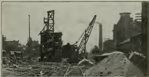
Portable Mixer Outfit Used in Placing Concrete Retaining Walls, and the Derrick Car Used to Handle Material from Cars to Hopper Bins
