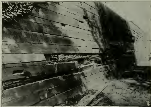
Condition of Wooden Bulkhead Replaced by the Concrete Crib Shown Below
