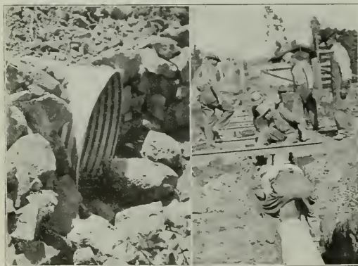
Fig. 9—A 48-in. Pipe Set on a 20-deg. Slope under a 25-ft. Rock Fill Showing Typical Boulders Passing Through this pipe
