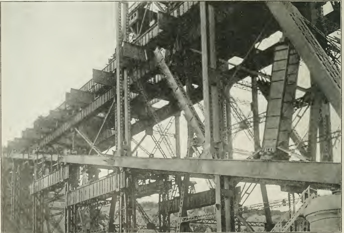
View of the South Shore Span Showing the Floor Supported on the Inside Falsework and the Bottom Chord on the Special Outside Falsework
