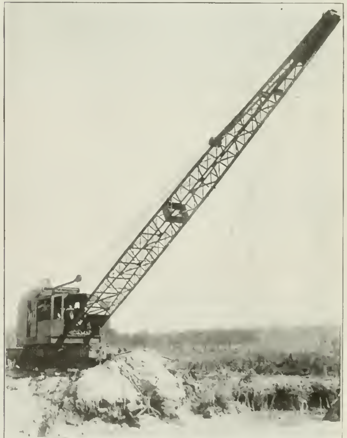
A 35-Ton Crane with a 70-ft. Boom Equipped with a 1 1/2 Yd. Drag Scraper Bucket
