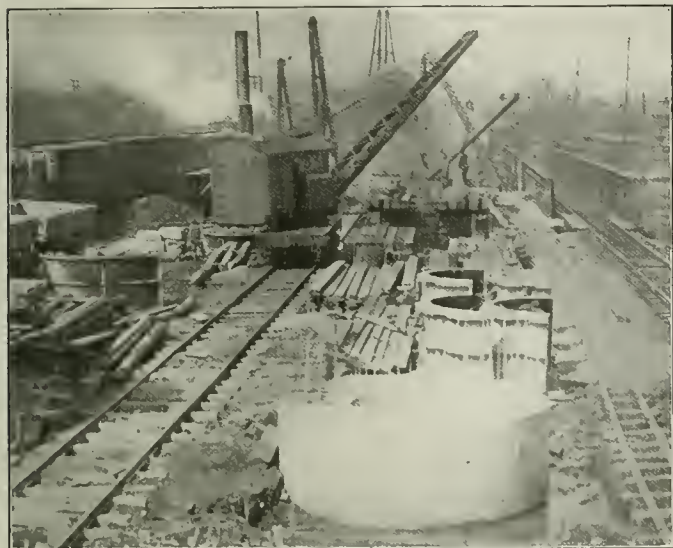
General View of Bridge Site, Showing Completed Cylinder Pier and Diverted Westbound Track
