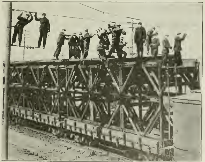
Special Car for Erecting Catenary Work; Removable Outriggers Make it Possible to Work Over Track Alongside Without Interruption to Traffic
