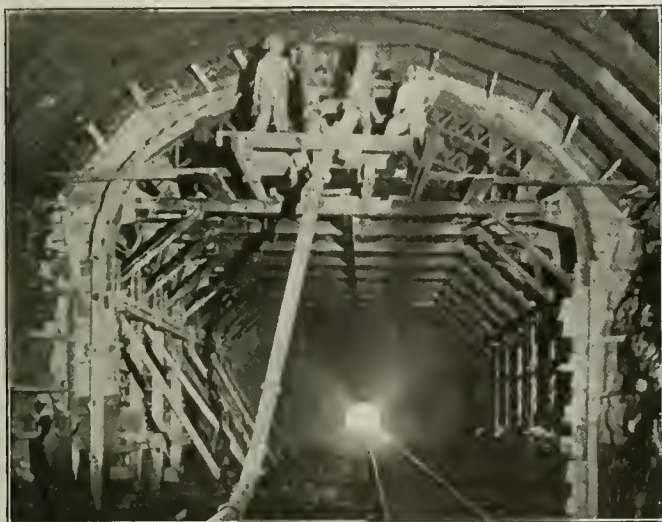
View Showing "Y" in Delivery Pipe, Forms and Roof Timbering
