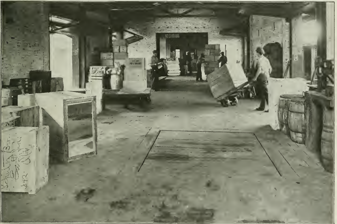
Wood Block Floor in South Chicago Freight House of Pennsylvania Lines, Laid in 1912
