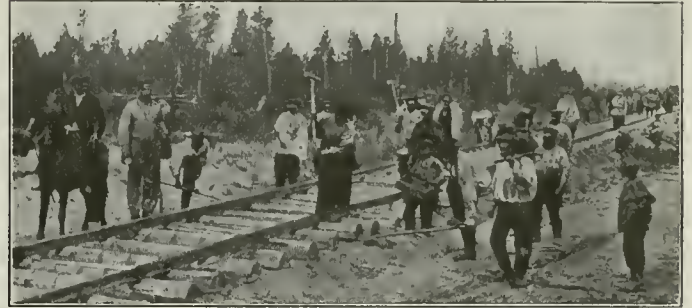
Laying New Track on Half-Round Ties
