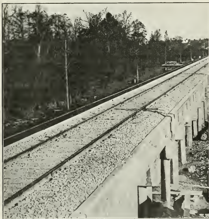
A Portion of One of the Illinois Central Concrete Trestles, Showing the Solid Ballasted Deck
