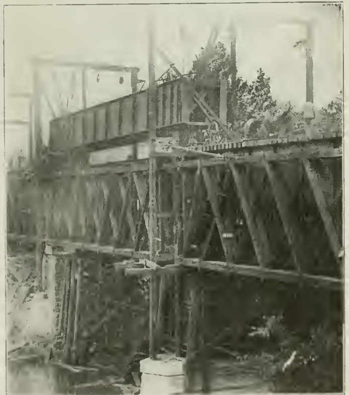
Renewing a Howe Truss with Two Girder Spans. The New Span on the Right Is in Place, the Other Is Supported from Overhead Bents During the Removal of the Old Floor System
