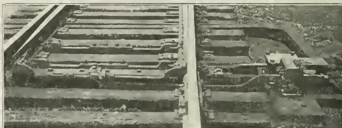
Fig. 6.—Garber Switch and Lock Movement
