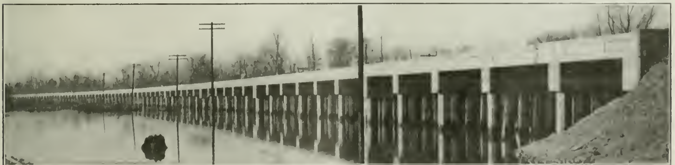
One of the Sections of Reinforced Concrete Trestle, Built on Concrete Pile Bents, in Double Tracking the Illinois Central North of Memphis
