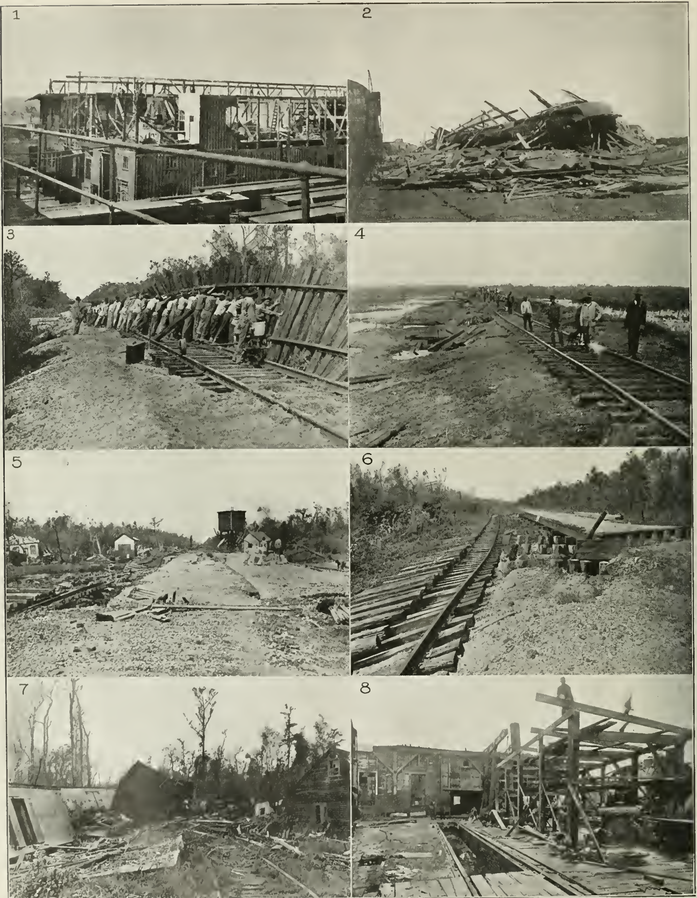
1) and (2) Sunset-Central Lines Car Shop and Paint Shop at Algiers, La. (3) and (4) Illinois Central Main Line Between Manchac and Hammond After Repair Work was Begun. (5) Pump Station and Tank at La Branch, La., Where Several Houses were Washed Away. (6) Showing Track Washed off Trestle and Turned Upside Down. (7) Showing Cars Washed off Track. (8) Government Yard Roundhouse After the Flood
