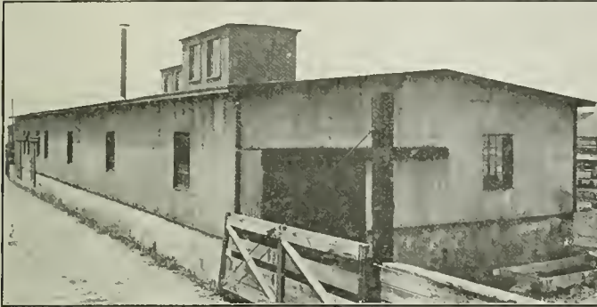
New York Central Sheep Sheds at Buffalo Covered with Corrugated Asbestos Sheets
