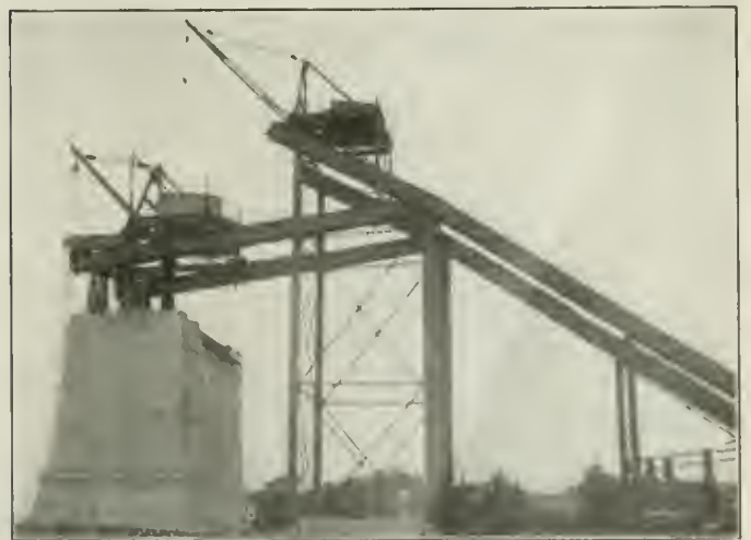
West Abutment of Hell Gate Arch, Showing Stayback Structure
