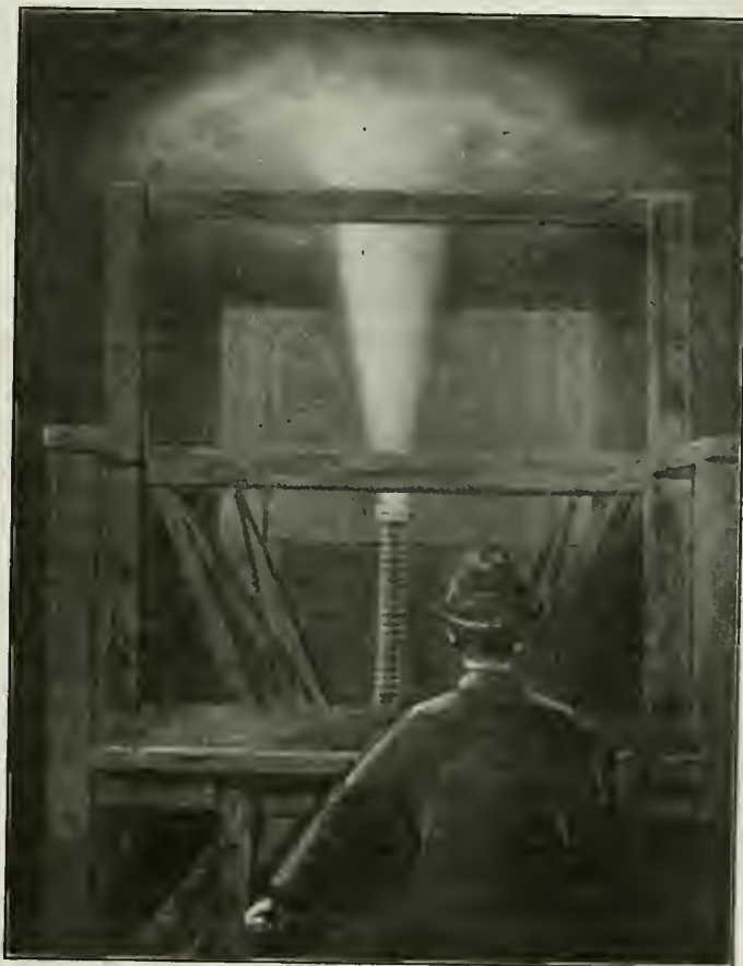
Placing SteamJetted Concrete on the Tunnel Lining
