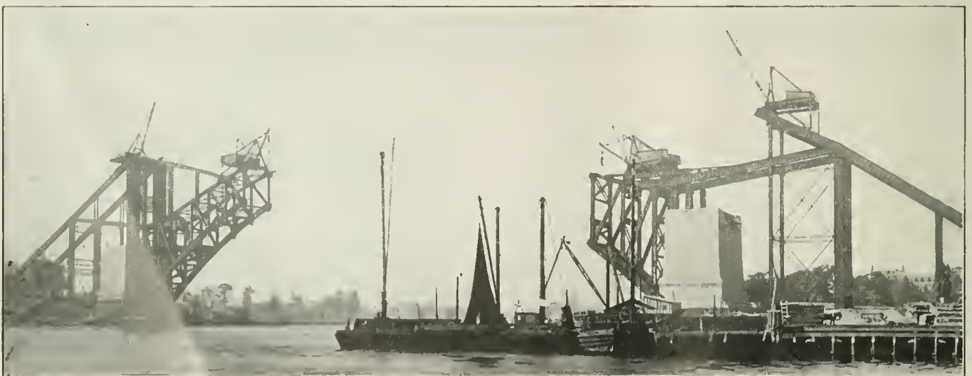
Progress on the Erection of the Hell Gate Arch. Second Set of Ties in Position on the East Side
