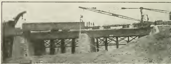
Placing 70-ft. Through Girder with Wrecking Crane and Derrick Car
