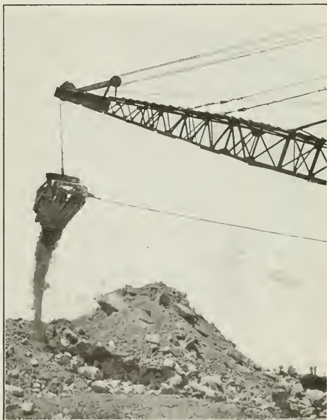
Dumping Beyond the Normal Radius of the Machine
