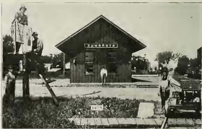
Sign Painting Crew with Outfit Motor Car and Crossing Sign Scaffold
