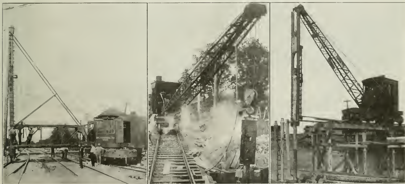
Methods of Driving Piles with a Locomotive Crane
