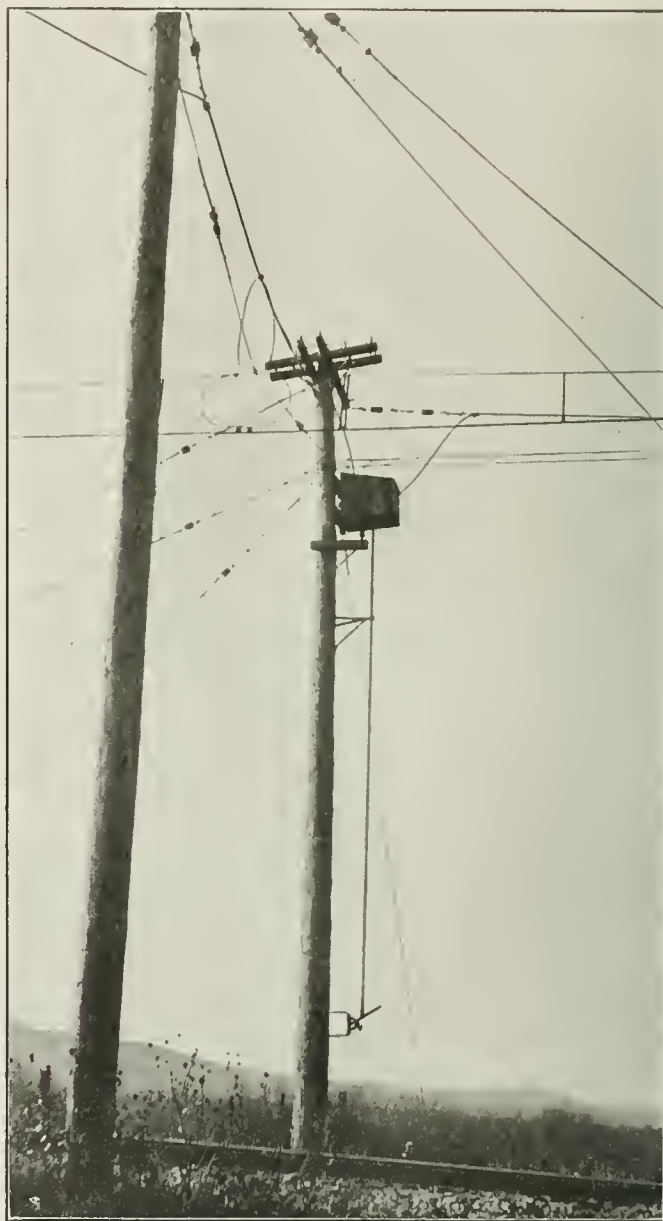
A Sectionalizing Switch Beyond the End of a Passing Track
