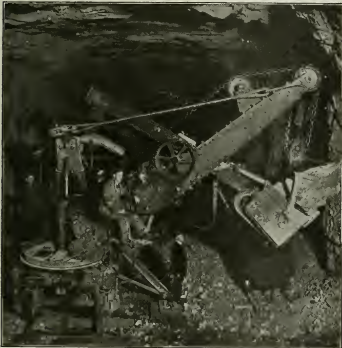
Shovel Removing the Bench Rock
