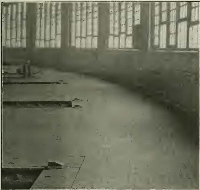
Installation of Wood Blocks in Lackawanna Roundhouse at Elmira, N. Y.
