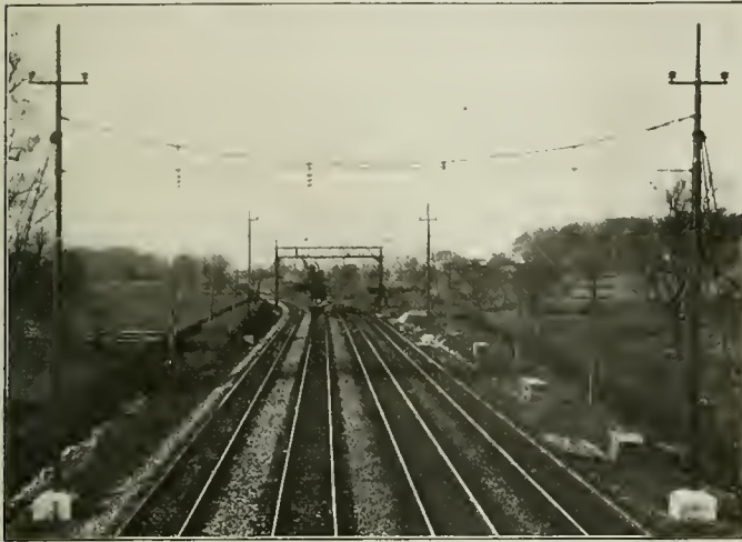
Tubular Cross-Catenary Bridge Before Longitudinal Wires Were Erected
