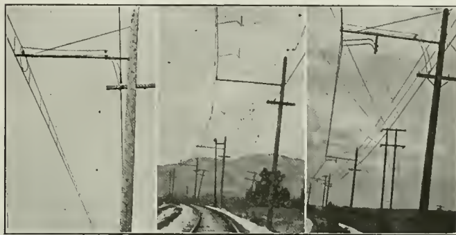
Standard Trolley Construction—Trolley Construction on Tangents with Feeder Tap (left); "Pull Overs" on a Heavy Curve (center); Steady Braces and Feeder Tap on Light Curve (right)
