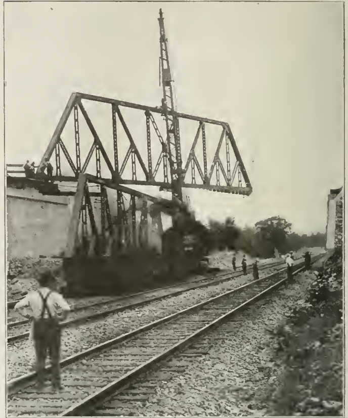
A 60-Ton Erection Crane with a 75-ft. Boom Handling a 132-ft. Highway Truss Weighing 28 Tons
