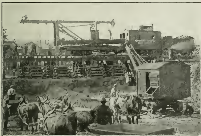
Replacing Tie Cribs with Pile Trestle at Subway
