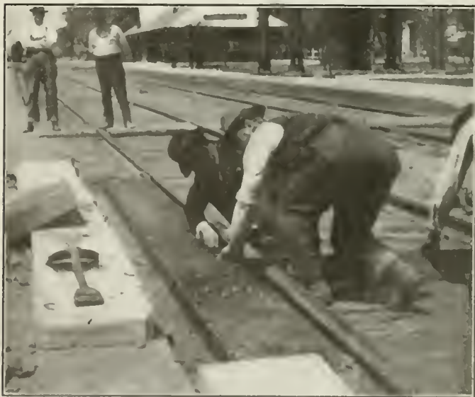
Preparing to Place the Concrete Crossing
