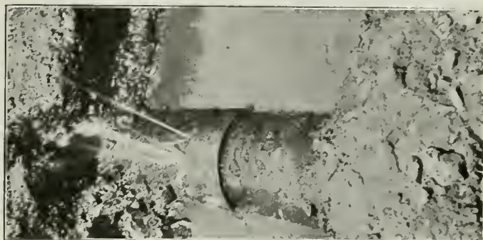
Leakage from a Buried Water Main
