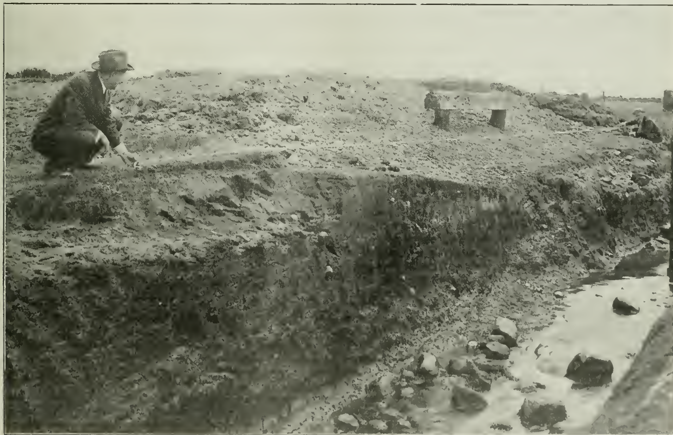
Excavation Across Embankment Showing Extent of Settlement
