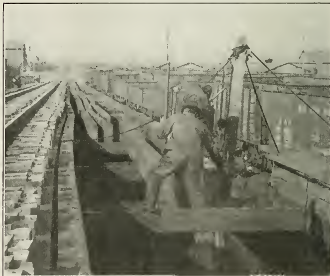
Hoisting New Stringers to Scaffold Alongside Trestle
