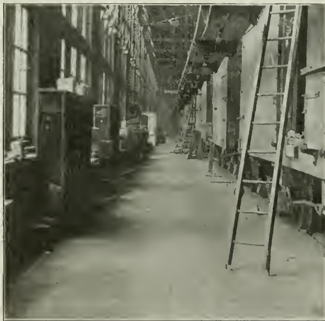
Creosoted Block Floor in Lackawanna Car Repair Shops at East Buffalo
