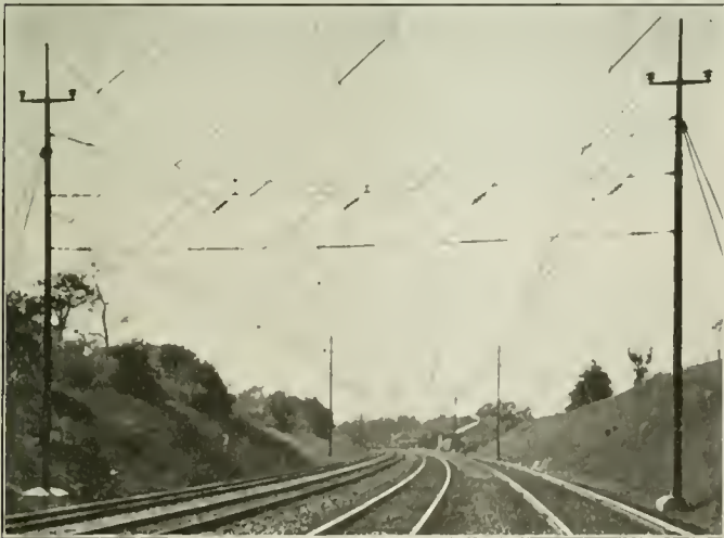
Catenary System Over Curved Track
