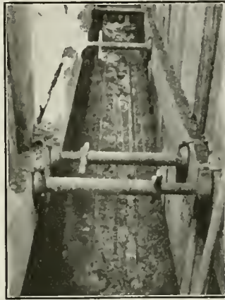
Fig. 5—Re-enforcing Bars in Bottom
