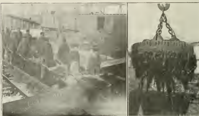
Handling 3,175 Lb. of No. 2 Wrought Iron Scrap by Hand and with a Magnet
