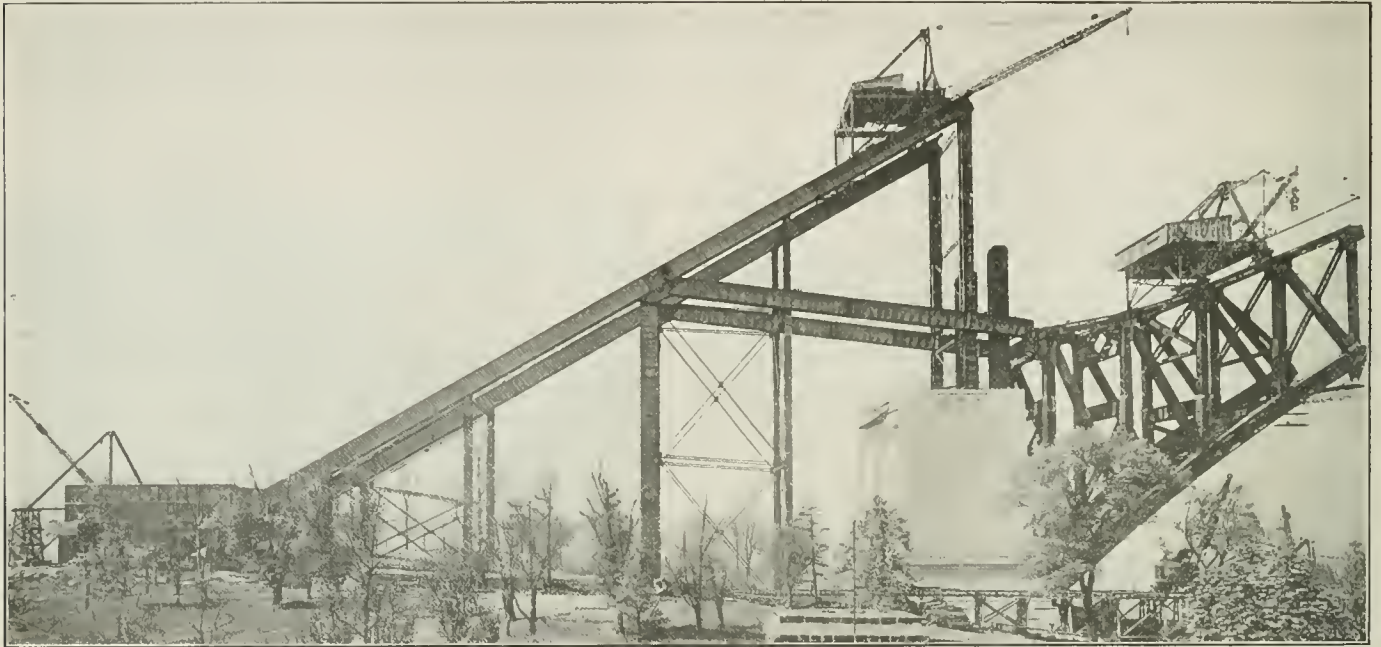
Hell Gate Arch, East Abutment and Backstay. First Set of Ties in Position
