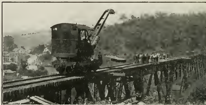
Renewing Ties on a Branch Line Viaduct
