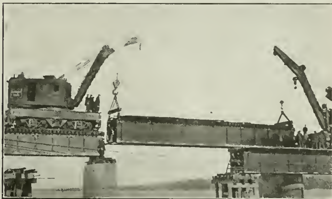
Moving Girder Spans from Temporary Piers to New Piers
