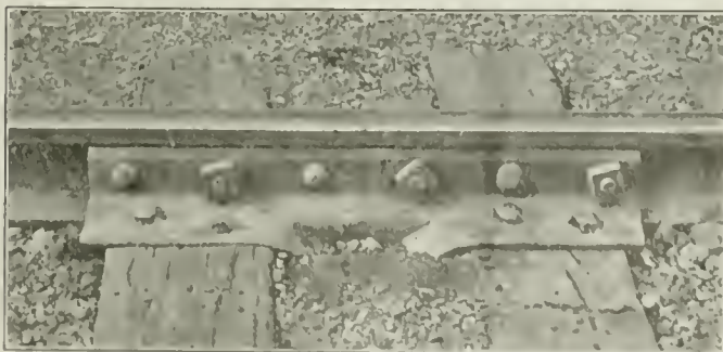
An Application of the Ballou Bolt Nuts to a Depending Flange Joint on the Norfolk & Western
