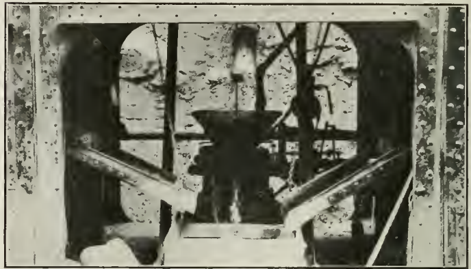
Central or Working Chamber of the Car Showing the Skip in the Foreground, the Mixer in the Rear and the Chutes on the Sides
