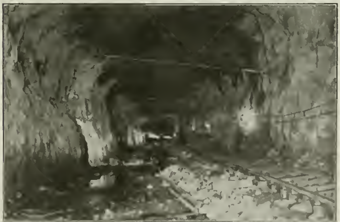
Tunnel Excavated to Full Section—Before Lining
