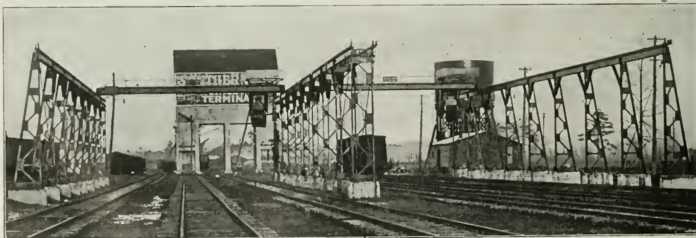
The Cinder Pits, with Craneways and Overhead Traveling Grab Buckets. Coaling Station in the Background
