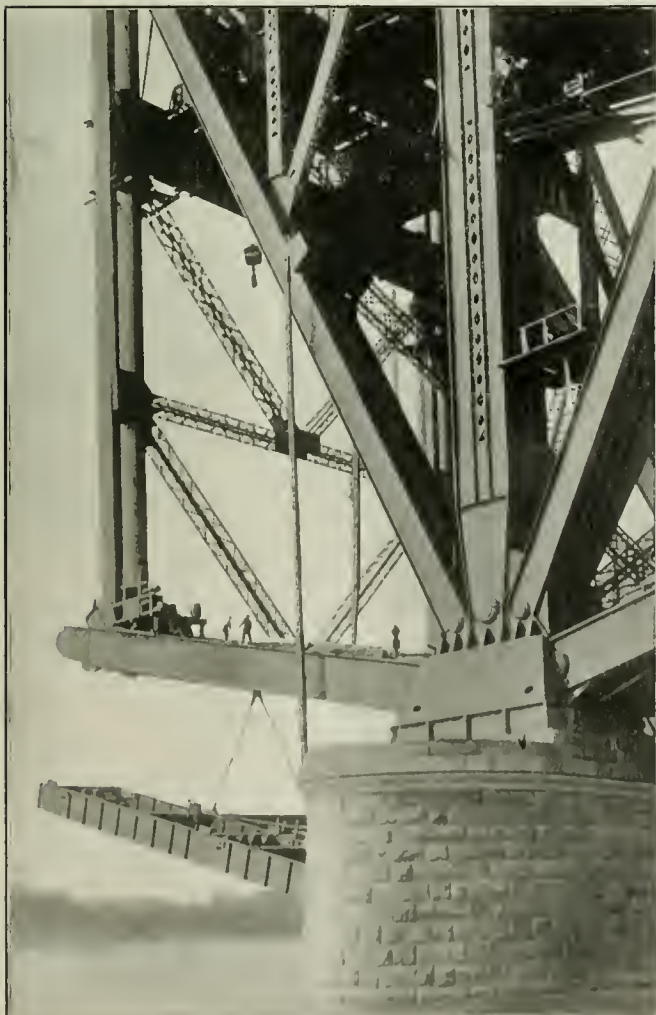
View of the North Cantilever Arm, Showing the Process of Moving the "Flying Bridge" Forward One Panel
