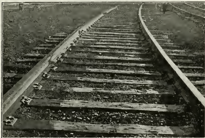
An Installation of Thomas Rail Anchor Tie Plates at Kansas City, Mo.
