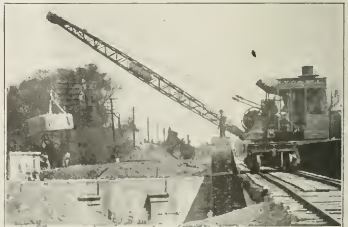
N. Y. C. & St. L. Crane on Cleveland Track Elevation Work Handling Excavated Material in a Skip
