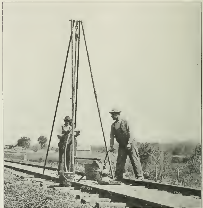
Wash Boring Outfit to Determine the Amount of Settlement of Embankment
