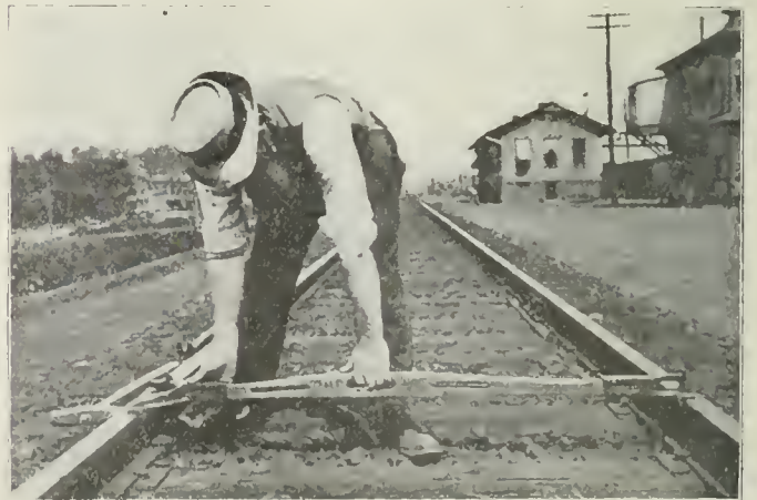
CORRECT WAY TO USE TRACK GAUGE Fig. 5
