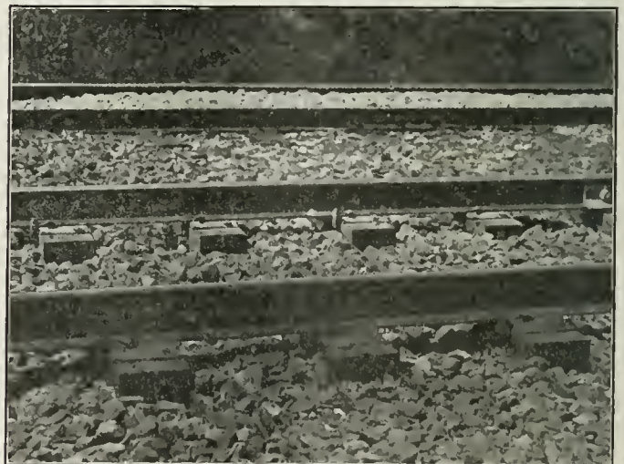
Standard Steel Ties in the Pennsylvania Tracks Near Parkesburg, Pa.
