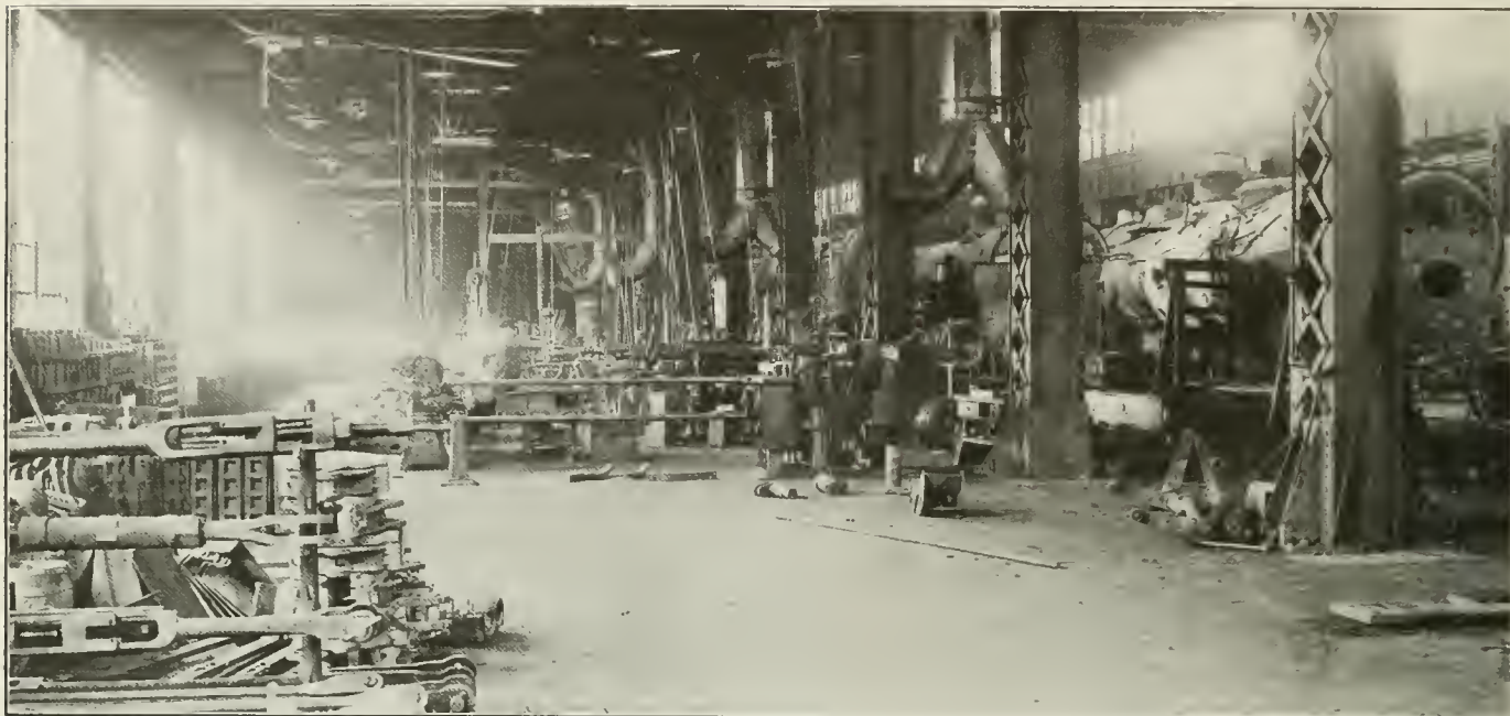
Block Floor in Locomotive Erecting Shop of Michigan Central at Jackson, Mich.
