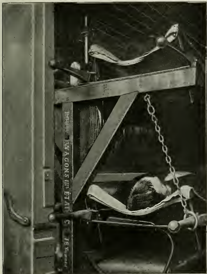
A Surgeon's Device for Carrying Wounded That Avoids Rebuilding Continental Passenger Cars
