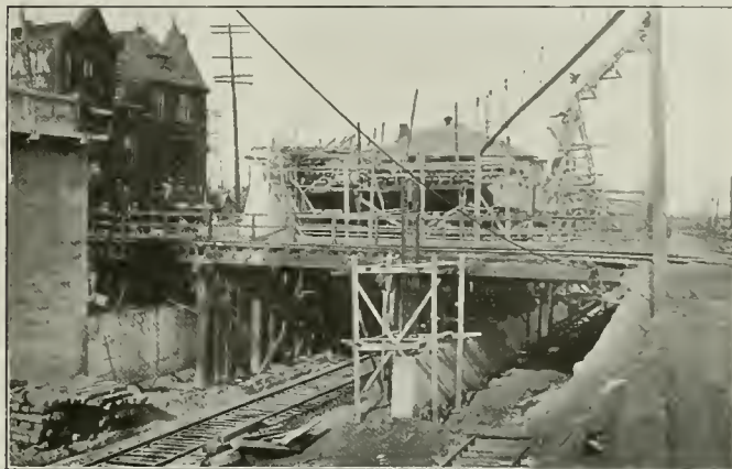
Construction View. Temporary Crossing of Street Car Tracks Over Missouri Pacific Westbound Tracks and at Grade with Missouri Pacific Eastbound Track
