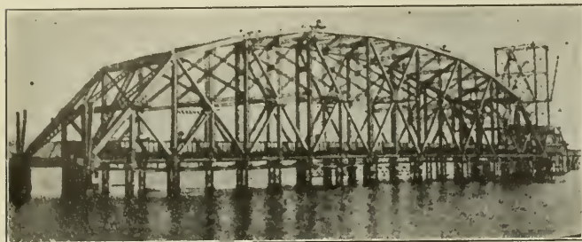
The Completed Suspended Span As Erected Three Miles Below the Site of the Bridge. The Staging Is Still in Place
