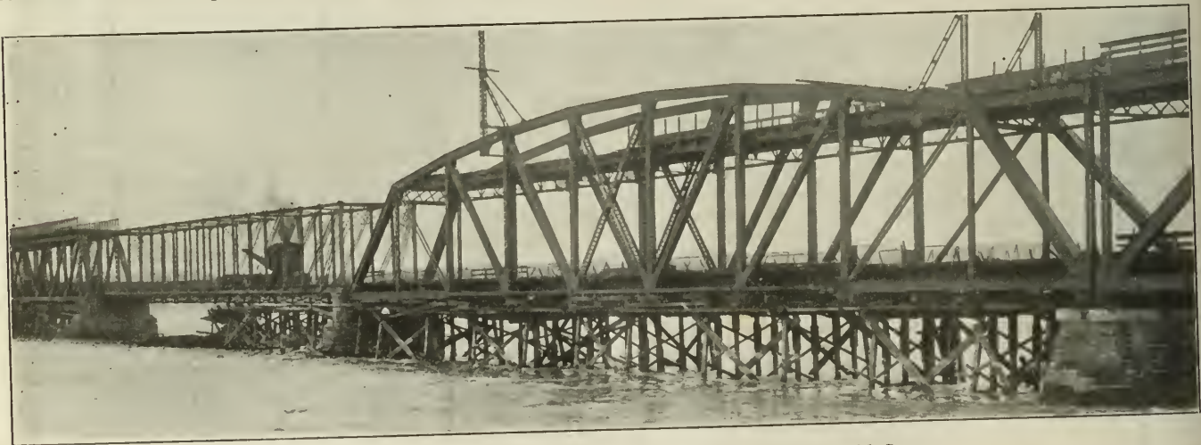
Locomotive Crane Placing False Work Under the Last Old Span
