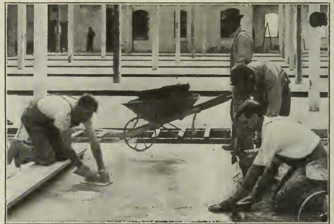
Laying Mastic Floor in Car Repair Shop, Chicago & North Western, Chicago, Ill.
