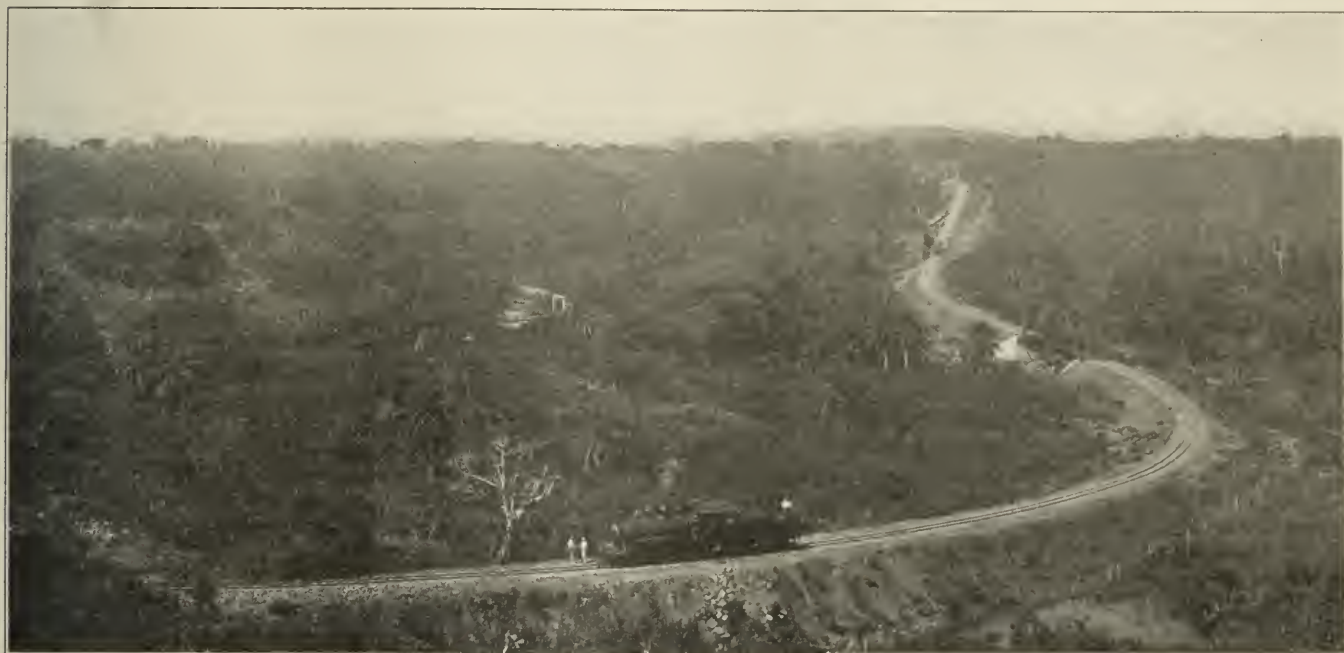
Crossing the Rio Grande Valley on the Boquete Line with Maximum Grades of 5 per cent and Curvature of 12 deg.
