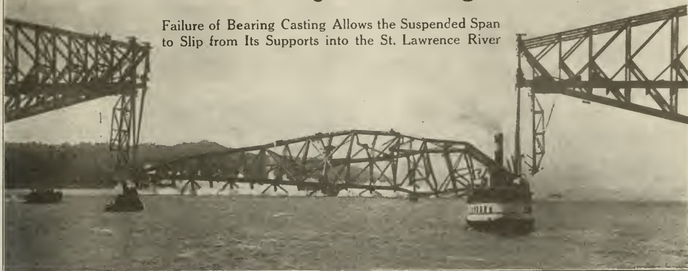
The Span at the Moment of Collapse, Showing the Southwest Corner Under Water Before the Other Three Had Left Their Supports. Photo copyrighted by International Film Service.
