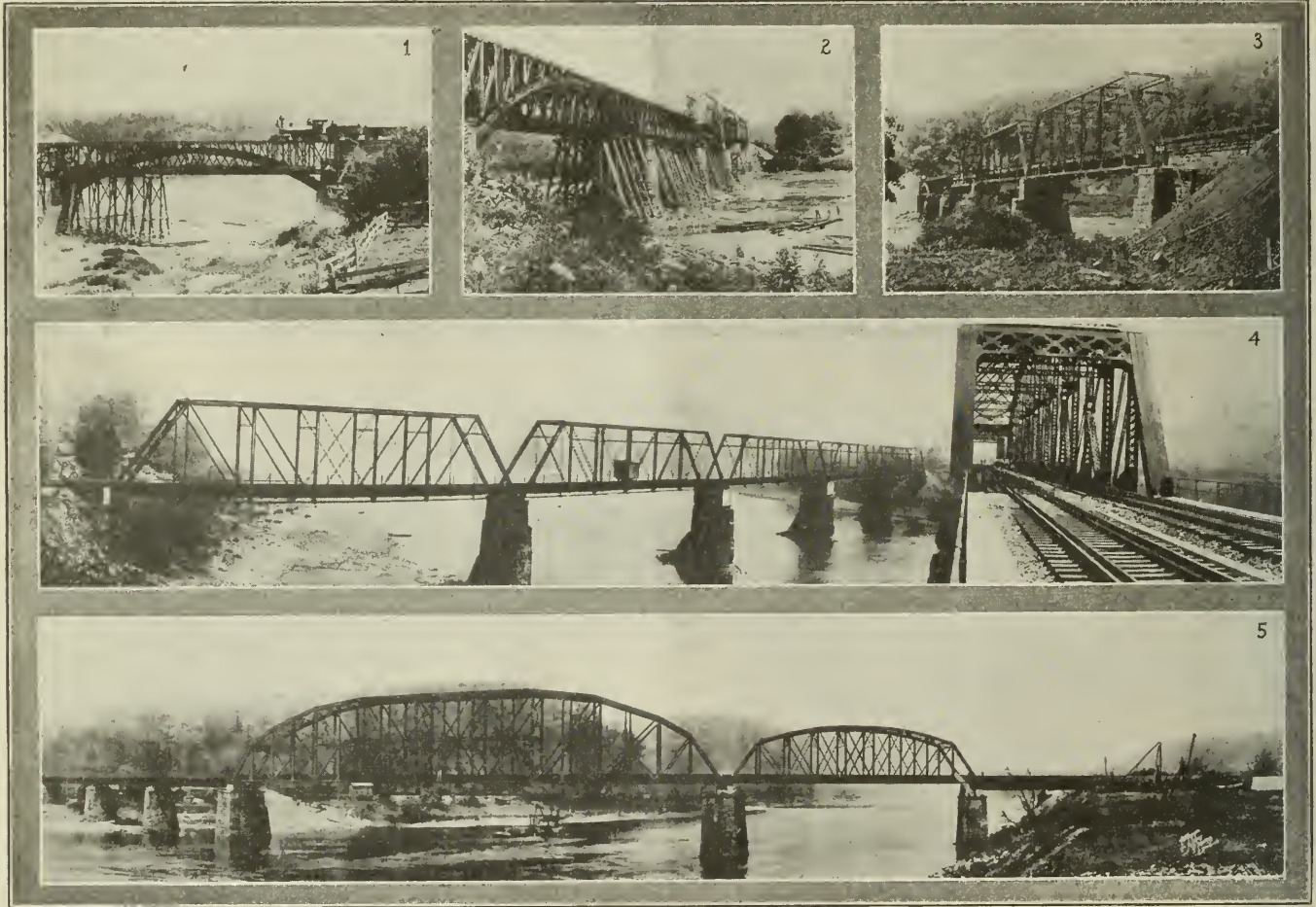
(1) The Original Wooden Bridge Erected in 1866, (2) Removing the Wooden Bridge in 1888, (3) The Five Span Single Track Steel Bridge, (4) and (5) The New Structure
