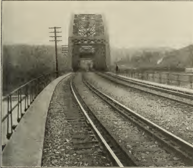
The Concrete Ballasted Deck on the Girder Spans
