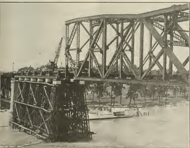
Erection Progress on Semi-Suspended Span Showing Canvas Covers Over the Sand Boxes
