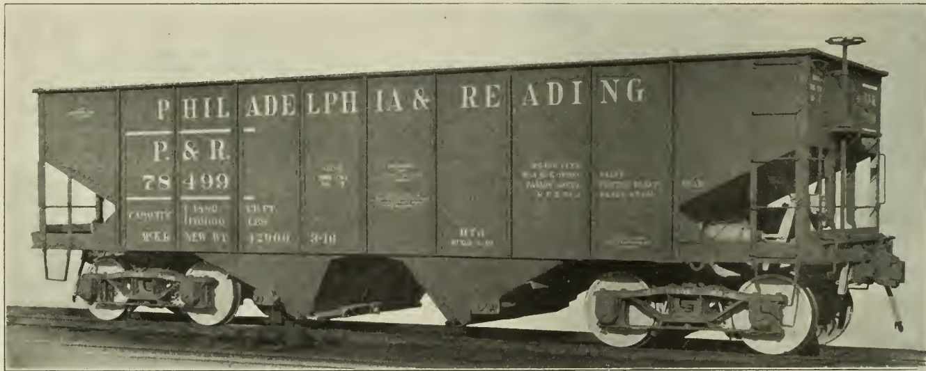
Philadelphia & Reading Hopper Car of 110,000 lb. Capacity
