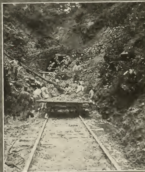
Debris Left by the Flood Track Spanning Break in Fill Mouth of Tunnel Choked by Debris
