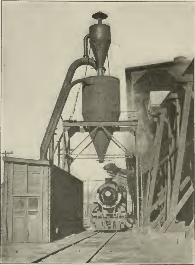
Fig. 5—Pulverizing Shed and Storage Tank at the North Western Coal Chutes
