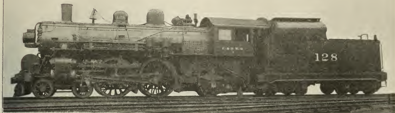
Atlantic Type Locomotive Which Burns Pulverized Coal
