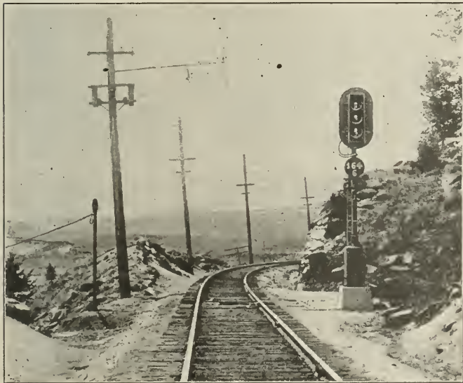
Typical Signal Location; Line Transformers, Cable Post, Impedance Bond
