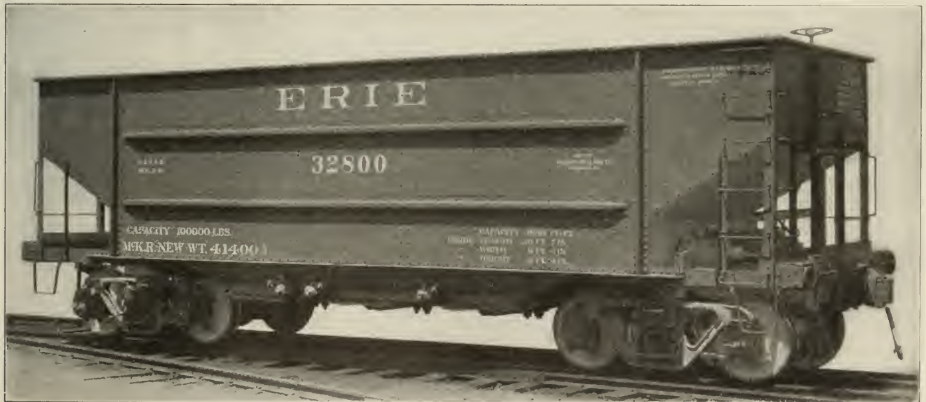
Erie Railroad 50-Ton Capacity Hopper Car
