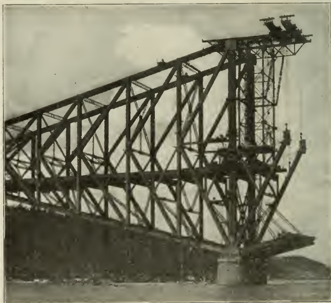
Traveler Erecting Material for the First Main Panel of Cantilever Arm
