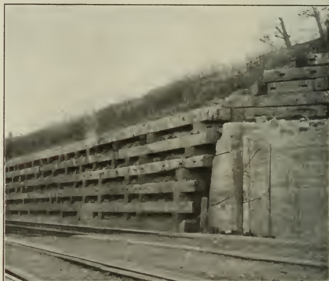
A Section of the Heavy Timber Crib Retaining Wall
