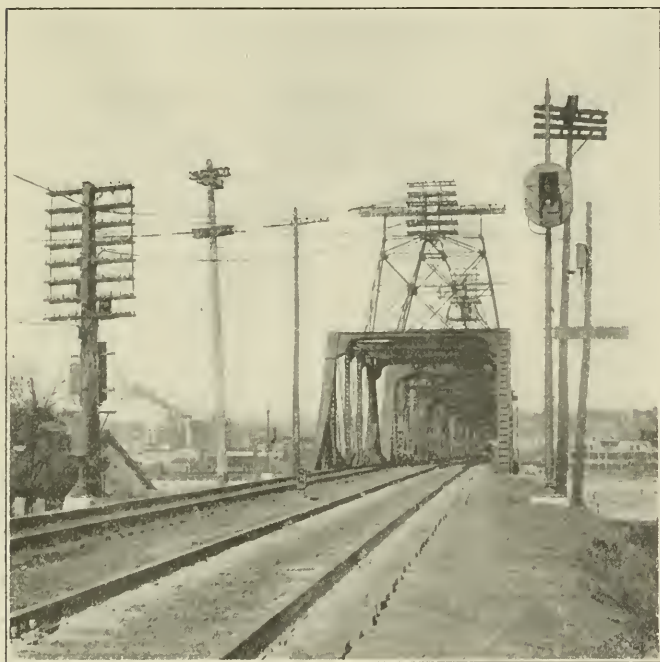
Home and Dwarf Light Signals at East End of Bridge
