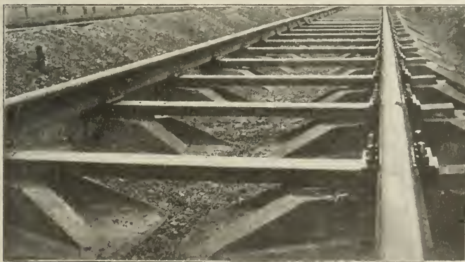
The Experimental Track with Ballast Removed
