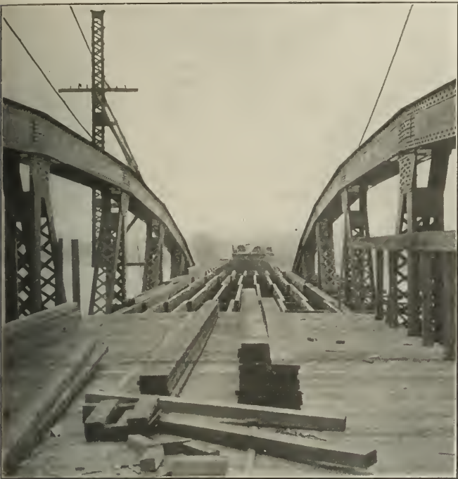
Highway Deck of One of the Two 154½ ft. Spans
