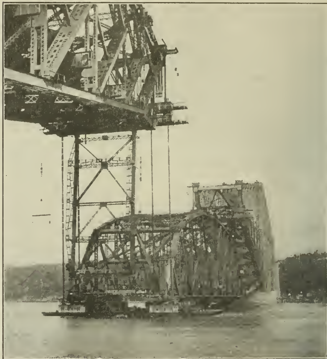
The Suspended Span In Position Ready for Hoisting. The Load Is Still on the Scows
