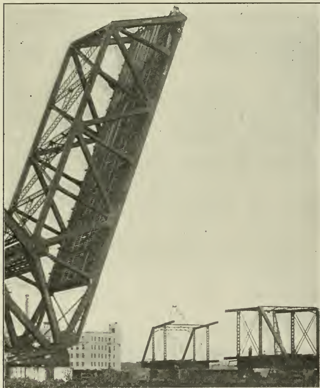
Old Swing Span Cut in Two to Clear Bascule Span
