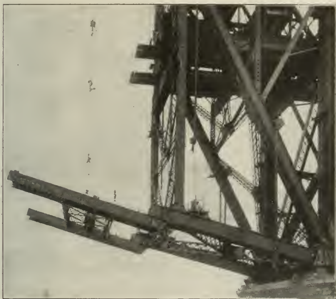
Erection Bridge Placed in Position to Receive Bottom Chords
