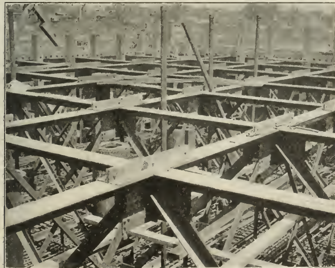
Steel Framework for the Caisson Slab
