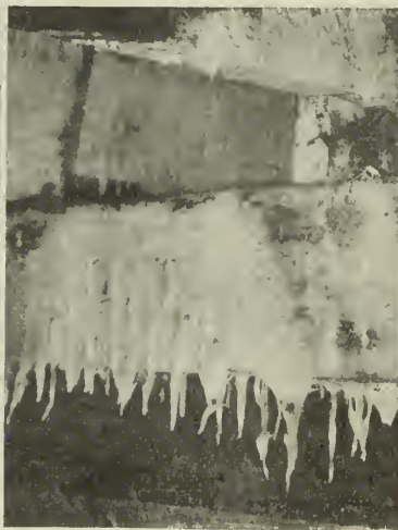
End of Douglas Fir Girder Embedded in Concrete Completely Rotted in 4½ Years. Mycelium Growing on Girders in a Basement. Severe Rot in Laminated Floor Laid Green and Covered with Plaster
