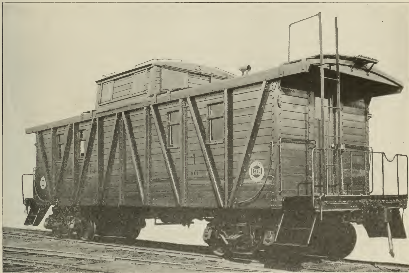
Steel Frame Single Sheathed Caboose for the N. C. & St. L.
