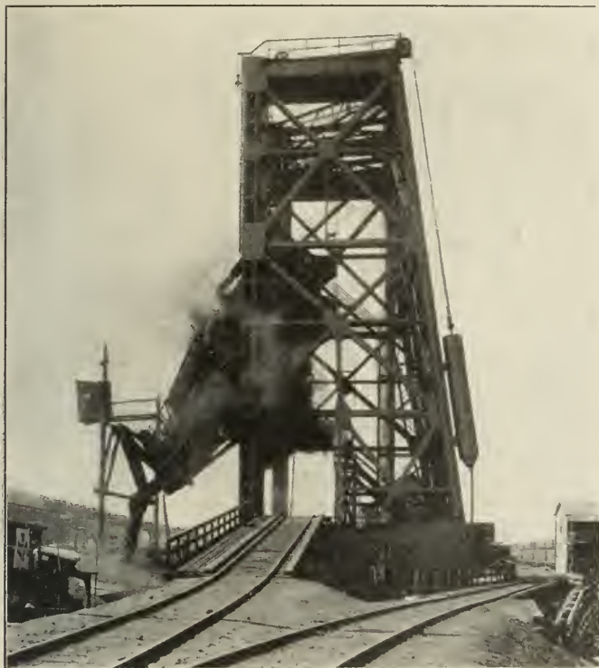
Side View of New Pennsylvania Car Dumper at Philadelphia, in Action
