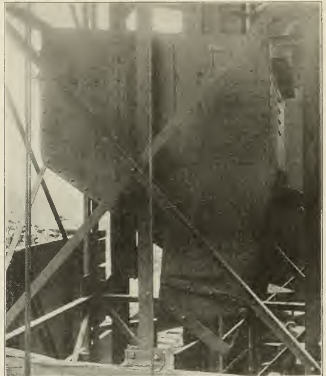
The Elevating Bucket in the Shaft
