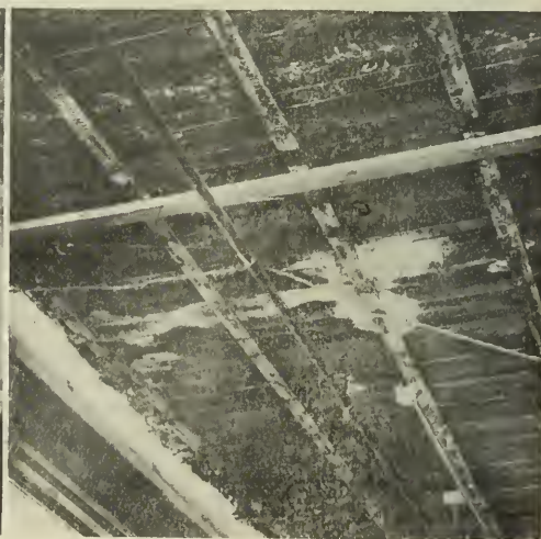
End of Douglas Fir Girder Embedded in Concrete Completely Rotted in 4½ Years. Mycelium Growing on Girders in a Basement. Severe Rot in Laminated Floor Laid Green and Covered with Plaster
