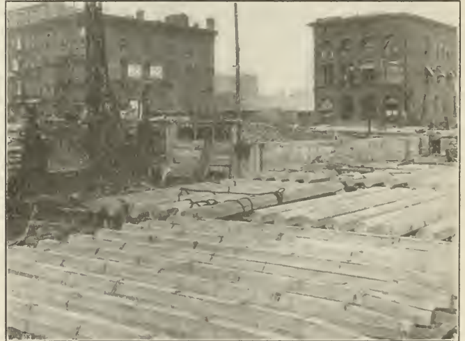
Concrete Piles Cast on the Ground
