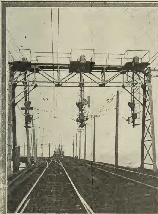
Double-Track Bridge Showing Suspended Signals
