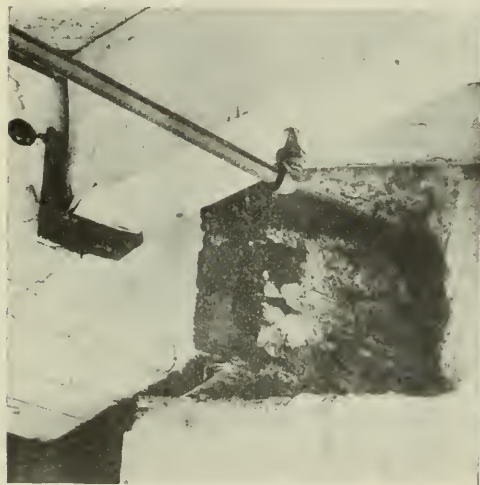
End of Douglas Fir Girder Embedded in Concrete Completely Rotted in 4½ Years. Mycelium Growing on Girders in a Basement. Severe Rot in Laminated Floor Laid Green and Covered with Plaster
