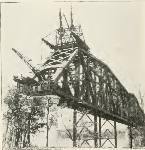
Creeper Traveler Standing on the Completed Kentucky Span
