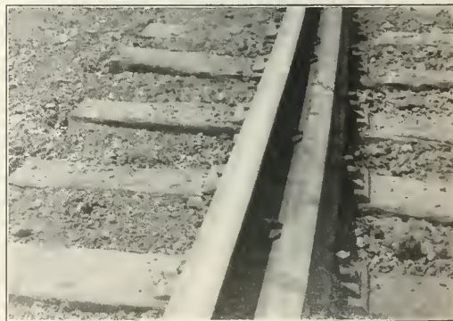
The Guard Rail Fastenings Installed in Track
