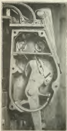
Fig. 1—Circuit Controller Box; Cover Removed Fig. 1a—Circuit-Control Apparatus
