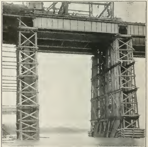
The Falsework Did Not Obstruct the Flow
