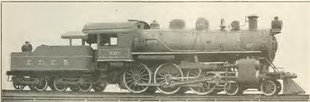
Pulverized Coal Burning Locomotive for the Central Railway of Brazil
