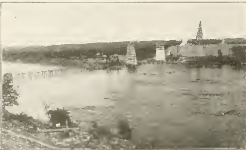
Concreting Piers from an Aerial Tramway
