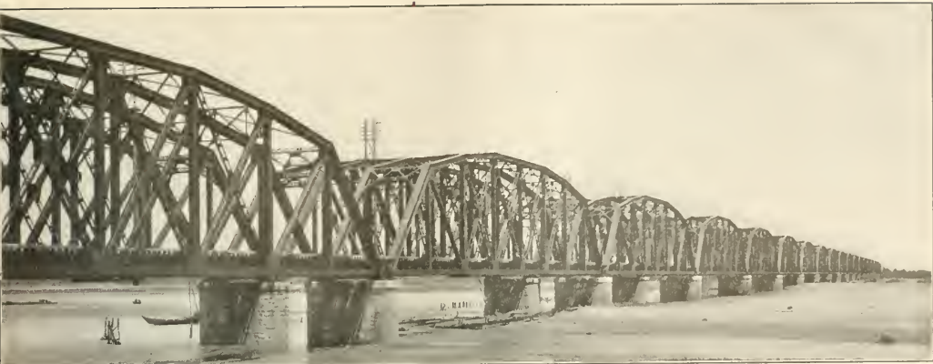
Tenryugawa Bridge (19 200-ft. spans), Tokaido Line.
