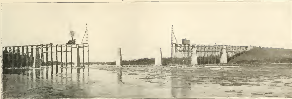
Driving the Temporary Bridge
