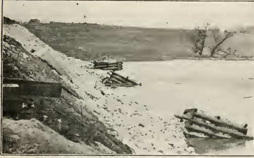
Rock Filled Cribs and Rip Rap to Protect Embankment
