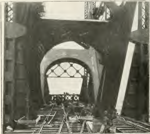
Heavy Portal Frames on Diagonals Over Middle Pier
