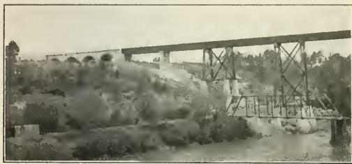
North End of Saluda River Viaduct Showing Arches, the Solid Concrete Pier, and Square Circular and Buttressed Pedestals
