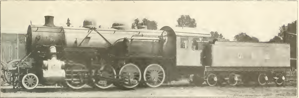
Locomotive No. 1, the First of 680 Consolidations for Service in France. Was Built in 20 Days
