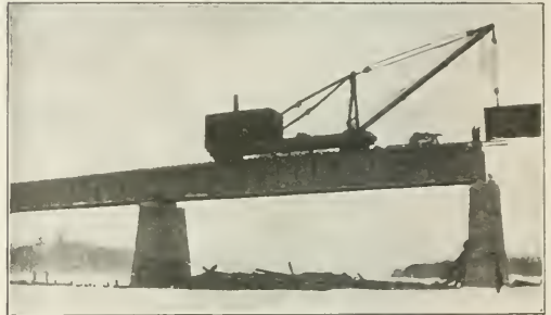
Placing a 100-Ft. Girder
