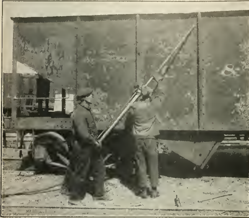
Rivet Cutting Gun Being Used in Steel Car Repairs
