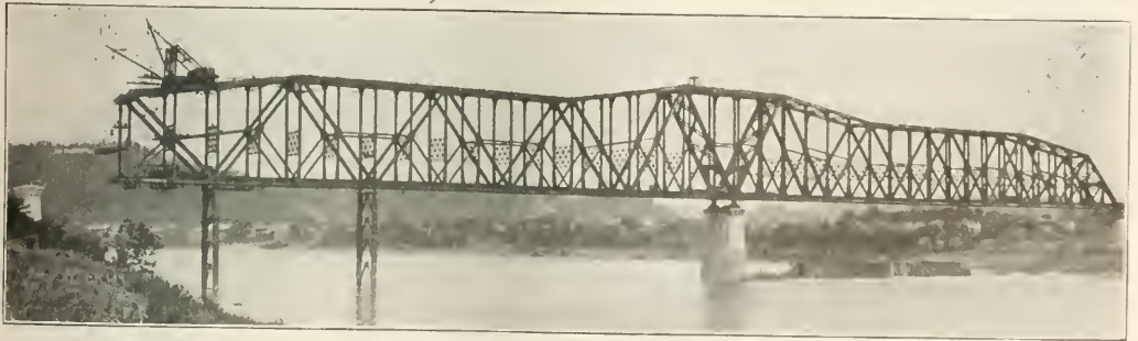
Ohio Span Completed, Kentucky Span Advanced by the Creeper Traveler While Carried on Two Temporary Bents
