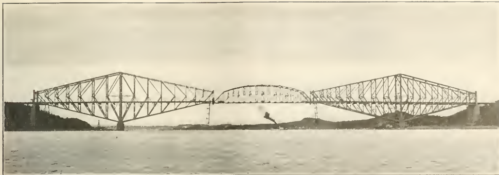
The Bridge Showing the Suspended Span in Place
