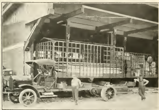
Motor Truck Chassis With Removable Truck Body and Chain Hoists
