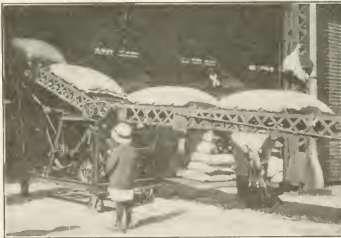
Fig. 2. Portable Electric Conveyors Pile to the Roof and May Be Placed at the Most Convenient Point
