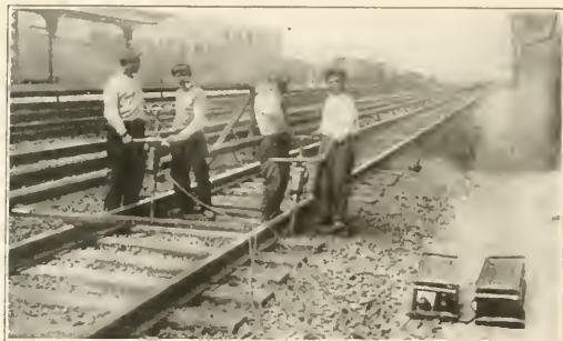
Tamping Track in the Electric Zone
