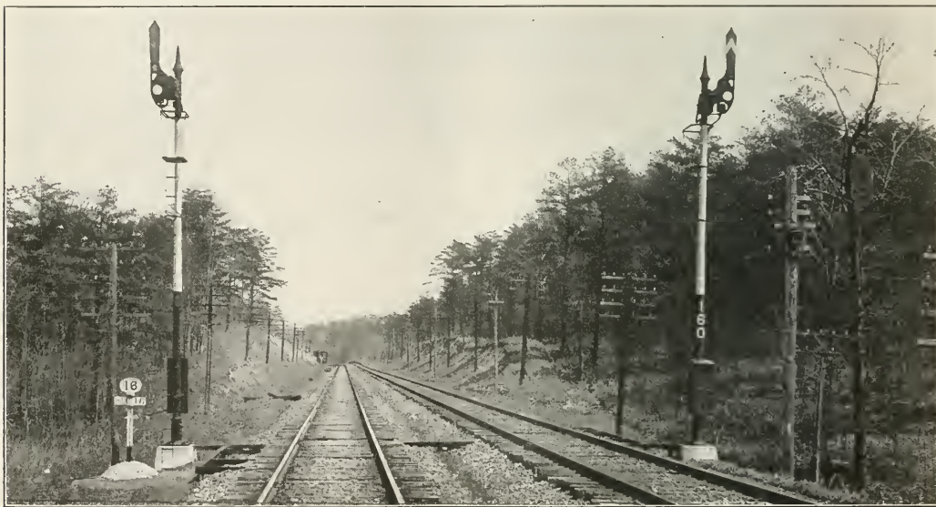
Typical Signal Location Showing A. C. Line at the Right
