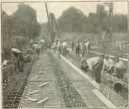
Placing the Reinforcement in the T-Beams and Floor Slab
