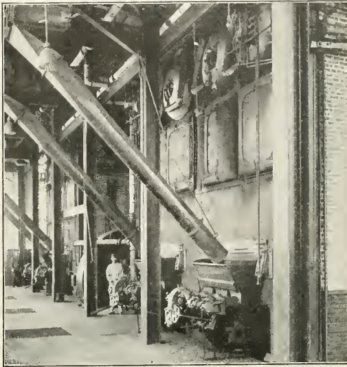
Fig. 2—Automatic Stokers and Coal Chutes in Boiler Room, Curtis Bay Power Plant
