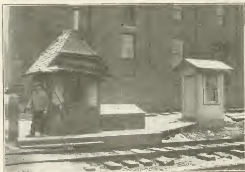
Kaustine Installation in a Separate Building for a Crossing Watchman
