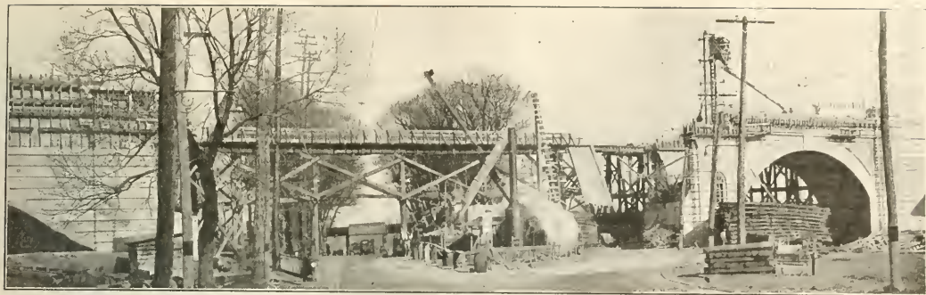
Queens Boulevard Bridge, Showing the Construction Plant at the Street Level
