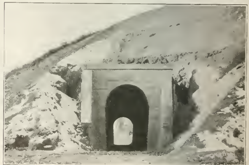
16-ft. Arch Culvert Under 1,000,000-cu. yd. Embankment
