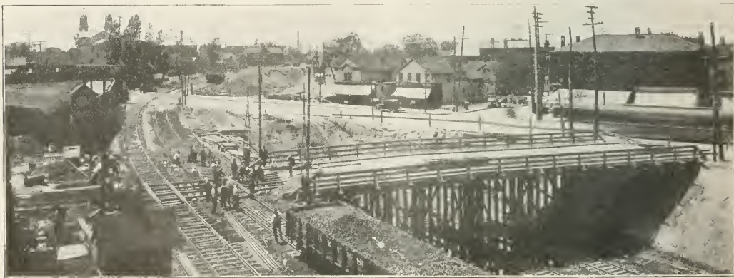
One of the Temporary Bridges Built to Carry Street Traffic Across the Cut
