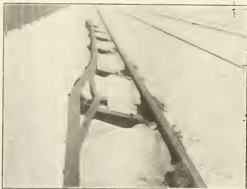
Fig. 2—Contact Bar After a Snowstorm—Looking to the Rear
