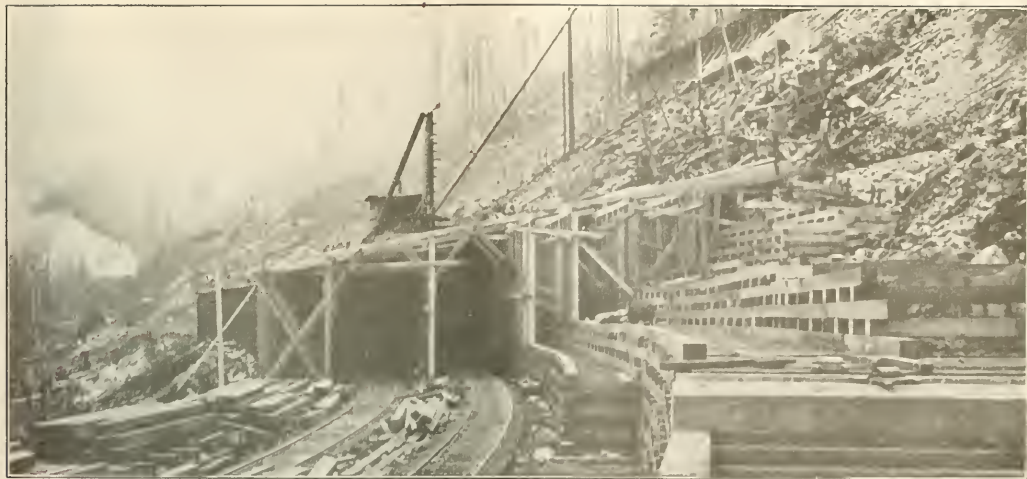
Timber Shed Construction
