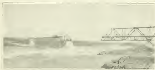
Beginning of Erection of the Northern Anchor Span, with the Traveler at the Floor Level
