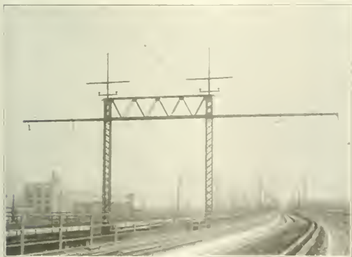
Fig. 5. Transition Structure Used Between Two Different Types of Trolley Construction
