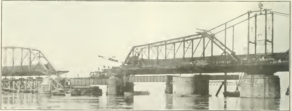
Fig. 10. The Gap Between the Draw Span and Fixed Span No. 3 After the Shift Had Been Completed
