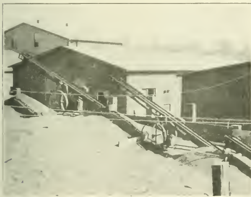
Increased Storage Capacity Is Gained by Using the Conveyor in Flights
