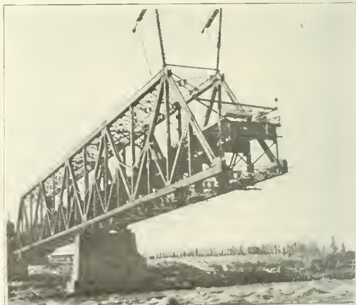
Southern Half of the Bridge Erected
