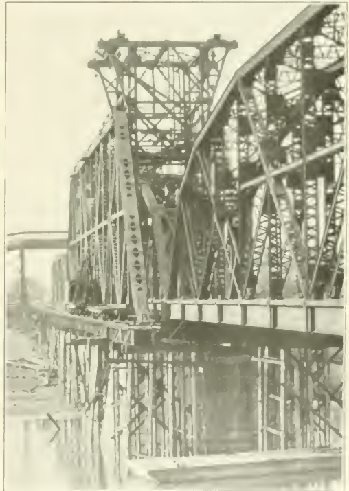
New 300-ft. Span Surrounding Old Span, Showing Also Gantry Traveler and a Derrick Car on Temporary Track
