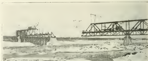
The Cableway with Its Equalizing Girder
