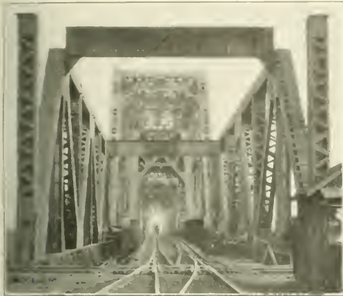
New 132-ft. Span in Foreground with Old 80-ft. Girder Span Still in Place
