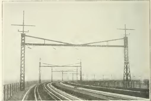
Fig. 8. Typical Trolley Construction for Use on Curves
