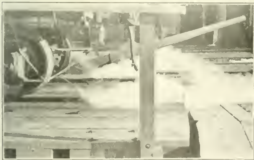
Steam Blowers Arranged to Clear Caterpillars from the Rails
