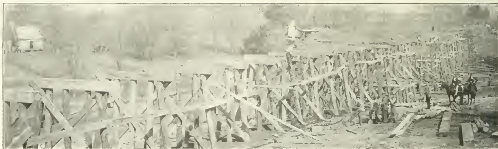
An 800-foot Trestle with Piles from Four States Completed in Five Days
