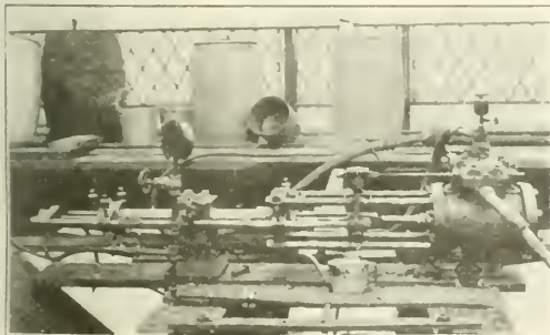
Fig. 7. One of the High Power Pumps Supplying Pressure to the Jacks
