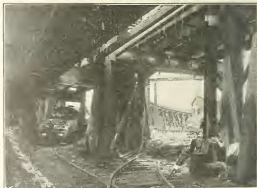
Specially Designed Trestle Bents at the Carnegie Tracks
