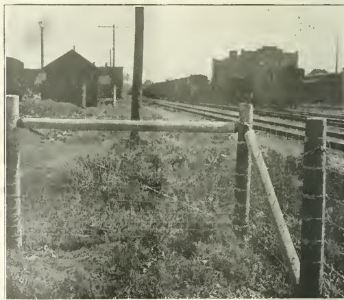
The Corner Post and End Post Arrangement
