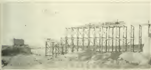
Falsework Under Construction for the Northern Anchor Span
