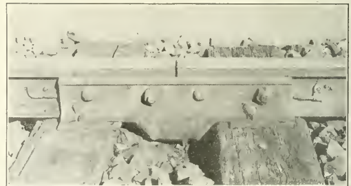
Fig. 9—Railroad Joint Showing Type of Bond Used. Note That Only a Small Amount of Copper Is Exposed
