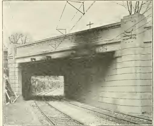
Fig. 8—Catenary Is Insulated from Overhead Highway Bridges by Post Type Insulators
