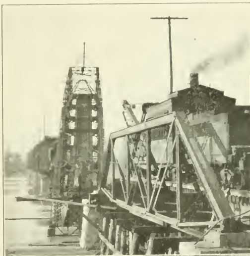
View Showing How the Span Swung in Tipping Down
