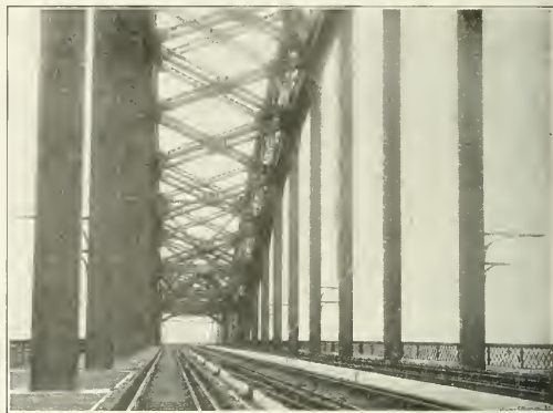
Fig. 3. Trolleys Are Supported on Hell Gate Bridge by Attaching the Cross Wires to the Steel Members of the Bridge
