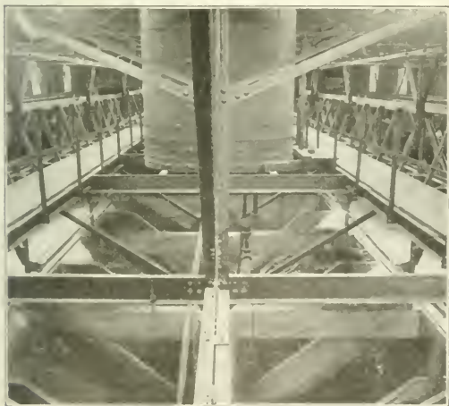
Arrangement of Chutes Over the Coal Pockets
