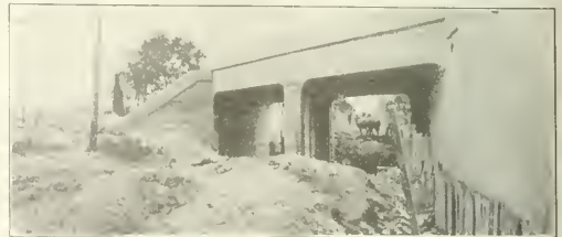
A Typical Flat Slab Bridge for County Highways
