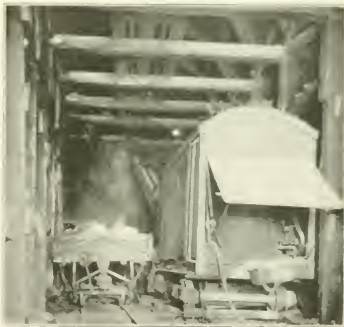
Air Operated Shovel Picking Up Muck at the West Bench
