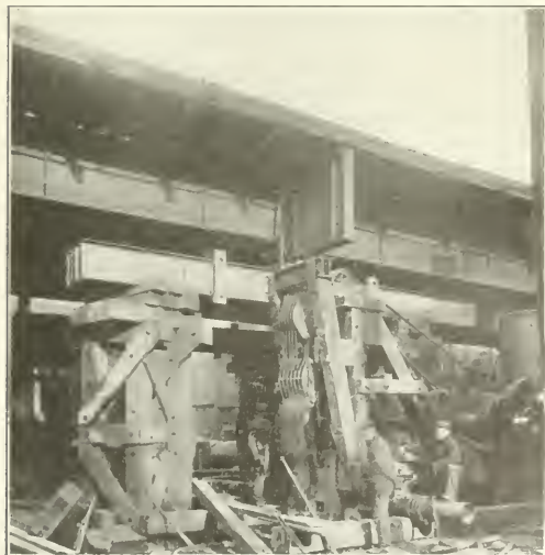
The Special Pile Driving Rig Used in Thirty-third Street
