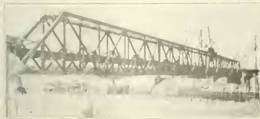
The Lower Members of the Portal Struts and Sway Bracing Were Omitted Temporarily for the Accommodation of the Derrick-Car
