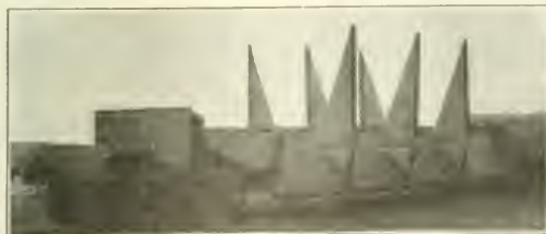
Ends and Floor Section Assembled and Side Gusset Straps in Place
