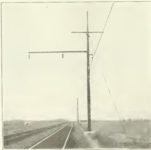
Fig. 7. Guyed Tubular Bracket Type Poles Are Used for Single and Double Track Construction
