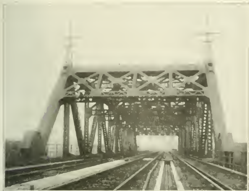
Fig. 4. On Bronx Kill Bridge, the Trolley Insulators Are Attached Directly to Overhead Steel Members
