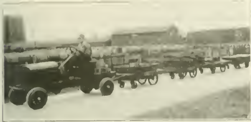
A Converted Ford Truck Hauling Trailers Loaded with Heavy Materials
