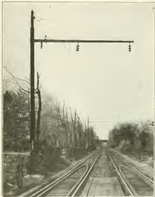
Fig. 5—Extra Heavy Tubular Pole Without Guys for Two Track Construction
