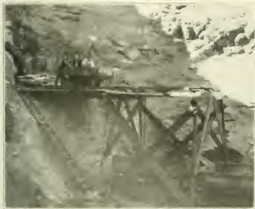
Dumping Muck from the East Heading Off a Trestle
