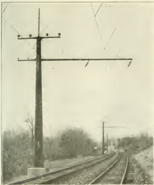
Fig. 4—Structural Pole Without Guys for Two Track Construction
