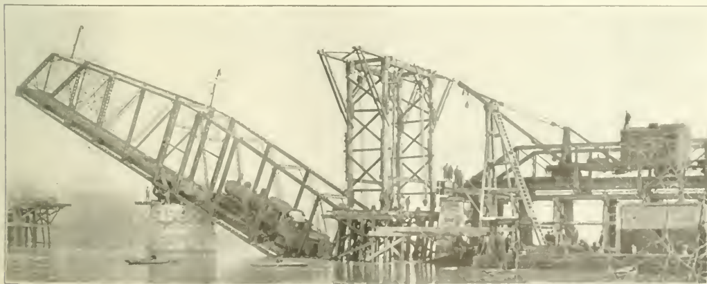
Method of Raising the Span
