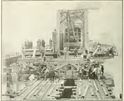
Fig. 11. Placing the Pony Bents to Close the Gap
