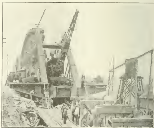
Fig. 5. Tearing Out the Falsework for the Main Track Between the Old and New Abutments. One of the Hauling Tracks Is Shown in the Foreground
