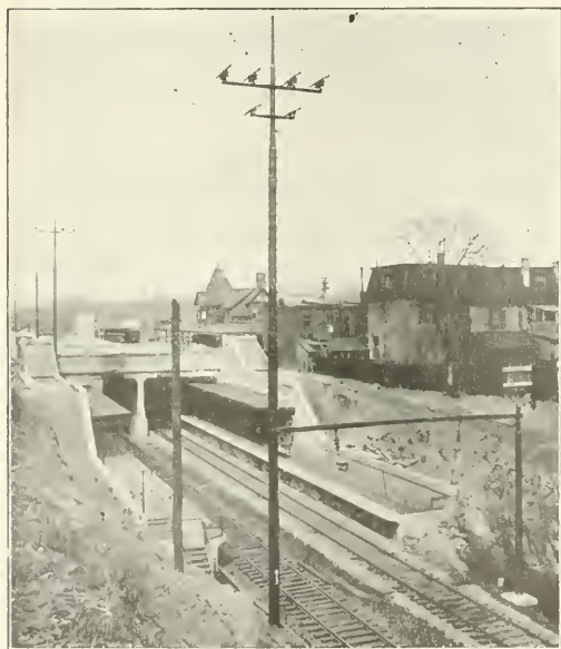
Fig. 2—Transmission Pole Carrying 44,000 Volt Line
