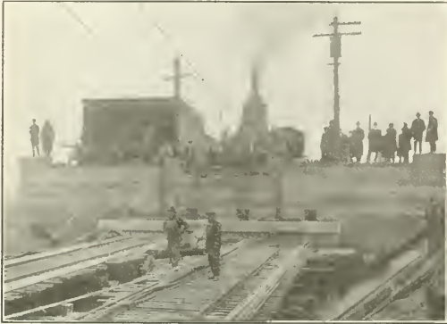
Fig. 9. The Motive Power, Steam and Electric Hoists at the West Abutment
