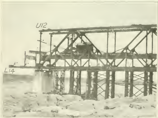
Southern Anchor Span Erected, and the Beginning of Cantilever Erection Showing the Temporary Supports for Panel Points
