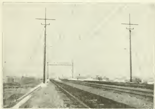
Fig. 6. Guyed Tubular Poles with Cross-Catenary Wires to Support the Trolley Are Used Where the Passenger Tracks Leave the Freight Line
