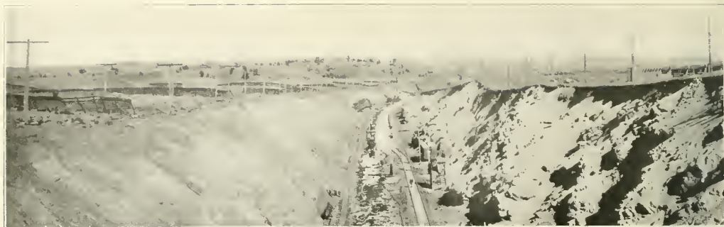
Temporary End of Double Track in the East Approach Cut of the Sherman Hill Tunnels
