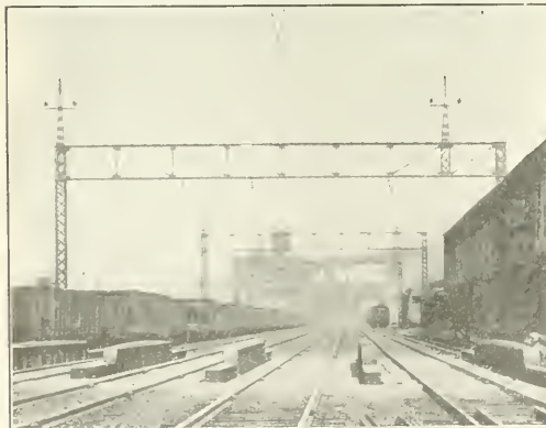
Fig. 7—Structural Bridge for Use Over Four Tracks
