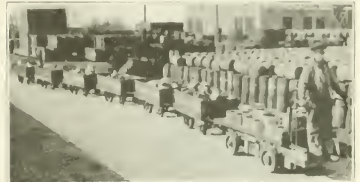
Electric Truck Hauling Six Trailers Loaded with 17,500 lb. of Brass
