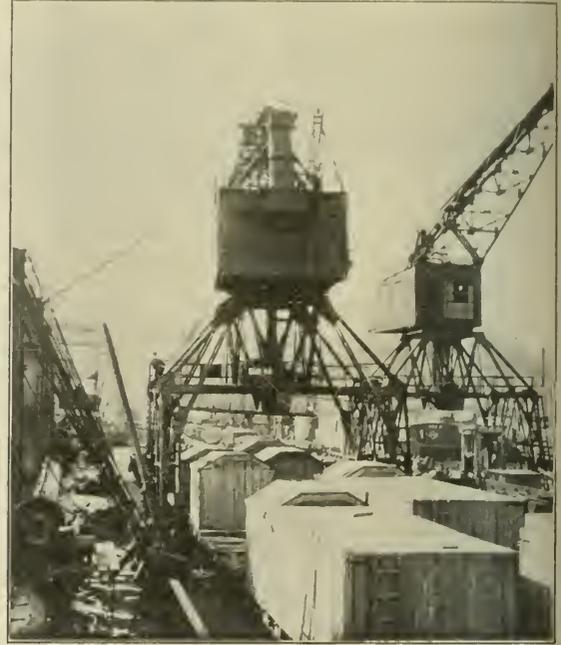
Type of Gantry Crane Used. Pier Is Equipped With Three Ten-Ton and One 20-Ton Cranes
