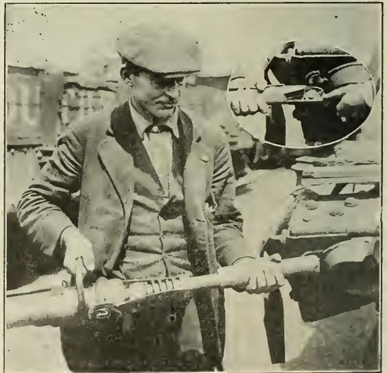
Rivet Catcher in Use and (in the insert) the Pocket Exposed
