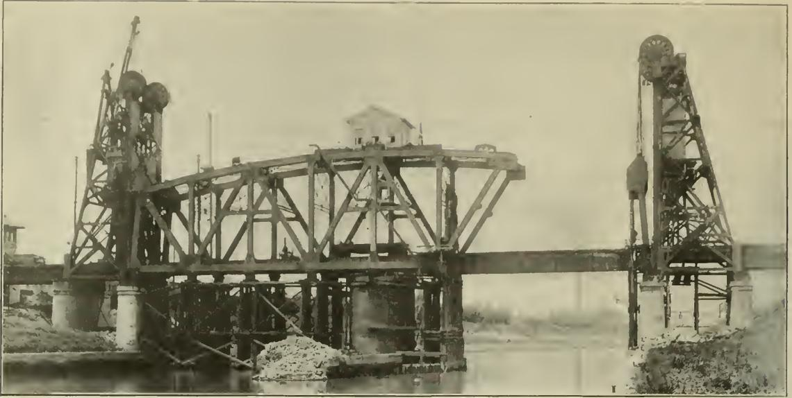
New Lift Span Partially Completed with Temporary Lift Span Still in Place
