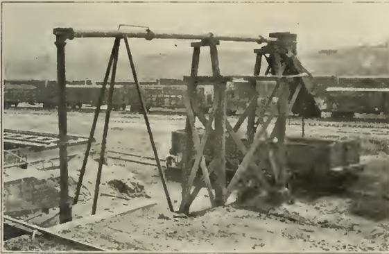
Conveyor Which Discharges Cinders Through a Pipe Line by the Action of a Steam Jet
