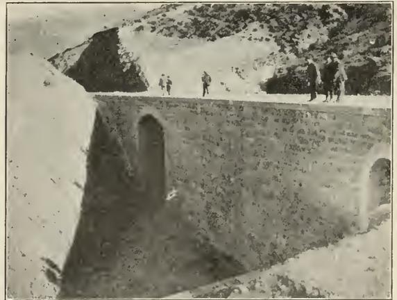
Fig. 2—Masonry Retaining Wall and Culvert at Jaca on the Line to Canfranc
