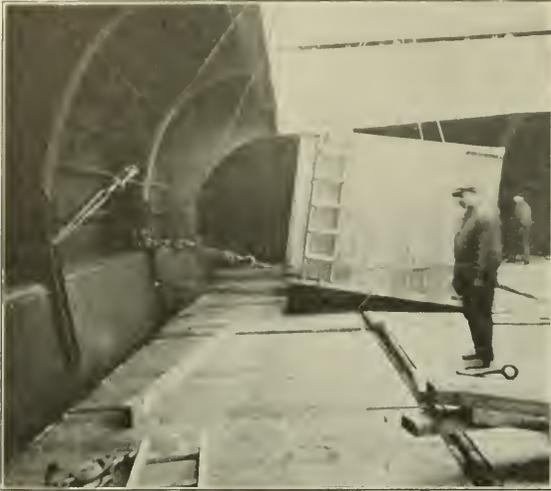
The Crane's Boom Was Not Long Enough to Reach the Off-Pier Side of the Ship and to Place the Boxes on this Side the Ship's Hoisting Apparatus Was Used to Pull Them to the Side as Shown in the Picture
