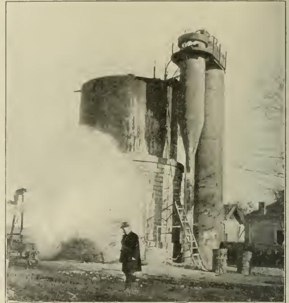
Fig. 9—Water Tank and Water Softening Apparatus
