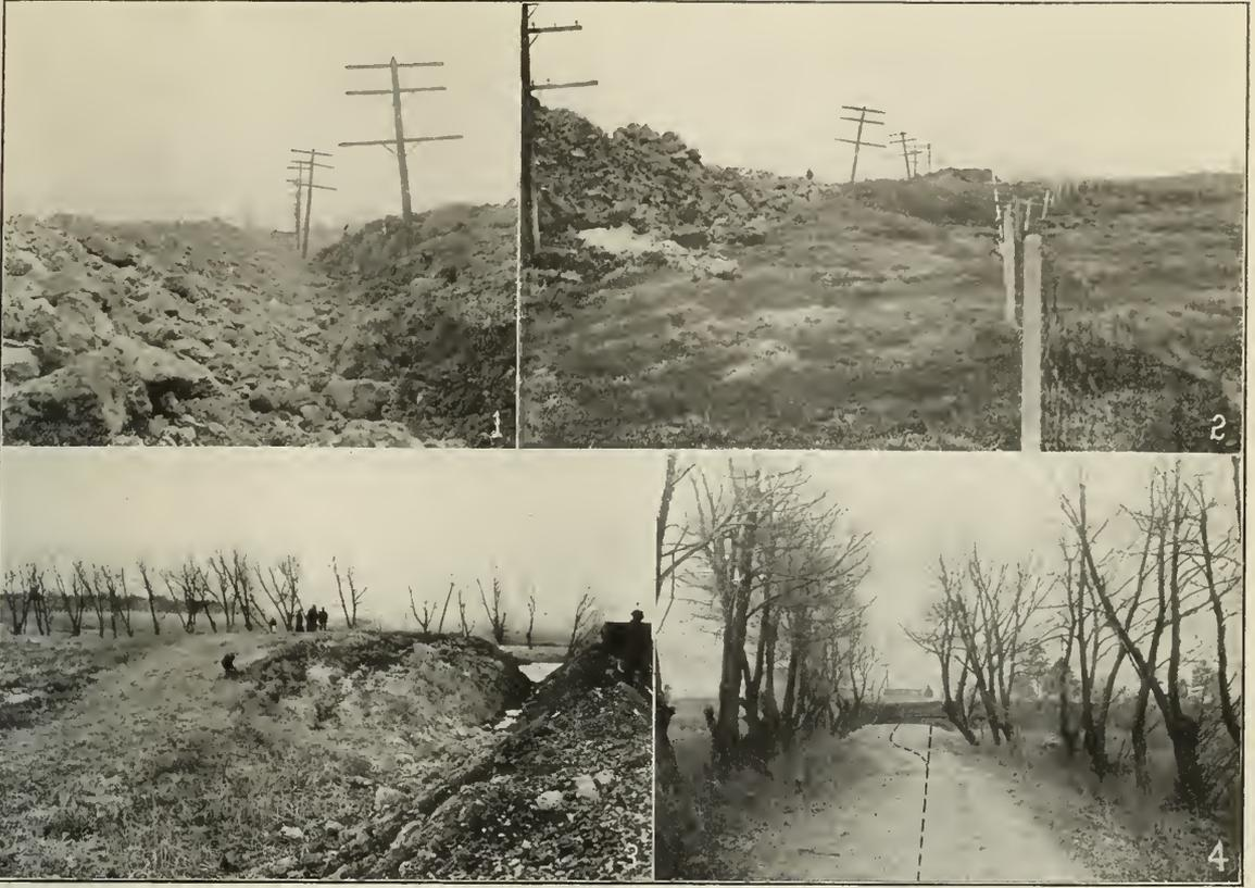
Fig. 1.—New Embankment on the Left, Upheaval of Peaty Soil on the Right. Fig. 2.—Fence Line Has Been Displaced from Position Indicated by the Dotted Line. Fig. 3.—Large Upheaval of Soft Material. Fig. 4.—Displacement of the Highway Indicated by the Dotted Lines.
