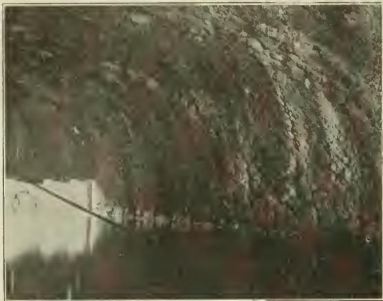
The Arch Soffit with the Concrete in Place
