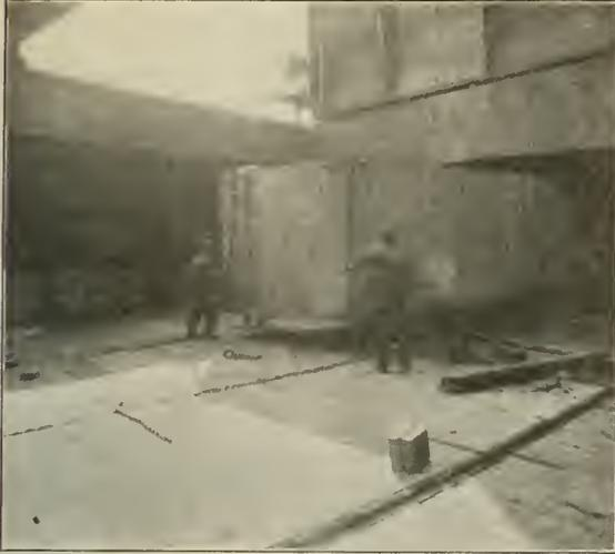
Box Containing Tender Tank Being Lowered Into the Ship's Hold. The Largest Parts Placed in This Manner Were the Boilers Which Weighed 20 Tons
