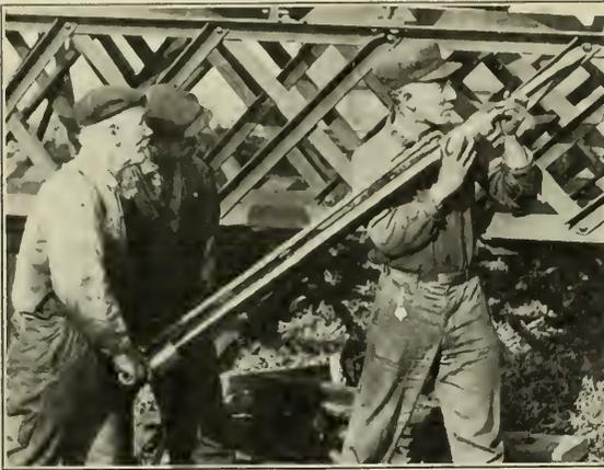
Using the Red Devil Rivet Cutter on Structural Steel Work
