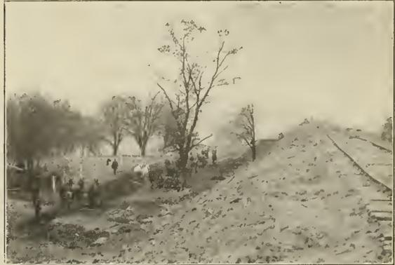
Building a Drainage Diversion Ditch Alongside the Eagle Creek Embankment
