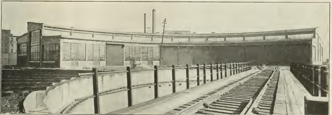
A Three-Section Roundhouse with a Single-Section Monitor
