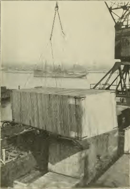
The Box Contains a Tender Tank and Weighs 14 Tons. The Picture Shows the Box Suspended Over the Cars on the Pier Preparatory to Swinging It Over the Ship's Side
