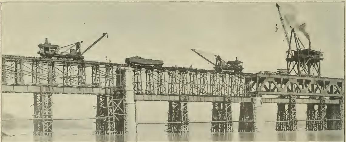
Falsework for the Erection of the Deck Truss Spans
