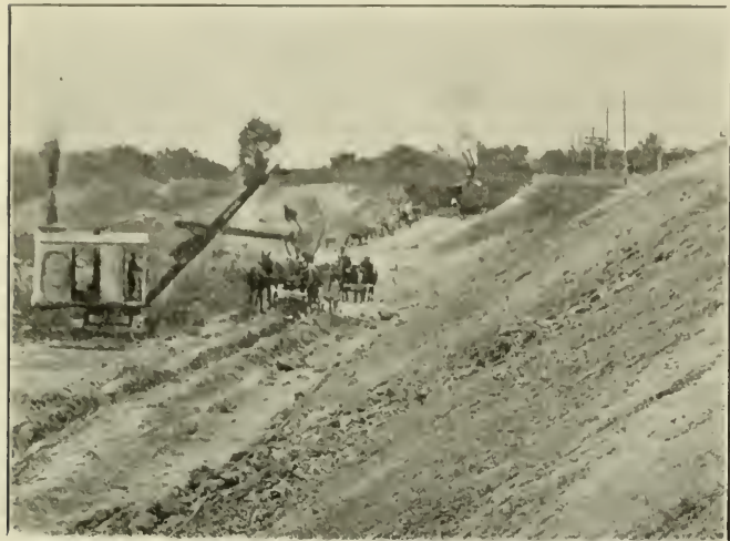
Grading with Revolving Shovels and Horse-Drawn Wagons
