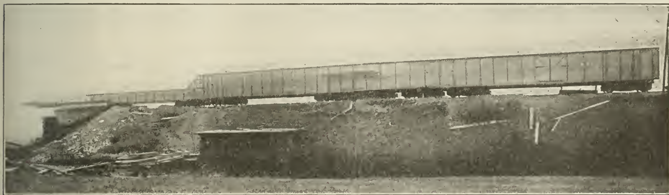
This Shows the Members of the Bridge Rivetted in Place and Ready to Extend Out Over the Span
