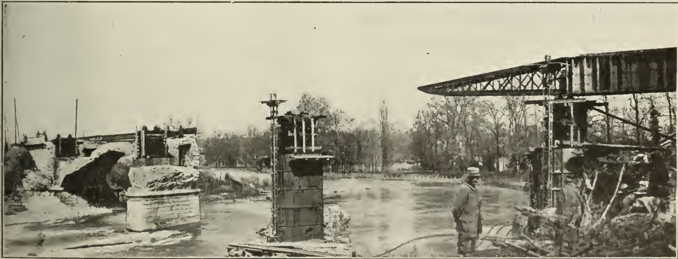
This Shows the Marcille Type of Bridge Ready to Be Swung Across the Span. It Will Be Noted That This is Somewhat Similar to the B. S. Type of Bridge
