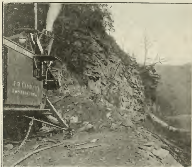
A Shovel Making a Cast-Over Cut
