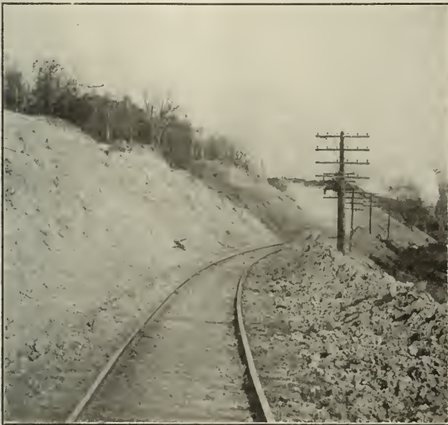
The Baltimore & Ohio Project Was Largely Side Hill Work. Old Line in the Foreground, New Line Above
