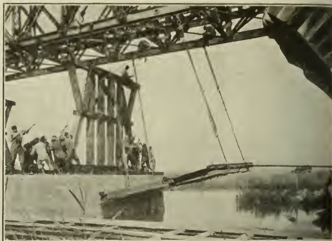
Method of Supporting the Henry Bridge During Construction
