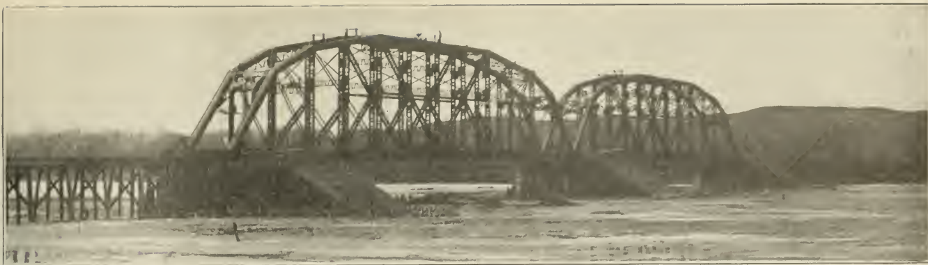
Two 300-ft. Spans on Pile Piers
