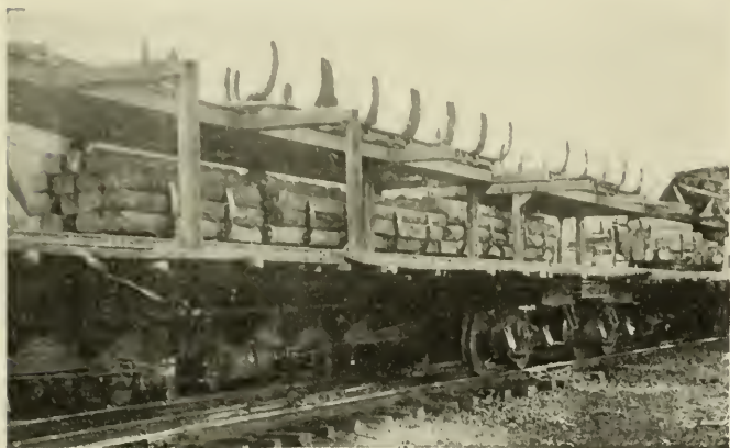
The Cars Carrying the Retort Tracks Have Two Decks
