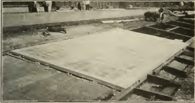
The Completed Roof in a Panel of the Train Shed Consists of Two Sections of Concrete Slab and One Section of Glass
