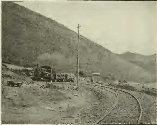
A Light Railway of 2 Ft. 6 In. Gage. This Scene Taken on the Antung-Mukden Railway (Since Converted to Standard Gage) Is Typical of the Light Railway Lines in Japan, Korea or Formosa
