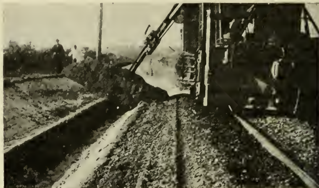
Outer Wing Extended Cutting Both Ditch and Slope. Shallow Cut
