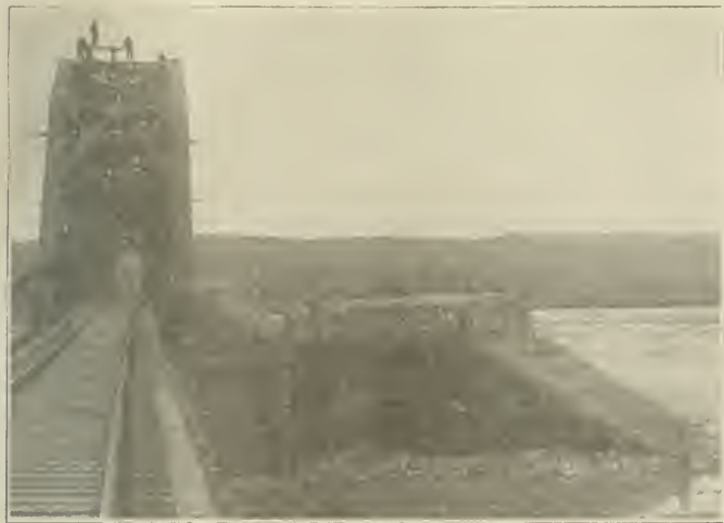
End View of the Bridge Showing One of the Ice Breakers With Its Concrete Covered Nose
