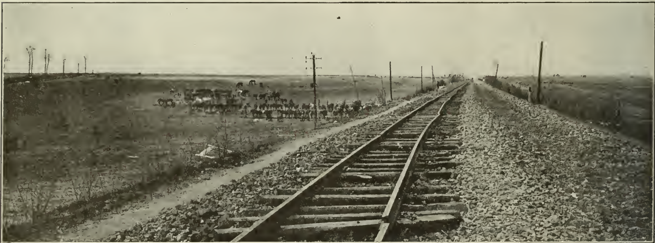
The Rail of a Single Track Line Damaged by Breaking the Middle of Every Rail
