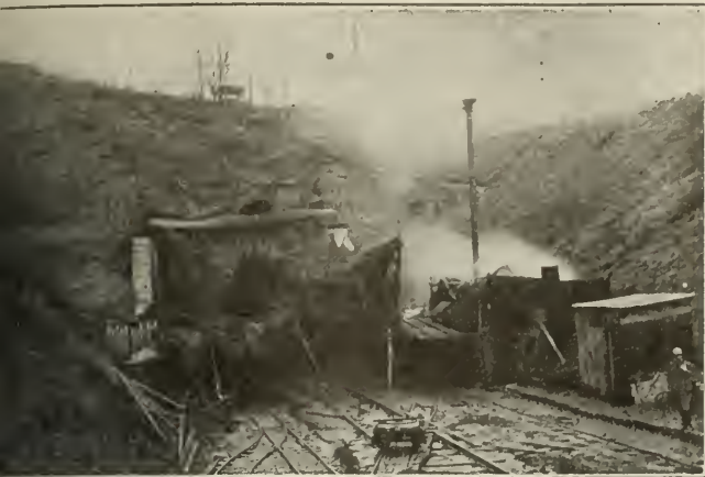
Damage Caused by Blowing Up a Tunnel Between Soissons and Laon. The Force of the Explosion Was so Great That It Will Be Noticed the Earthwork Above the Tunnel Has Settled Down in the Vaults
