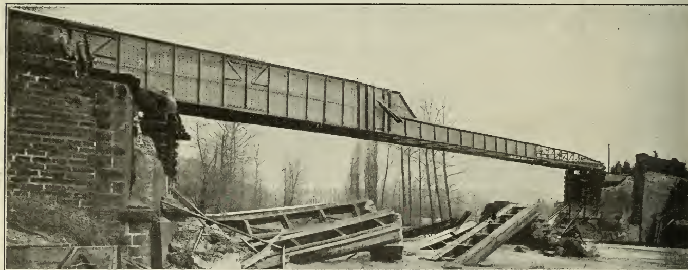
The Last Step. The Light Guiding Structure on the End of the Span Serves to Support the Weight of the Bridge on the Opposite Shore
