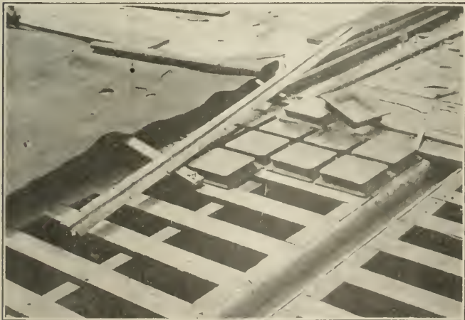
The Forms, the Glass and the Copper Expansion Joints
