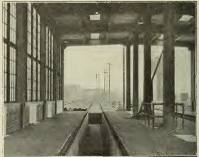
One of the Inspection Pits Covered by a Reinforced Concrete Shed
