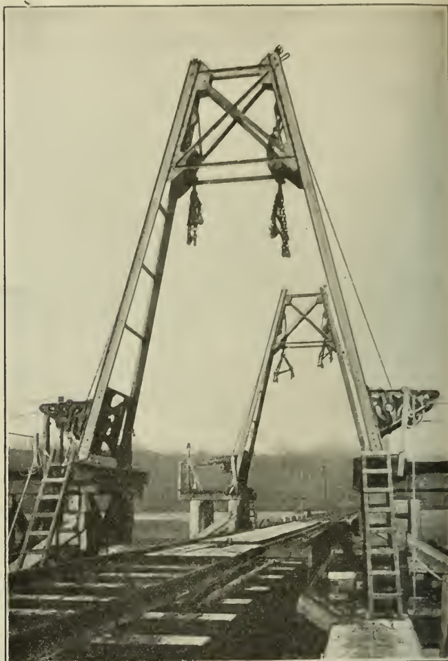
A Closer View of the Lifting Apparatus for the Lift Bridge Shown in Fig. 9
