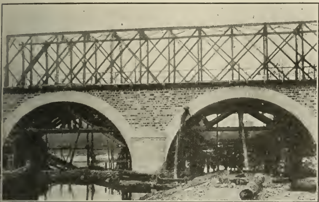
This Shows How the Permanent Bridge Has Been Constructed Under the Temporary Henry Type Bridge Without Interference with Traffic
