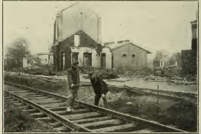
All That There Is Left at the Station of Hollain. Bent Rails Will Be Noted by the Platform. The Belgian Workmen Are Applying Their Screw Spikes.
