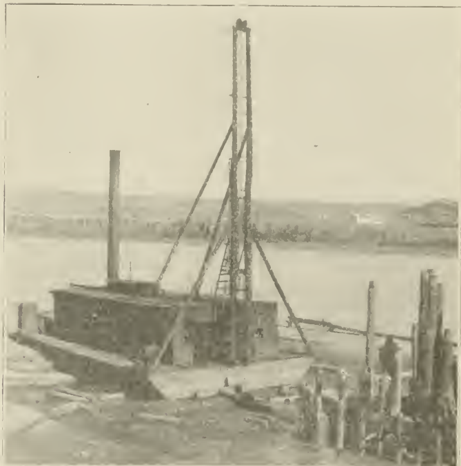
Type of Barge Driver Used for All Piles That Could Not Be Driven from the Trestle
