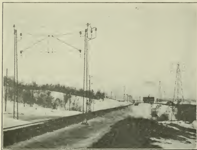
Contact Wires Overlap at Section Divisions
