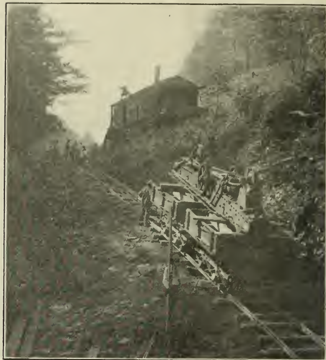
Moving Narrow Gauge Equipment Up a 20-Per Cent Grade at Belva
