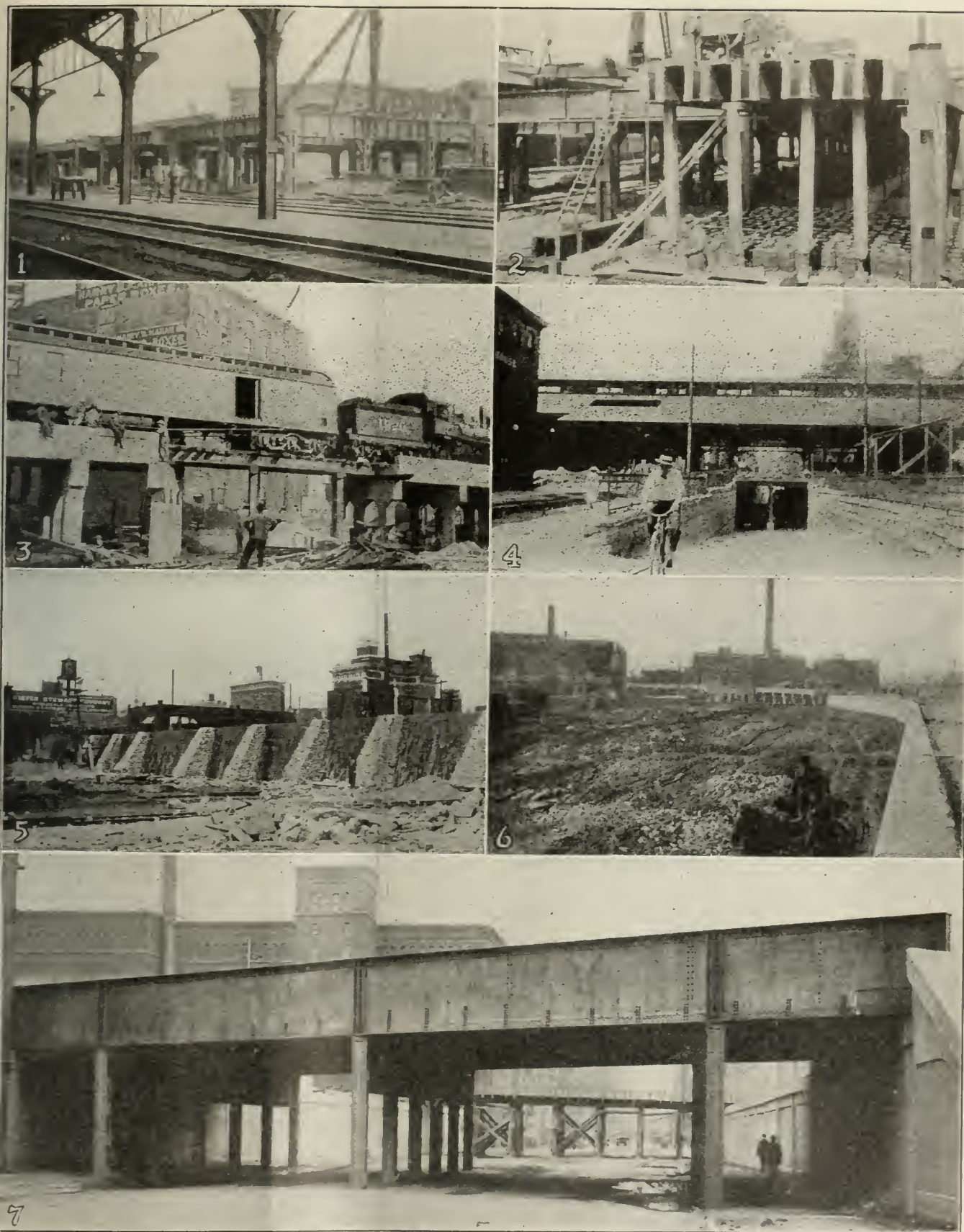
Fig. 1—Erecting the First Section of the New Trainshed. Fig. 2—Methods of Shoring the Trainshed Steel. Fig. 3—The Illinois Central Viaduct. Fig. 4—The Old Tunnel at Illinois Street. Fig. 5—Dry Packing Piers and Waterproofing. Fig. 6—Retaining Wall East of Capitol Avenue. Fig. 7—Indianapolis Union Wye Track Bridge Over Pennsylvania Street.
