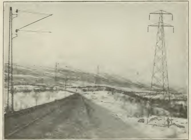
Typical Catenary and Power Line Construction on the Kiruna-Riksgränsen Electrification
