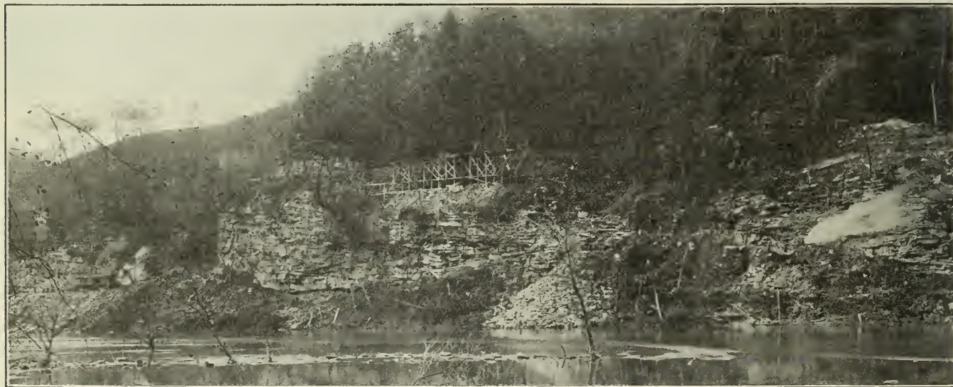
Drilling from a Trestle in Preparation for a Big Shot Between Stations 41 and 46. This Entire Cliff Was Shot Down at One Time
