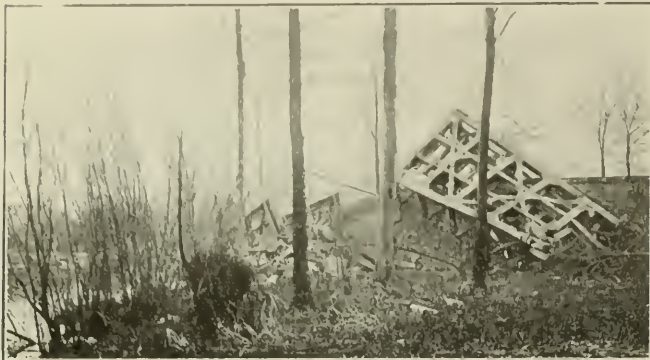
A Somme Bridge. This Damage Was Done by Dynamite. The Force of the Explosion Was so Great That the End of the Bridge Resting on the Left Bank of the River Was Thrown Completely Across the River and Is Shown Upside Down at the Right of the Illustration
