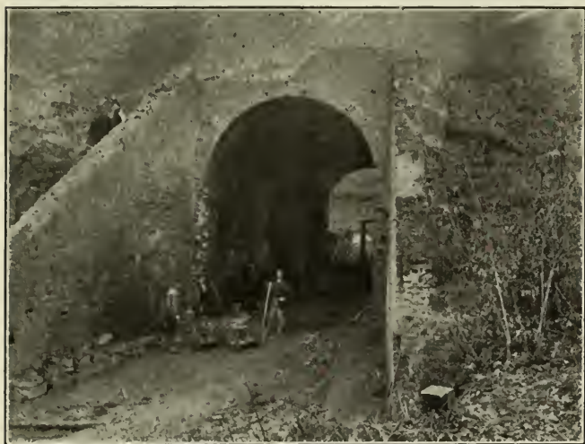
A Masonry Culvert Near Angre Destroyed by Mines Set in Its Walls in Three Places.
