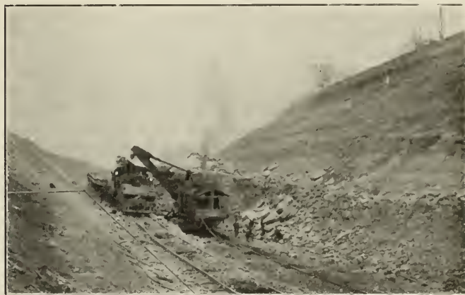
Steam Shovel at Work in the Huffman Cut
