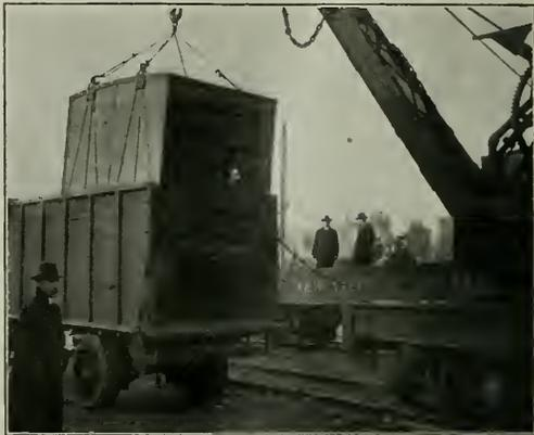
Loaded Container Being Lifted from Motor Truck
