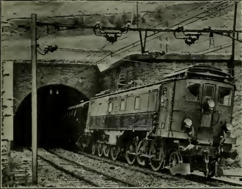
Passenger Train at South Portal of the St. Gothard Tunnel, Swiss Federal Railways, 1921. Locomotive Develops 2250 h.p. from a 15,000-Volt, Single-Phase Trolley
