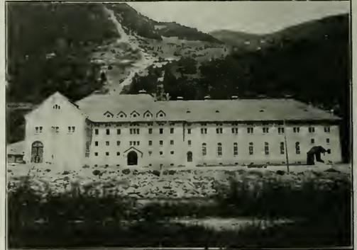
The Ritom Power Station. Pressure Pipe Lines from Lake Ritom Are Brought Down Through Cleared Space in the Timber Shown in the Rear
