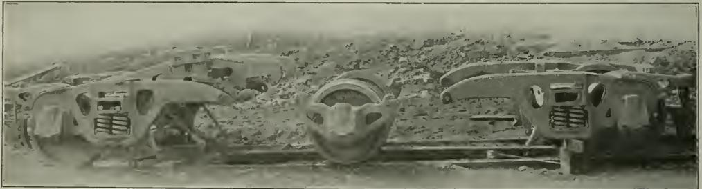
Fig. 3—Center Wheels Ready for Removal
