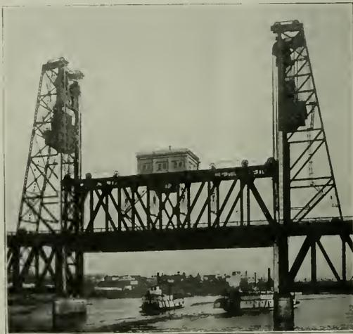
A Further Elaboration of the Vetical Lift Span. The Harriman Bridge at Portland. A Lift Span with a Lower Lifting Deck
