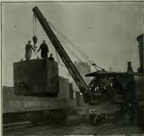
Locomotive Crane Placing a Loaded Container on the Car
