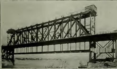
An Elaboration of the Lift Span Idea. The North Kansas Bridge Over the Missouri River with a Lifting Lower Deck
