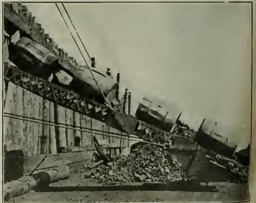
The Lower End of the Main Conveyor Hoisting Package Freight from the Deck of a Barge
