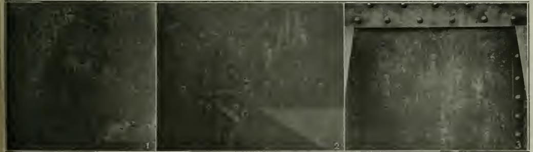
1. Badly Deteriorated Coating. 2. An Example of Paint Coat Subjected to Abuse by Pounding and Scratching. 3. Typical Pitted Surface After Brushing and Scraping
