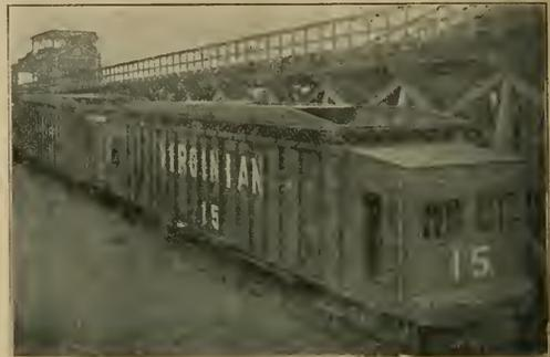
The 120-Ton Tractor Cars Used with the Tandem Dumping Machine at the Sewalls Point Pier
