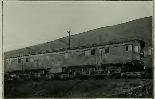
Fig. 2. The Quill-Gear Passenger Locomotive Built by the Westinghouse Electric & Manufacturing Company
