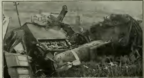
A Head-on Collision on the Cambrian Railway, Wales, Resulting from Failure of Employees to Obey Rules Under Staff System of Operation
