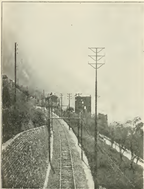
Line from Lecco to Colico, Showing Wooden Poles Used in 1901 for Supporting the Contact Wires
