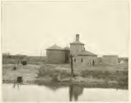
A 10,000 Gal. per Hour Intermittent Softener
