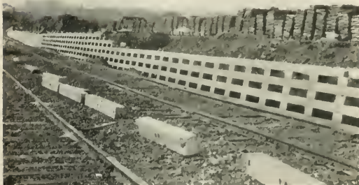
Constructing the Concrete Cribbing Along the Loading Dock
