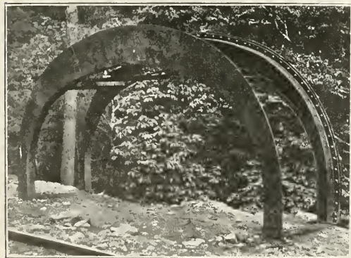
A Pair of the Tunnel Shield Arches Before Applying the Lagging
