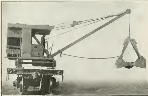
The Truck Body Can Be Shifted on the Axles, Reducing the Clearance to 6 ft. 6 in.
