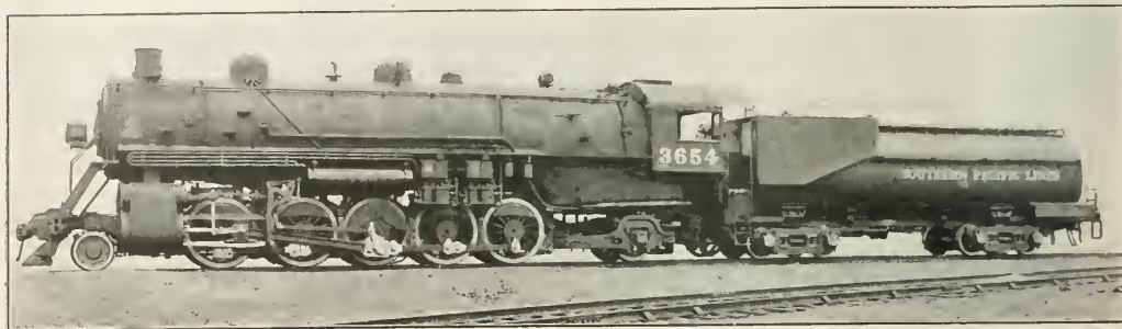
Santa Fe Type Locomotive for Handling 1,000 Tons on 2.4 Per Cent Grades
