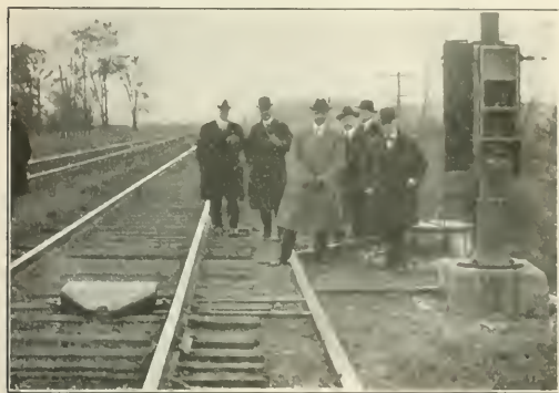
G. R. S. Automatic Train Control—Track Member
