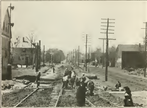
Laying the New Temporary Track Alongside of the Old Line
