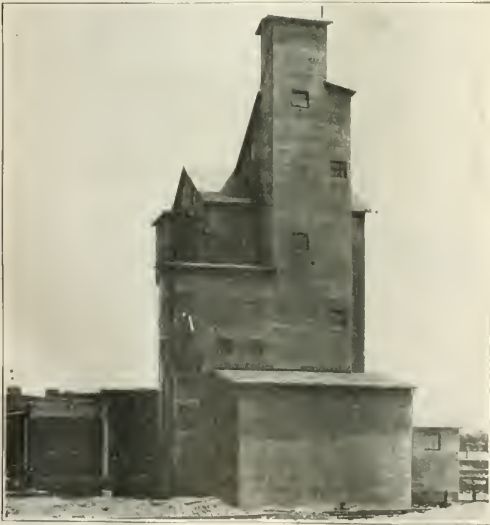
The Plant from the Receiving Track Side Showing the Concrete Cover Over the Track Hopper
