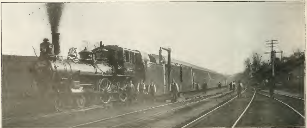
Experimental Train on the Baltimore & Ohio in 1900 Designed to Reduce Atmospheric Resistance
