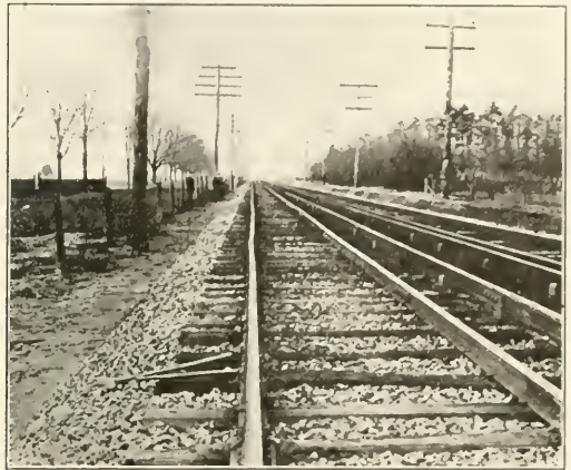
Fig. 11. Tangent Track Kinked by Electric Locomotive No. 10,002
