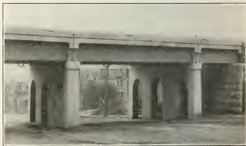
Street Subway in Montreal Involving the Use of 36 Ft. Slabs for the Roadway Spans
