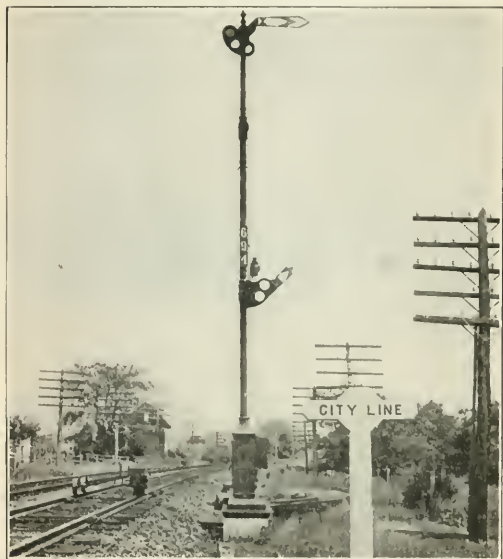
Fig. 1. Baltimore & Ohio Automatic Block Signal with Auxiliary Arm
