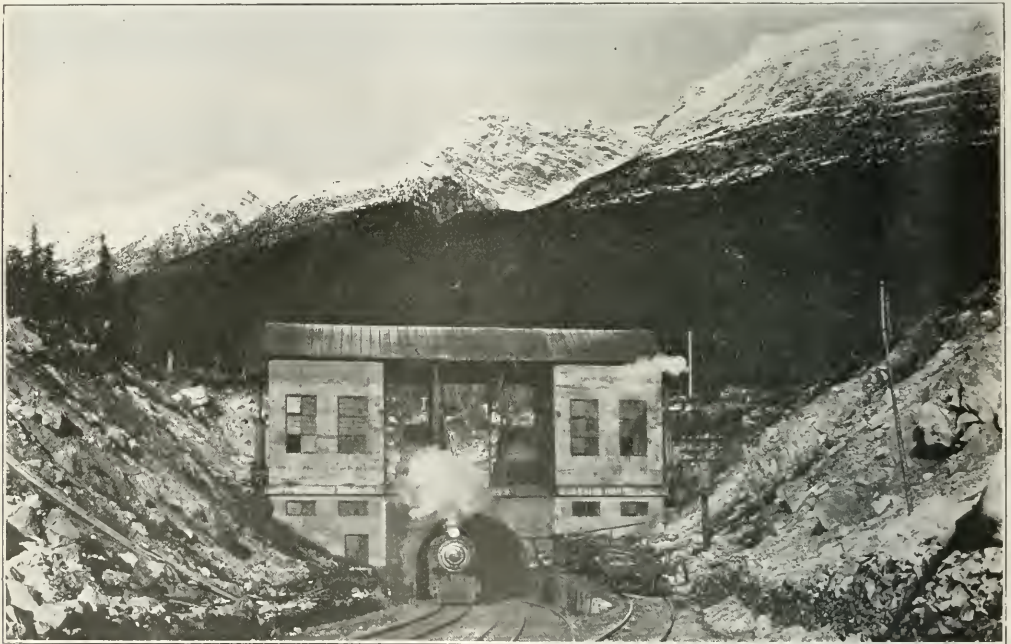
West Portal of Tunnel, Showing Fan House and Fans; Selkirks Mountains in the Background
