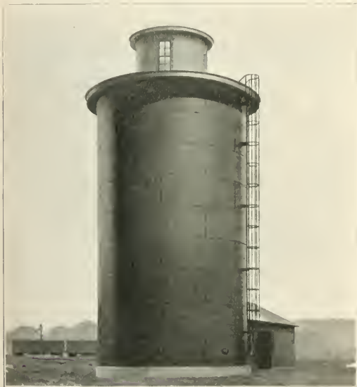
A 10,000 Gal. per Hour Continuous Softener
