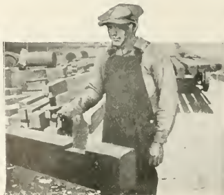
Brush treating mortise of timber which was framed after creosoting
