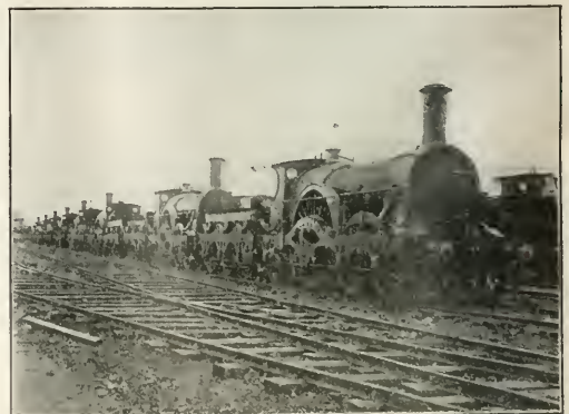
Scrapped Because of Excessive Size When Seven-foot Gage Was Abolished. Great Western, England, 1892.
