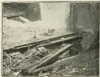
Decayed intermediate sills and flooring
