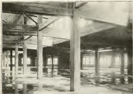
Interior View of Second Floor of North Unit. Floor in Process of Curing
