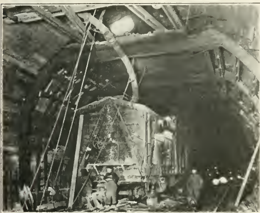
View Showing Pioneer Form, also Mixing Apparatus Ready for Placing Concrete
