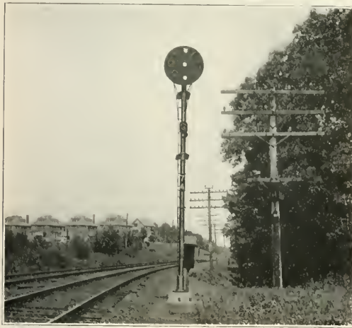
Position-Light Signal with Circular Background
