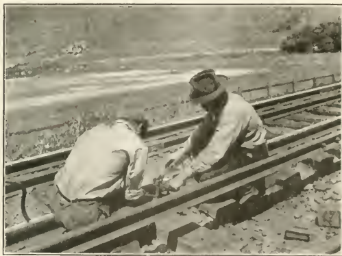
Soldering Bonds on the Running Rail. Third Rail Is Shown in Foreground
