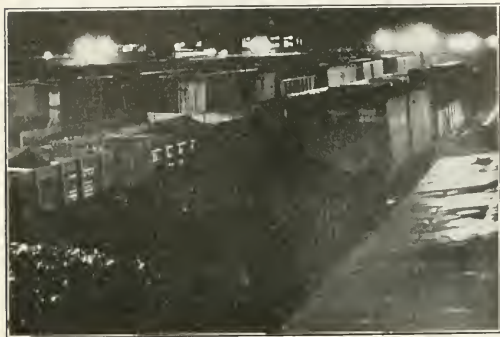
Fig. 7.—Night View of Yard Lighted by 600 c. p., 6.6-20 Ampere Series Mazda C Lamps in Dome Reflectors and Rippled Globes, Mounted 22 Ft. High and Spaced Approximately 175 Ft. Apart
