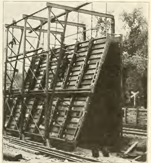
One of the Steel Forms Which Is Being Used Between the Old Line and the Temporary Tracks
