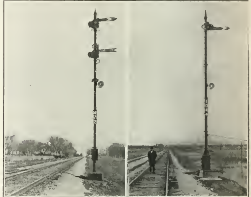
Fig. 4—Illinois Central.—On the left a lower quadrant signal; on the right, an upper quadrant.
