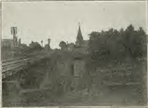
Fig. 3. Another Sambre Bridge in Belgium. Temporary Trestle for One Track While the Permanent Bridge, at the Right of the Picture, Is Being Rebuilt. Here Both Piers and Abutments Are of Masonry
