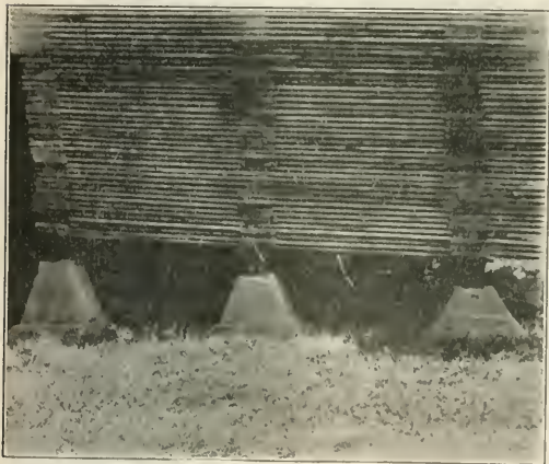
Concrete Foundation Piers and Timber Sills
