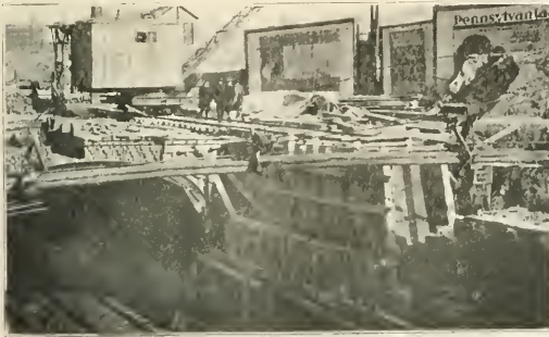
The Concrete Work Was Kept Close Up to the Masonry
