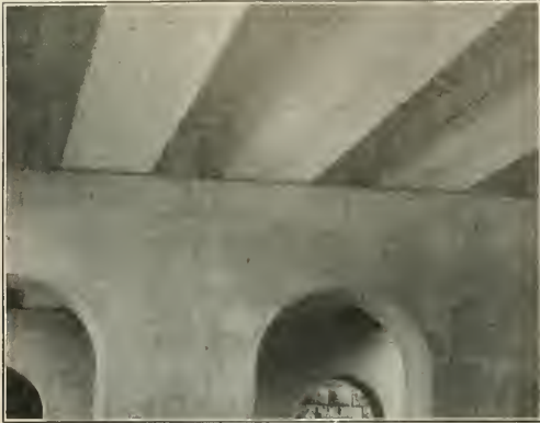
View Underneath, Showing the T-Beam Construction
