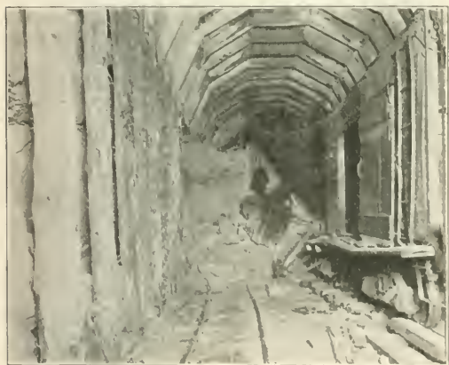
Clearing Out the Bench in the St. Alban's Tunnel
