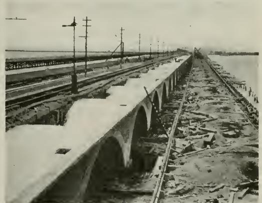
Filling on Portion of the Arches First Completed Was Held by a Temporary Retaining While Remaining Section Was Being Built
