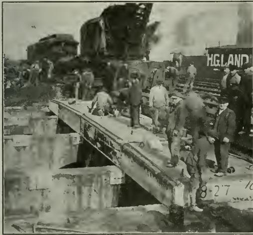
Placing the Slabs in Position—Note the Shoulder on the Slabs for the Protection Coating
