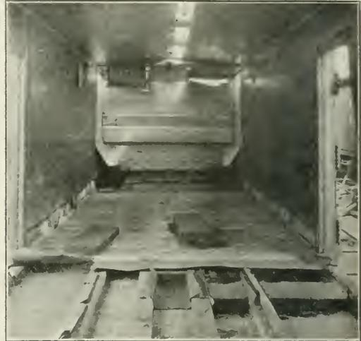
Fig. 5—Method of Applying Insulation and Waterproofing in Floor
