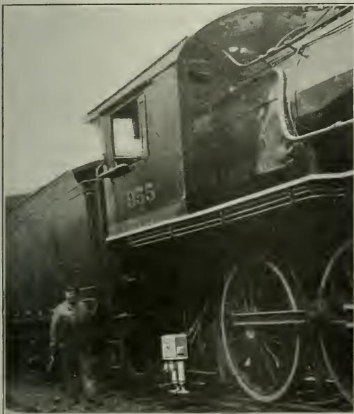
Automatic Stop Apparatus on Locomotive 955
