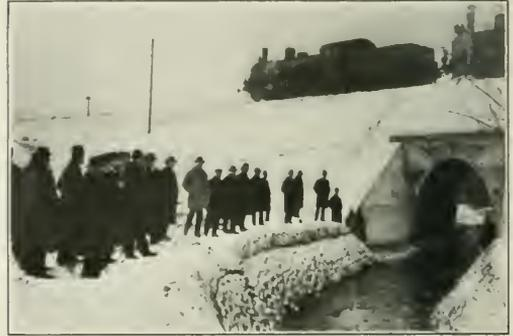
A Fill and Culvert on the New Line
