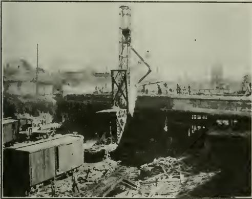
The Mixer Plant at Work, Vacant Track on the Right Reserved for Material Cars and Locomotive Crane
