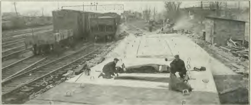
Waterproofing the Pre-Cast Slabs on the Casting Platforms
