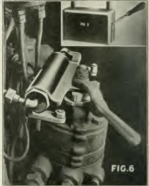
Automatic Cylinder on Brake Valve and Acknowledging Contactors
