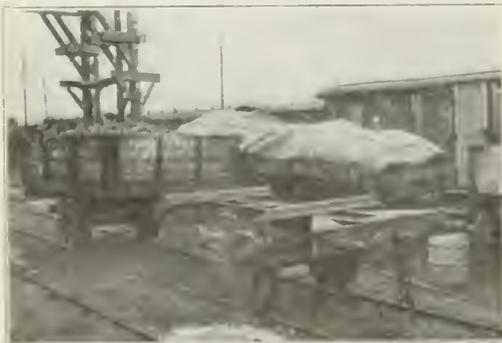
A Polish Container Car for Coal Service; One Section of Body Removed to Show Construction of Underframe
