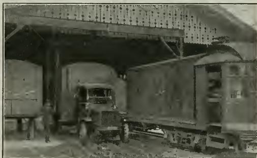
Container Ready to Be Removed from Motor Truck Chassis
