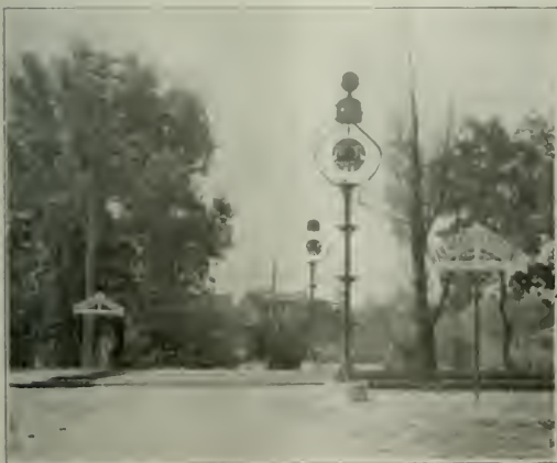
Highway Protected by Signs and Movable Visible Audible Signals
