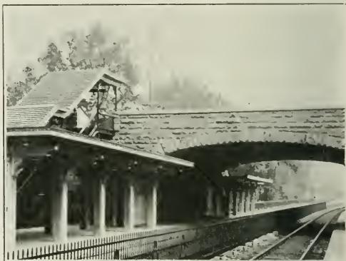
Fig. 13—A Stone Faced Concrete Arch at Glen Ridge, N. J.
