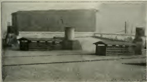
Alternate Installations of Two Types of Smokejacks
