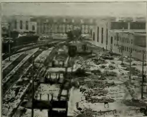
The Arrangement of the Three Ashpits on the Inbound Tracks
