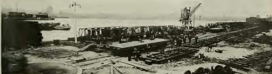
Erecting American 30-Ton Cars at Danzig
