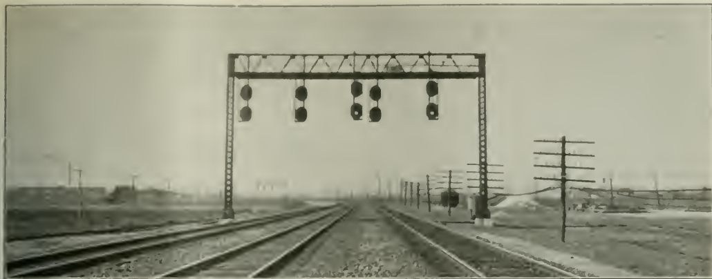
Looking Westward with Both Reversible Track Signals Showing Green (White in Illustration)
