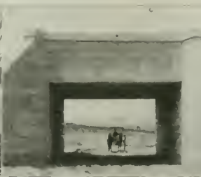
Three Types of Undercrossings Fig. 7—Flat Top for Limited Clearances
