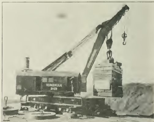
The New Crane Has a Capacity of 400,000 lb.
