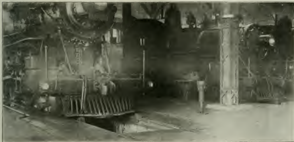
Boiler Washout Section, Showing Depressed Drains, Post Cranes, Etc.
