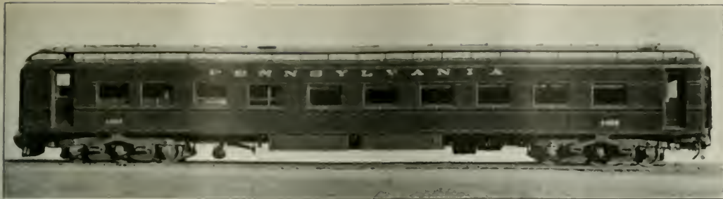
Latest type 12-in. I-beam car for the Pennsylvania System
