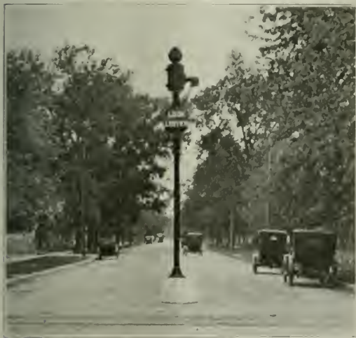
Three-Position Wig-wag and Audible Warning Signal Located in Center of Street
