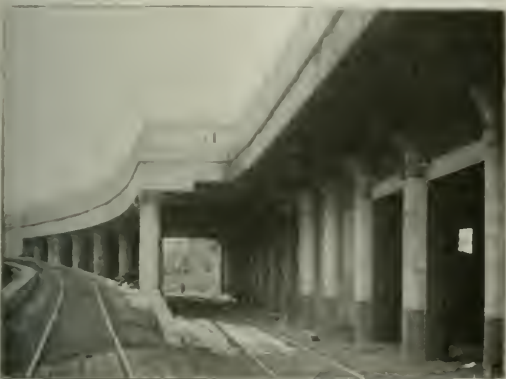
Fig. 4—Showing Flat Slab Construction at Buffalo
