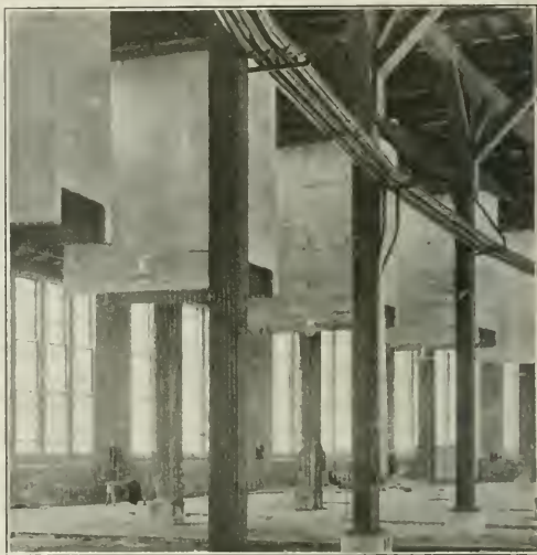
Fig. 47—Reinforced Concrete Smoke Jacks in a Roundhouse at Scranton, Pa.
