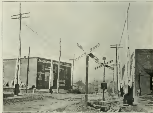
Audible Warning, Crossing Signs and Gates Protect This Crossing
