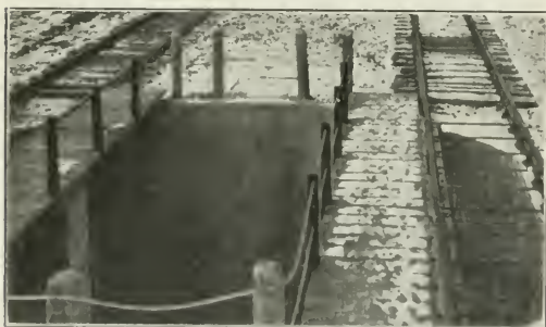
One of the Wet Ashpits Before It Was Placed in Service
