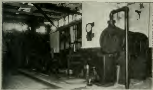
Fig. 1—The Test Plant, Showing Boiler (at left), Booster and Condenser
