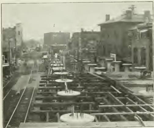
The "Neck of the Bottle" Looking North East, Temporary Tracks on the Left, New Three-Track Concrete Viaduct on the Right
