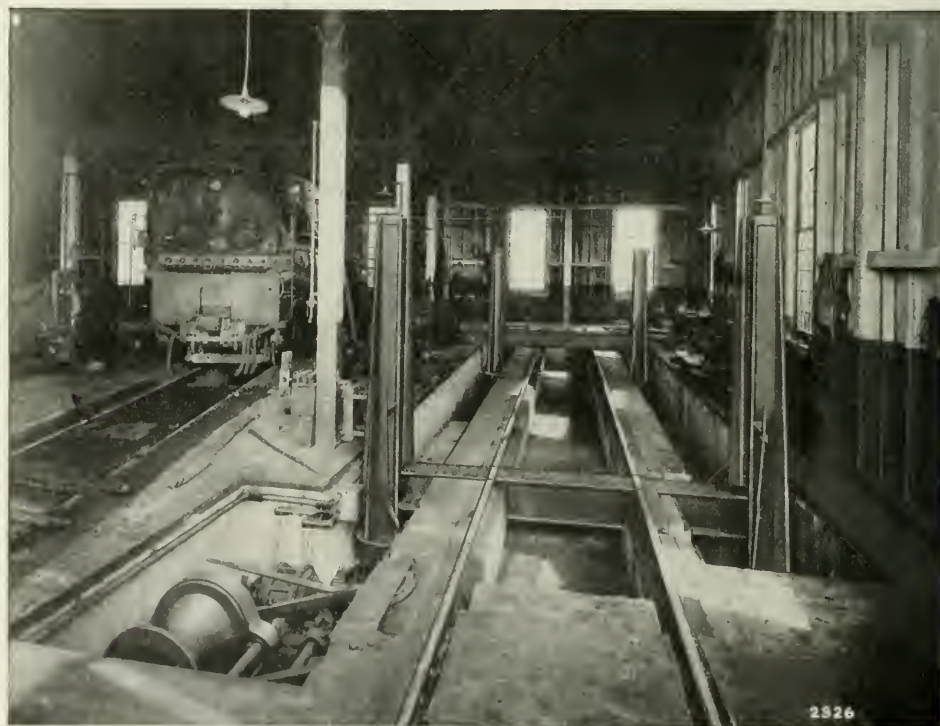
End view of Four-Jack Locomotive Hoist showing lifting beam lowered into slot in foundation; hauling winch in foreground. Lehigh Valley R. R., Lehigh, Pa. This company is using six Whiting Hoists
