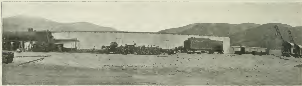
Erecting 2-10-2 Locomotives, Built by Baldwin
