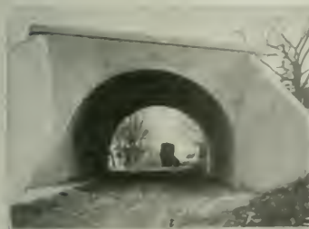
Fig. 6—Typical 30-ft. Semi-Circular Arch
