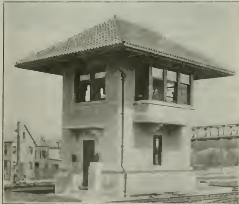
Fig. 36—An Admirable Application of Concrete to a Signal Tower at Montclair
