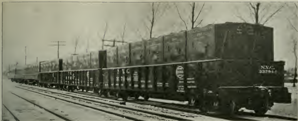
Gondola Cars with Slight Modifications Are Well Adapted for Holding Containers
