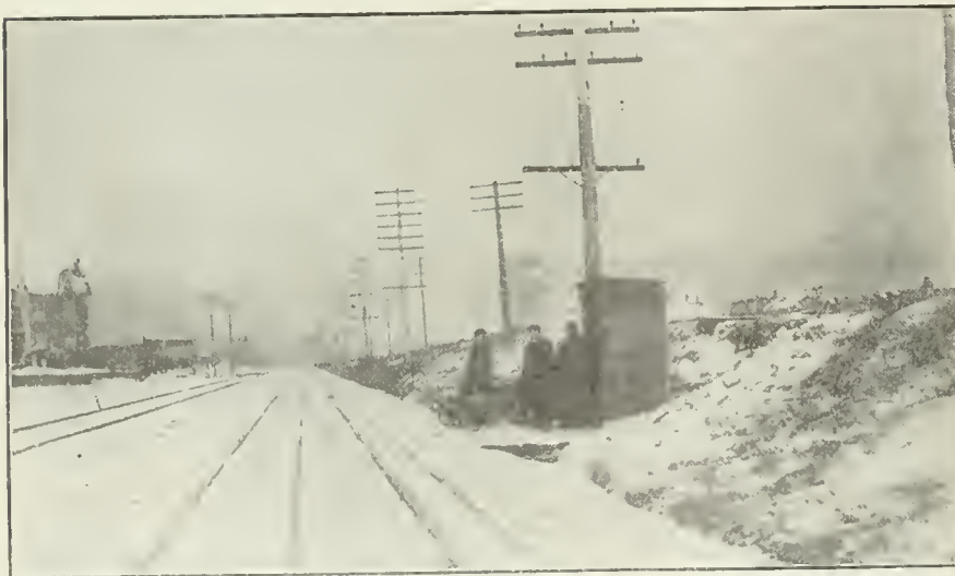
TRACK. GENERATOR BOX, "WAVE WIRE" IN CENTRE, AND "PICK UP" AT END OF TIES.
