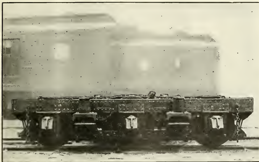
NEW PENNSYLVANIA STEEL CAR, SIX-WHEELED TRUCK.
