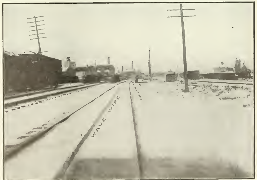
TRACK SHOWING WAVE WIRE AND PICK-UP WIRE.
