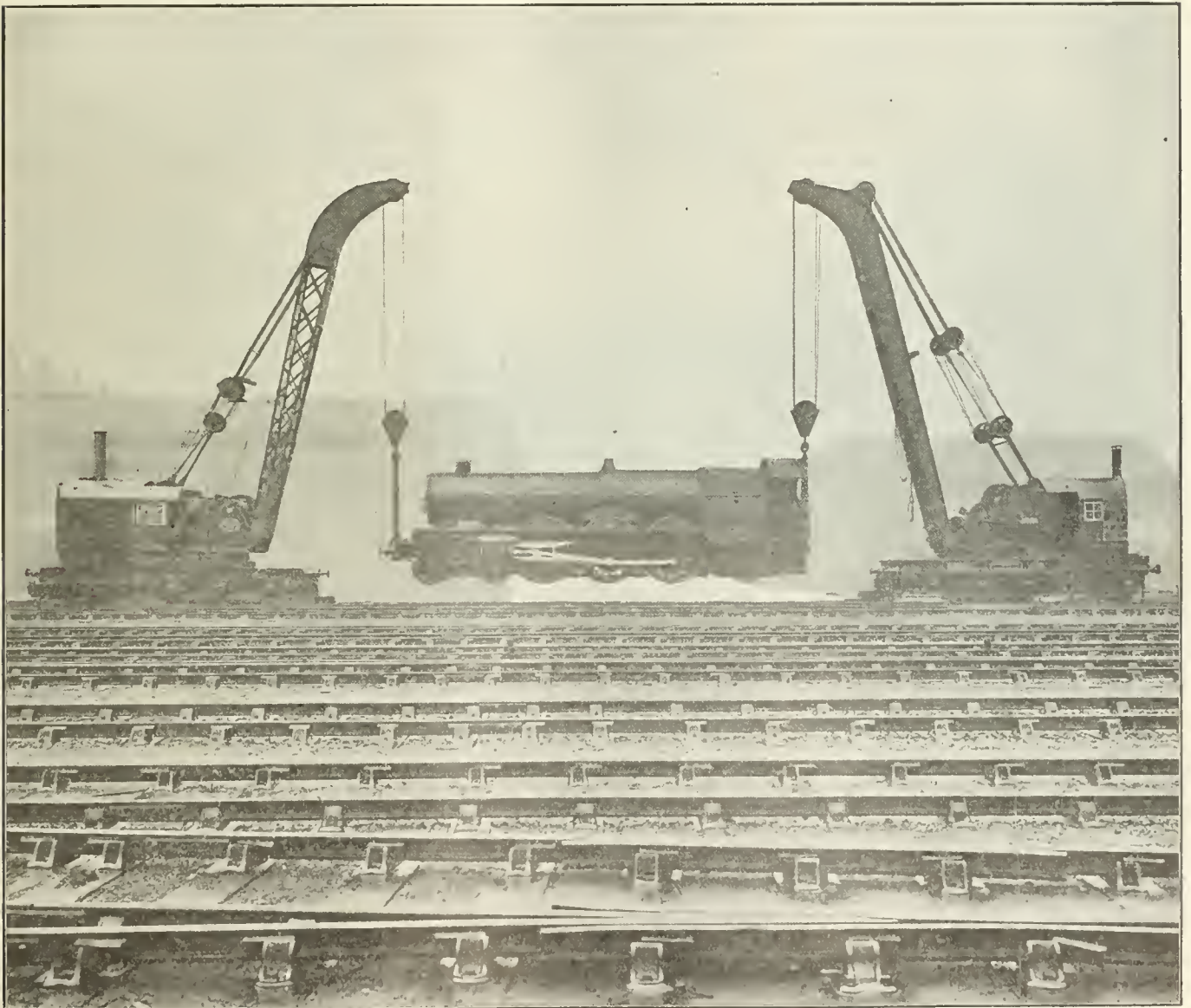
GREAT WESTERN ENGINE "GREAT BEAR," WEIGHING 194,884 LBS., LIFTED BY TWO WRECKING CRANES.
