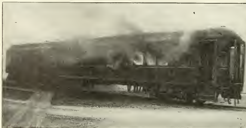
PENNSYLVANIA PASSENGER STEEL CAR DURING FIRE TEST.
