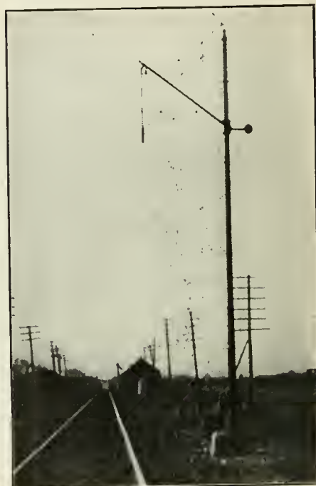
SIGNAL CLEAR AND SWINGING CONTACT UP.
