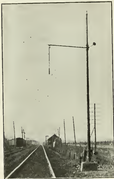
SIGNAL STOP. SWINGING CONTACT DOWN.
