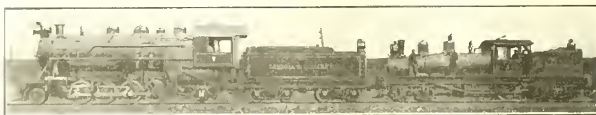
LIMA "SHAY" SWITCHER COUPLED TO CAMBRIA & INDIANA 2-8-2 USED AS THE "LOAD."
