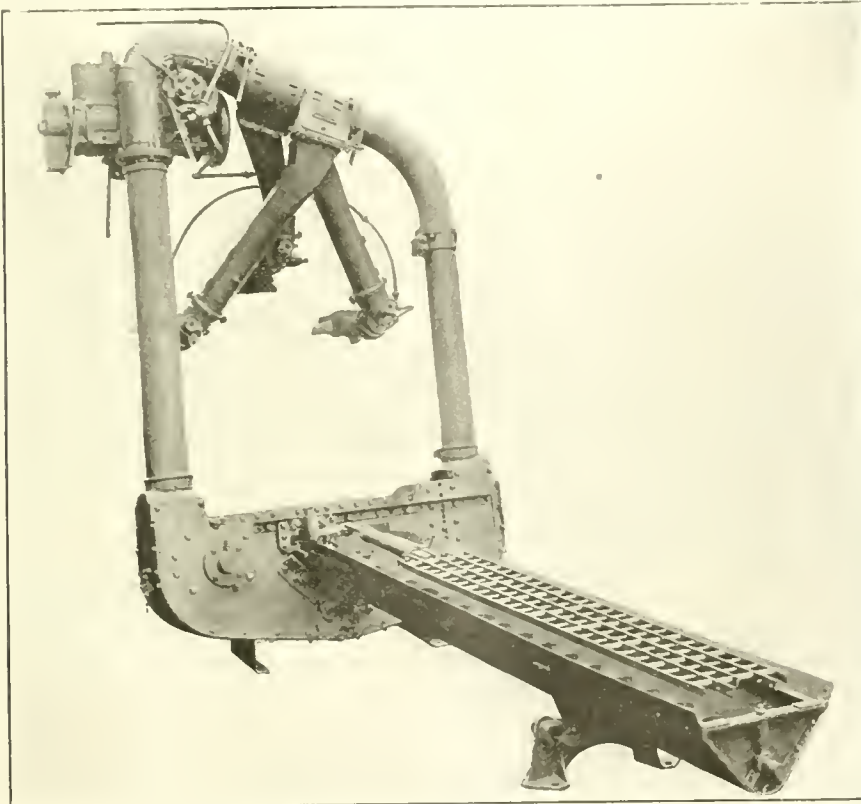
MECHANISM OF THE STREET LOCOMOTIVE STOKER.
