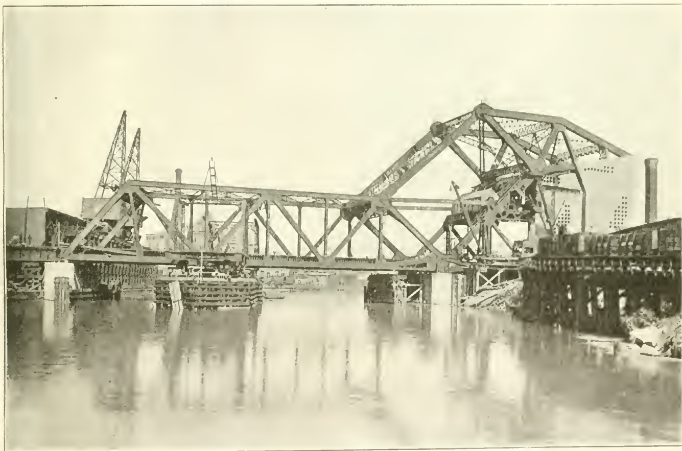
CHICAGO & NORTH WESTERN RAILWAY BASCULE BRIDGE OVER THE CHICAGO RIVER NEAR DEERING, ILL. VIEW SHOWS BASCULE BRIDGE IN POSITION, READY FOR TRAFFIC
