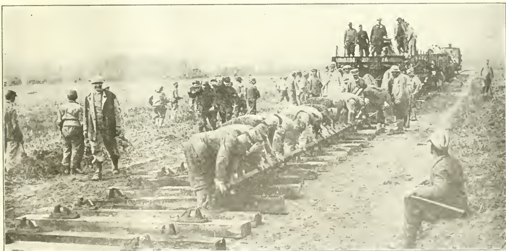
ALLIED ENGINEER REGIMENT LAYING RAILS BEHIND THE BATTLE LINE IN FRANCE
