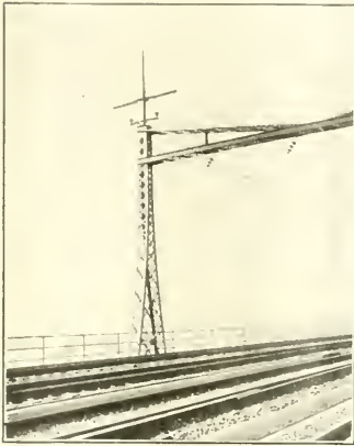
TROLLEY BRIDGE ON VIADUCT WITH LATTICE POST.
