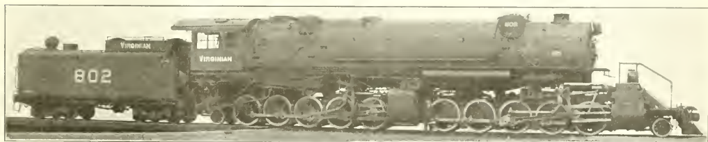
HEAVY MALLET LOCOMOTIVE FOR THE VIRGINIAN RAILWAY
