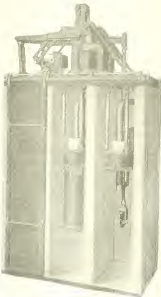
FIG. 1. FRONT VIEW OF CIRCUIT BREAKER
