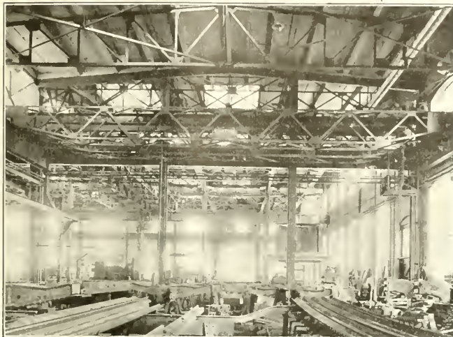
OVERHEAD SHOP CRANE WITH LATTICE GIRDERS AND SAFETY DEVICES.
