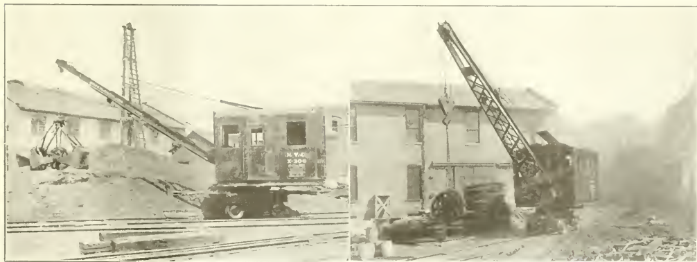
GASOLINE CRANES USED FOR HANDLING COAL, ASHES AND MATERIAL, N. Y. C. LINES
