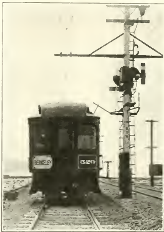
CAR WITH DEAD MAN'S HANDLE STANDING AGAINST STOP SIGNAL.
