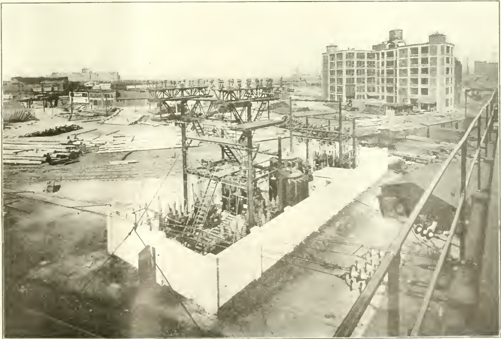
OUTDOOR TRANSFORMER STATION AT NORTH PHILADELPHIA—P. R. R. ELECTRIFICATION
