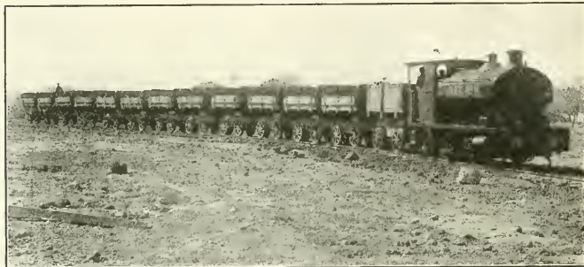
FIG. 1. CONSTRUCTION TRAIN ON BOMBAY DEVELOPMENT FITTED WITH M. C. B. COUPLERS
