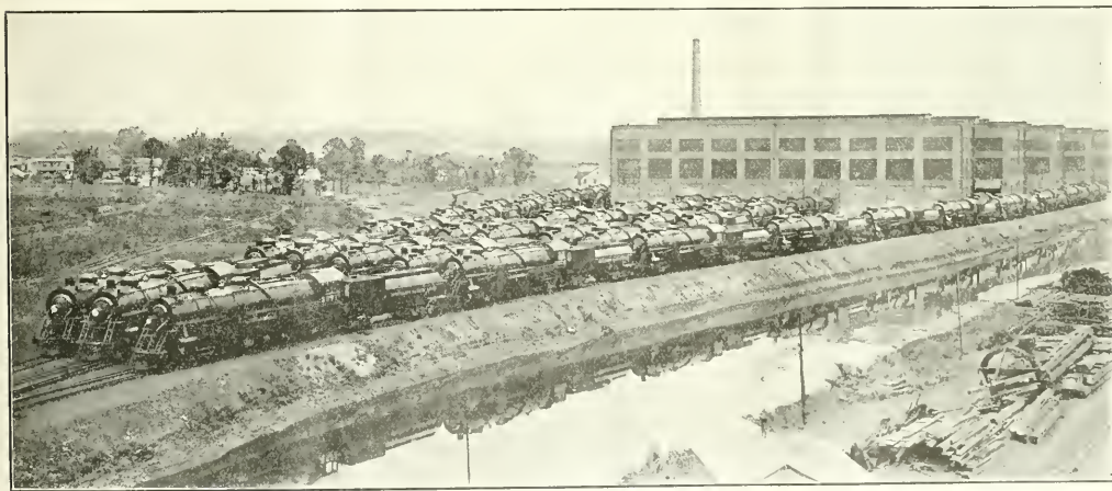
FIFTY 2-10-2 TYPE LOCOMOTIVES FOR THE SOUTHERN PACIFIC LINES ASSEMBLED AND READY FOR DELIVERY AT THE BALDWIN LOCOMOTIVE WORKS
