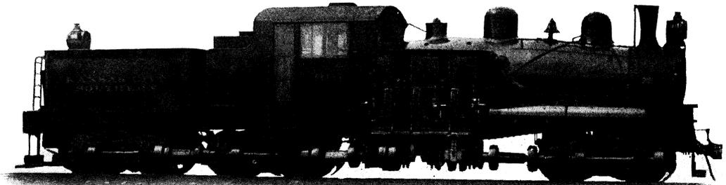
FIG. 2. 140-TON GEARED LOCOMOTIVE FOR SWITCHING ON 7% GRADES AND 60° CURVES; KANSAS CITY SOUTHERN RY.
