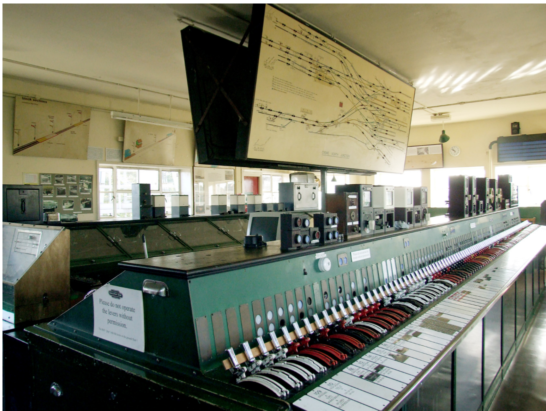
The inside of Crewe North Junction Signal Box - decommissioned in 1985. Note the track plan and the three routes radiating out from the twelve platform (track) station..
