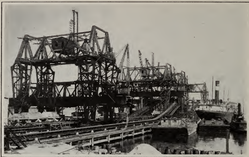
THREE OF THE LOADING TOWERS IN OPERATION. WHEN THIS PICTURE WAS TAKEN THE ONE IN THE FOREGROUND WAS IN COURSE OF CONSTRUCTION
