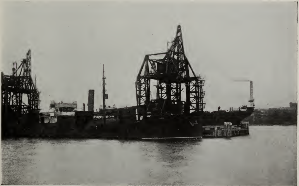
LOADING PLANT IN THE WORLD. IT HAS A LOADING CAPACITY OF 12,000,000 TONS STEEL AND IS ELECTRICALLY OPERATED
