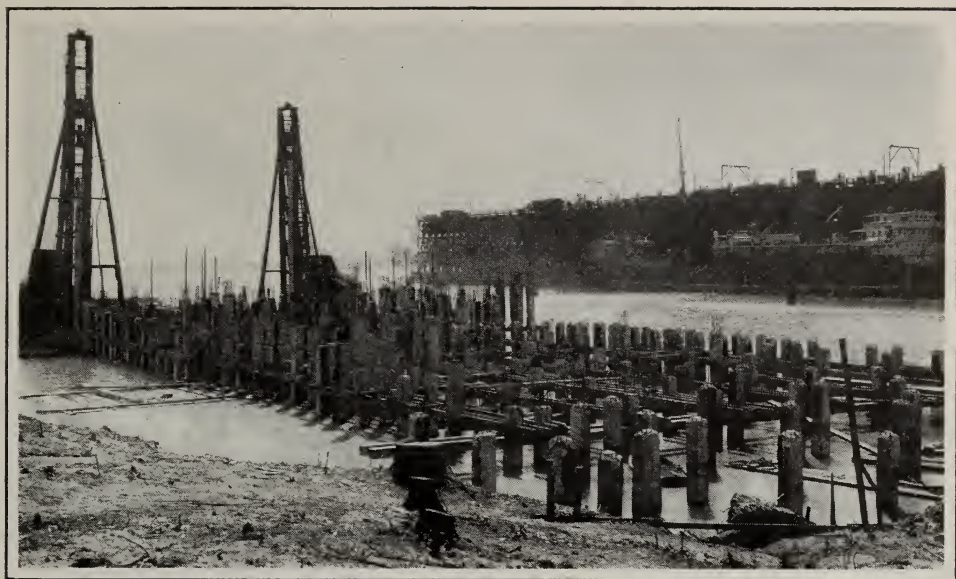
2—THE FIRST STEP IN THE CONSTRUCTION OF THE PIER. PILES IMMEDIATELY AFTER BEING DRIVEN, HELD IN POSITION BY CLAMPS
