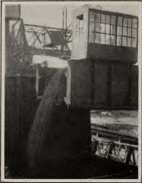
COAL BEING LOADED INTO HOLD OF VESSEL FROM LOADING TOWER
