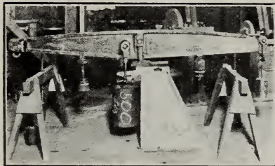
20—Middle extension lever of old type track scale arranged from sealing. Weight 300 pounds.
