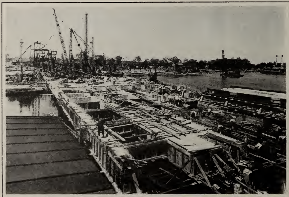
3—FOUR MONTHS LATER—THE PIER NEARING COMPLETION. THIS PICTURE SHOWS THE CONCRETE GIRDERS AND DECK WHICH SUPPORTS THE COAL LOADING MACHINERY
