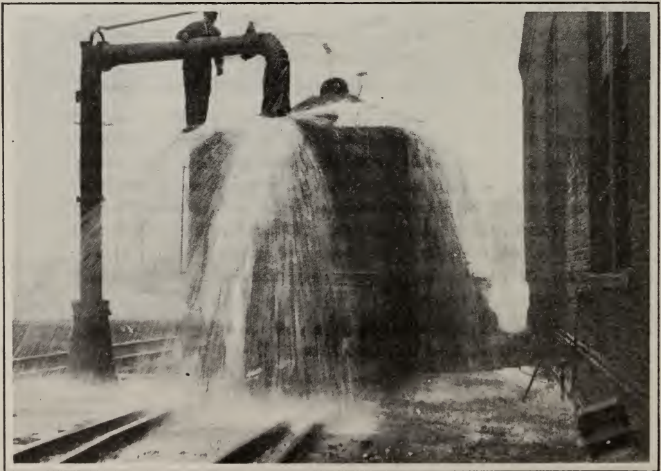
FIGURE 1—CARELESSNESS IN FILLING TANKS RESULTS NOT ONLY IN WASTE OF WATER, BUT IN DAMAGE TO TRACK
