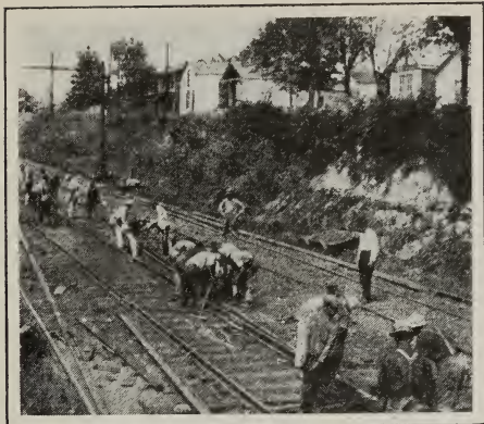
LAYING NEW RAIL EAST OF WHITMAN, IND.
