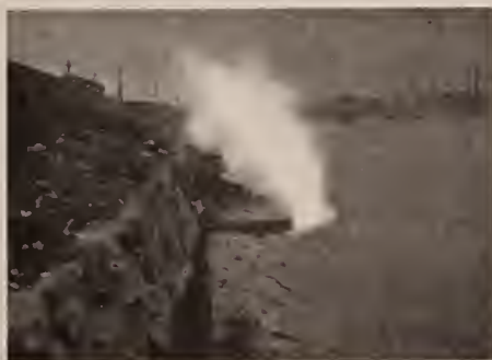
Common steam leaks which waste much coal
