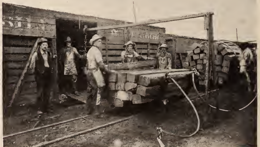
Loading treated ties for shipment, Angier tie loader. Left to right: Foreman G. C. Conley, "Jerry" Setor, Andrew Creek, "Joe" Locknar, and Andro Plen, and "Old Faithful Kate," who keeps three such crews supplied without delay
