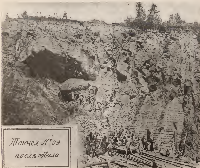
The retreating Bolsheviki did this job well—the blowing up of the railroad tunnel No. 39 along Lake Baikal. Over 50,000 pounds of powder were used for this explosion
