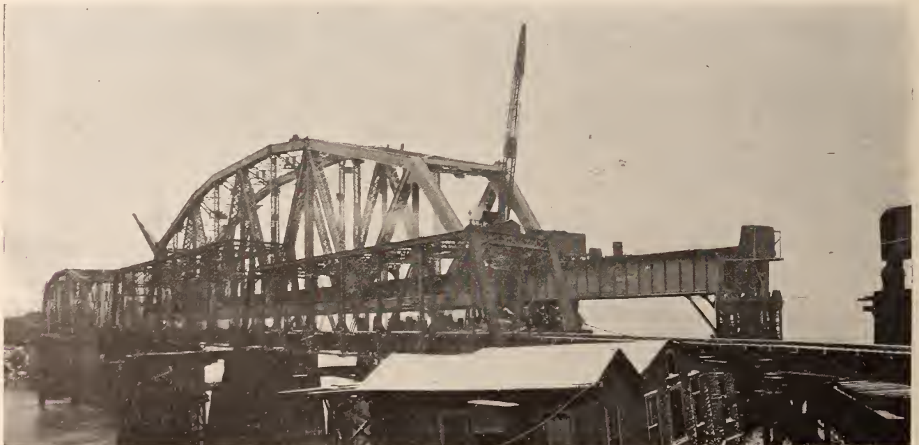
No. 2—In distance is new 261-foot truss span in place at low level. New 134-foot truss span in temporary position at high level. Traffic carried on two old truss spans in the foreground and the 261-foot span
