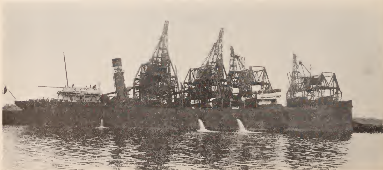
A good picture of the four loading towers. The boat was loaded so fast that the crew had just five minutes leeway in getting rid of its water ballast
