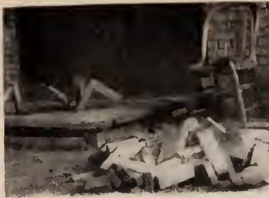
No. 3—Insecure and inadequate blocking which should not be used
