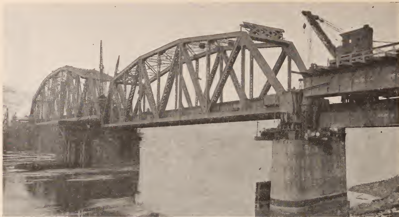
No. 5—In distance 434-foot span in final position—261-foot span being jacked approximately midway between high and low positions
