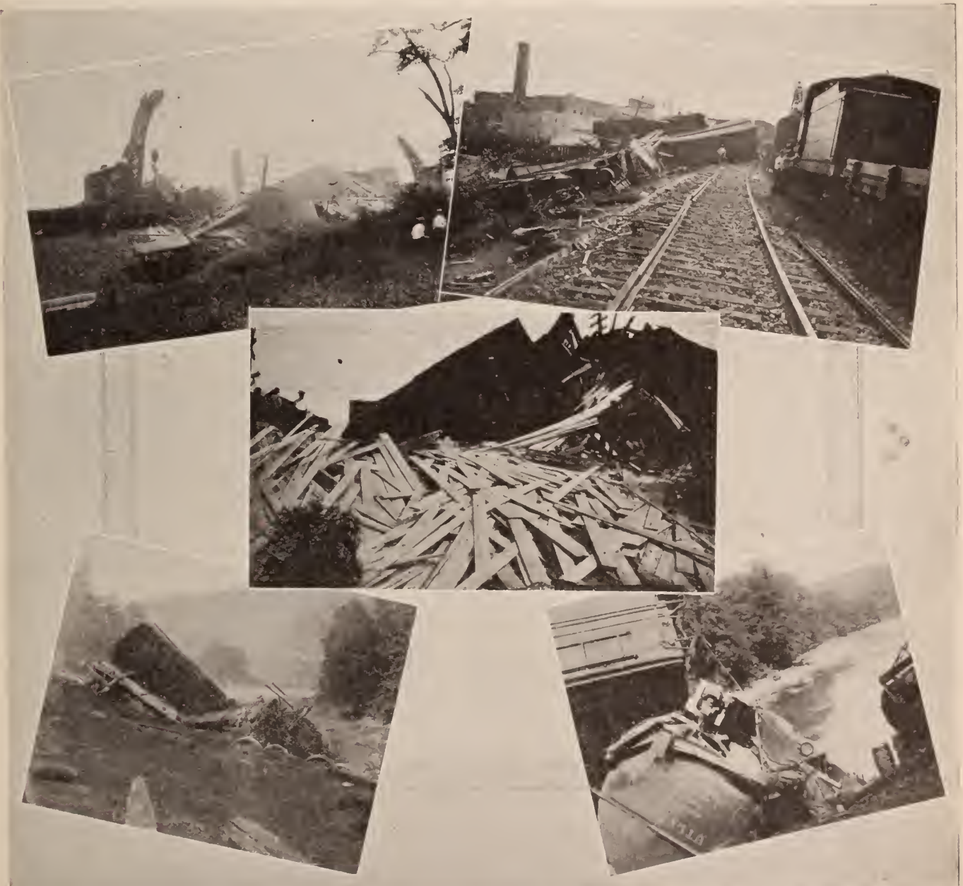
Top to bottom, left to right: Crane cleaning up the right of way; track cleared and ready for section men; lumber lost in derailment, a large part of which can be salvaged; a bad spill along a river bed; the same picture showing loss of gasoline-loaded tank cars
