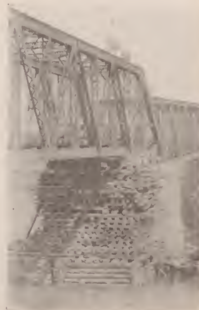
Two views of Irkut River bridge showing fallen span and process of cribbing up to track level. The River here is deep and swift
