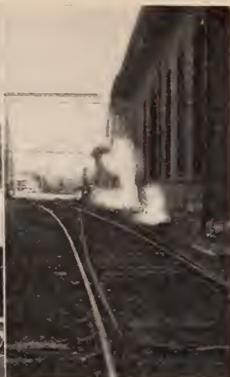
Steam leak resulting from a bare steam line buried in the ground—a great coal waster
