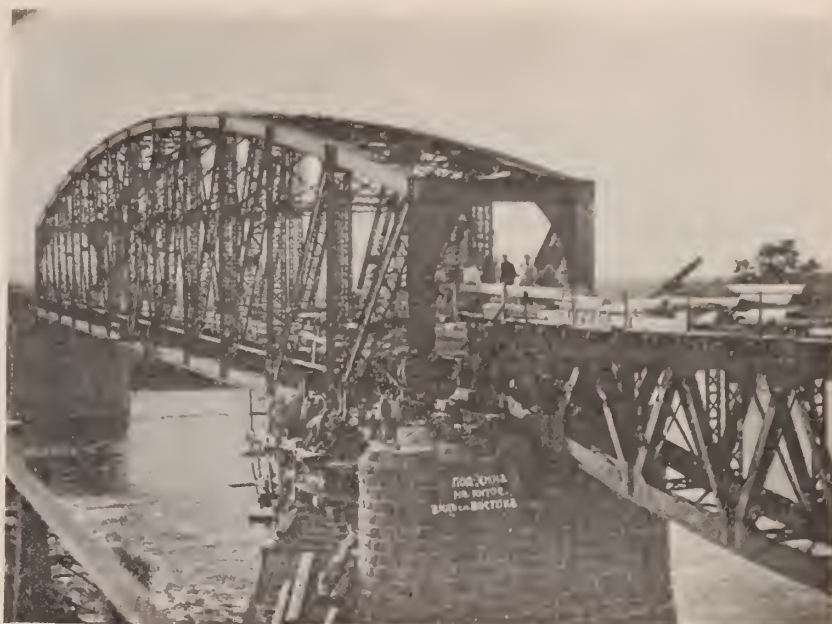
Process of reconstruction work on Kitoi River bridge. Note the cribbing up with railroad ties
