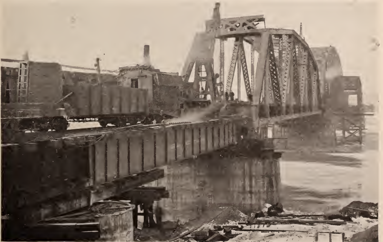
No. 4—New 434-foot truss span in final position, old truss spans rolled out and new 261-foot truss span being jacked. View taken when span was approximately five feet above low position
