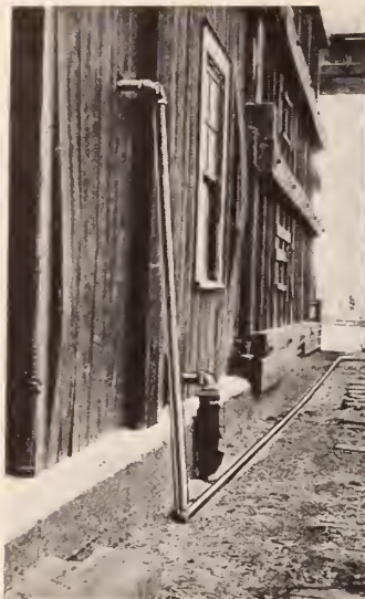
Uncovered steam lines waste coal
