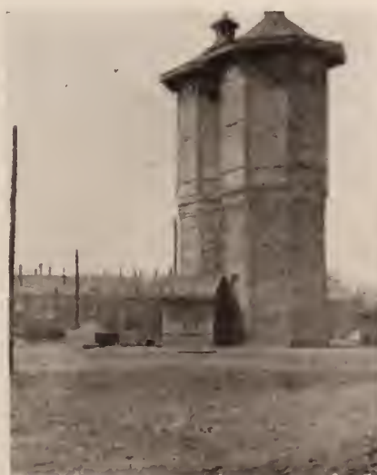
Type of water tank on Trans-Siberian Railway. At many of the smaller stations there are two of these, one at each end of the station grounds, with from three to eight stand pipes
