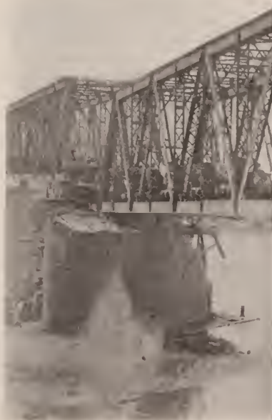
Two views of Irkut River bridge showing fallen span and process of cribbing up to track level. The River here is deep and swift
