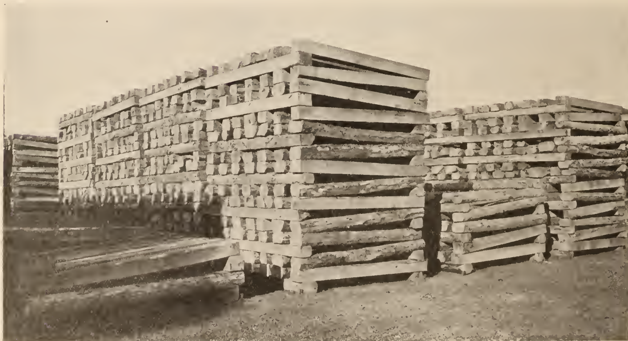
Standard method of piling ties
