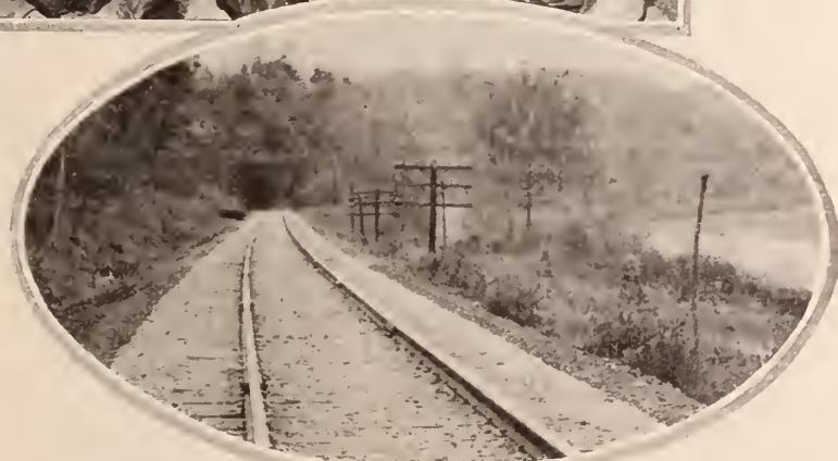
View of standard track west of No. 23 Tunnel, west end, Parkersburg Branch, Monongah Division. This is the first class B standard gravel track that Ira E. Baker and crew of Kanawha Station (as seen in the upper picture) have built in his twenty years' experience as section foreman
