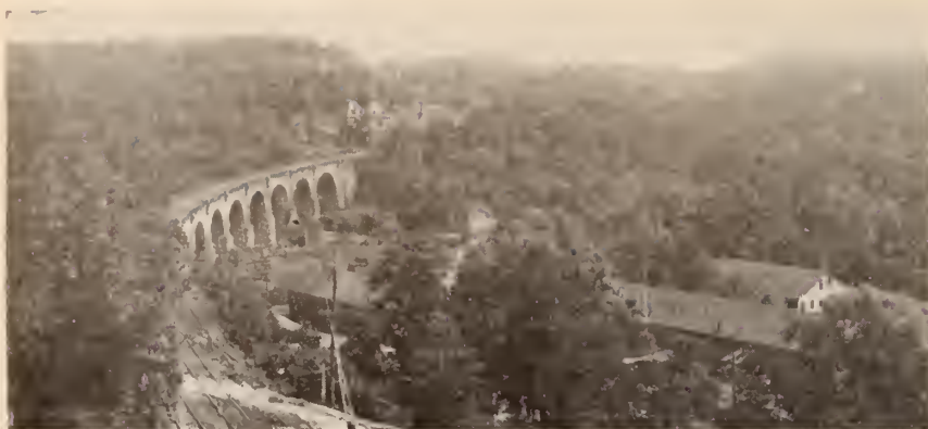
The Thomas Viaduct was once called "Latrobe's Folly," but is still in service—one of the oldest stone-arch railroad viaducts in the world
