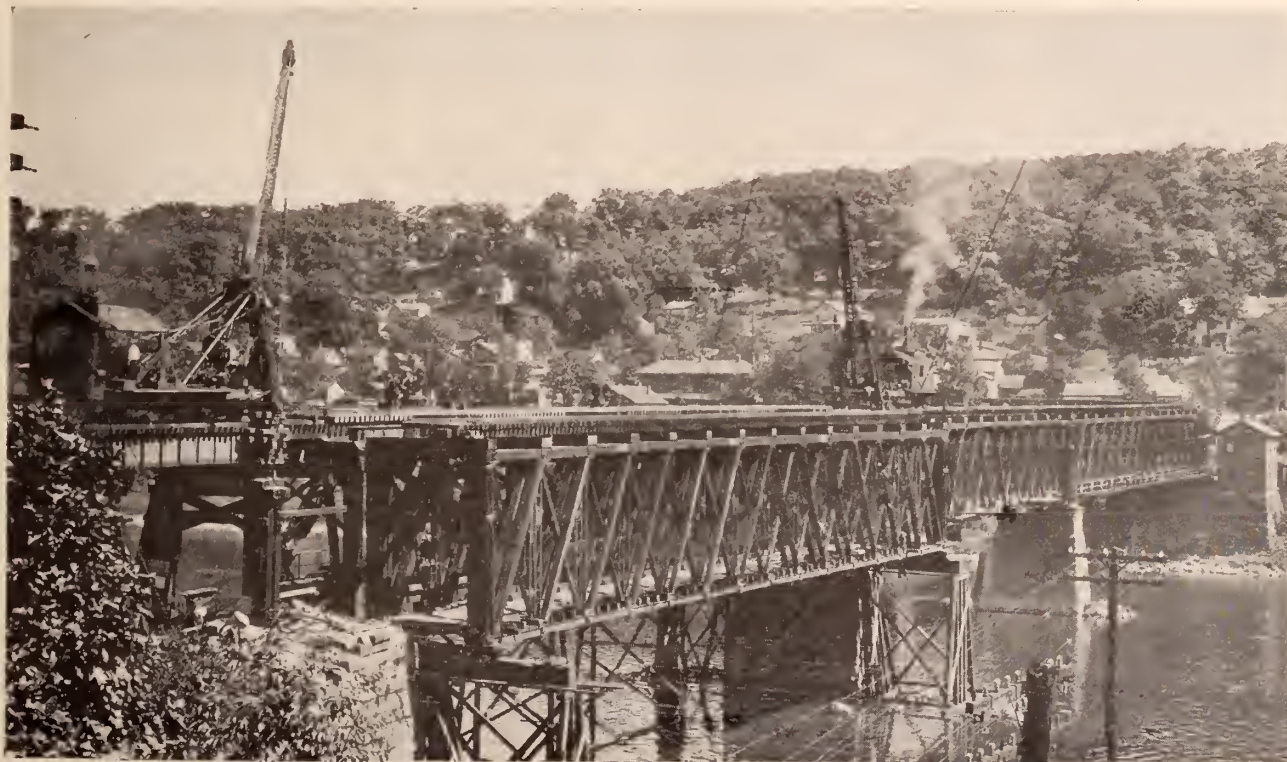
Foxburg Bridge—General view of structure from east end, after conclusion of rolling operation, August 21, showing old span in rolled-out position on falsework, and new span in place
