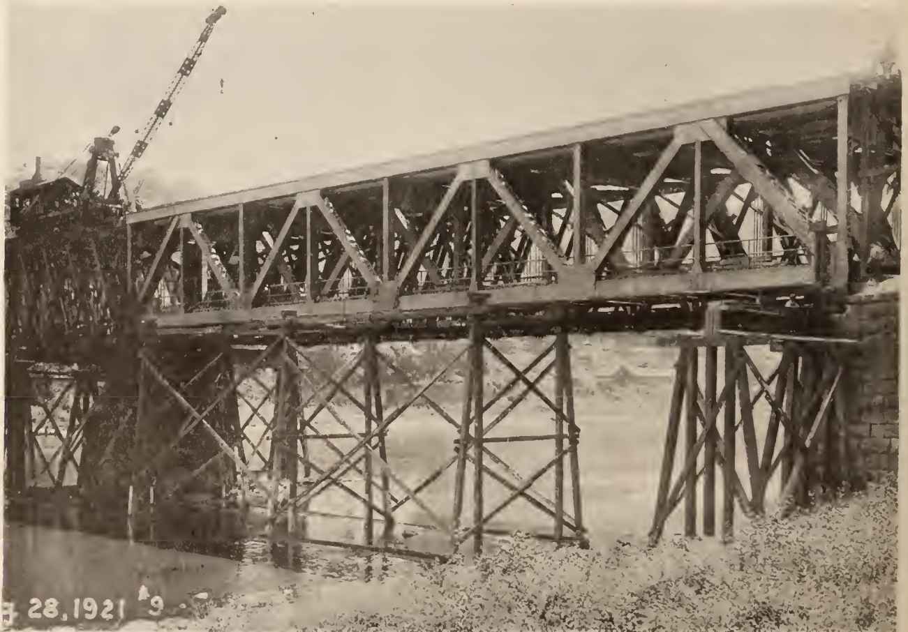
Foxburg Bridge—View from east end immediately after rolling operation on August 21, showing new east span in final position
