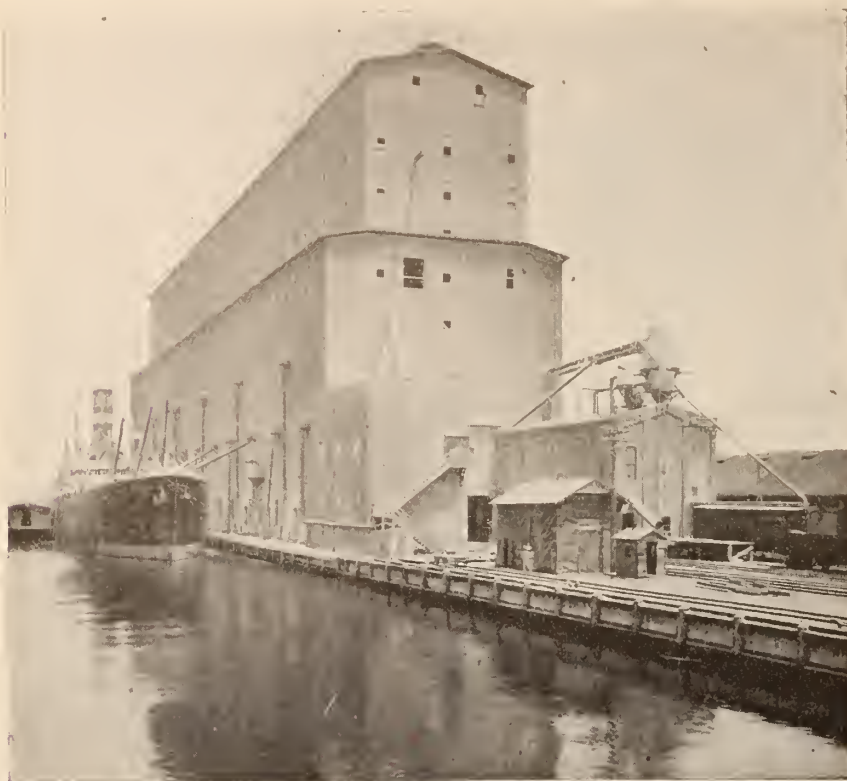
Figure 2—Elevator "C" with some of the dust collecting apparatus on top of Screening House to the right
