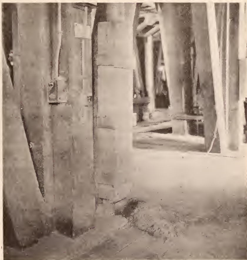
Figure 6—Typical dust collection pickup
