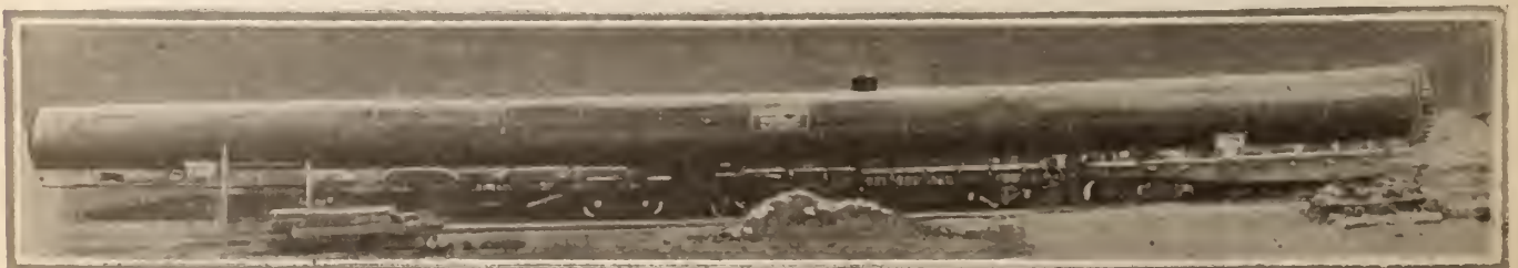
It took four flat cars to handle this creosoting tank from Indiana Harbor to Demmler—an all daylight movement
