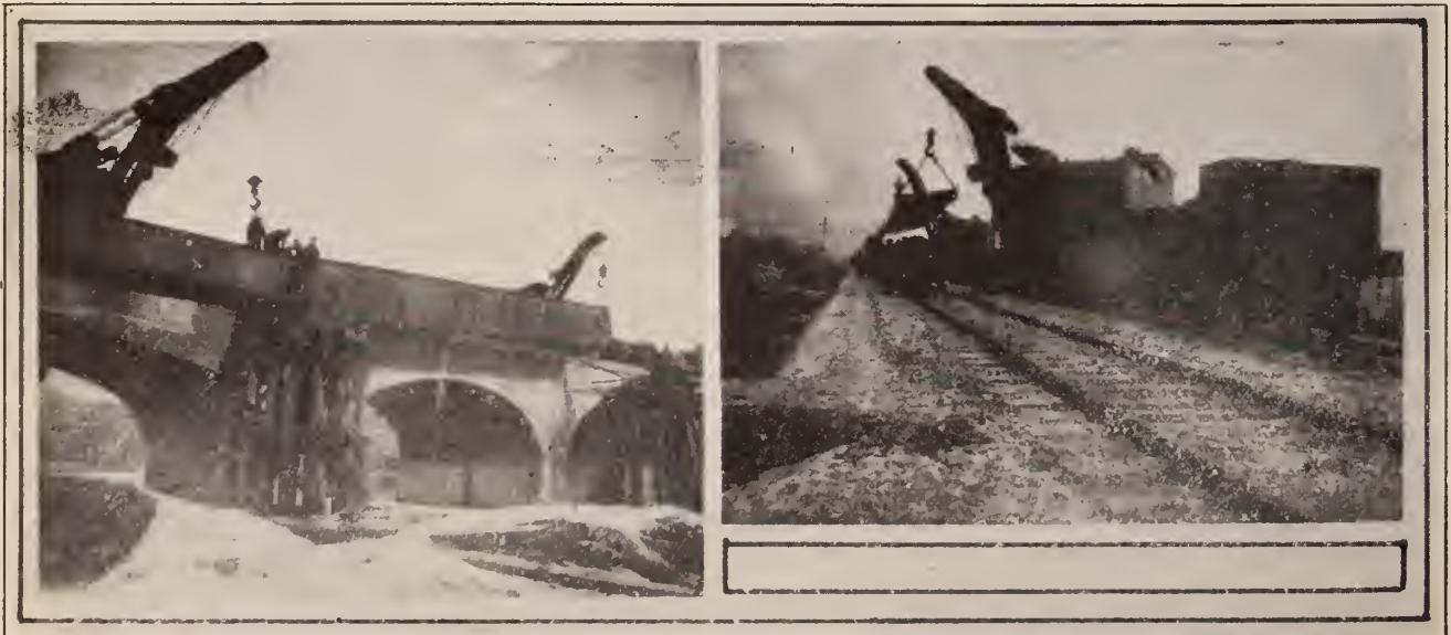
Dismantling the old trestle, which carried traffic while the bridge at Viaduct Junction was being reconstructed in 1908. This will be of particular interest to "Old Timers"
