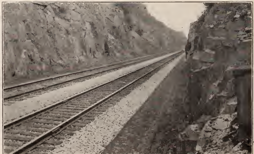
Standard track and roadbed, Havre de Grace Cut, Baltimore Division, East End
