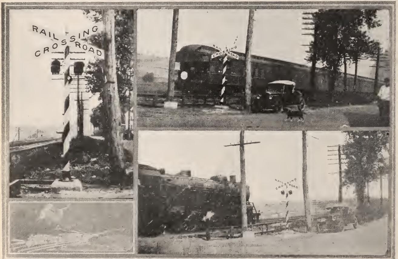
Left: Standard method of protecting highway crossing by the use of flashlight signals, Baltimore and Ohio Railroad at Lansdowne, Md. Upper right: No. 6 passing Lansdowne. Lower right: Engine of No. 506. Note the absence of smoke
