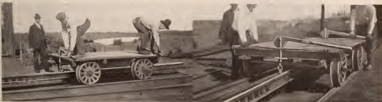
Labor saving device for lifting frogs and rails, the invention of General Foreman J. D. Drennan, Lorain Yard
