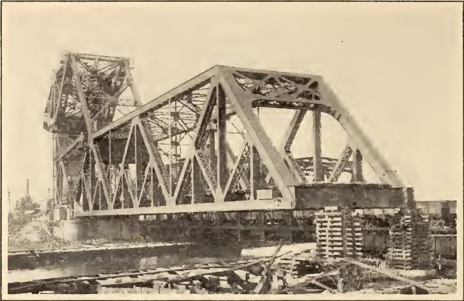
The bridge, recently completed for the Baltimore and Ohio Railroad across the Calumet River at South Chicago, is said to be the largest single leaf bascule in the world. Its span is 235 feet in
