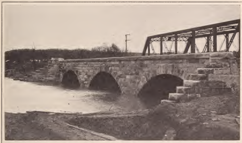
THREE TRACK STONE ARCH BRIDGE 55 OVER SLEEPY CREEK
