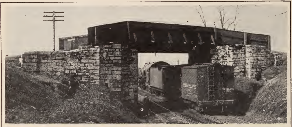
OLD FREDERICK BRIDGE, SHOWING POOR CLEARANCE FOR TRAINS, SIDE AND TOP
