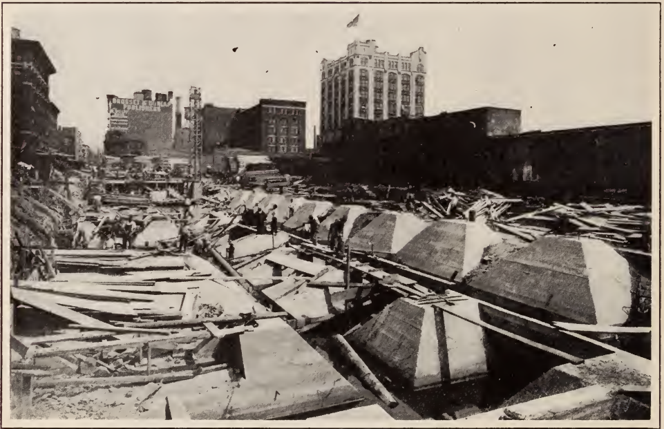
MASSIVE CONCRETE BLOCKS USED IN FOUNDATION OF NEW YORK WAREHOUSE
