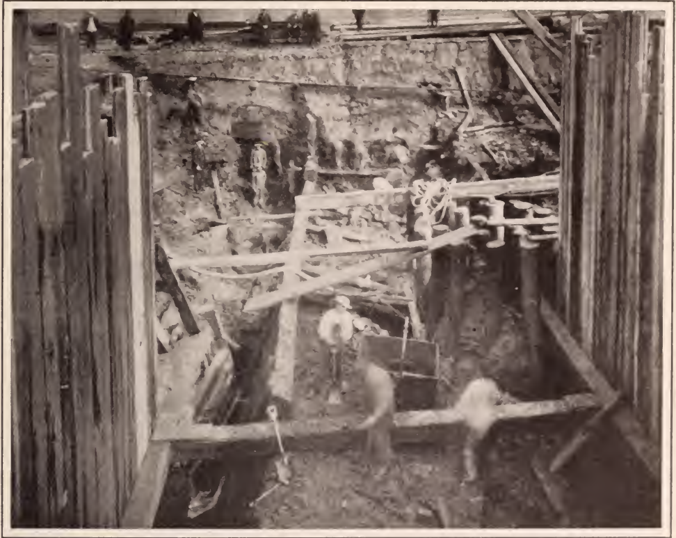
DIGGING FOUNDATION FOR WAREHOUSE
