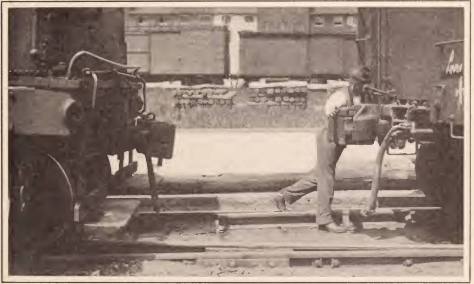
DON'T ADJUST KNUCKLE WHEN CARS ARE COMING TOGETHER. MR. WILLARD HAS SAID HE WOULD RATHER HAVE CARS BUMP ANY NUMBER OF TIMES THAN TO HAVE THIS PRACTICE CONTINUED
