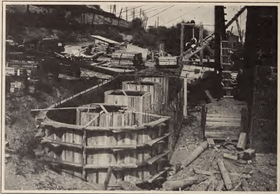
BRIDGE 74, FIG. 3, SHOWING SECTION OF FORMS AND REINFORCING RODS IN PLACE
