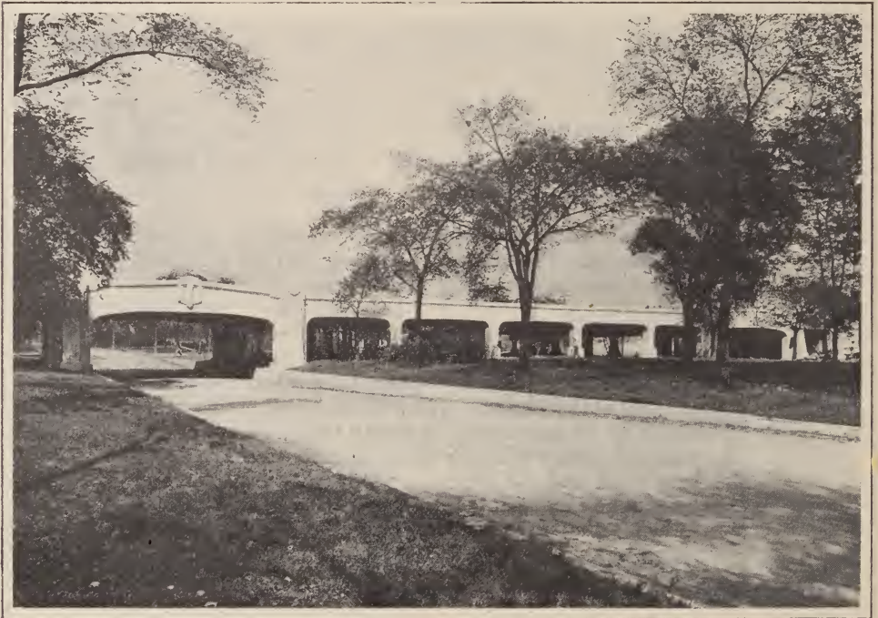
BALTIMORE AND OHIO CHICAGO TERMINAL RAILROAD BRIDGE OVER INDEPENDENCE BOULEVARD—STEEL BRIDGE WITH BOTH SIDES ENCLOSED IN CONCRETE
