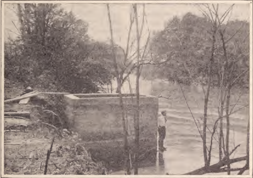
INTAKE AT POTOMAC RIVER FOR SUPPLYING WATER TO THE TIMBER TREATING PLANT AND MAIN LINE ENGINES PASSING GREEN SPRING
