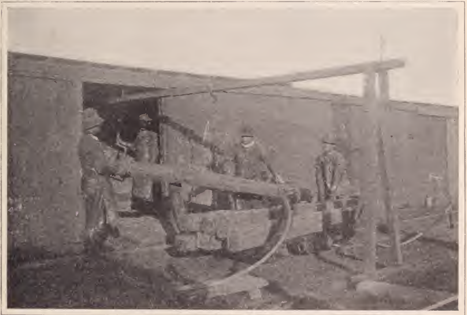
THE ANGIER TIE LOADER IN OPERATION AT GREEN SPRING
