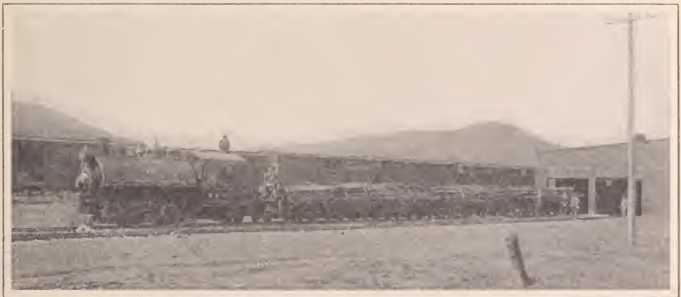
PULLING A CHARGE OF TREATED TIES FROM RETORT
