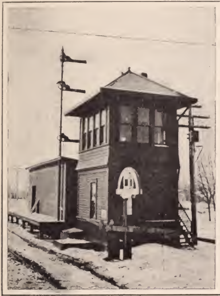
TWELVE LEVER INTERLOCKING PLANT AT PRINCESS BAY, S. I.
