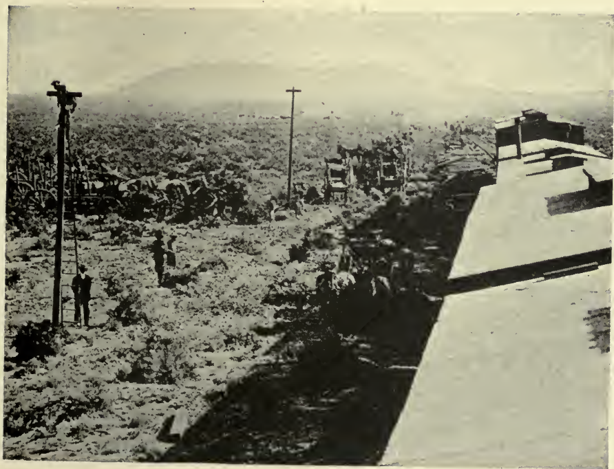
BUILDING THE TELEGRAPH LINE Central Pacific R. R., Humboldt Desert, 1868
