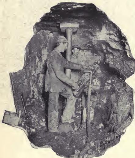
DRILLING IN A TUNNEL, QUARTZ MINING
