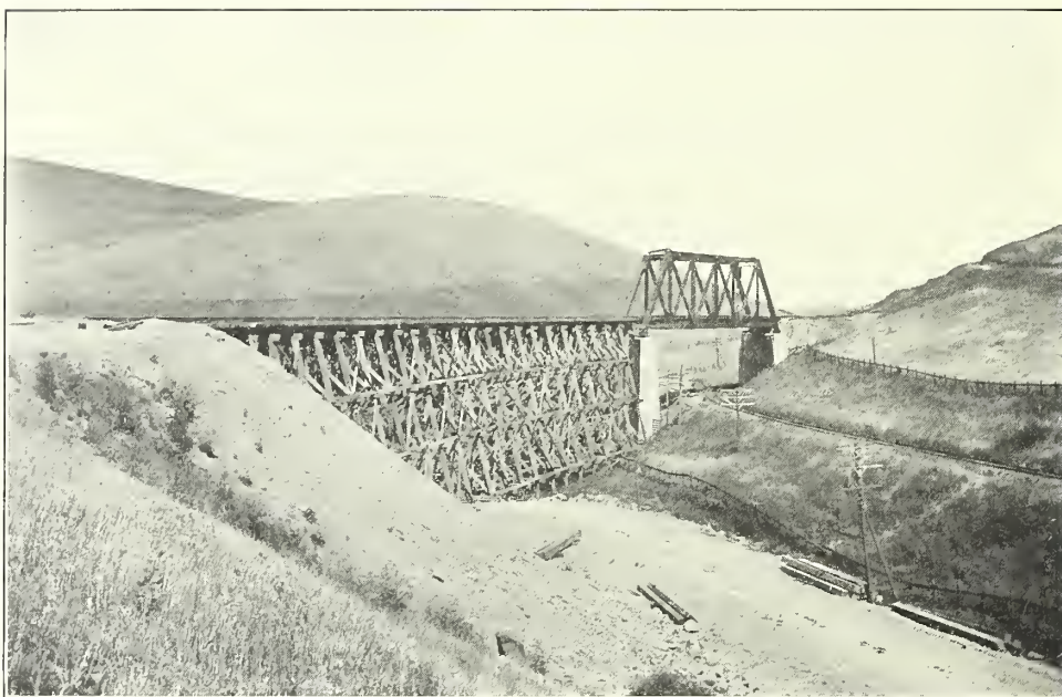
WESTERN PACIFIC CROSSING SOUTHERN PACIFIC BY STEEL AND CONCRETE BRIDGE
