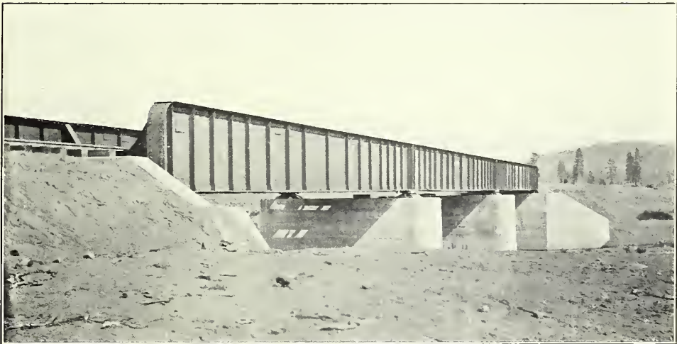
TYPE OF PLATE GIRDER BRIDGE
