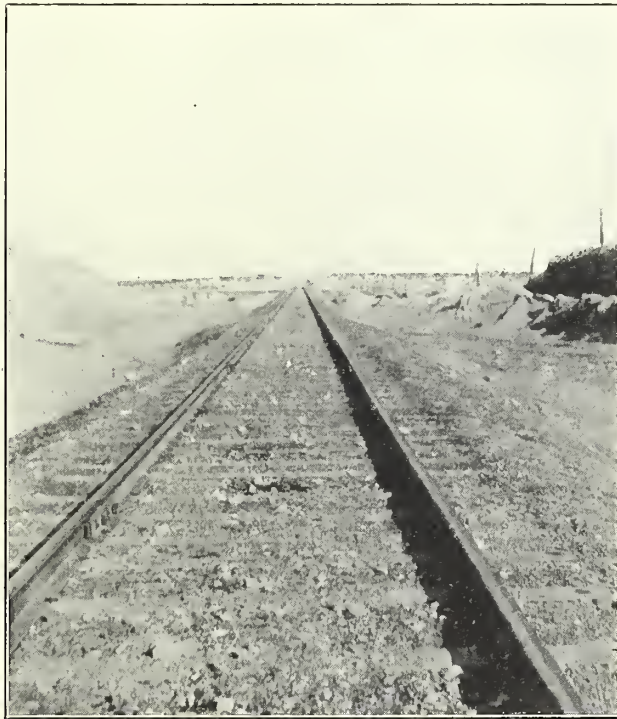
STRAIGHT LINE SHOWING HEAVY ROCK BALLAST
