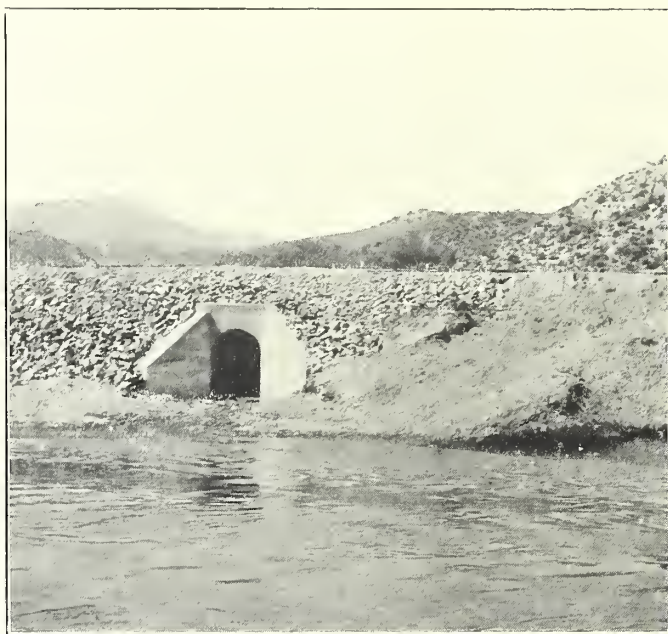
STANDARD CONCRETE CULVERT
