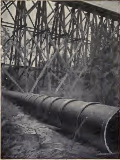
48 inch Lock Joint Pipe installed under 62 ft. Trestle. View before fill was placed.
