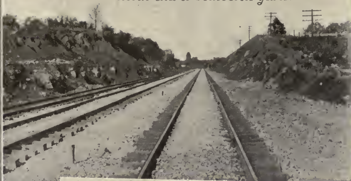
Dulaney Ky., showing south bound track completed and excavation being made for north bound track on lower level.
