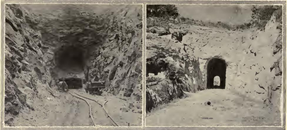
*Tunnel on the Dawson Cut-Off, Looking South—Note Method of Construction at Left*
