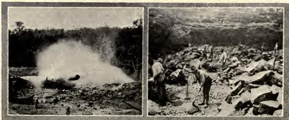
Left: Flushing Soil From Top of Asphalt by Hydraulic Pressure. Right: Open Quarry, Showing Face of Ledge and Asphalt in the Rough.
