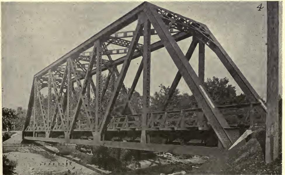
No. 4—This view shows a 150-foot span at Pond River, near Bakersport, Ky. This represents the most modern practice in the construction of truss spans. All of the members of this truss are stiff members, and all joints are riveted, making an extremely rigid span.
