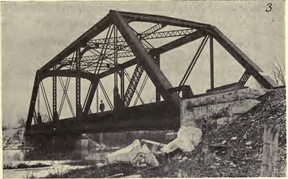
No. 3—The combination span, No. 2, was replaced in 1897, at the time this portion of the line was double-tracked, with the span shown above. This is a steel truss with pin-connected joints and is still in service.
