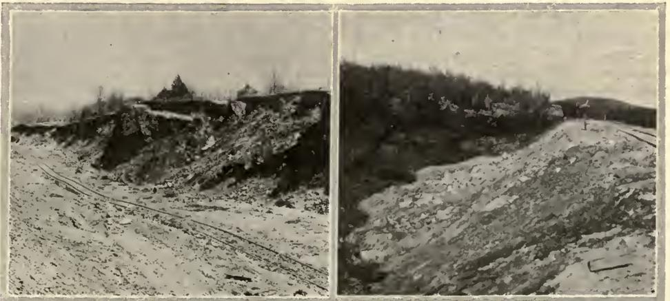
Slides—One in a Cut and One on a Fill—in Kentucky Division Grade Reduction
