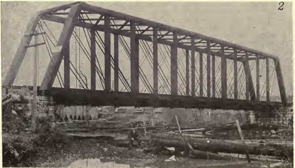
No. 2—The span shown in picture No. 1 was replaced in 1879 by the span pictured above. This was a combination span having timber for all stiff members and wrought-iron rods for tension members. The floor beams were of wrought iron and stringers of wood. A great many of these spans were built about that time, but they have now all been replaced. The last span of this type, at Hodgenville, Ky., was replaced in 1918.
