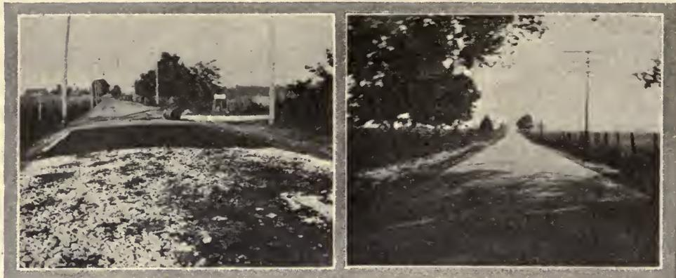
*Left: Warren County, Kentucky, Road in Course of Construction, Showing Three Stages of the Work—Limestone Base and Asphalt Surface Before and After Rolling. Right: The Completed Asphalt Road.*
