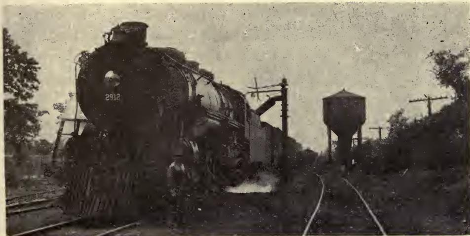
*Our Most Modern Equipment: Central Type Locomotive Taking Water at Bloomington, Ill., From 12-inch Telescopic Water Column, Connected With 100,000-Gallon Conical Bottom Steel Water Tank at the Right.*
