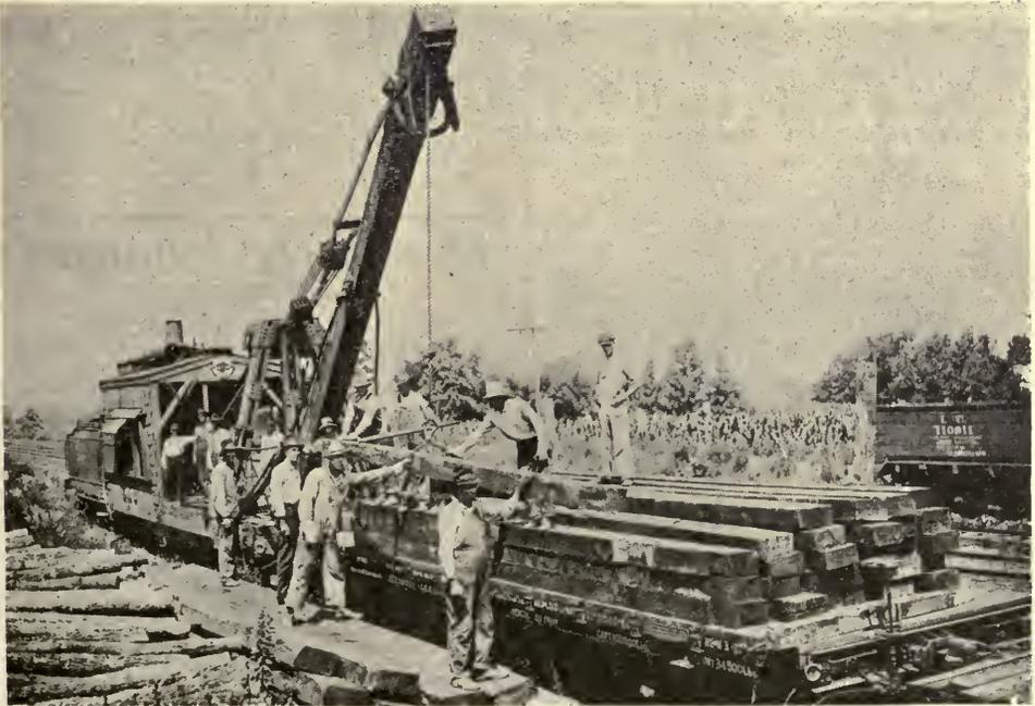
Pile driving gang, with Pile Driver X-2, in charge of Foreman George Smith, on the St. Louis division. There were 180 piles driven in Big Muddy Bridge in seven days; 42 piles driven at Big Bay in 1½ days, and 72 piles driven at Gale in 3 days—or a total of 310 piles driven in 11½ days, an average of approximately 26 piles a day.
