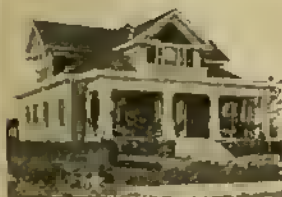
A No. 1-22-W IDEAL Boiler and 422 ft. of 38-in. AMERICAN Radiators, costing the owner $195, were used to Hot-Water heat this cottage.
