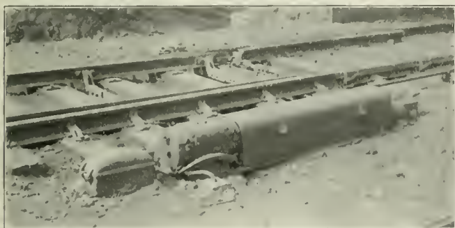
Fig. 4—Union Switch &amp; Signal Company's Electric Switch Movement.
