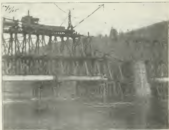
Morning of Dec. 6th (not Dec. 5th). Derrick car placing rangers on top of intermediate tier. Five horses to meet.
