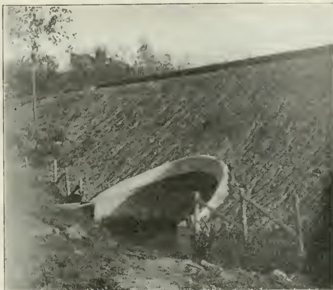
Fig. 2—Diagonal View of Horse-Shoe Arch.
