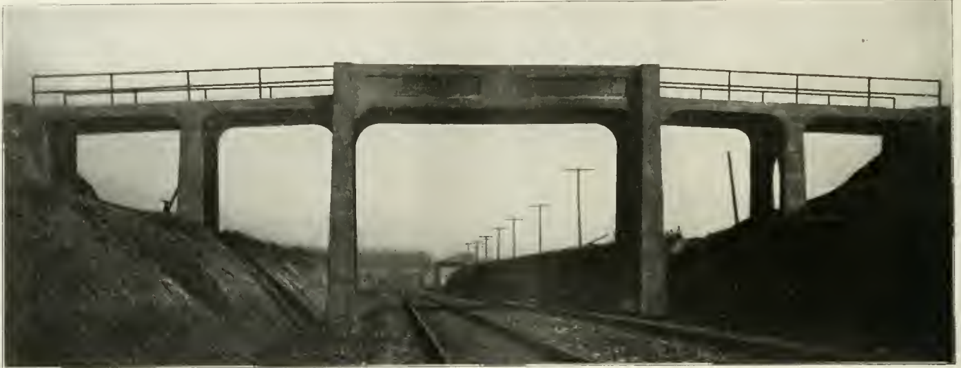
Reinforced Concrete Highway Bridge Over Tracks of the Big Four near Binney, Ill.
