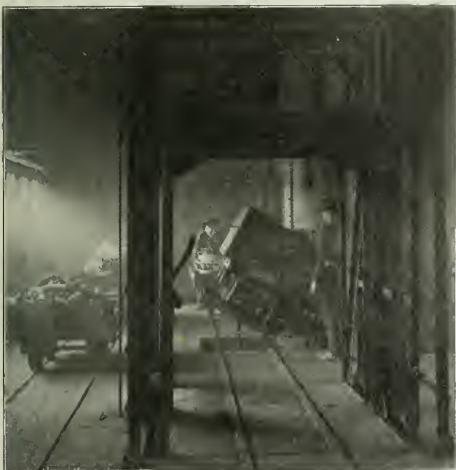
Automatic Dump Car Charging Cupola.
