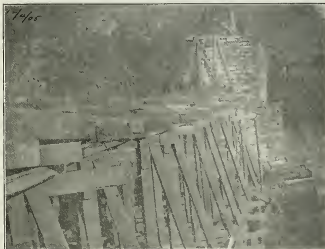
Dec. 4th. East span looking east. First ten tiers of horses are in place; the top tier lying flat, to be ended up by patent pile driver. This tier of fourteen horses was put together and ended up in thirteen hours.
