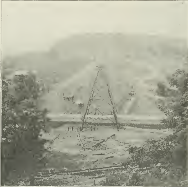
Fill at Collier's Run. 60 ft. Deep; Showing 10-ft. Arch Culvert in Course of Construction.
