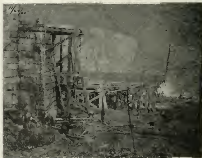
Nov. 24th. Temporary trestle in the west span fairly started, showing method of erecting in stepped tiers. The horses were framed flat and ended up with block and fall from hoisting engine on top of abutment.
