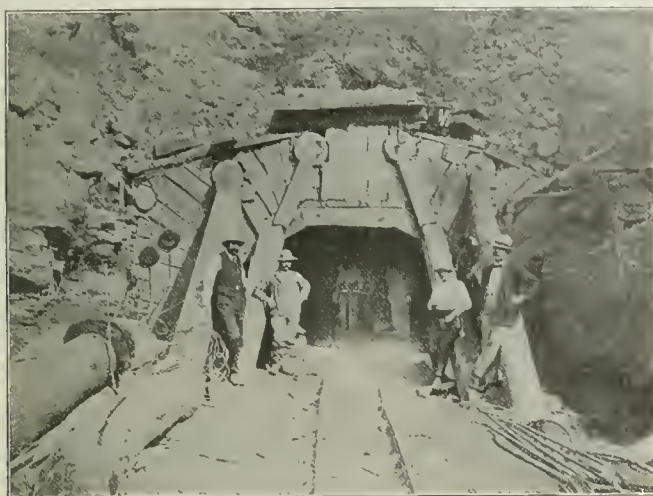
West Heading of Knobley Tunnel Showing Timber Bracing.
