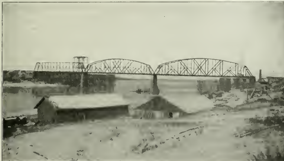
First and Second Spans Erected and Falsework Under Old Third Span.
