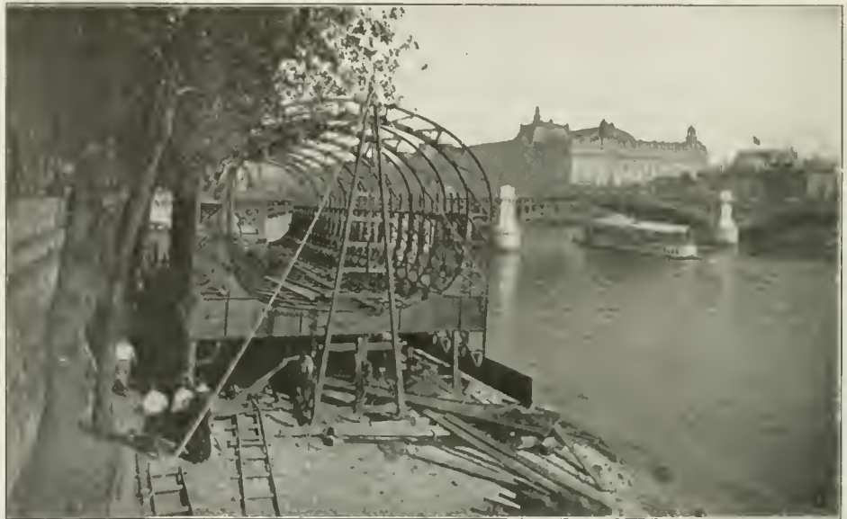
Fig. 1—The First Caisson on the Mounting Stage.
