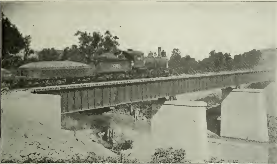
Licking-Creek Bridge; Three 80-ft. Plate Girder Spans on Concrete Piers and Abutments.
