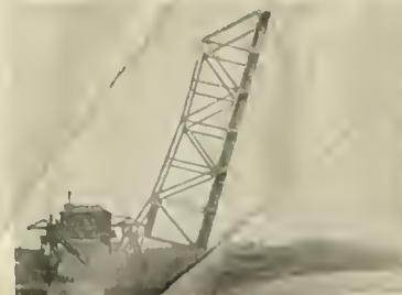
Single-Track Railroad Scherzer Rolling Lift Bridge, across Cuyahoga River, Cleveland, O., for C. C. & St. L. Ry., in partly open position.
