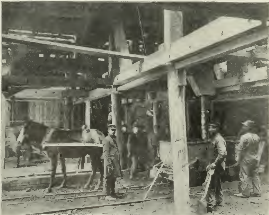
Timbering and Spoil Trucks Beneath Fulton Street.
