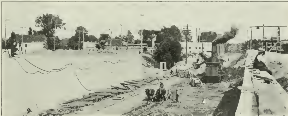
Track Depression in Detroit Street and Nickel Plate Grade Separation.
