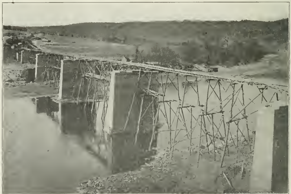
Fifth Crossing of the Potomac River Showing Temporary Trestles Used for Depositing Concrete for Bridge Piers.
