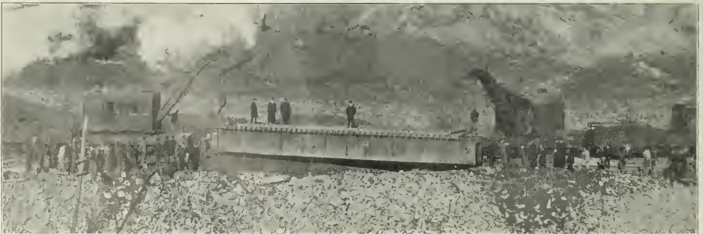
Fig. 11—Lifting Bridge 68 from Old Location.
