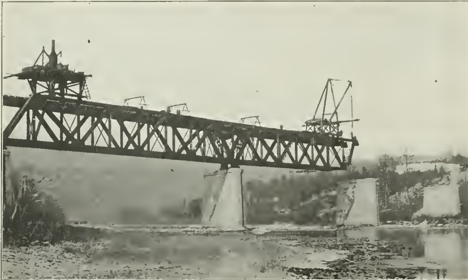
Second Crossing of the Potomac River Showing Cantilever Erection of 150-ft. Spans.
