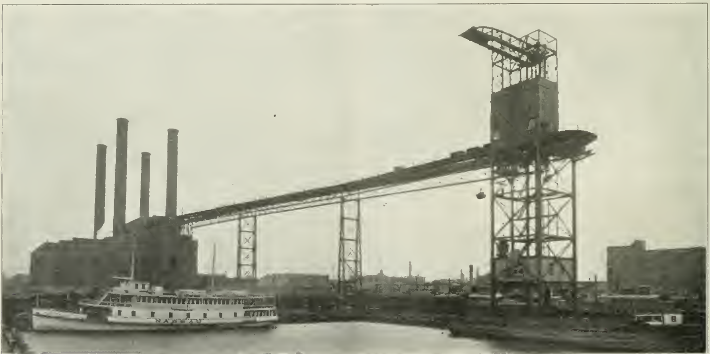
General View of Long Island City Power Station from River, Showing Coal Tower in Operation—Pennsylvania Railroad.
