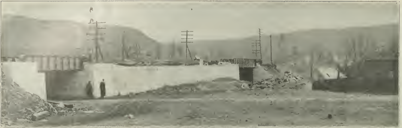
Fig. 8—(Left to Right) Bridge 66, Bridge 67 and No. 6 Arch. Wall Necessary as Additional Right of Way Could Not be Secured.
