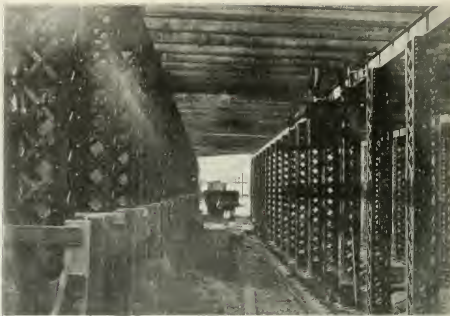
Showing Steel Columns in Piers and Forms in Place for Concreting Curtain Walls —Detroit Street and Nickel Plate Grade Separation.
