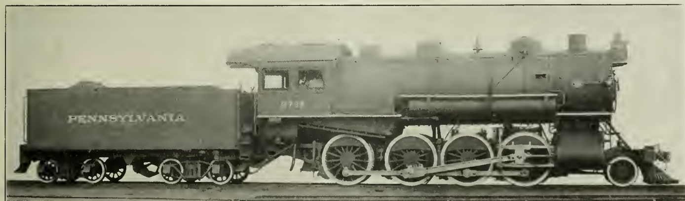
Consolidation Locomotive with Walschaert Valve Gear. Built by The American Locomotive Co.
