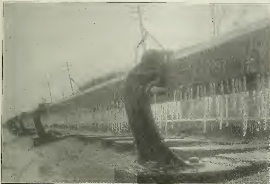
Sleet formation on Under-Running Third Rail; Three-Piece Protection.
