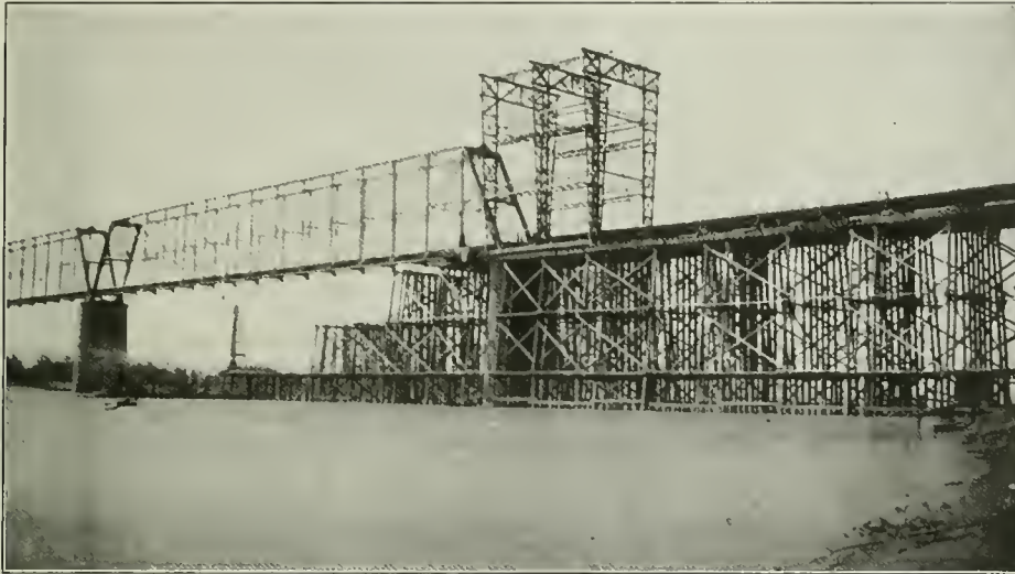
Falsework and Traveler Used in Rebuilding the Bismarck Bridge.
