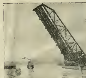
Double-Track Scherzer Rolling Lift Bridge, over Cuyahoga River, Cleveland, O., for N. & S. S. Ry., in partly open position.
