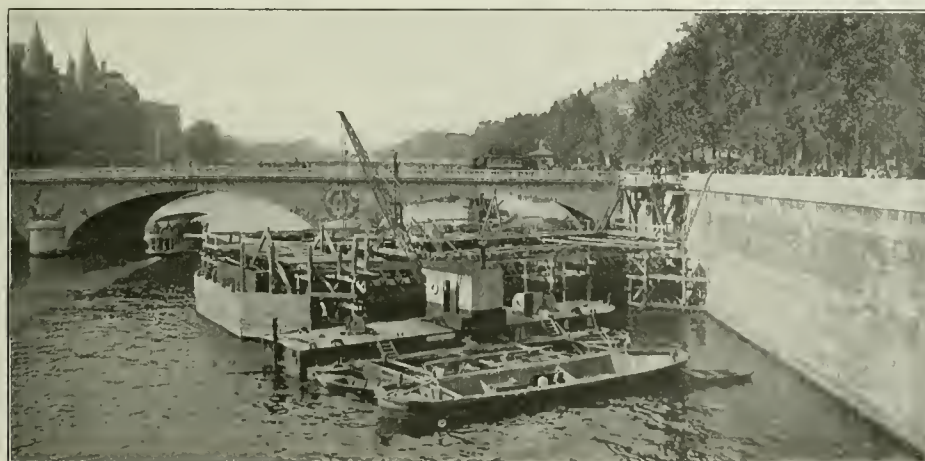
Fig. 4—The Caisson Ready to be Sunk.
