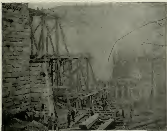
Nov. 26th. Temporary trestle two days later. Men working on runway on which girders for iceway were carried into place.
