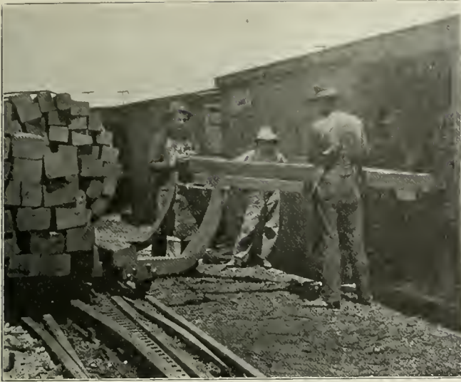
Loading Treated Ties into Box Car.
