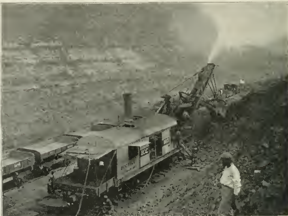
From stereograph by C. L. Chester; Copyright, 1906, by Underwood & Underwood, New York. West Bank of Culebra Cut, Looking South—Bucyrus Steam Shovel at Work.
