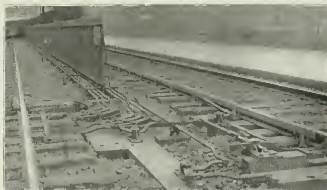
Fig. 7 Signal Rod (Pipe) Line and Fence, Showing Deflector Bars.
