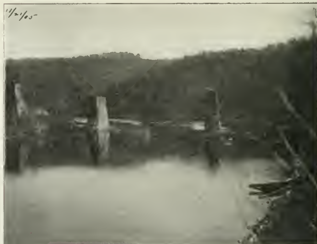
View from up-stream. West pier still smoking. Wreckage around west pier and between east pier and east abutment.
