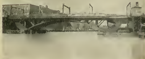
Highway and Electric Railway Scherzer Rolling Lift Bridge across Chicago River at North Halsted Street, Chicago, in the closed position.
