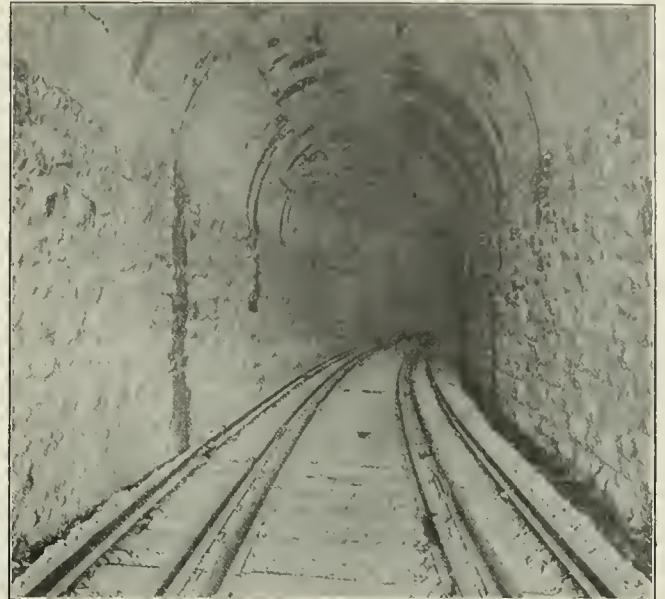
In From North Portal—Masonry and Concrete Section.
