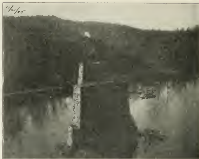
Looking west from east abutment. Wreck of old bridge lying in river on the right. This wreckage lay in the line of the bridge and had to be pulled out of the way before the new bridge could be started.
