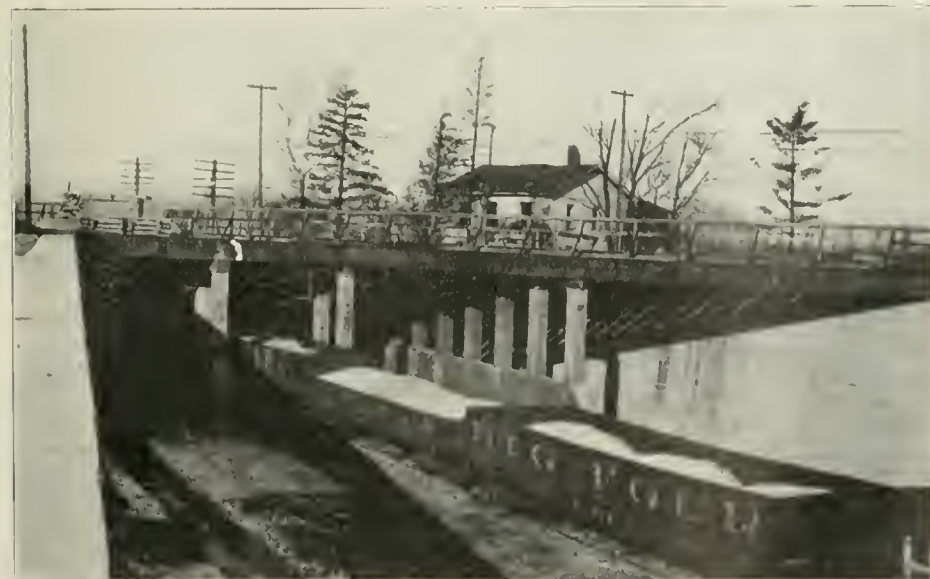
Concrete Curtain Walls Completed and Columns Encased in Concrete—Temporary Floor and Railing for Use During Winter—Detroit Street and Nickel Plate Grade Separation.
