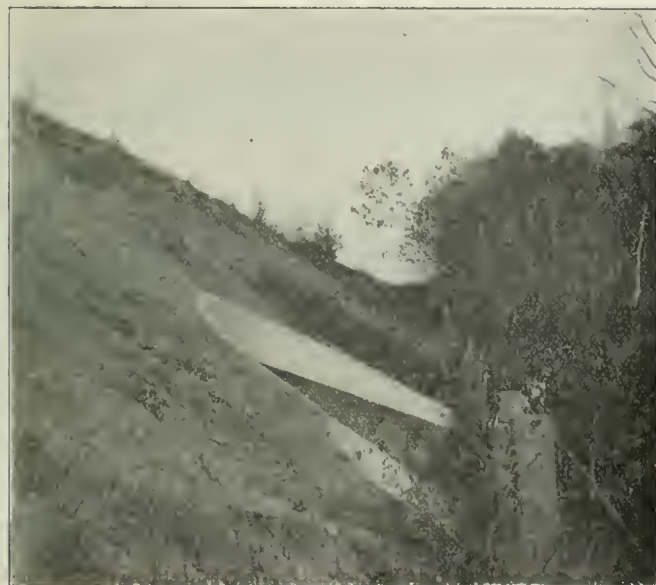
Fig. 3—Side View of Horse-Shoe Arch, Showing Fit of Shoulder to Side Slope.
