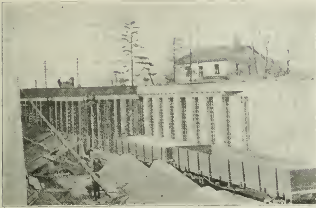
Steel Erected and Concreting of Curtain Walls in Progress —Detroit Street and Nickel Plate Grade Separation.
