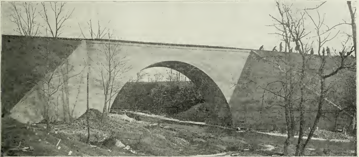
New 55-ft. Double Track Reinforced Concrete Arch Over Stony Creek—Chicago & Eastern Illinois
