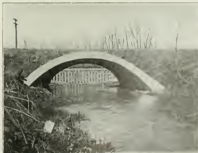
Fig. 6—Funnel-Shaped Horse-Shoe Arch.
