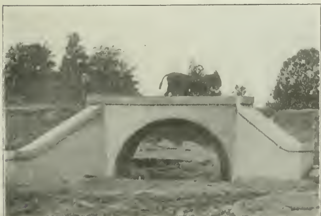
Fig. 5—Concrete Arch With Wings and Spandrel.
