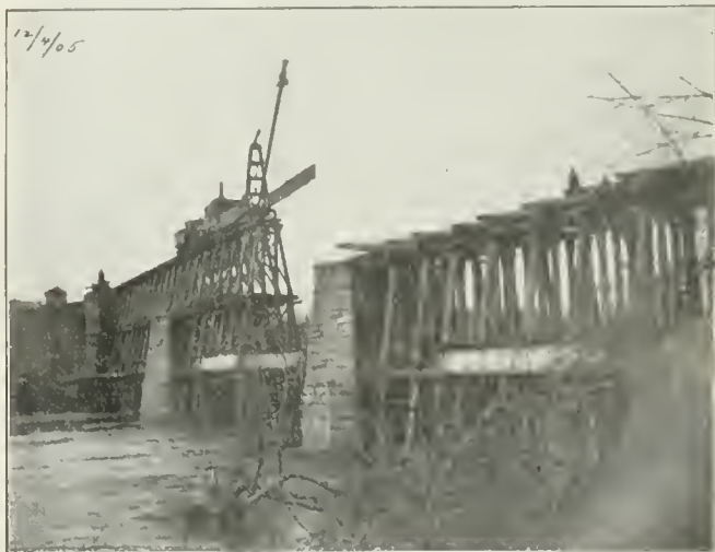
Afternoon of Dec. 4th. Placing last girder in east trestle of center span. Ready to end up top tier of east span.
