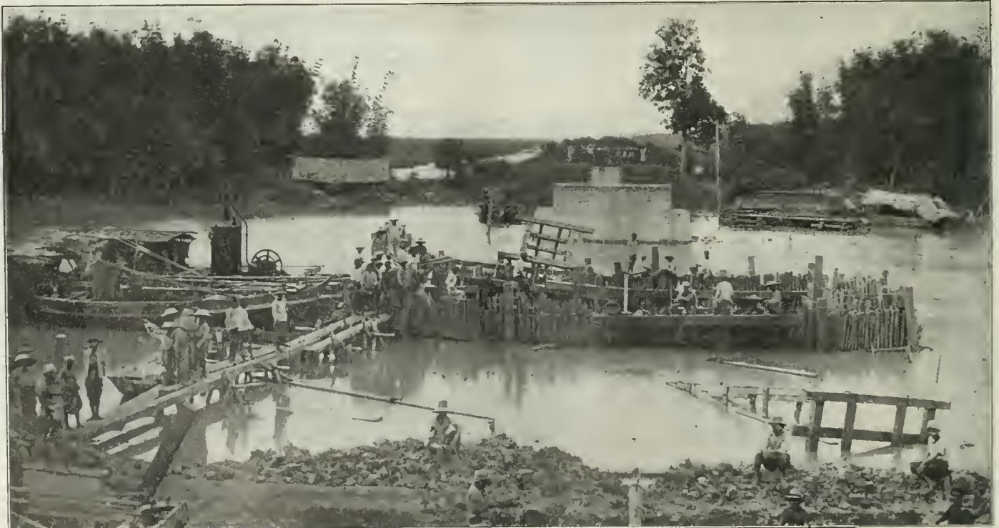
Building the Abutments and Piers of the Ban Po Bridge.
