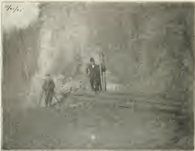
Nov. 21st. At foot of east abutment. Debris on left is rock scaled off abutment by heat of the fire.
