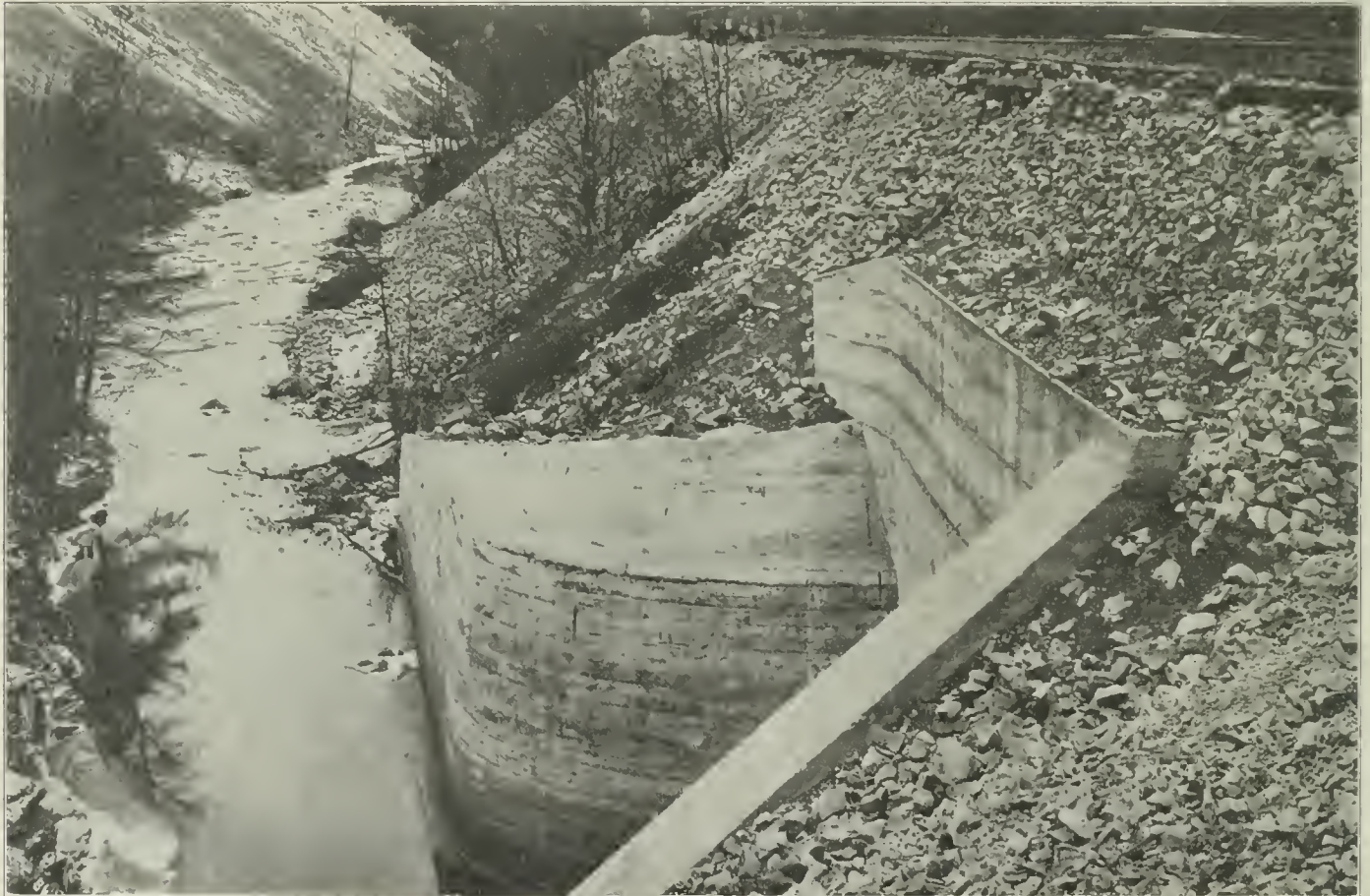
Fig. 2—Concrete Arch West of Tunnel Yet to be Extended for Two Tracks. Narrow Gage Track for Small Cars Carrying Material from Tunnel Shown on Edge of Bank.
