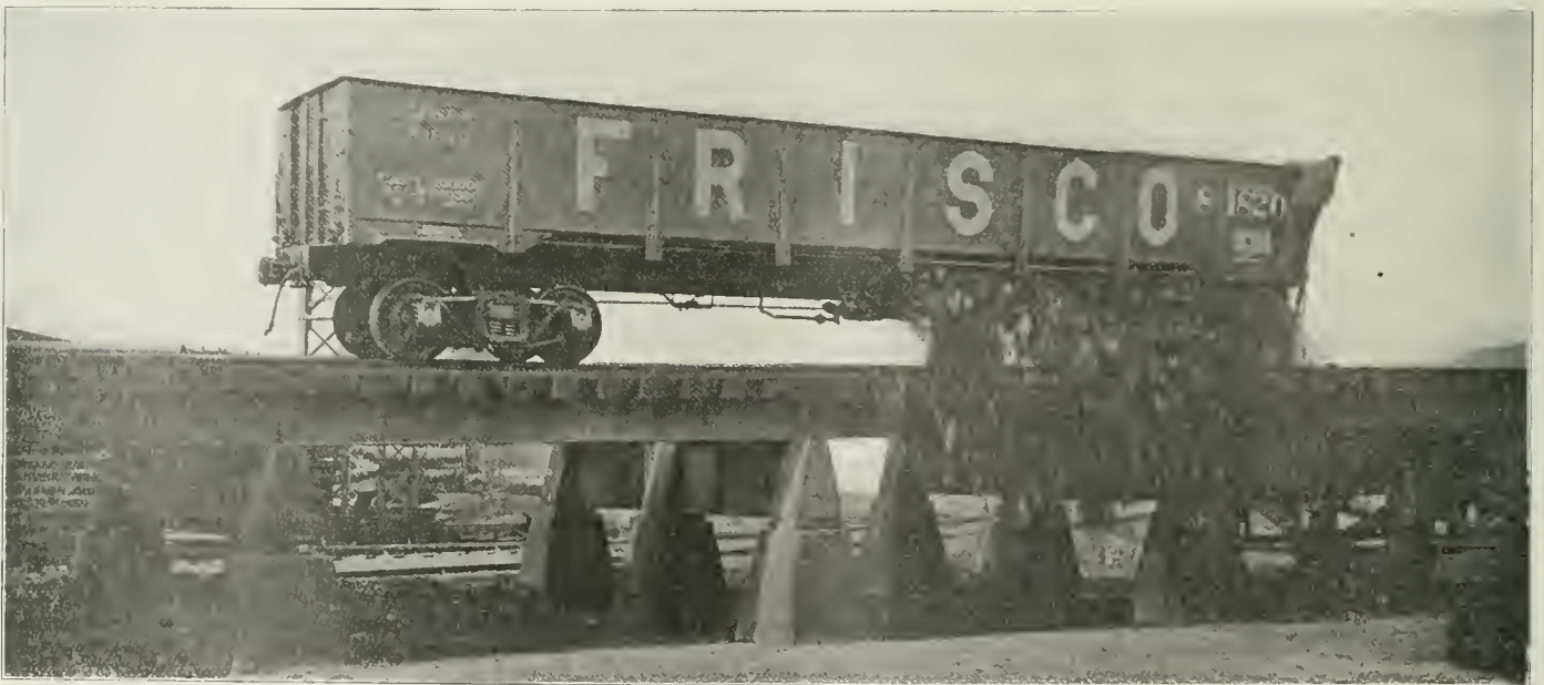
General Service Drop Bottom Gondola Car Discharging Load Through Four Doors.
