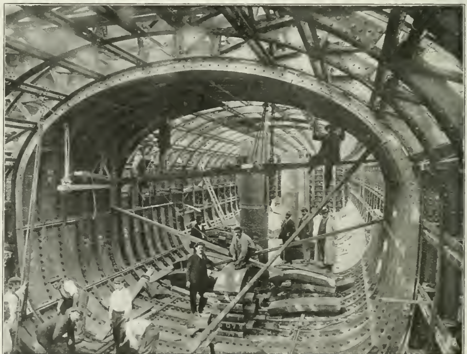
Fig. 2—Putting in Place the Cast-Iron Lining of the Caisson.
