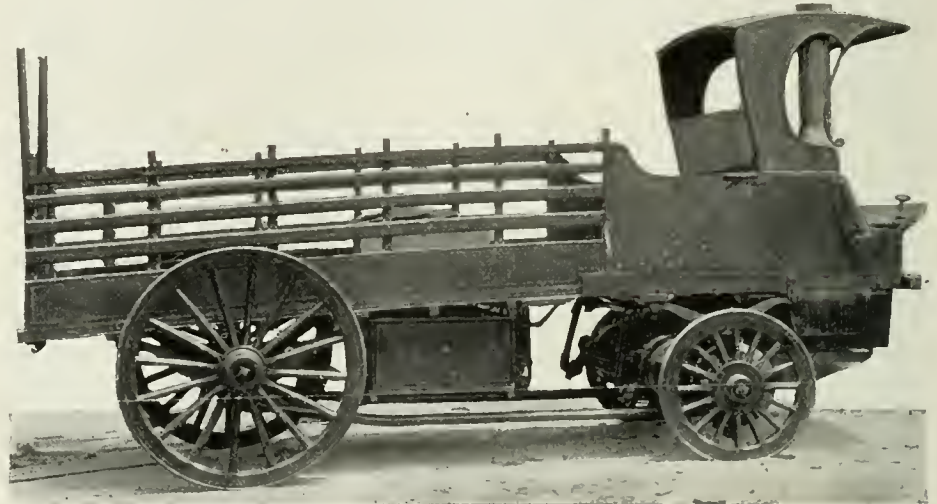
8-Ton Steam Motor Truck with Halsey Motors.
