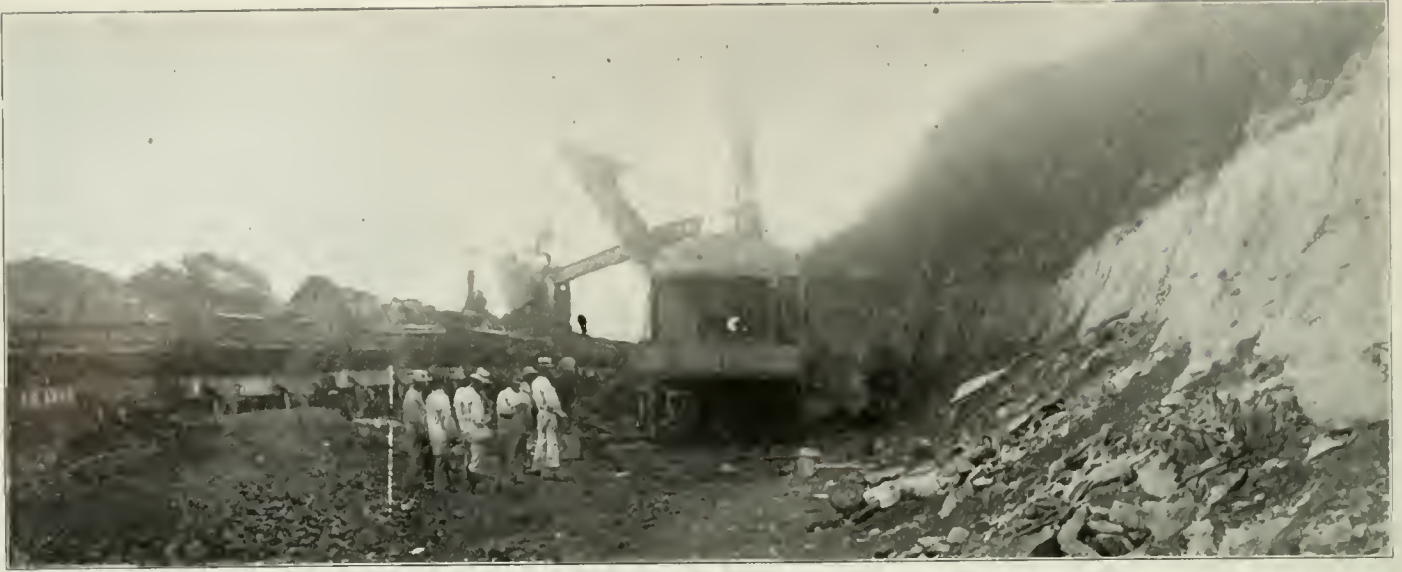
From stereograph by C. L. Chester; Copyright, 1906, by Underwood & Underwood, New York Bucyrus Steam Shovel ( 3\frac{1}{2} Yards Dip) in Operation—Soft Clay Rock in Foreground—Similar Rock Was Blasted by the French Canal Company.
