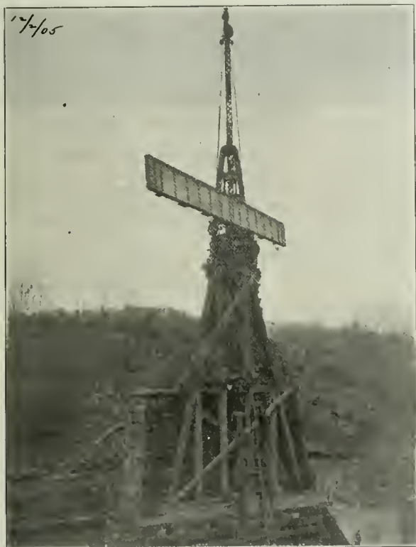
Dec. 2d. Looking west. Derrick car placing an 8-ton girder in center iceway.
