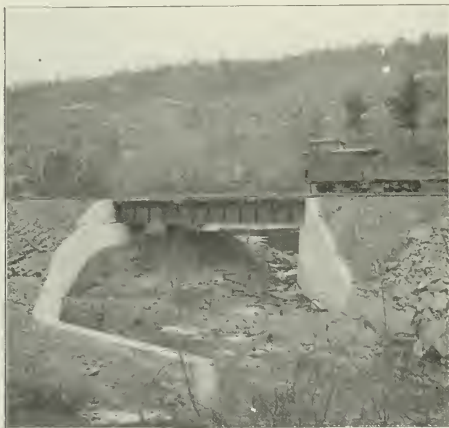
Fig. 12—Bridge 68, New Location; New Masonry Includes Wing Wall to Protect Water Company's Pipes.
