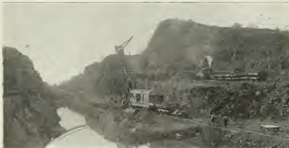
From stereograph by C. L. Chester; Copyright, 1906, by Underwood & Underwood, New York. French Cut for Lock at Bas Obispo—Steam Shovel and Dirt Train at Work.
