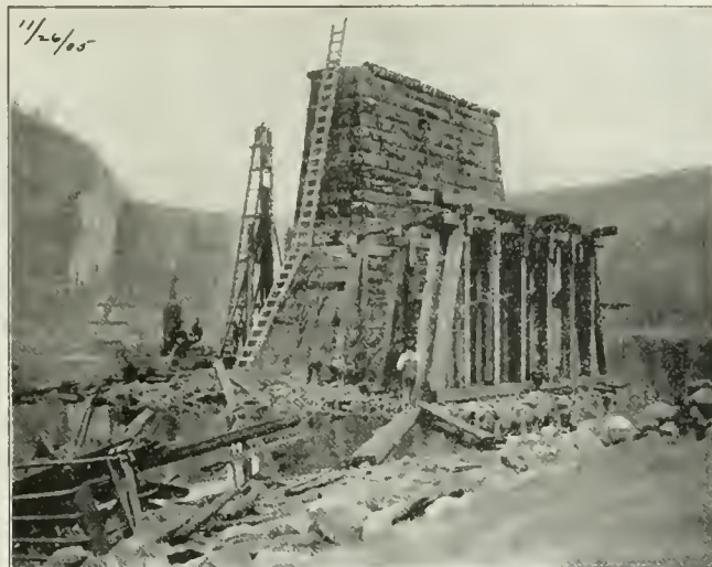
Construction at west pier showing frame bents erected on rip-rap on the west side and pile-driver at work on piles for center span bent. The bottom was rock ledge on the west side of the pier so that piles could not be driven there. Wreckage in foreground at the left.
