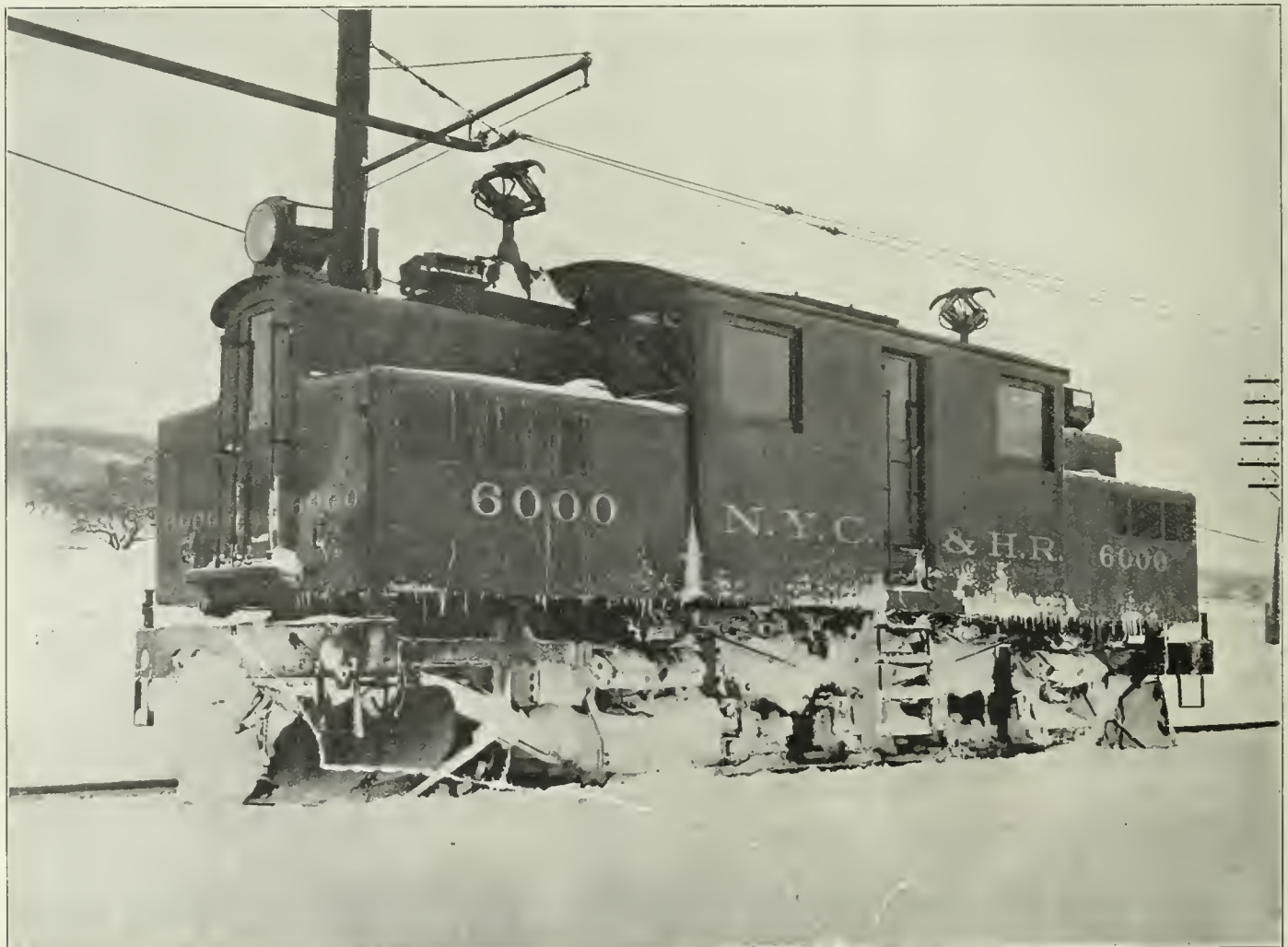
Elevation of Locomotive, Showing Flangers.
