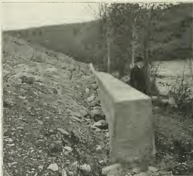
Fig. 13—Retaining Wall to Protect Water Supply Reservoir.
