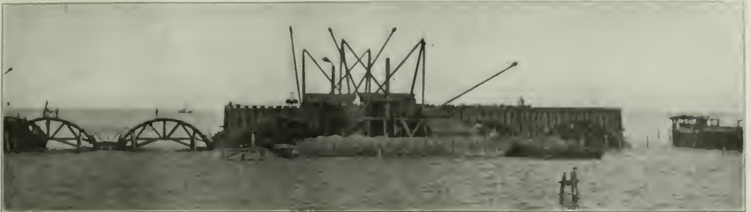
Long Key Viaduct under Construction; 184 Concrete Arches.
