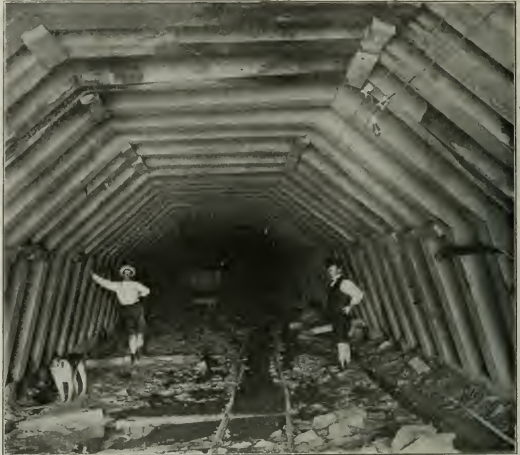
Method of Timber Framing Heading in Burton Tunnel.
