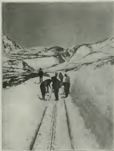
Clearing Snow on Rack Section of Argentine Trans-Andine.
