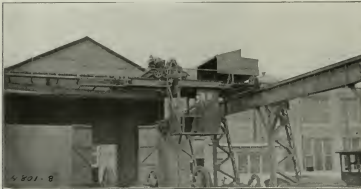
10-Ton Crane and Runway over Tire Storage Yard.
