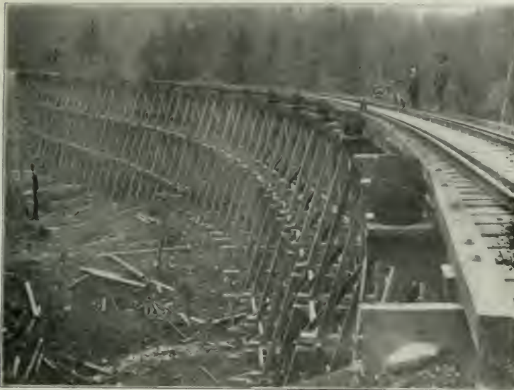
Three-Story Wooden Trestle; Deepwater Railway.
