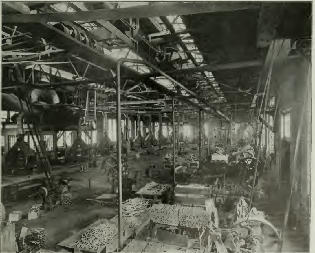
Union Pacific Blacksmith Shop at Omaha. Material cars serving machines, in foreground.
