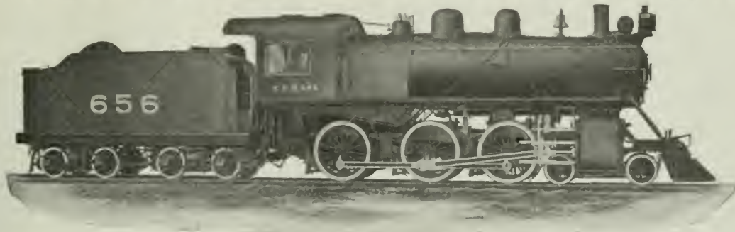
Ten-Wheel Locomotive with Superheater; Canadian Pacific Railway.
