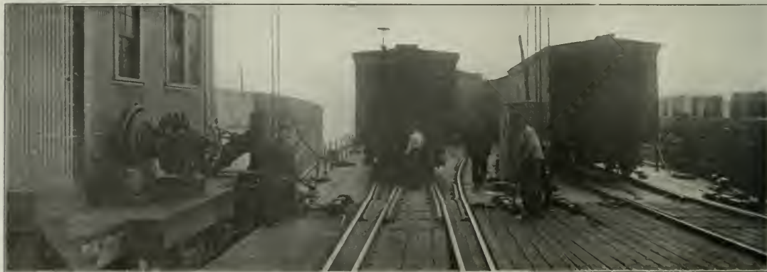
Transfer Bridge at Greenville Yard, Showing Lidgerwood Slip-Drum Hauling-In Winch.
