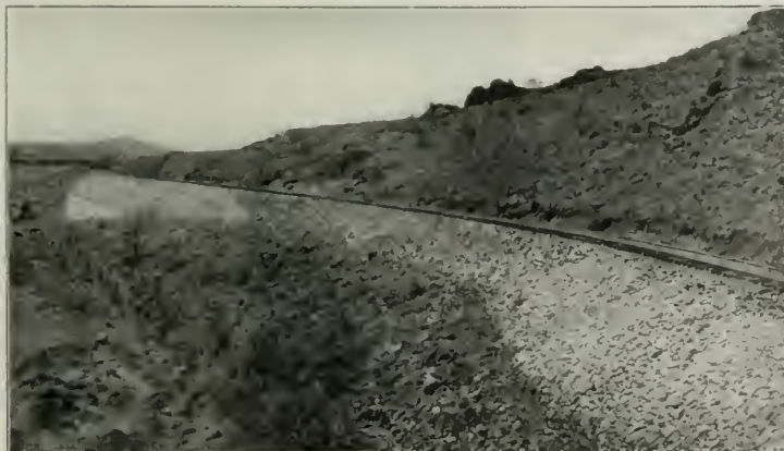
Mountain Construction, Showing Riprap Work.
