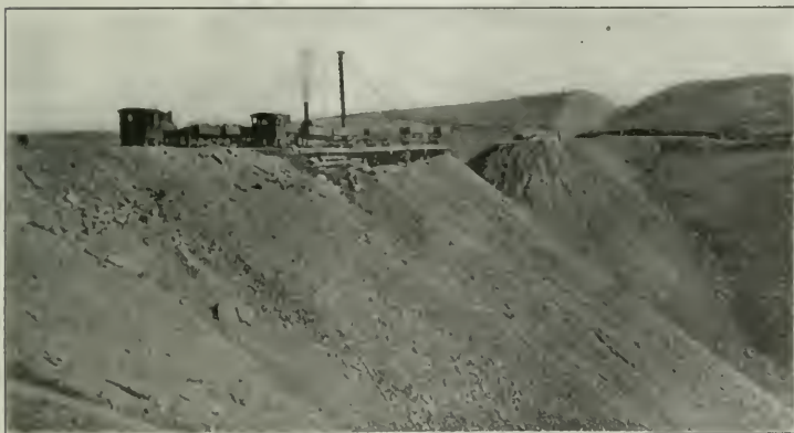
Unloader Used on High Fills; by E. B. & A. L. Stone Co.; Western Pacific.
