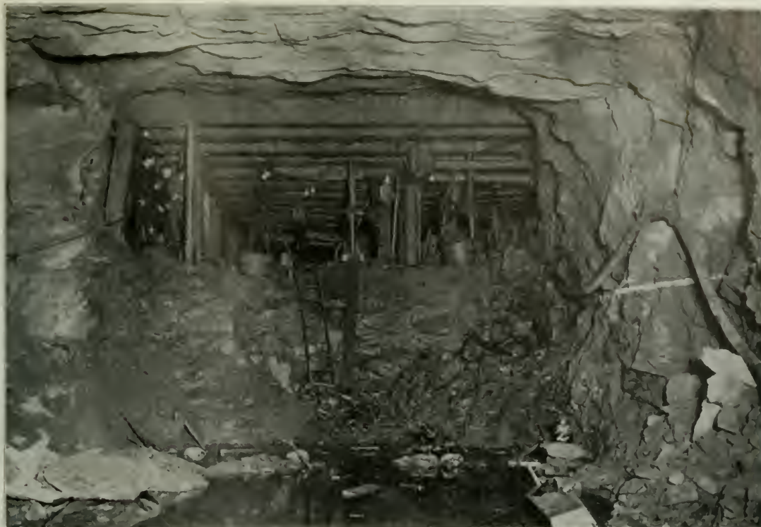
Fig. 2—Heading of Double Track Tunnel in Solid Rock.
