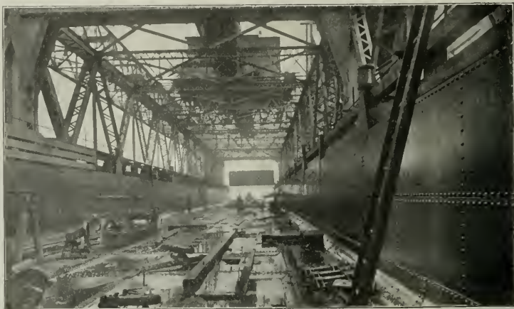
View in the Trough During Construction of Ship Lift.
