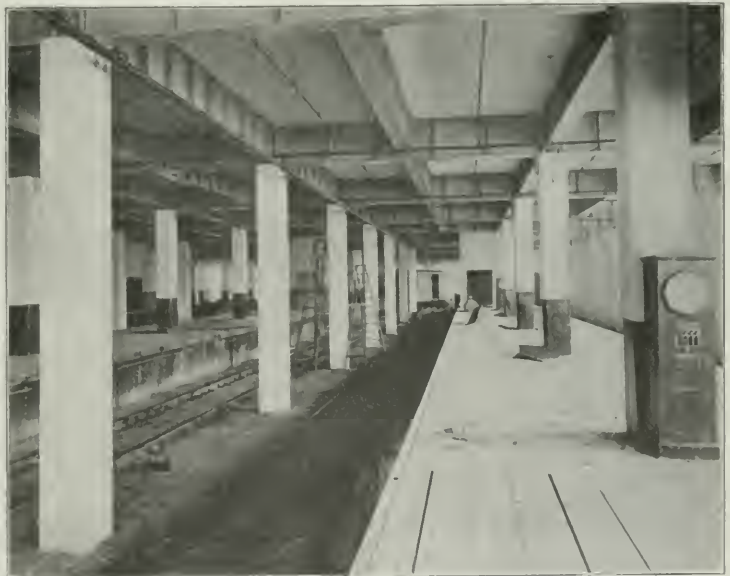
Track Floor of Warehouse. Showing Tracks and Platforms.
