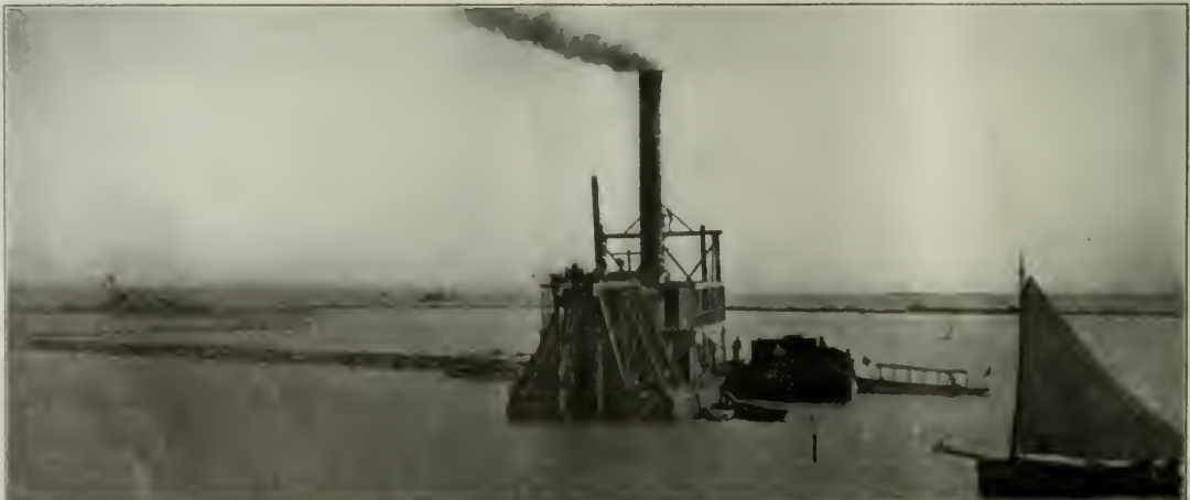
Hydraulic Dredge Throwing Up Embankment in Shallow Water.
