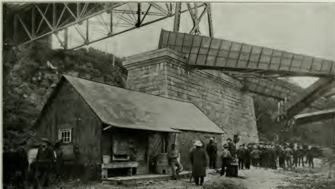
Anchor Pier, Showing Anchor Arm Supports Still Fast to the Masonry.
