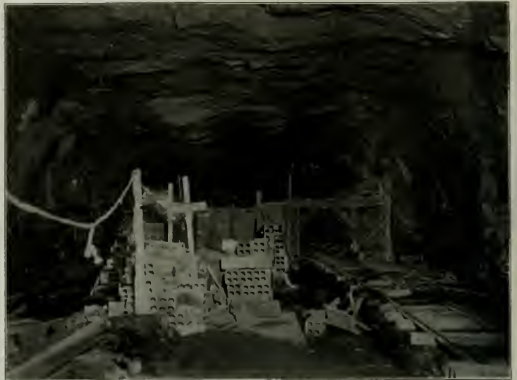
Fig. 4—Placing Forms for Concrete Side Walls.
