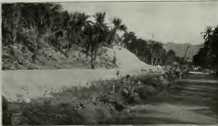
A Side Hill Cut and Fill; Philippine Railways.
