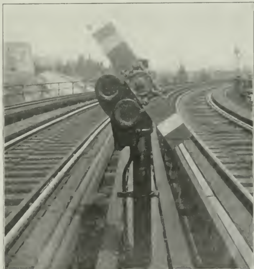
Fig. 4—Centrally Pivoted Semaphore Signal for Express Track at 110th Street.
