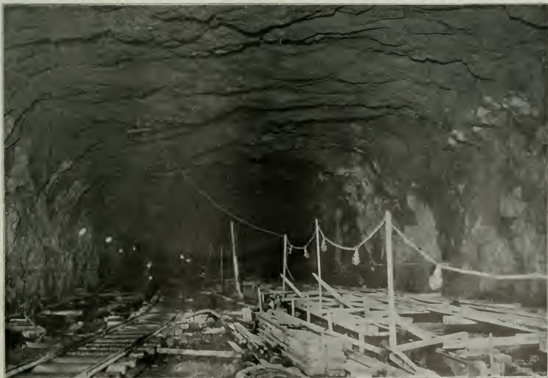
Fig. 3—Completed Excavation for Two-Track Tunnel in Solid Rock.
