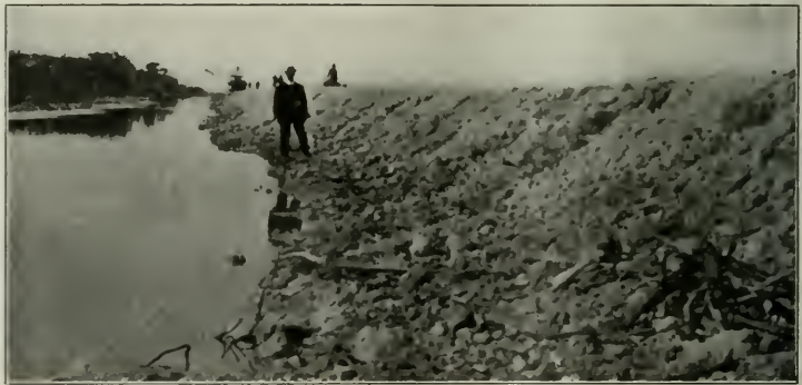
Embankment Thrown Up by Dredging.
