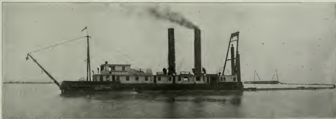
Hydraulic Dredge Francis T. Simmons, Built by Atlantic Equipment Company for Lincoln Park Commissioners, Chicago.
