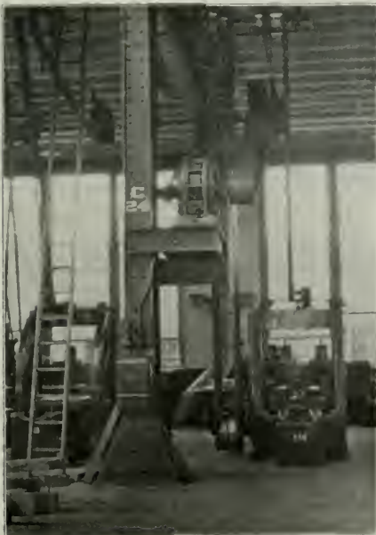
Motor Bracket on Intermediate Column.
