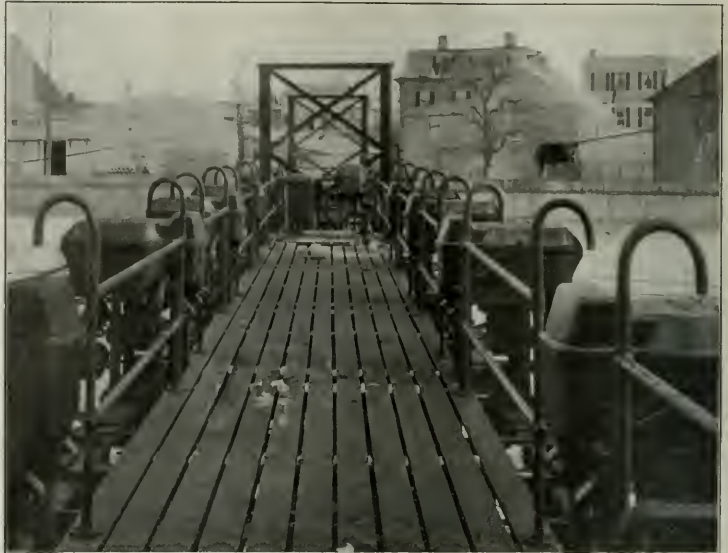
Deck of Anchor Bridge, Showing Circuit Breakers and Other Auxiliary Apparatus.
