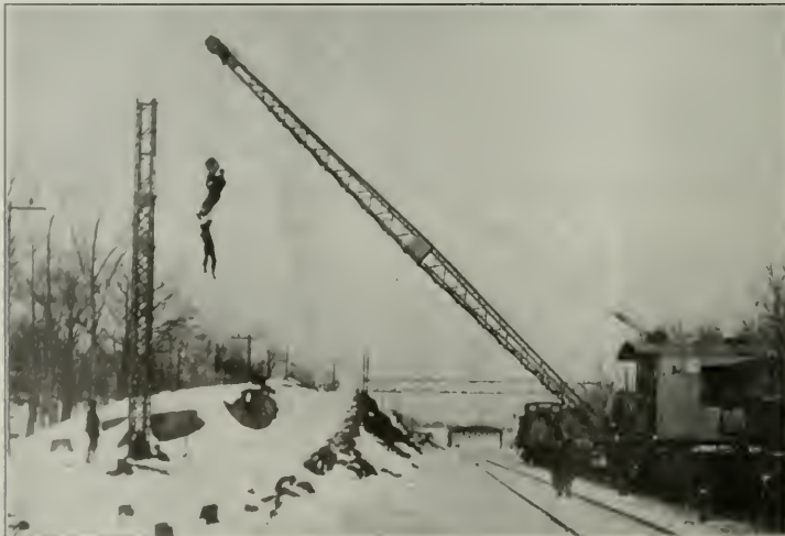
Method of Erecting Bridge Columns with Locomotive Crane.
