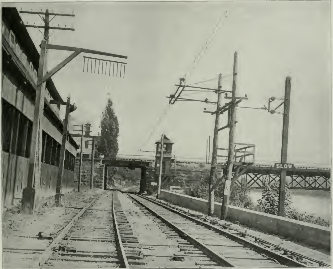
Overhead Catenary Construction at Clarissa Street Bridge, Rochester, Showing Section Break and Bridge Warning.
