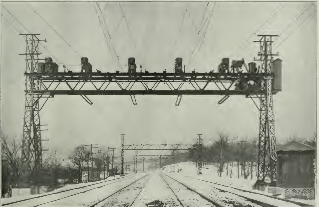
Four-Track Anchor Bridge with Circuit Breakers and Section Breaks.
