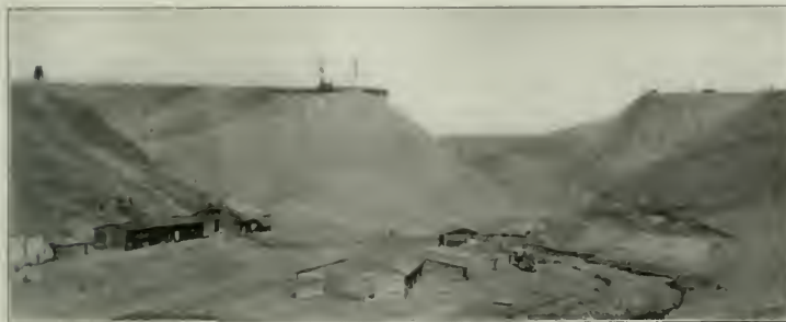
High Fill on Line of Western Pacific; Unloader at Work.
