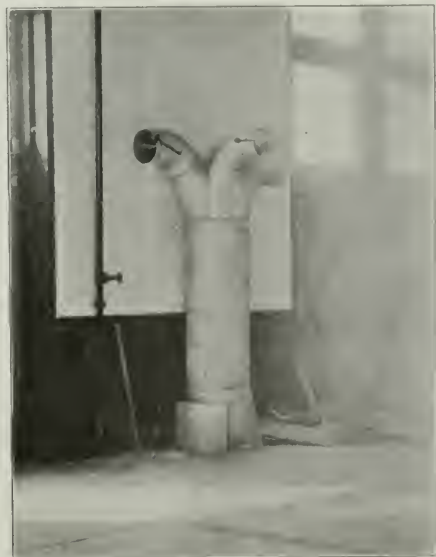
Riser from Heating Duct.
