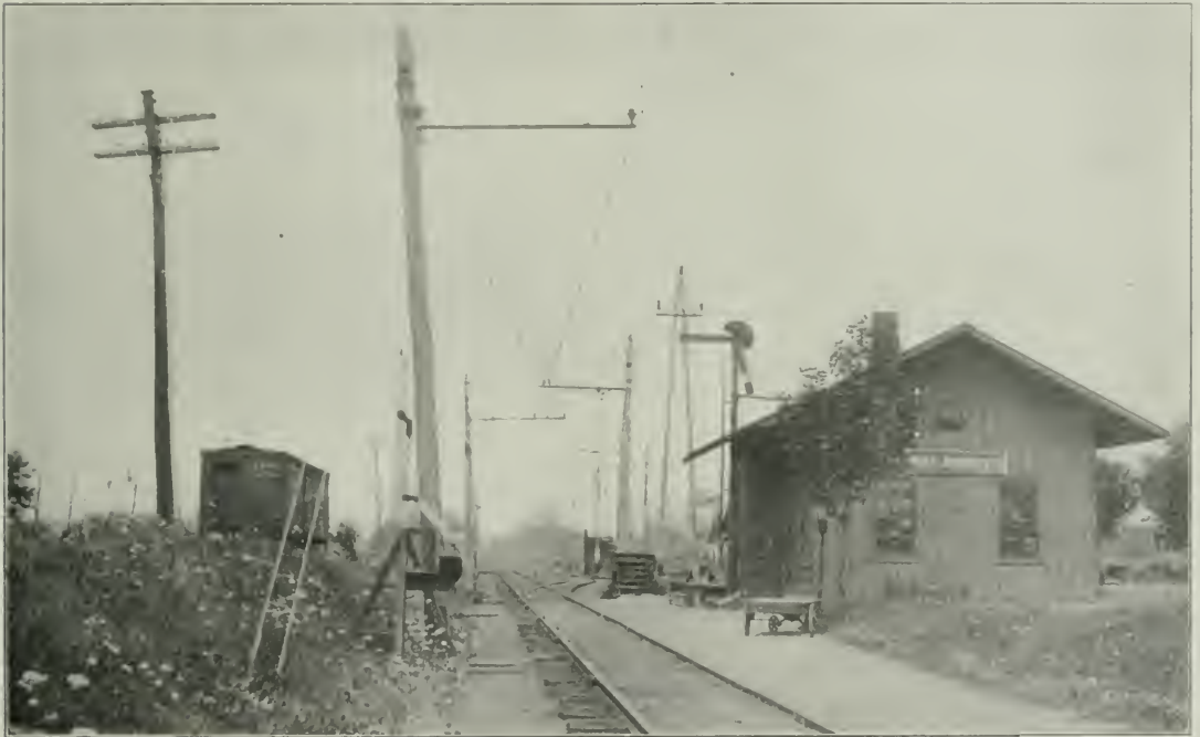
Overland Bracket Construction for Main Line and Siding at West Henrietta.
