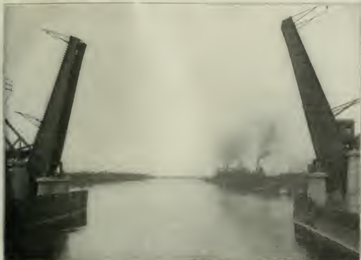
Rail Bascule Bridge in Open Position.
