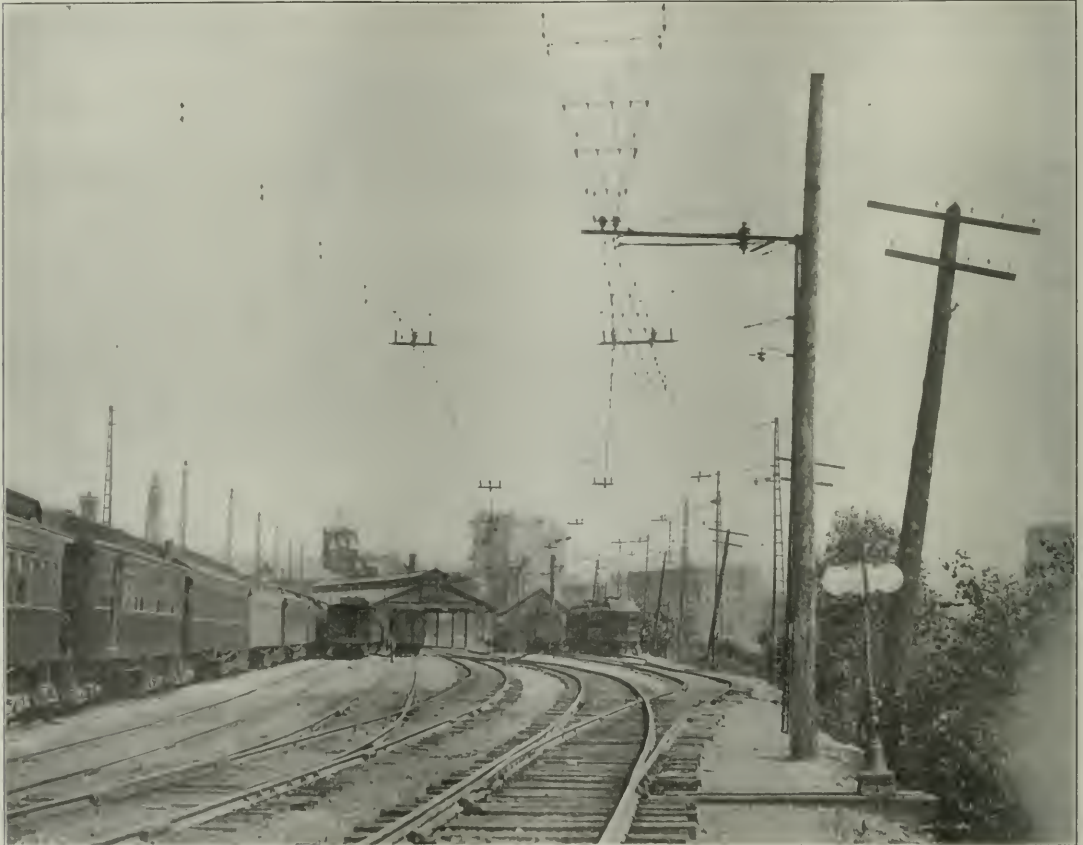
Rochester Terminal Yard, Four Tracks Electrified, Showing Overhead Span Construction.
