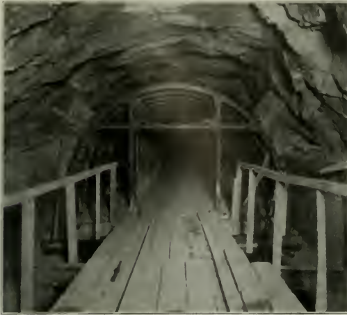
Fig. 6—Steel Forms for Tunnel Arch.
