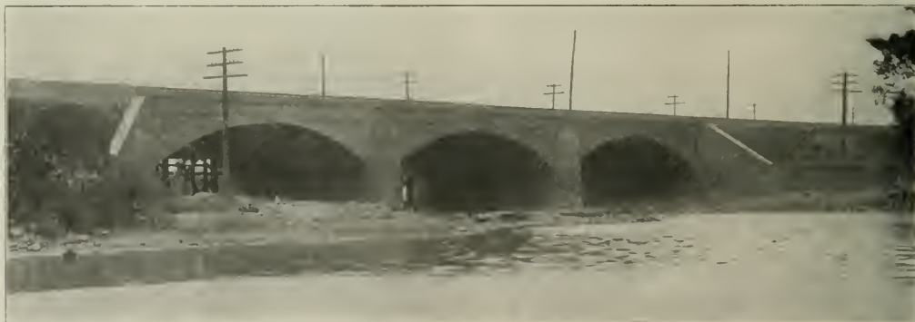
Fig. 10—Concrete Arch Over Eagle Creek; Vandalia Track Elevation.
