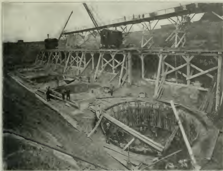
Shafts for Ship Lift While Being Built.
