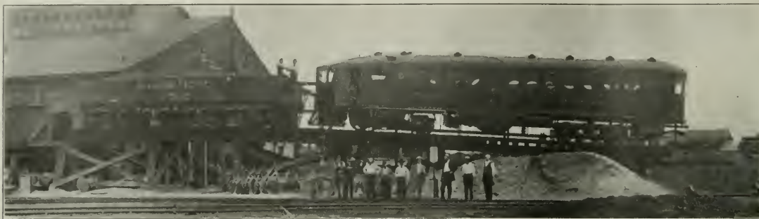
Motor Car No. 10 Pushing a Loaded 40-Ton Coal Car Up a 7.6 Per Cent. Incline.
