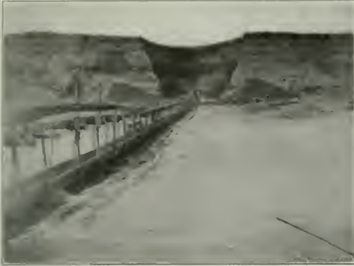
Hydraulic Excavation of a Deep Cut near St. John's.
