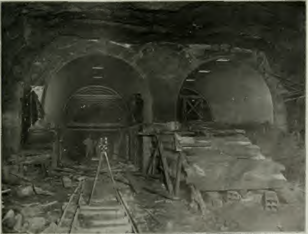
Fig. 7—Completed Section of Standard Twin Tunnels.
