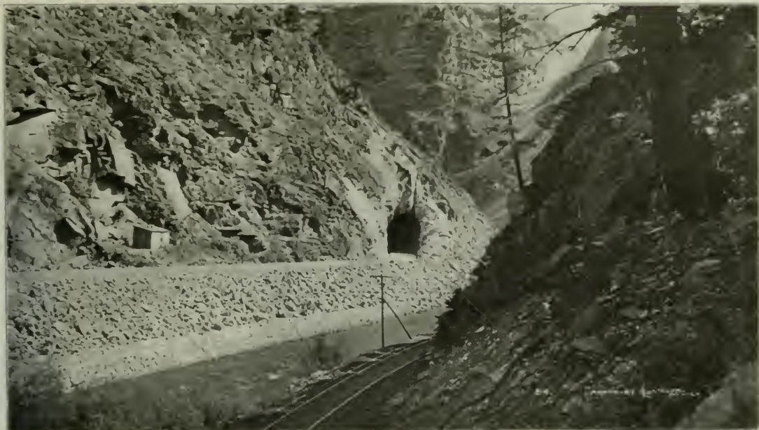
Belden from the East; Retaining Wall and Tunnel on New Second Track.
