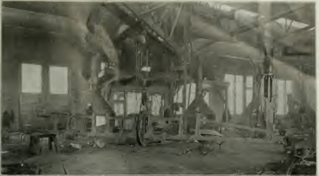
Frame Fire and Foreman's Office. Team track at left is for moving heavy repaired forgings.
