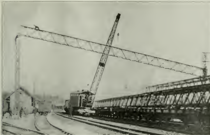
Erecting a Long Trolley Bridge Truss in the Yards.
