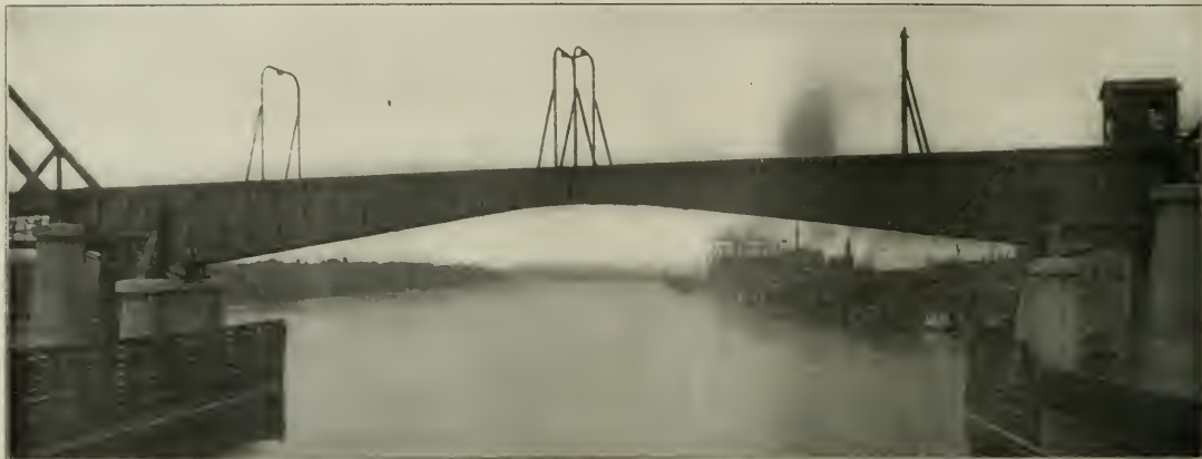
Rall Bascule Span in the Illinois River Bridge at Peoria for the McKinley Interurban Syndicate.
