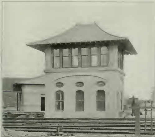
Concrete Interlocking Tower at Naugatuck Junction.
