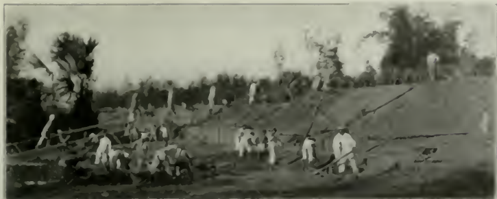
Grading a Fill from Borrow Pits.
