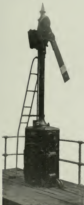
Fig. 3—High Semaphore Solenoid Signal for Manhattan Elevated.
