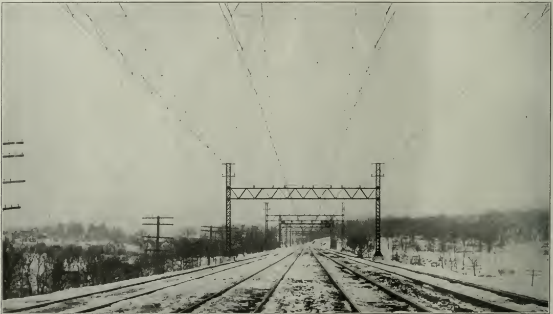
Overhead Catenary Construction over Four Tracks; New York, New Haven & Hartford.
