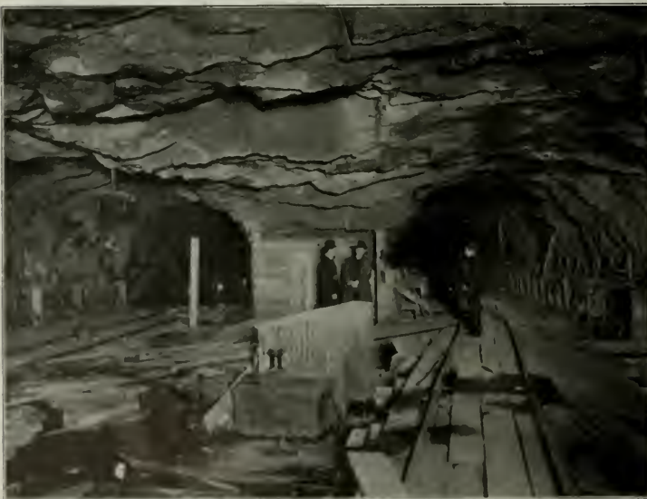
Fig. 5 View in Tunnel near East River Shaft Showing Central Rock Wall.
