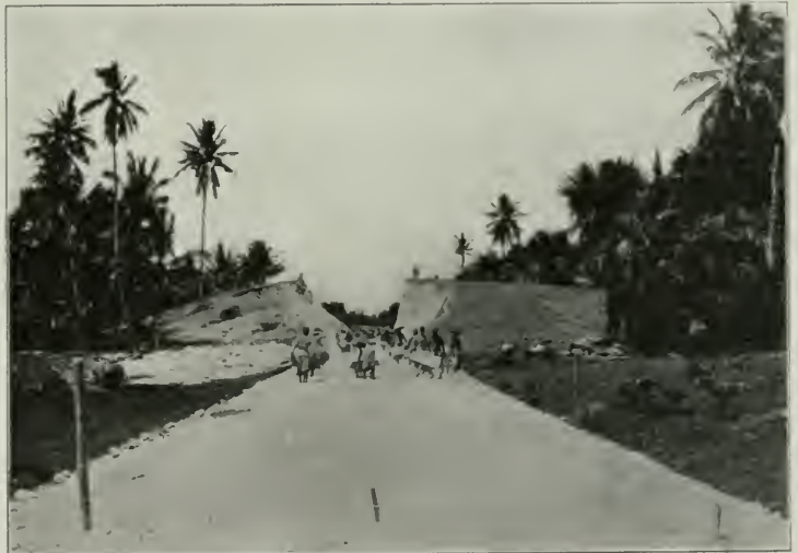
Finishing a Cut and Fill to Standard Width of 15 Feet.
