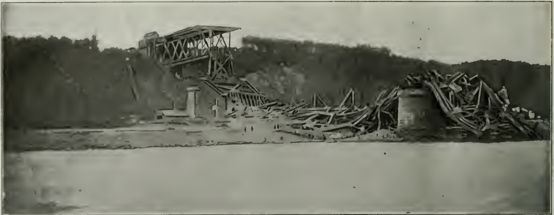
View of the Wreckage from the River, Showing Approach Span Left Standing.
