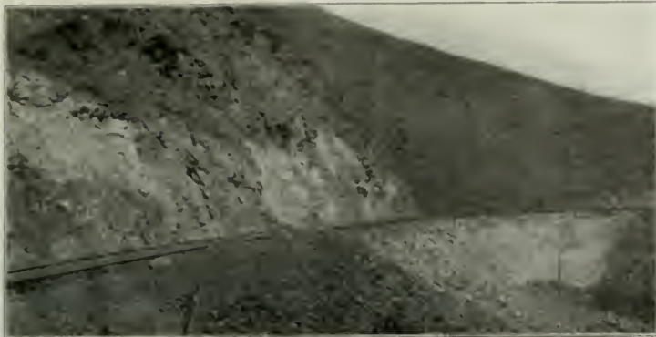
Mountain Construction, Showing Riprap Work.
