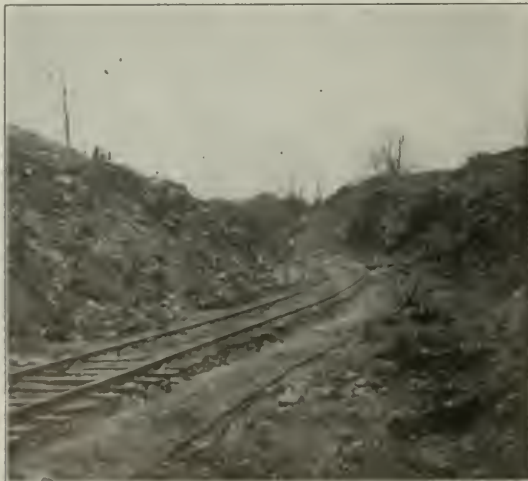
Big Cut, Where the Most Serious Sliding Occurred.
