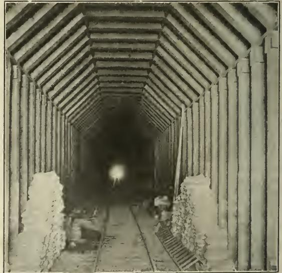
Interior of a Timber Lined Tunnel
