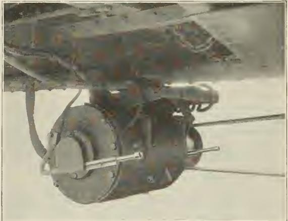
Generator with Thermometers Applied to Bearings
