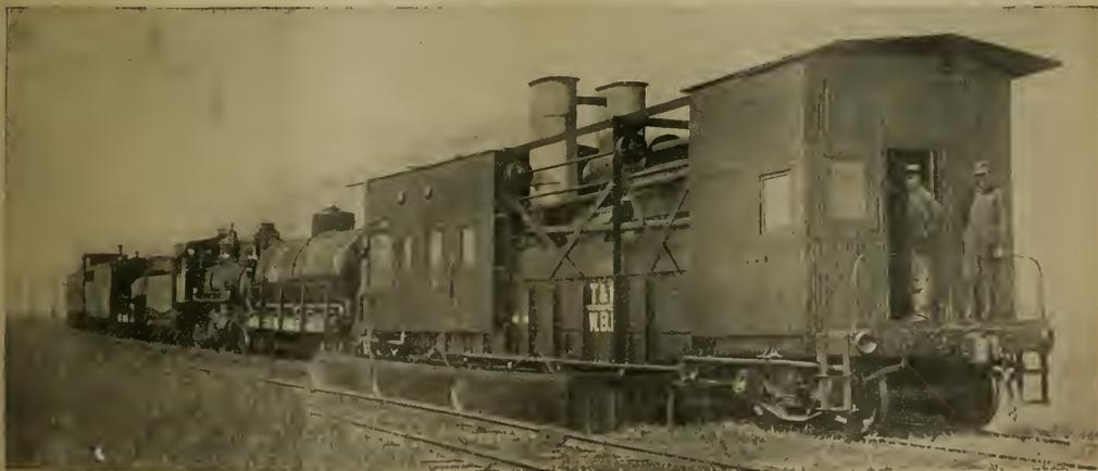
The Weed Burning Outfit Complete with Burner in the Foreground, Followed by Tank Cars, Locomotive, etc.
