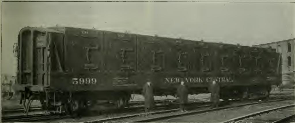
New York Central Container Car Designed for Handling Express Matter, Equipped with Passenger Trucks and Buffers and with Air, Steam, and Signal Line for Passenger Train Operation
