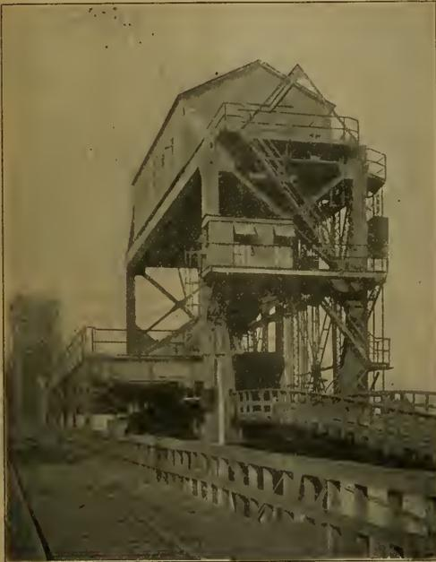
**There Are Two Car Dumping Machines at Sewalls Point Pier. This Tandem Dumper Handles in One Operation Two 55-Ton Cars or One 120-Ton Car**
