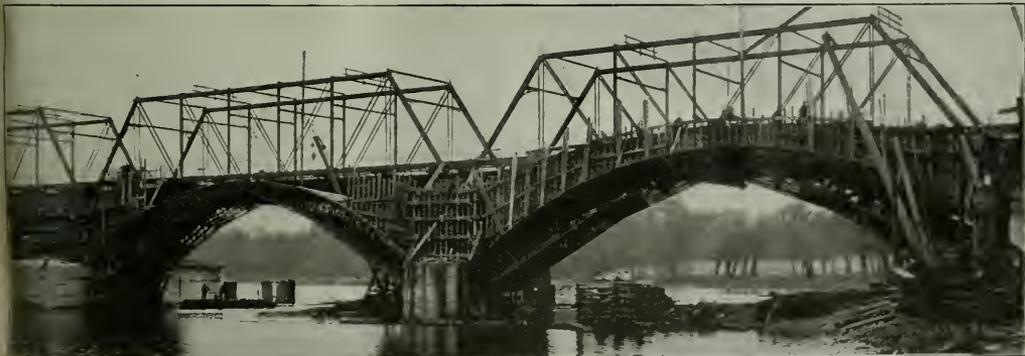
Turning Two Arches at One Time with Steel Centering
