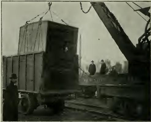
Loaded Container Being Lifted from Motor Truck
