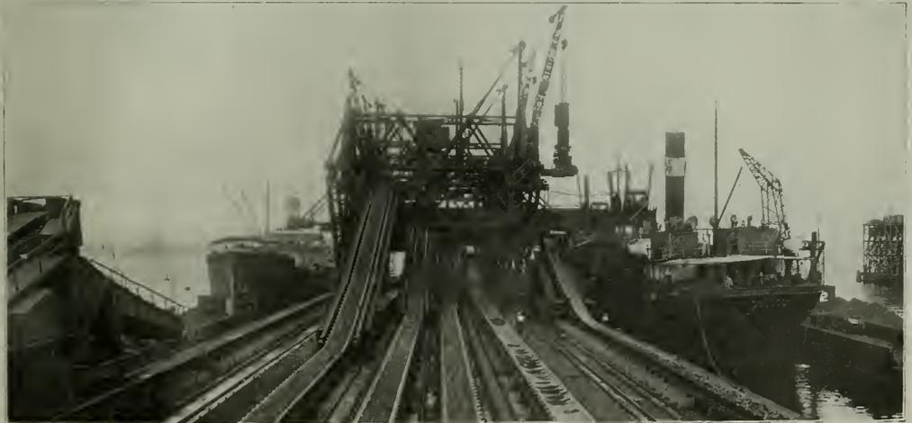
A View of the Pier, with Three of the Six Belts in Operation
