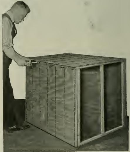
Using a Twister to Close and Seal a "Four-One" Box
