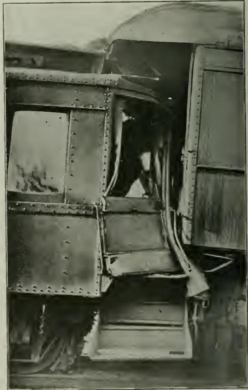
First Stage of Telescoping of Steel Cars
