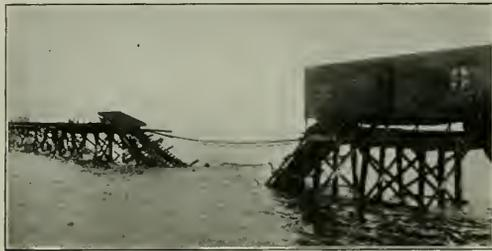
Dock at Oleum, Calif., Which Failed in 1919 and Plunged Several Cars into the Bay
