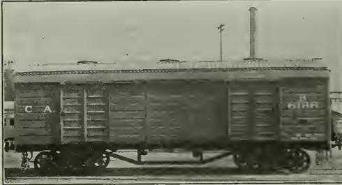
A Pressed Steel Grain Car on the Central Argentine—
