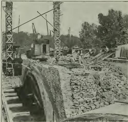
Constructing the Masonry Wall to Retain the Stone Packing
