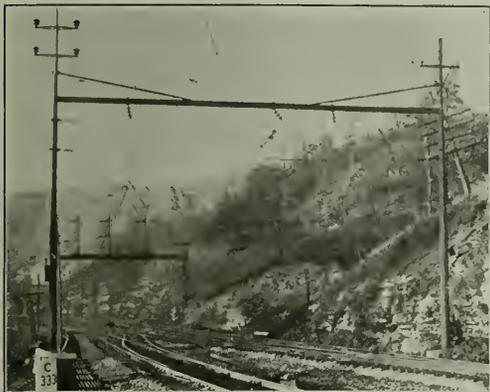
Typical Overhead Construction on the Norfolk & Western
