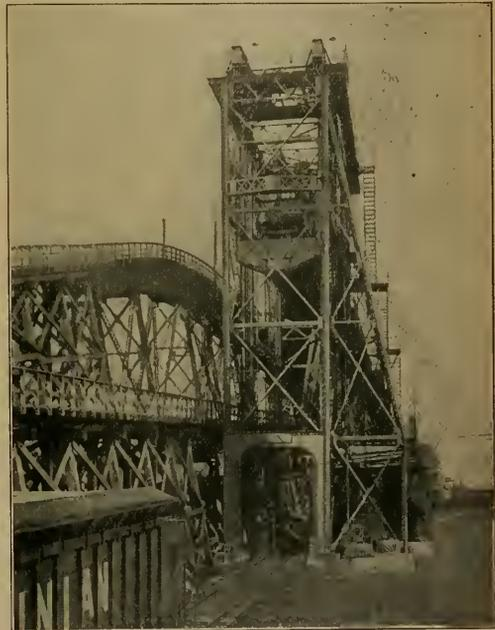
**The Elevator Which Carries the Heavy 120-Ton Tractor Cars to the Top of the Pier. The Inclined Track to the Left Is the Barney Incline Used by the 60-Ton Tractor Cars; the Center Track Is That by Which the Tractor Cars Return to the Foot of the Pier**
