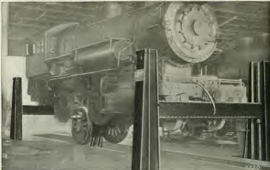
*Whiting Four-Jack Locomotive Hoist, Capacity 200 tons. View shows hoist in operation removing a single pair of drivers. In shops of Baltimore & Ohio R. R., Garrett, Ind.*
