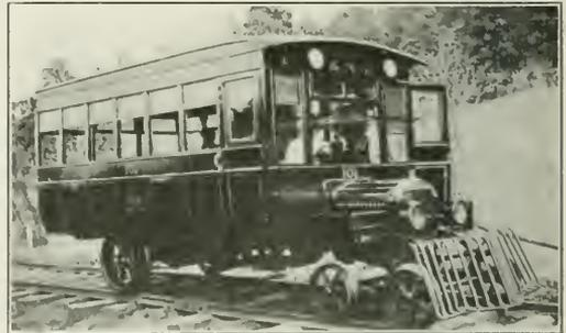
Gasoline Motor Car, in Service Since 1919 on the T. K. & N.
