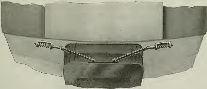
Outside Connected Top Diaphragm Buffing Mechanism
