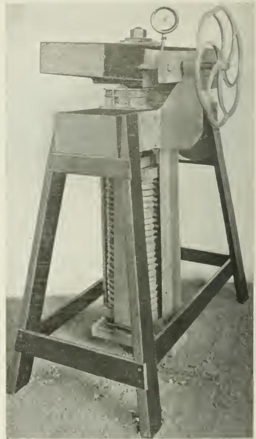
Machine for Determining The Frictional Resistance of Truck Side Bearings
