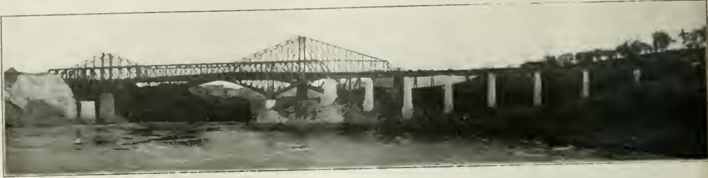
The New Bridge Is Flanked on the West by a Viaduct of Eight Deck Girder Spans
