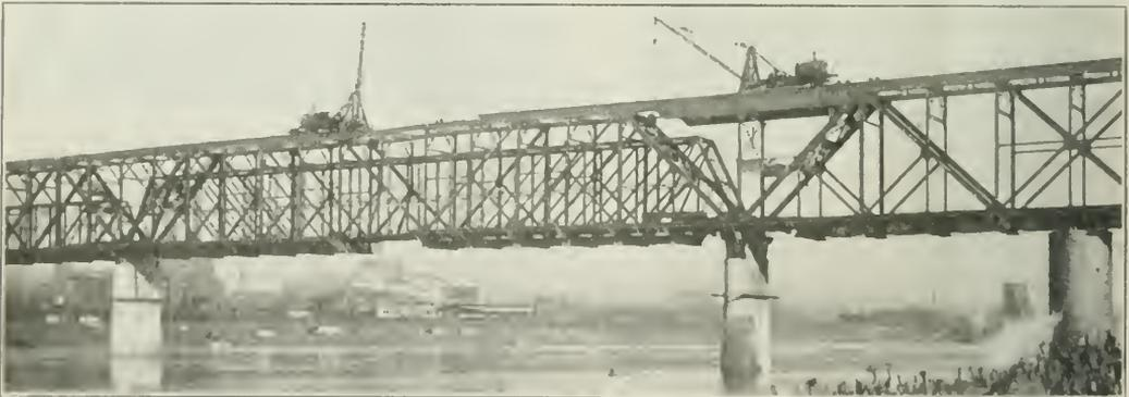
Closing the Gap in Span 3—Note the Kinks in the Bottom and Top Chords at the Ends of the Closing Panel
