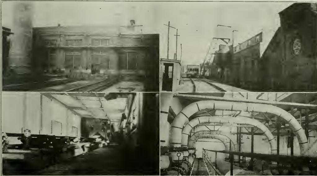
Above—Two Exterior Views of the Power Plant. Lower Left—Belt Conveyor for the Coal Handling Equipment. Lower Right—View Above the Boilers Showing the Steam Headers
