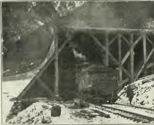
The Snow Sheds Are Built Primarily for Protection from Slides
