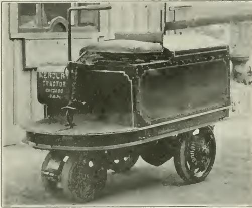
Fig. 1—Mercury Type L Tractor with Twin-3 Steering Arrangement
