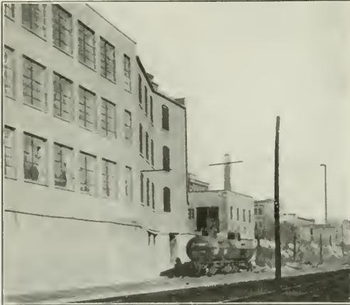
Industrial Building Underpinned by a Retaining Wall. Service Track Provided on the Depressed Level
