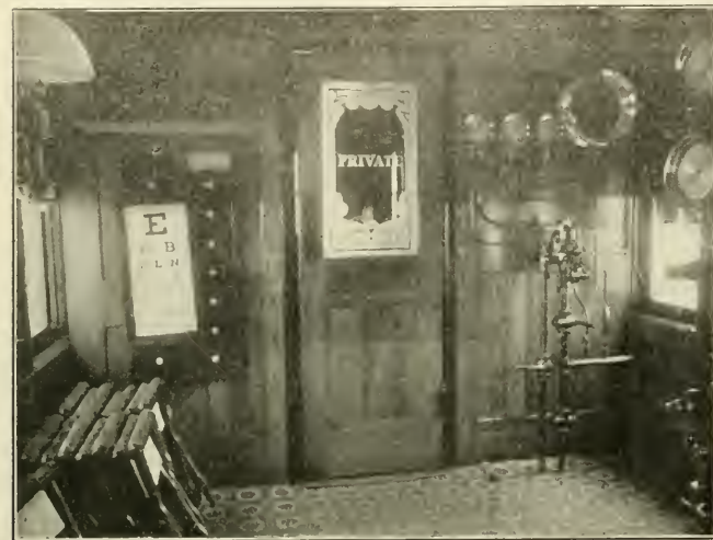
Fig 3—TEXAS & PACIFIC RAILWAY AND INTERNATIONAL & GREAT NORTHERN R. R. AIR-BRAKE INSTRUCTION CAR—VIEW SHOWING BRAKE VALVE AND GAGES.
