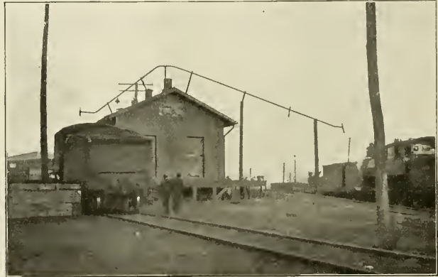
SAND HOUSE AND CONVEYING PIPES AT THE 8TH STREET ROUNDOUSE OF BALTIMORE & OHIO R.R., PHILADELPHIA, PA.
