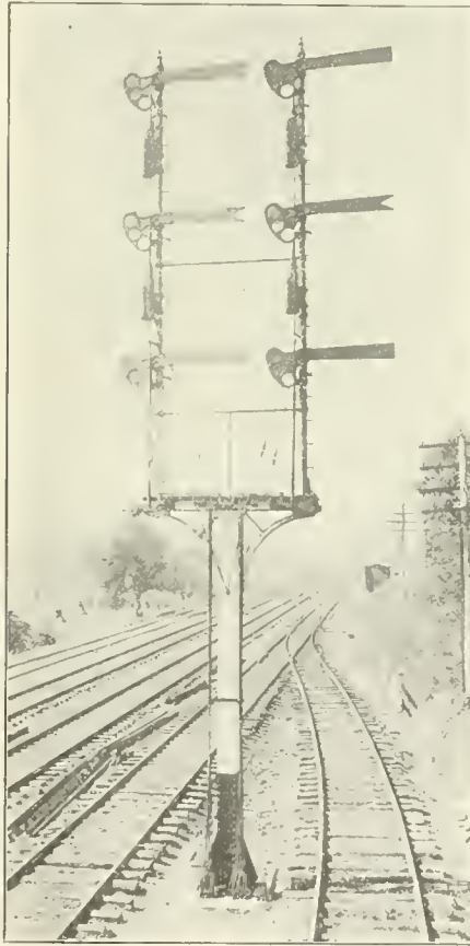
SINGLE POST WITH AUTOMATIC AND INTERLOCKING SIGNALS.
