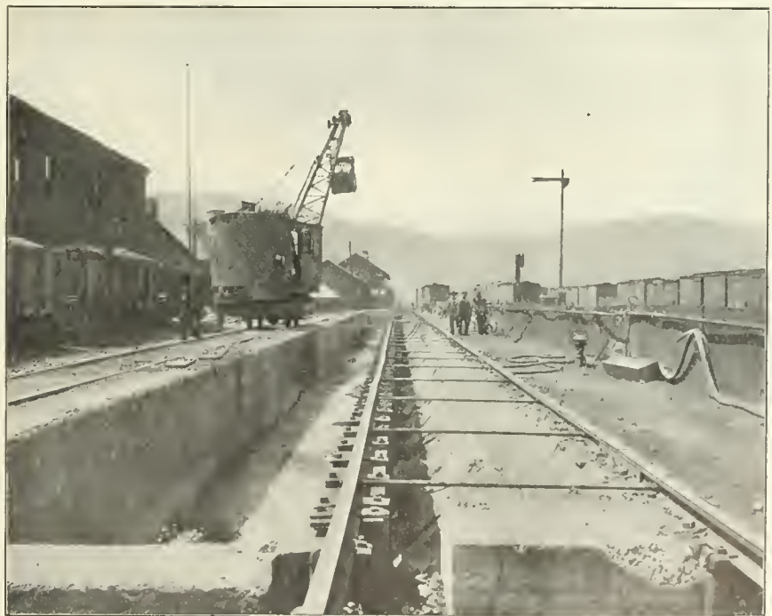
ERIE CINDER PIT SHOWING INCLINED WALL UNDER TRACK.
