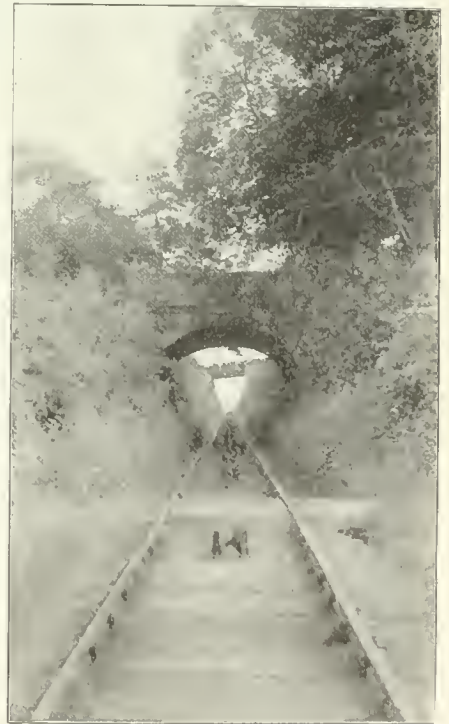
SWANNINGTON INCLINE, LEICESTER & SWANNINGTON RAILWAY, ENGLAND. GRADE 1 IN 17; PULLEYS FOR ROPE IN CENTRE OF TRACK.
