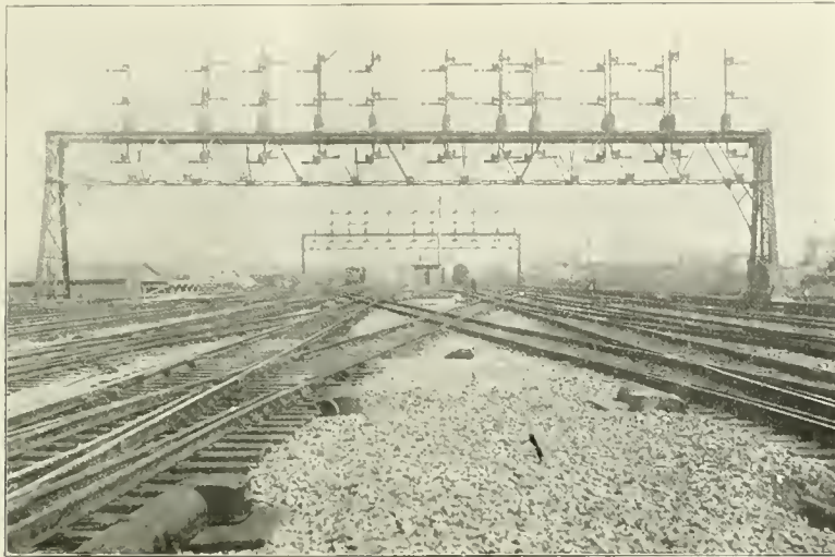
LOOKING NORTH TOWARD NEW YORK AVENUE, SIGNAL BRIDGE K IN THE FOREGROUND.
