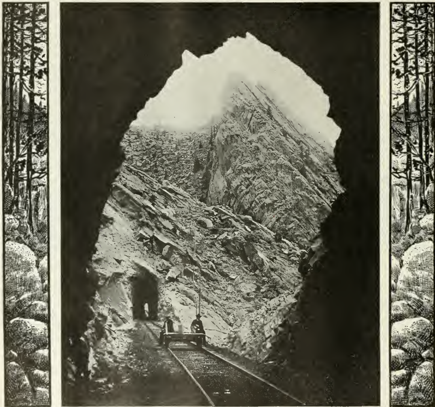
VIEW FROM ONE OF THE MANY SHORT TUNNELS ON THE DENVER, NORTH-WESTERN & PACIFIC.
