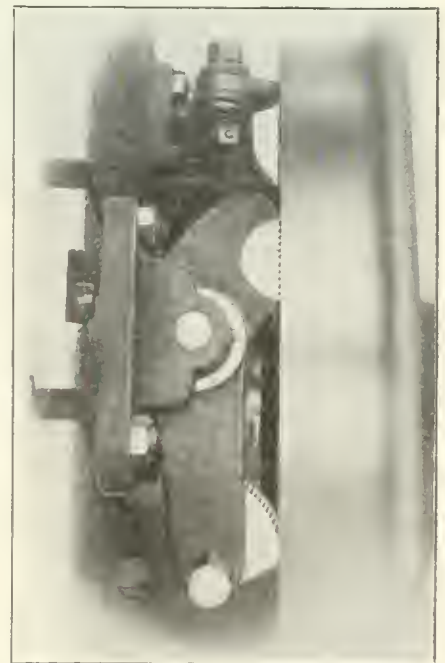
SELLERS WHEEL GRIP AND DRIVE FOR CAR WHEEL LATHE.
