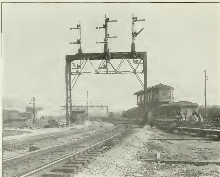
LOOKING NORTH, FOOT OF K STREET, INTERLOCKING SIGNALS.
