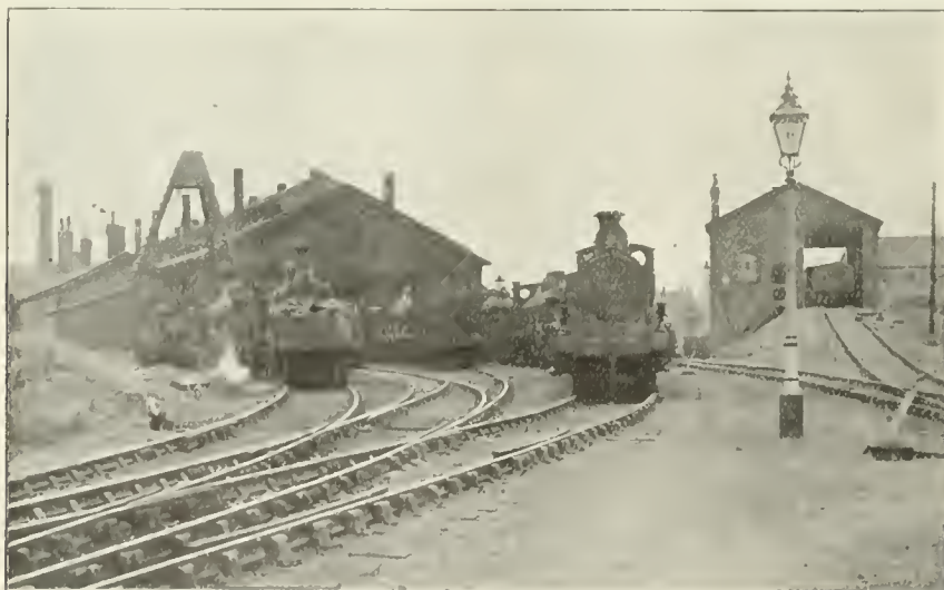
COALVILLE ENGINE HOUSE, MIDLAND RAILWAY, ENGLAND.
