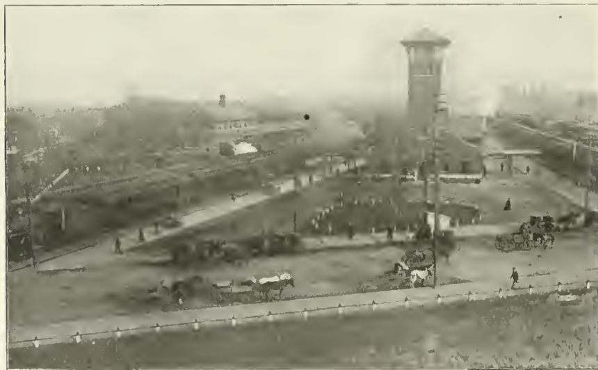
UNION STATION AT FREMONT, NEB., C. & N. W. AND U. P. TRACKS.
