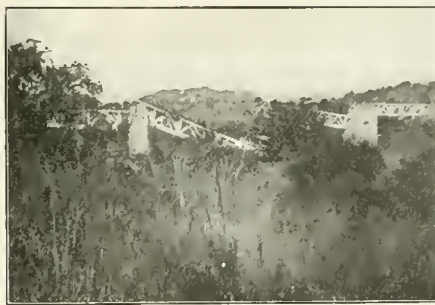
BRIDGE GIRDER DOWN.
