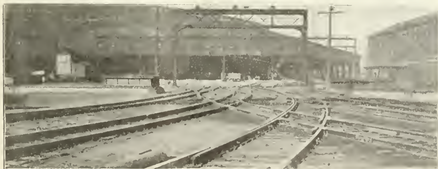
LOOKING NORTH TOWARD TRAIN SHED, EAST SIDE, ST. LOUIS TERMINAL.
