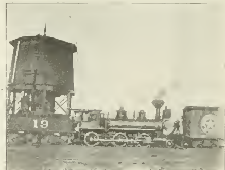
AT THE WATER TANK.
