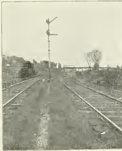
UPPER QUADRANT, THREE POSITION SIGNAL.
