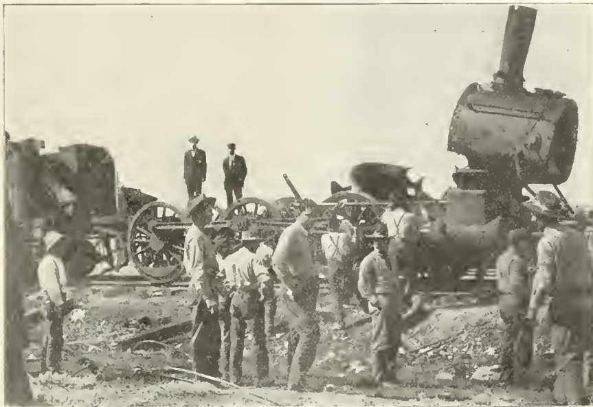
ENGINE STANDING ON TRACK WITH BOILER BLOWN AWAY.
