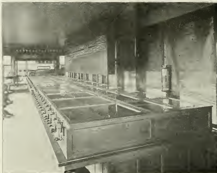
ILLUMINATED TRACK MODEL IN K STREET TOWER.
