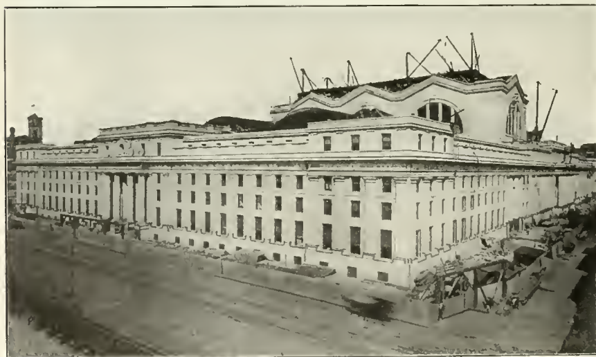
EIGHTH AVE. FACADE, NEW PENNSYLVANIA RD. STATION IN NEW YORK.
