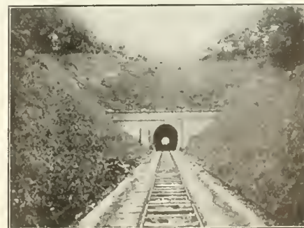
KONAKASHIMA TUNNEL, JAPAN.
