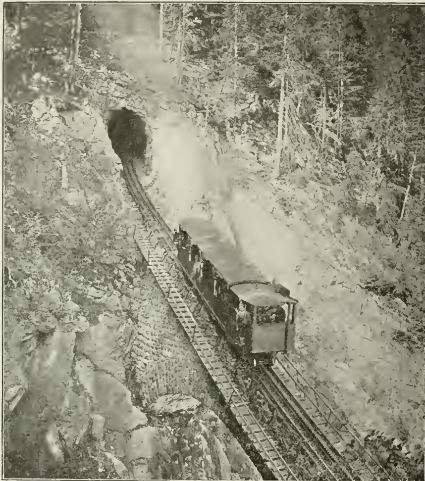
BRIDGE AND TUNNEL ON THE HEAVY CLIMB.
