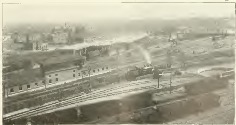
K STREET SIGNAL TOWER AND ELECTRIC PLANT.
