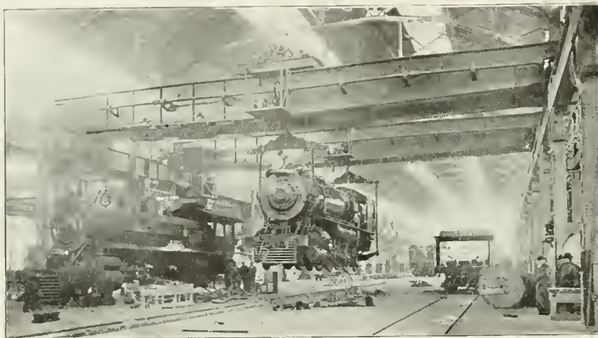
CRANE IN THE SANTA FE SHOPS. MADE BY THE WHITING FOUNDRY EQUIPMENT COMPANY, OF HARVEY, ILL.
