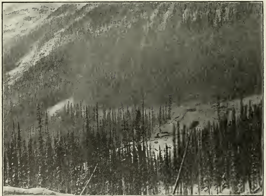
PORTAL OF SPIRAL TUNNEL NEAR THE KICKING HORSE RIVER.
