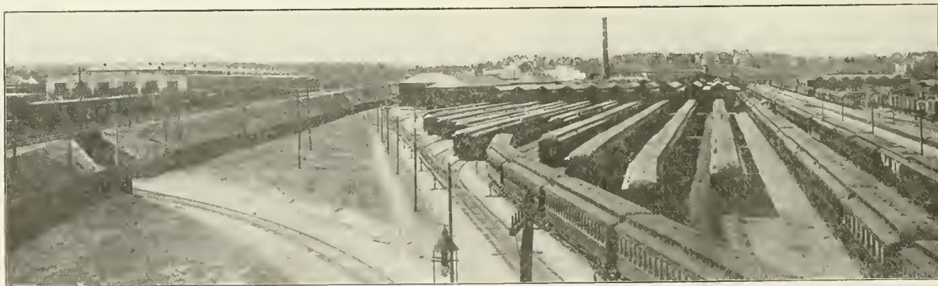
VIEW OF THE READVILLE SHOPS OF THE NEW YORK, NEW HAVEN & HARTFORD RAILROAD.
