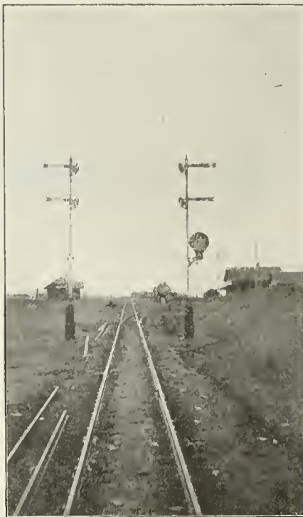
U. P. SIGNALS DOUBLE LOCATION NEAR SHERMAN, WYO. BANJO SIGNAL INDICATES DIVERGING ROUTE.
