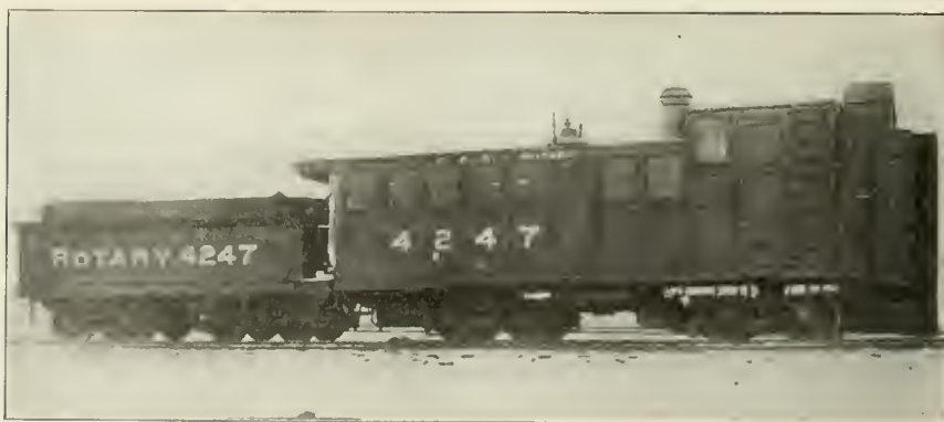
PREPARING FOR THE WINTY BLASTS. THE ROTARY.
