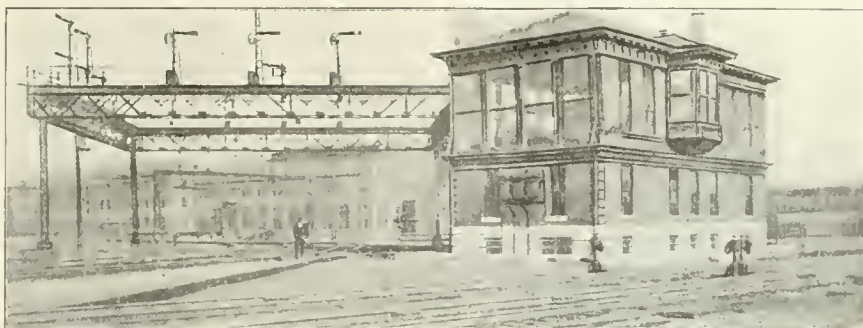
INTERLOCKING TOWER AT ENTRANCE TO ST. LOUIS TERMINAL.
