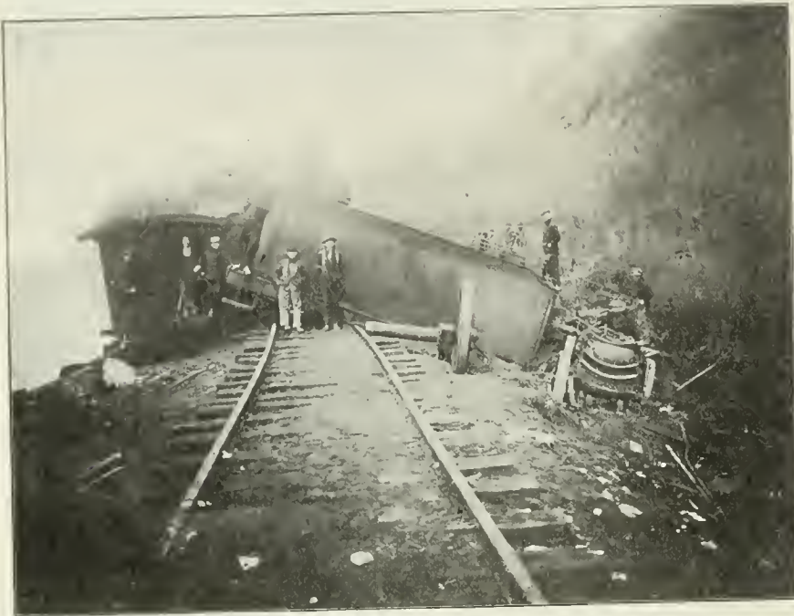
ROAD BLOCKED WITH DEBRIS FROM EXPLOSION.
