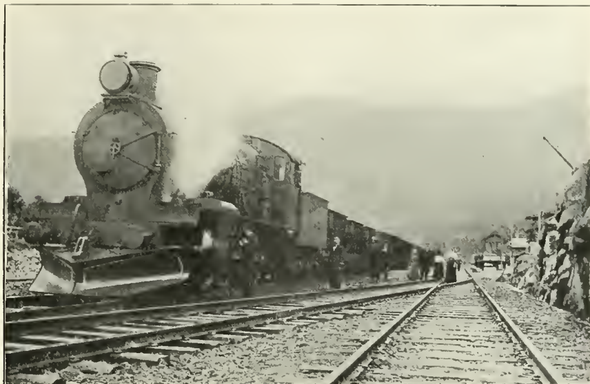
ORE TRAIN AT NARVIC STATION, OFOTEN RAILWAY.
