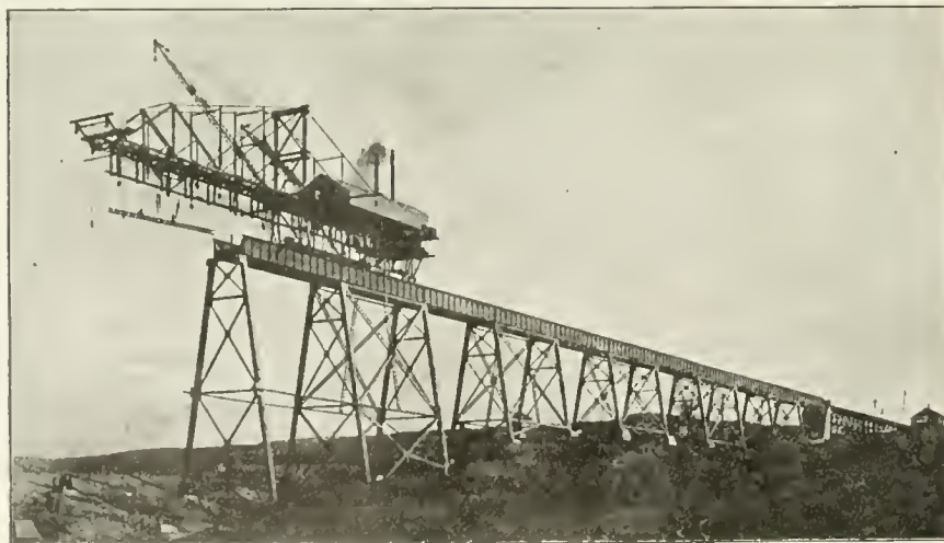
SIDE VIEW OF LETHBRIDGE VIADUCT ON THE C. P. R.
