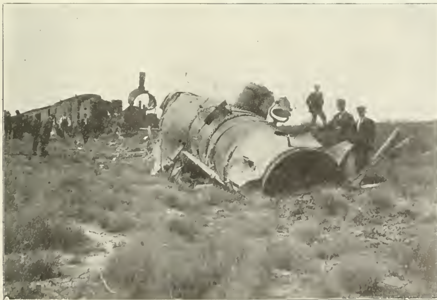
EXPLODED BOILER LYING ON THE PRAIRIE AWAY TO ONE SIDE OF TRACK.
