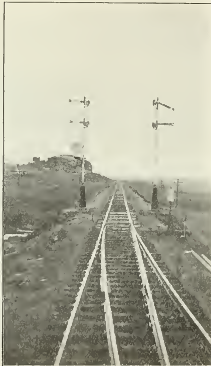
UNION PACIFIC SIGNALS AT DALE CREEK, WYO. EXAMPLE OF DOUBLE LOCATION.
