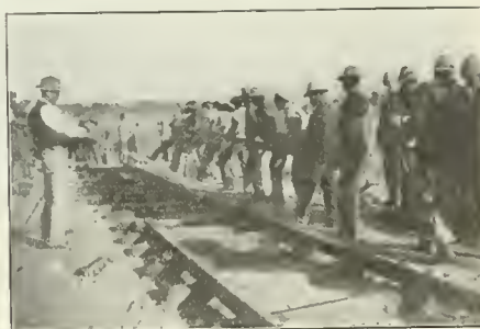
TRACK LAYING IN SOUTH AFRICA.
