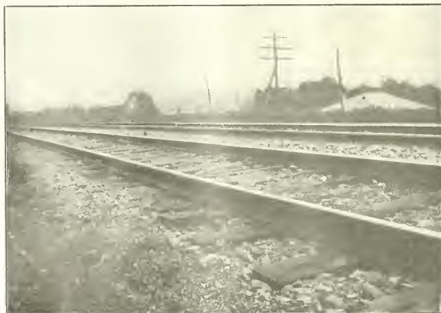
STANDARD ROCK BALLAST TRACK, C. & O.
