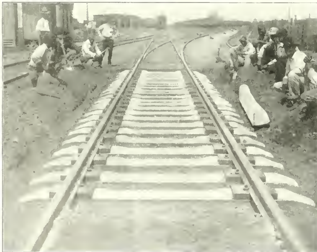
RAILROAD TRACK Laid WITH PERCIVAL CONCRETE TIES.
