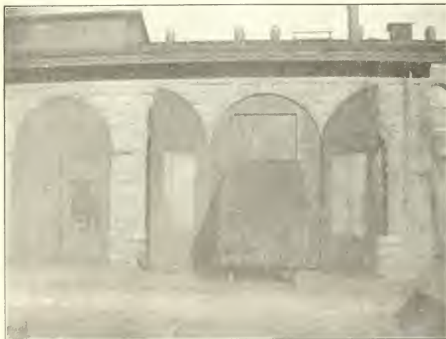
FIG. 2. STORM DOOR ON WHEELS WITH CAVITY FOR FLUES.
