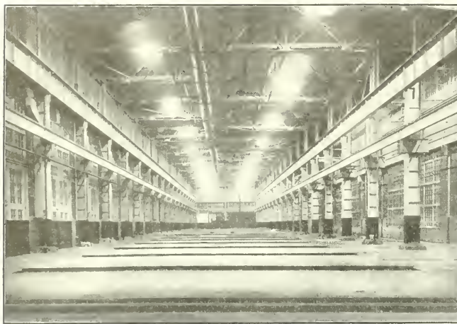
FIGURE 1. ERECTING SHOP LIGHTED BY COOPER HEWITT LAMPS.
