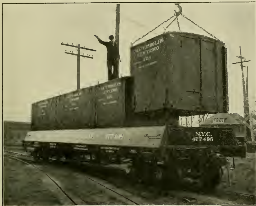
UNLOADING A CONTAINER FROM THE FREIGHT TYPE OF CONTAINER CAR
