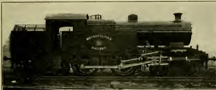
4-4-4 TYPE LOCOMOTIVE FOR THE METROPOLITAN RAILWAY OF LONDON, ENGLAND.
