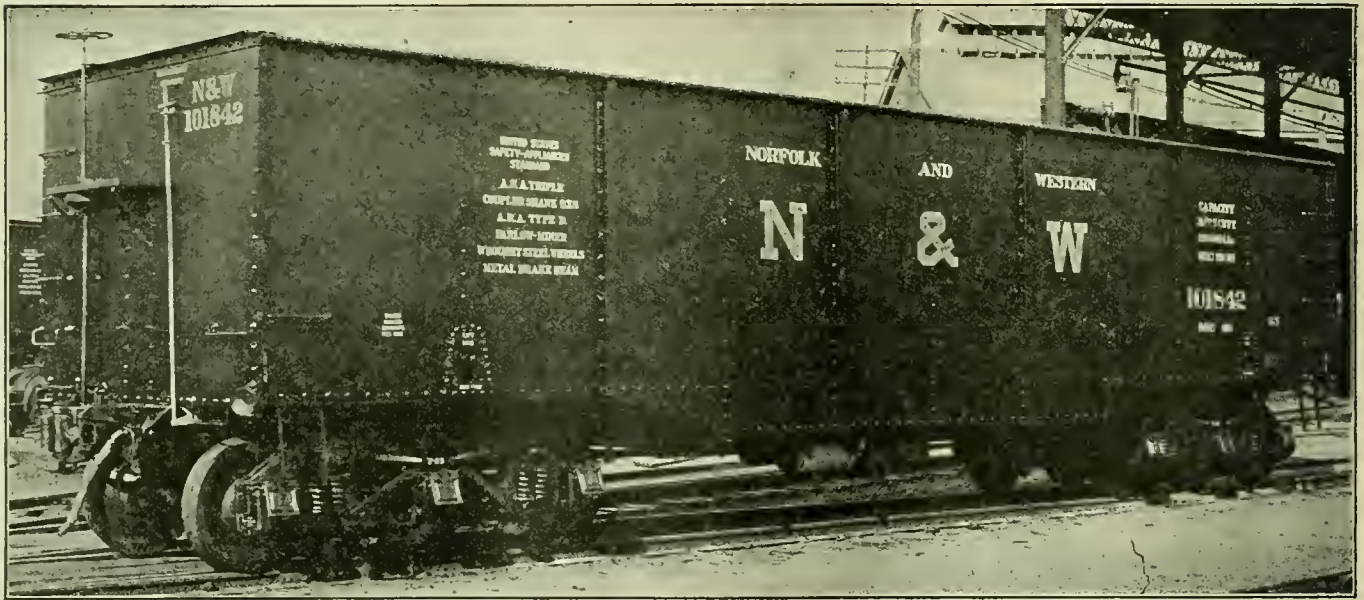
ONE-HUNDRED-TON CAPACITY COAL CAR OF NORFOLK & WESTERN R. R. EQUIPPED WITH AUTOMATIC STRAIGHT AIR BRAKES AND N. & W. SIX-WHEELED TRUCKS
