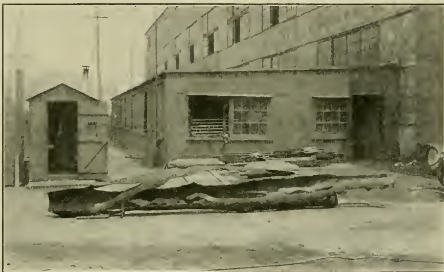
VIEW SHOWING RESULTS OF EXPLOSION IN COMPRESSED AIR LINE
