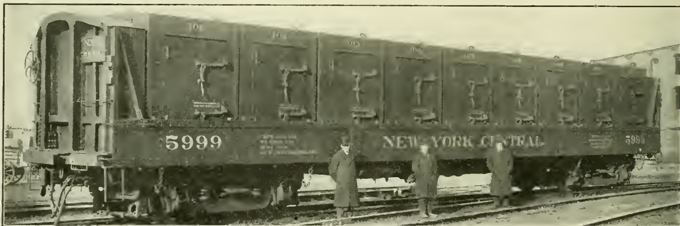
THE EXPRESS-TYPE CONTAINER WITH THE CONTAINERS IN PLACE. THE STEEL SIDES OF THE CAR PREVENT THE DOORS OF THE CONTAINER FROM BEING OPENED
