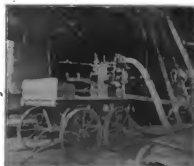
PORTABLE BOILER TESTER.
