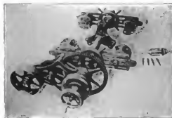
Portable Cylinder Boring Bar and Fixtures.
