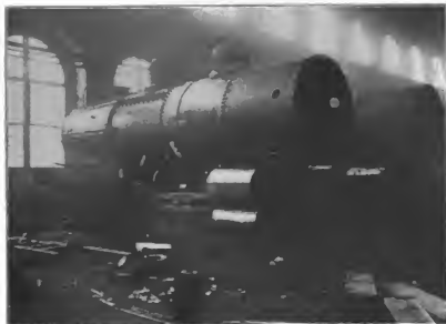
FIG. 5. FASTENING THE BOILER.
