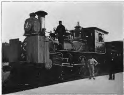
TESTING SLIP OF DRIVING WHEELS.
