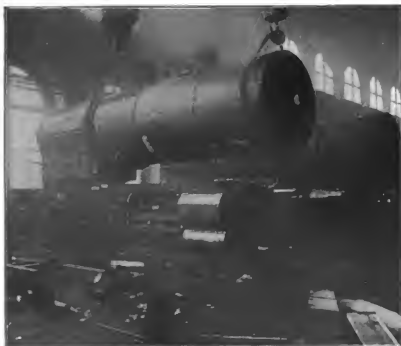
FIG. 4. PUTTING BOILER IN PLACE.
