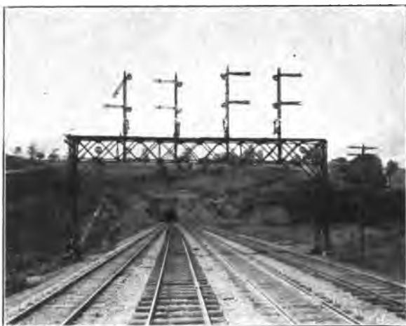
A typical signal bridge.
