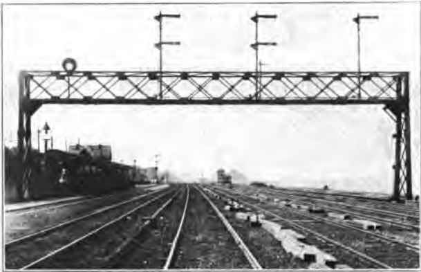
Mechanically interlocked home semaphore signals and a disc signal on a signal bridge. Semaphores in "Stop" position. Disc signal seen from rear.
