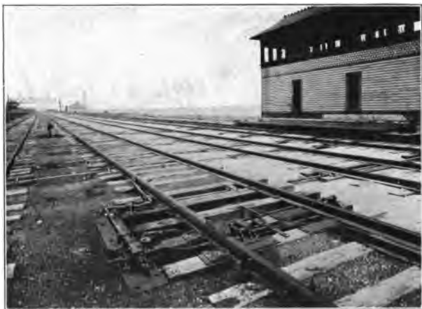
An interlocking derail, showing a switch and lock movement.
