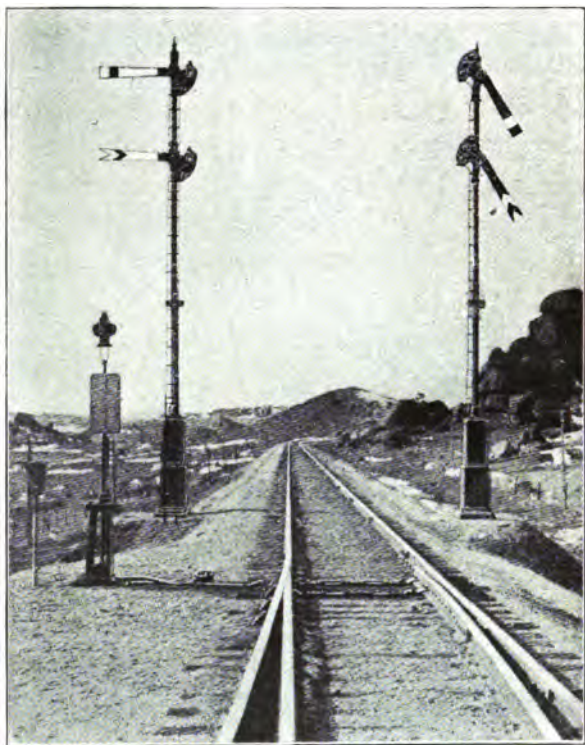
A double automatic signal location on single track.
