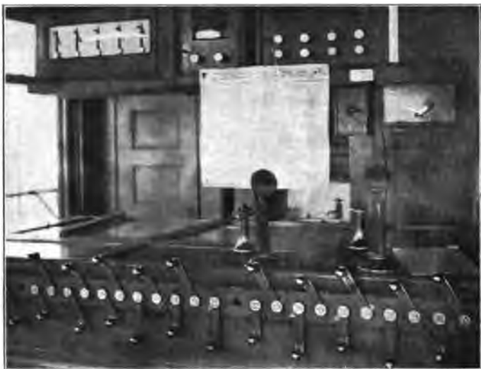
Section of electro-pneumatic interlocking machine, showing also indicators and train announcing devices.
