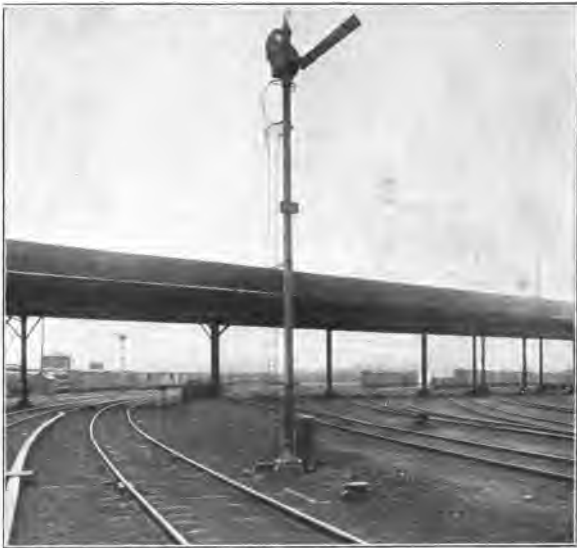
Upper quadrant signal indicating "Proceed at limited speed".
