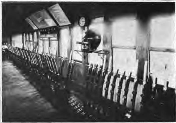
Interior of tower, showing levers and indicators. The interlocking machine is of the vertical locking type.
