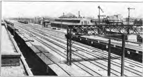
Electrically operated interlocked semaphore signals on a signal bridge. Upper blade indicates "Proceed on main line route".
