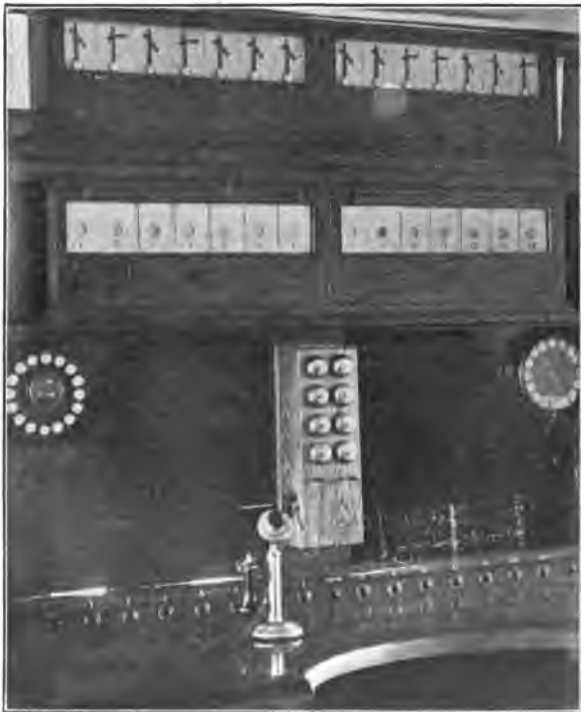
A group of indicators in a tower. By means of these indicators a tower-man is enabled to note at a glance the positions of trains on the tracks governed by his machine.
