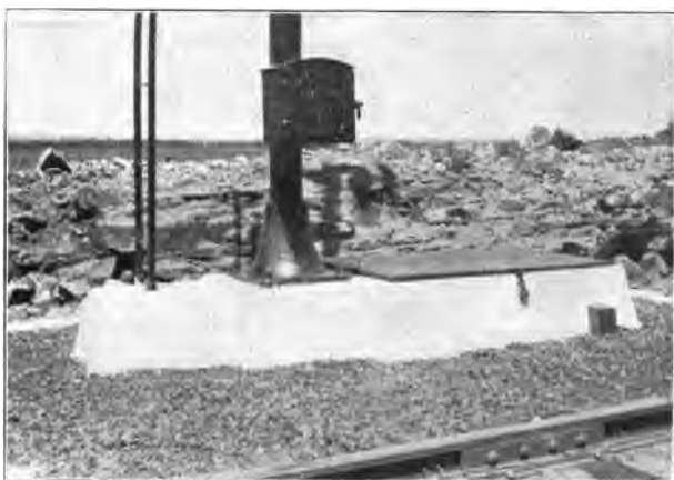
Base of an automatic block signal showing one method of constructing a foundation for the signal post. The box on the post contains the relays which govern the signal mechanism. The primary batteries which furnish current for the operation of the signal are housed in the foundation. Bond wires for the electrical connection from one rail to another may be noted in the lower right hand corner of the picture.
