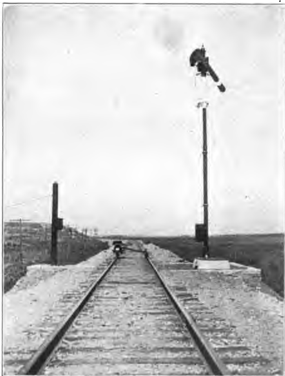
Single blade automatic block signal giving "Clear" indication. This indication is in the lower right hand quadrant.
