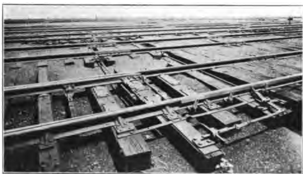
An interlocking switch, showing a facing point lock.
