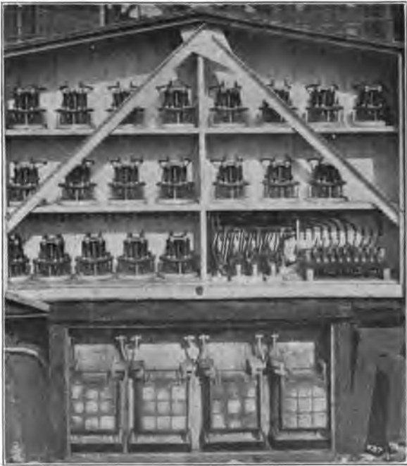
A group of relays and storage batteries governing automatic signal circuits.
