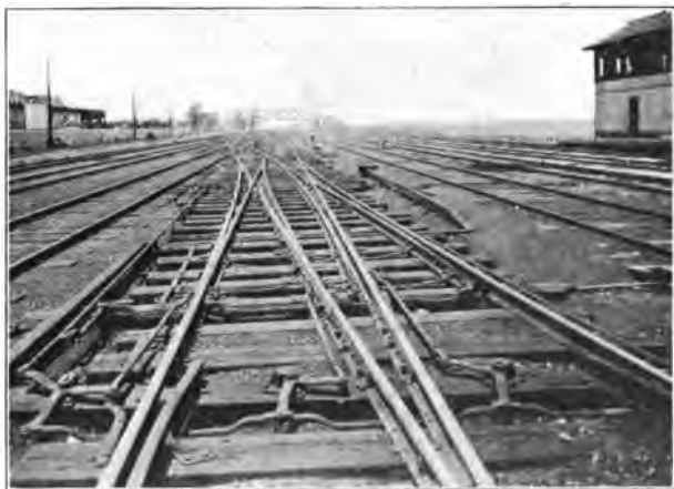
An interlocked double-slip switch.
