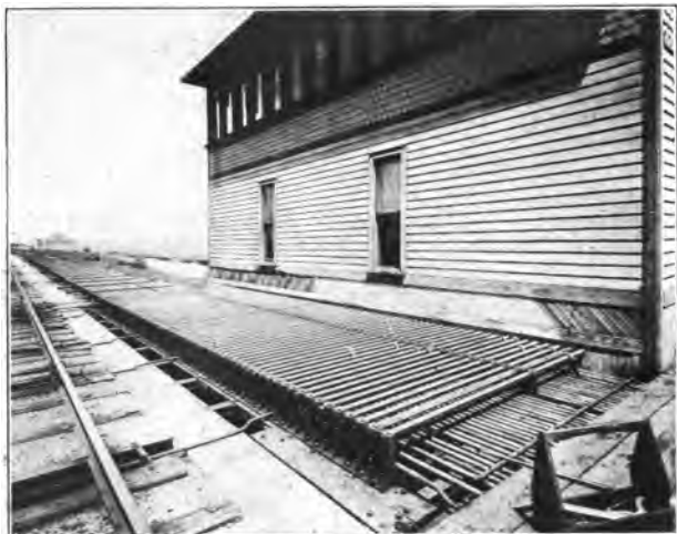
A close view of a lead-out of the rocker-shaft type.
