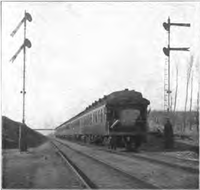
A double automatic signal location. The train on the right hand track has just entered the block, and the signals have, therefore, just assumed the "Stop" position. Signals on the left hand are indicating "Two Blocks Clear" for a train running in the direction opposite to that of the train shown.
