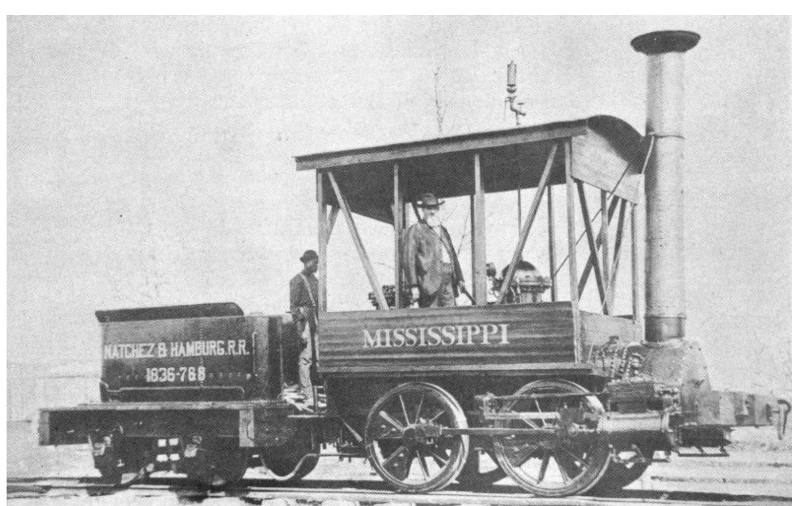
Figure 48.—Mississippi, probably built in the 1830's, with tender of a later period. Photo may have been taken after locomotive was rebuilt for exhibition at World's Columbian Exposition at Chicago, in 1893.
