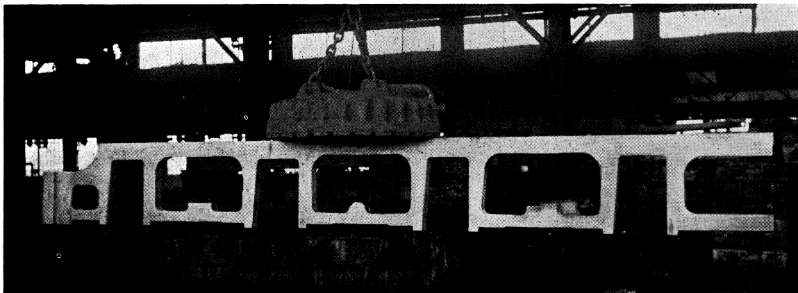
ONE OF FORTY VANADIUM CAST STEEL FRAMES FOR SOUTHERN PACIFIC MIKADOS OHIO STEEL FOUNDRY COMPANY, MAKERS
