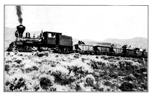
24-ton Shay Locomotive on Empire Copper Co. Railroad. This road contains 6 per cent combined with 34 degree curves.
