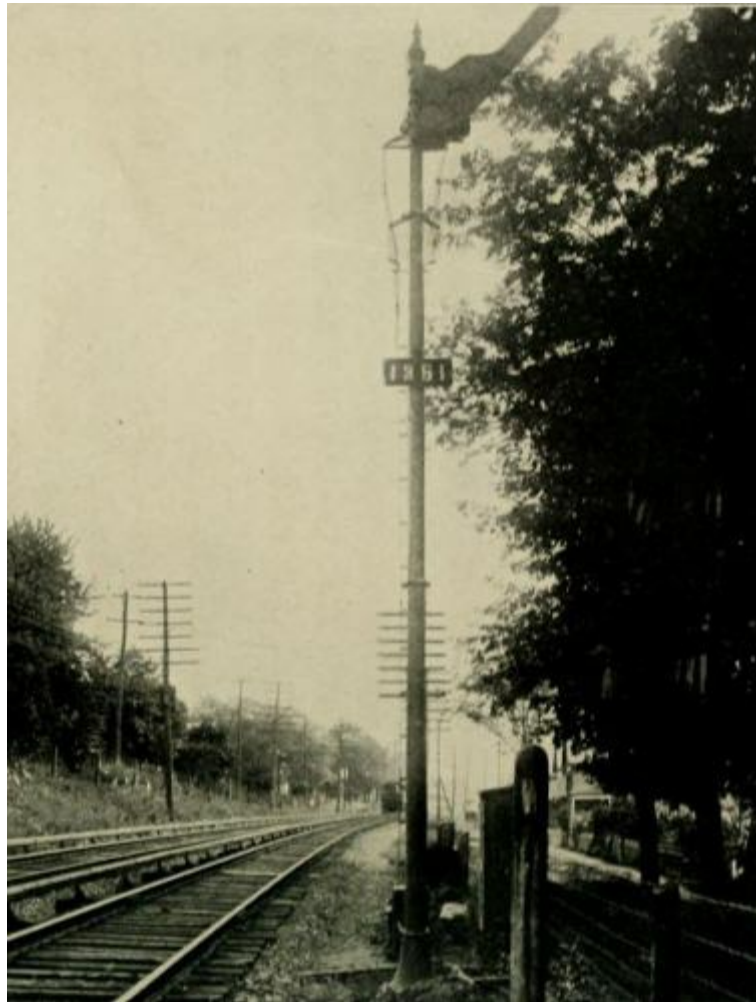
THE NEW YORK CENTRAL IS ADOPTING THE NEW FORM OF "UPPER QUADRANT" SIGNAL
