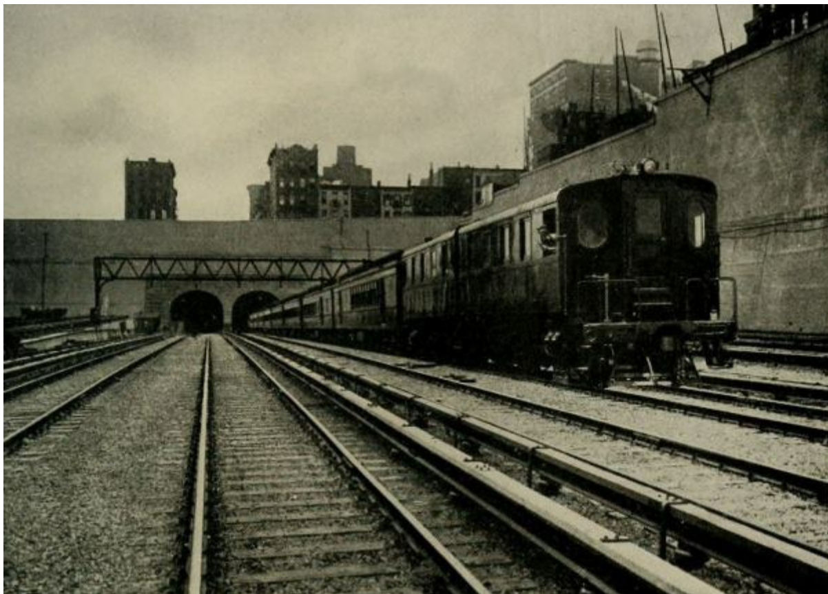
A HIGH-SPEED ELECTRIC LOCOMOTIVE ON THE PENNSYLVANIA BRINGING A THROUGH TRAIN OUT OF THE TUNNEL UNDERNEATH THE HUDSON RIVER AND INTO THE NEW YORK CITY TERMINAL
