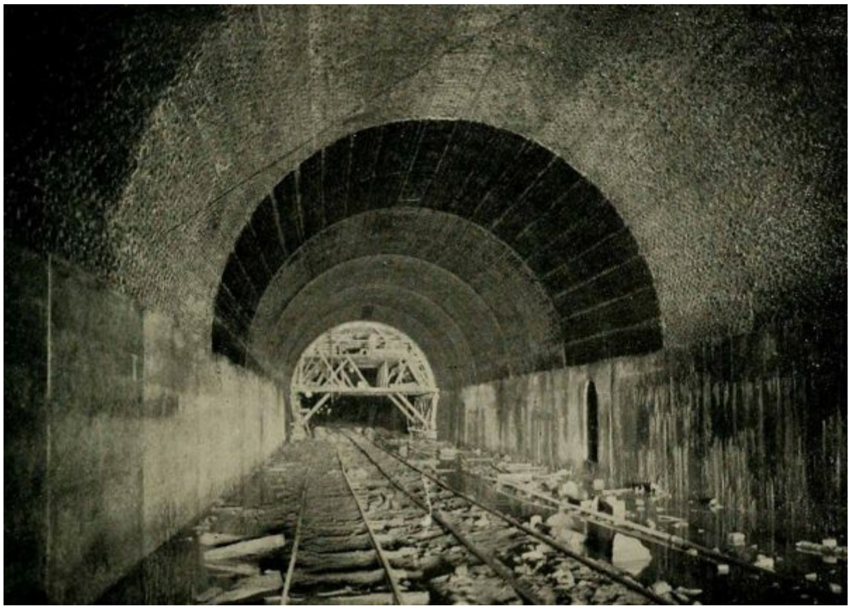
FINISHING THE LINING OF A TUNNEL
