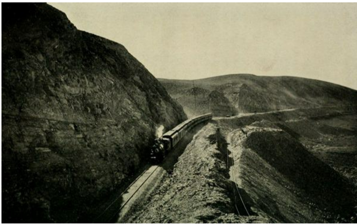
IMPRESSIVE GRADE REVISION ON THE UNION PACIFIC IN THE BLACK HILLS OF WYOMING. THE DISCARDED LINE MAY BE SEEN AT THE RIGHT
